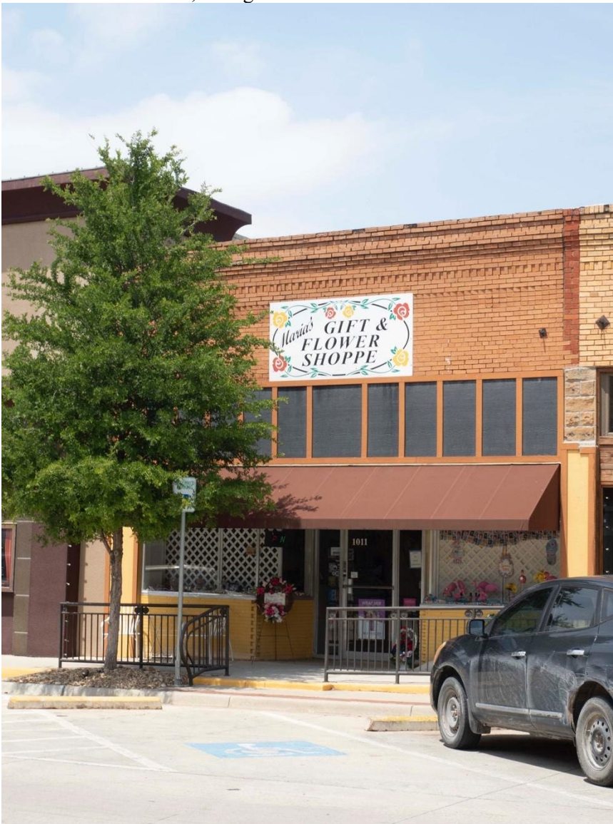
Photo 21. Resource 23, facing northwest.
