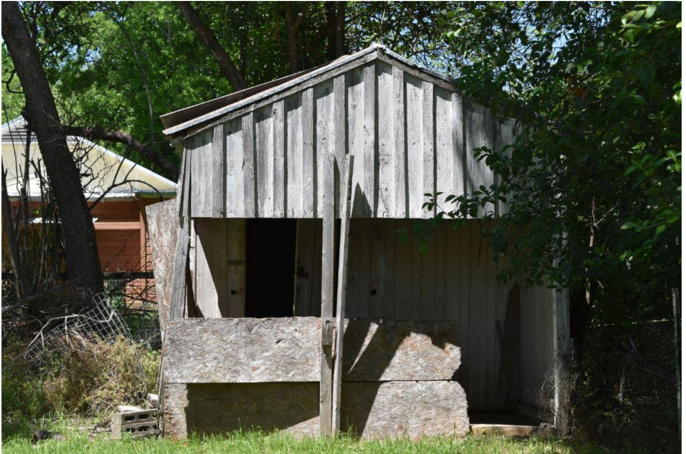
Photograph 20. A ca. 1910 outbuilding at 129 Nance Street (Map ID #12B). View looking northwest.
