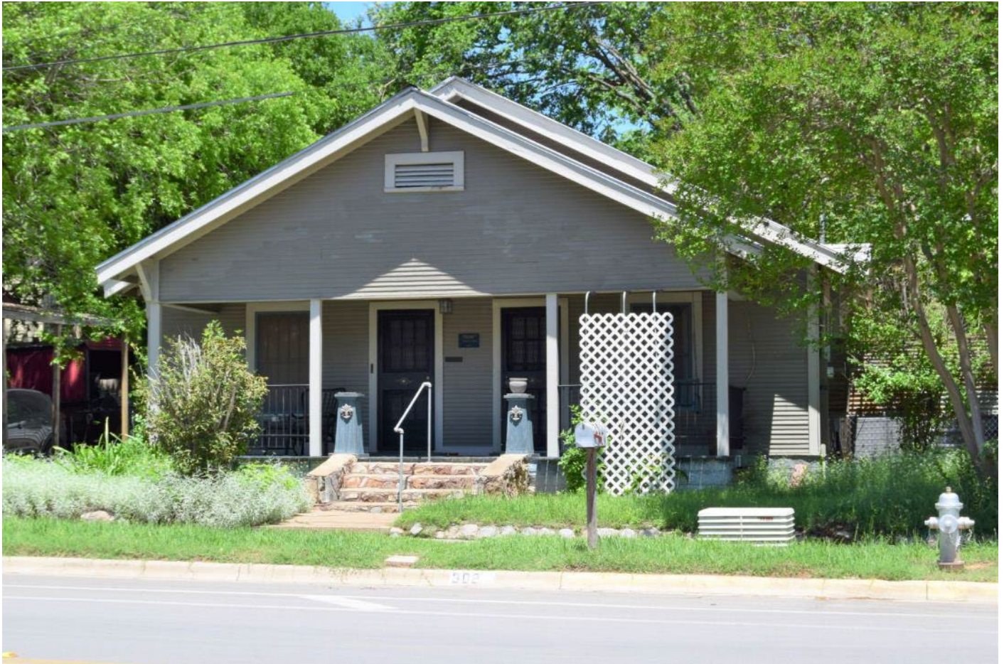
Photograph 17. A ca. 1925 bungalow-form house at 302 West Martin Luther King Drive (Map ID #18). View looking north.
