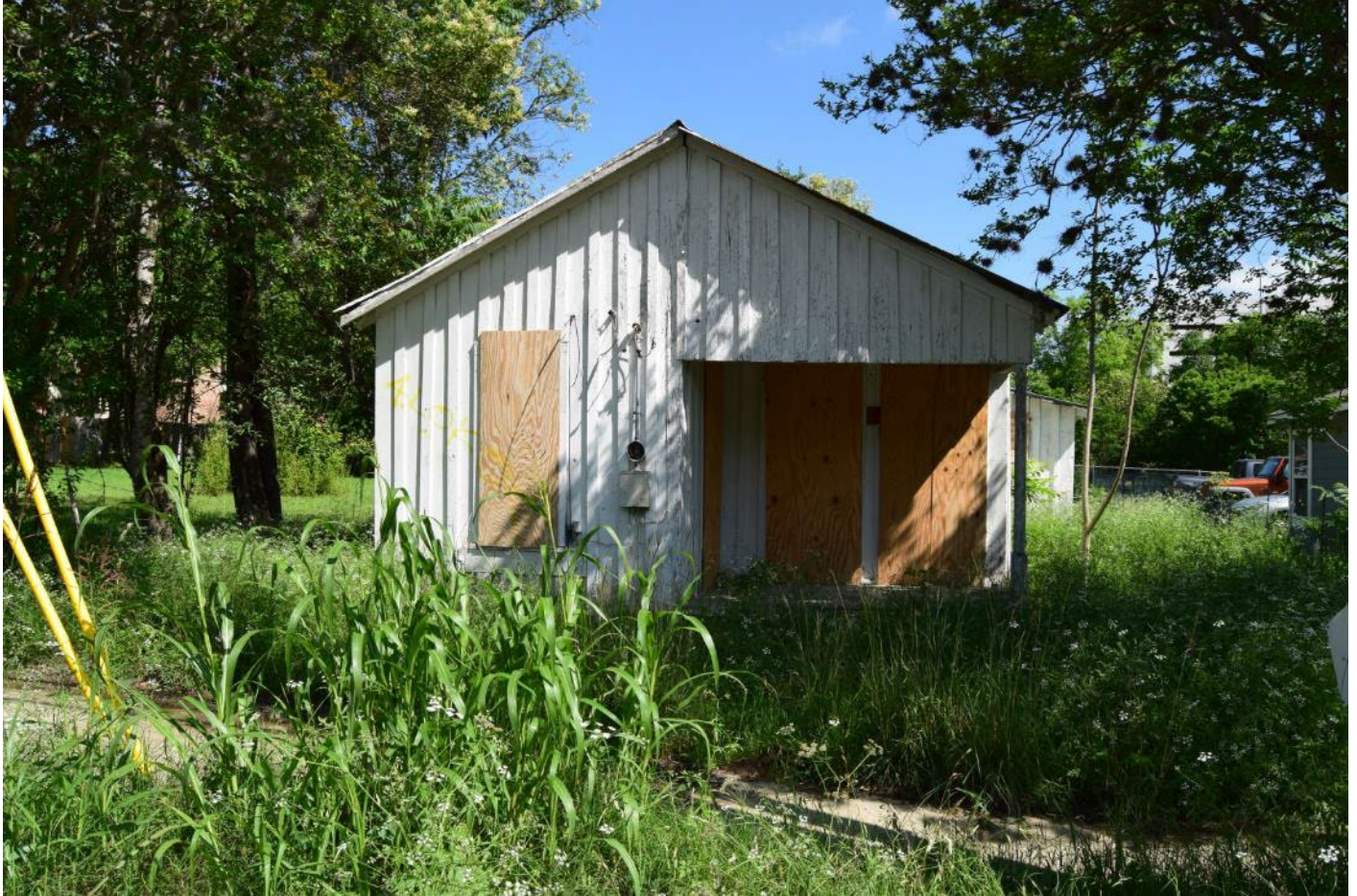
Photograph 14. A ca. 1910 National Folk-form house at 218 West Martin Luther King Drive (Map ID #25). View looking north.
