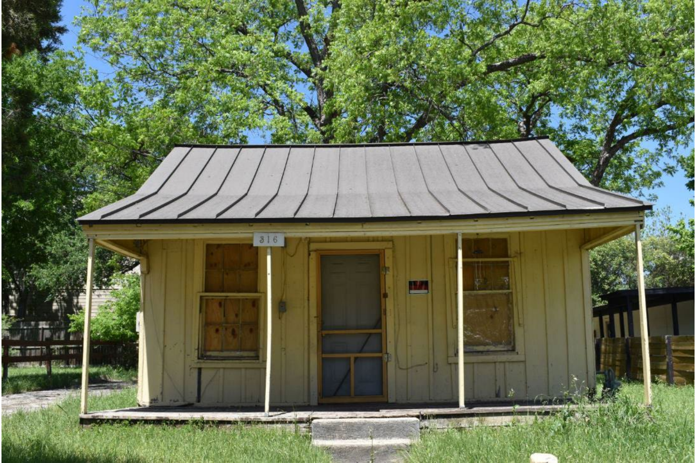
Photograph 13. A ca. 1910 National Folk-form house at 316 West Martin Luther King Drive (Map ID #14). View looking north.
