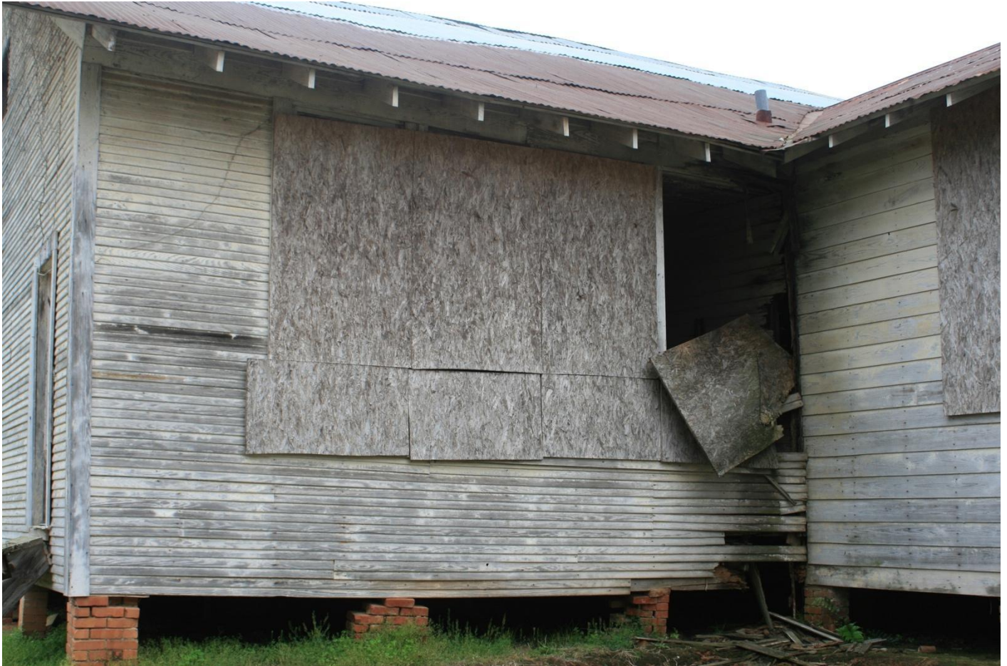
Photo 11 Northwest elevation, camera facing east.
