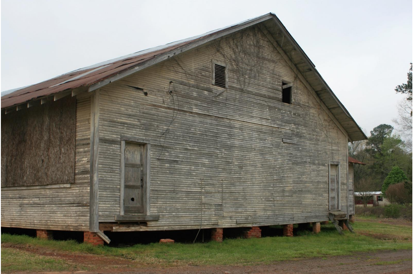
Photo 9 Northeast elevation, camera facing south.
