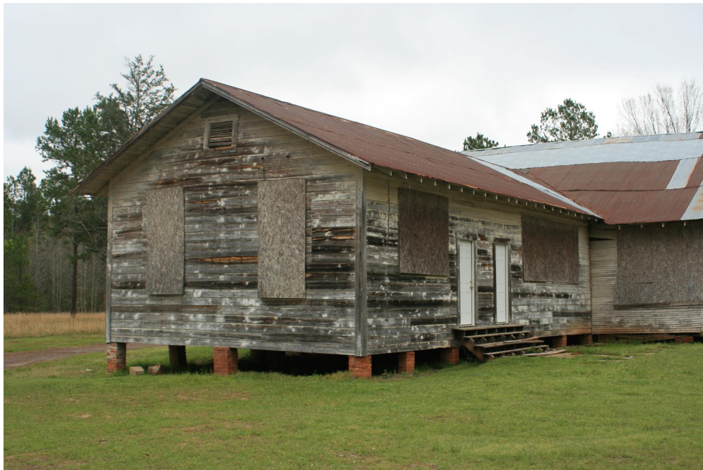
Photo 15 Southwest elevation, camera facing northeast.
