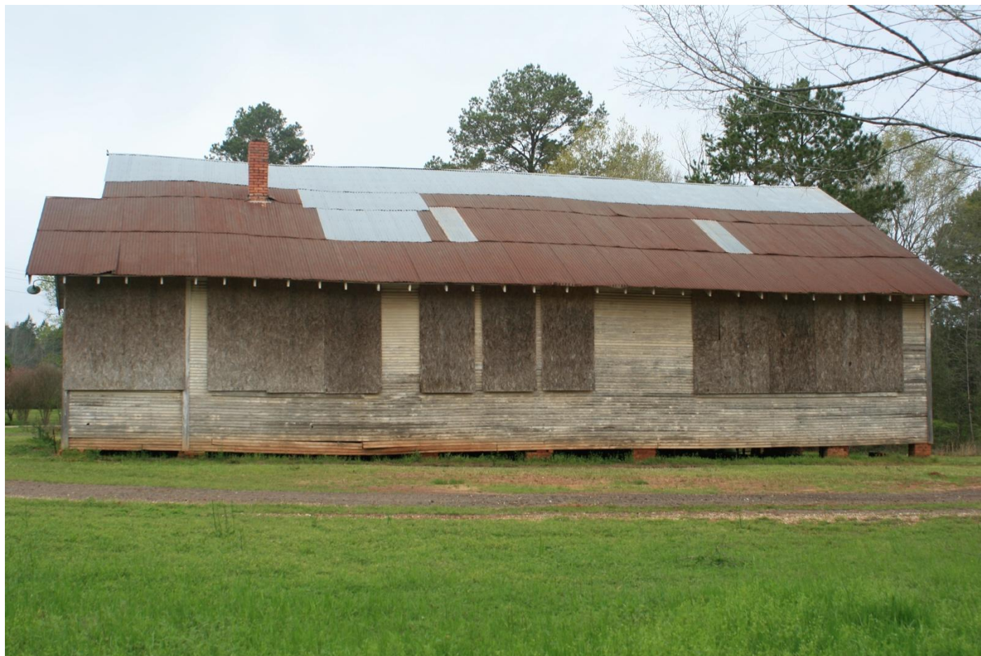
Photo 6 East elevation, camera facing west.
