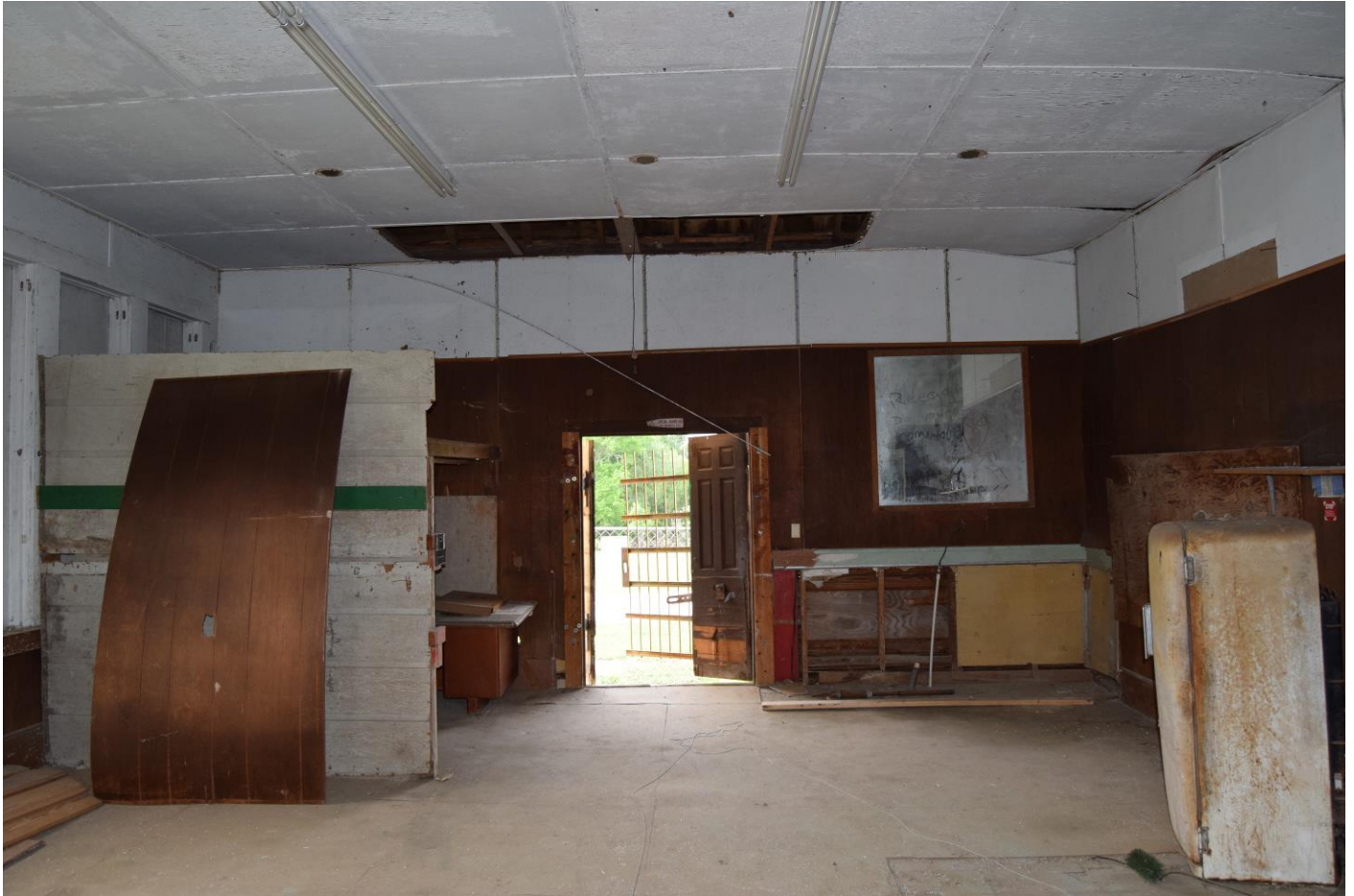
Photograph 11. Southwest interior wall, view facing southwest towards entrance.
