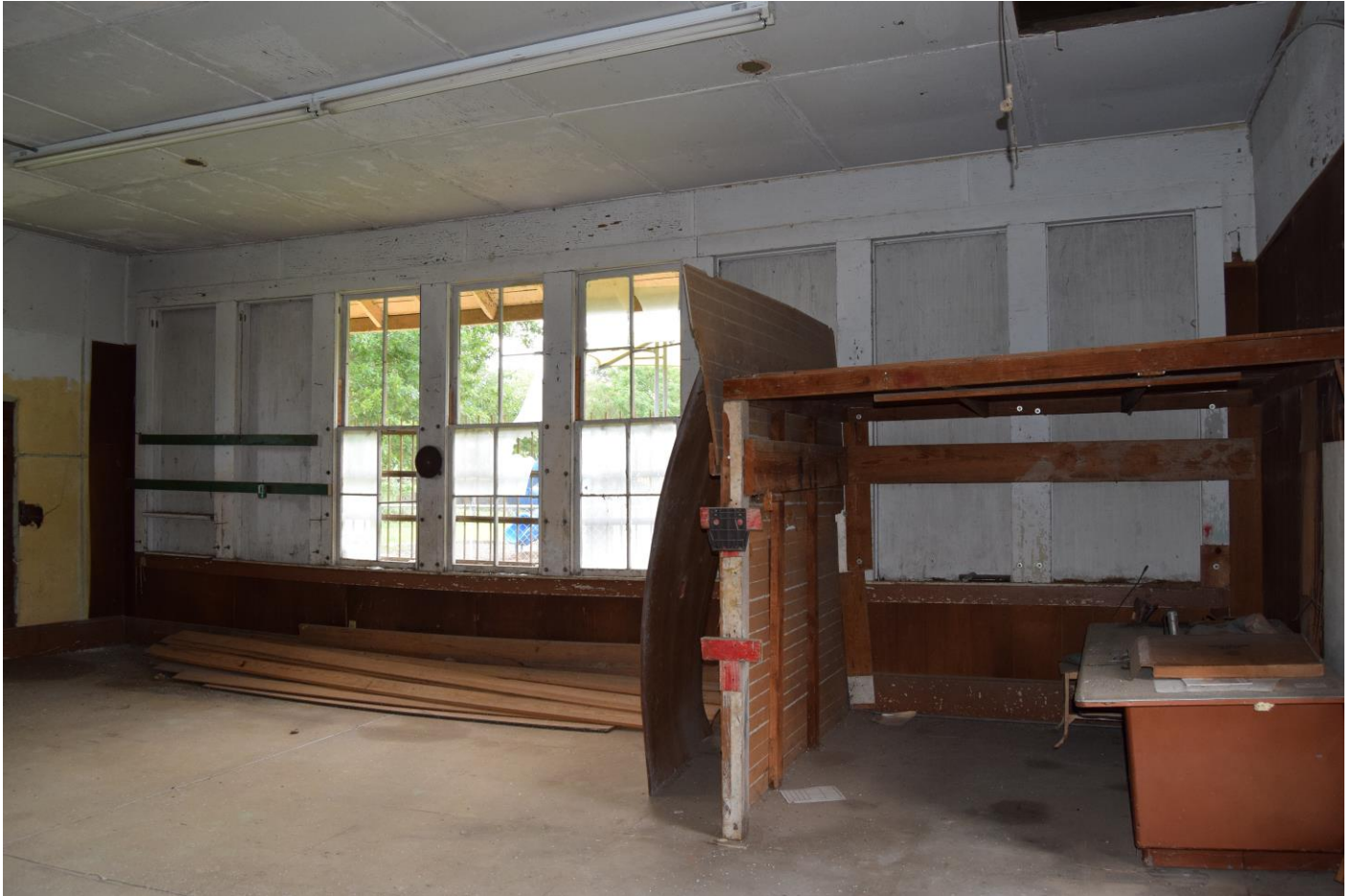
Photograph 13. North end of southeast interior wall, view facing east.
