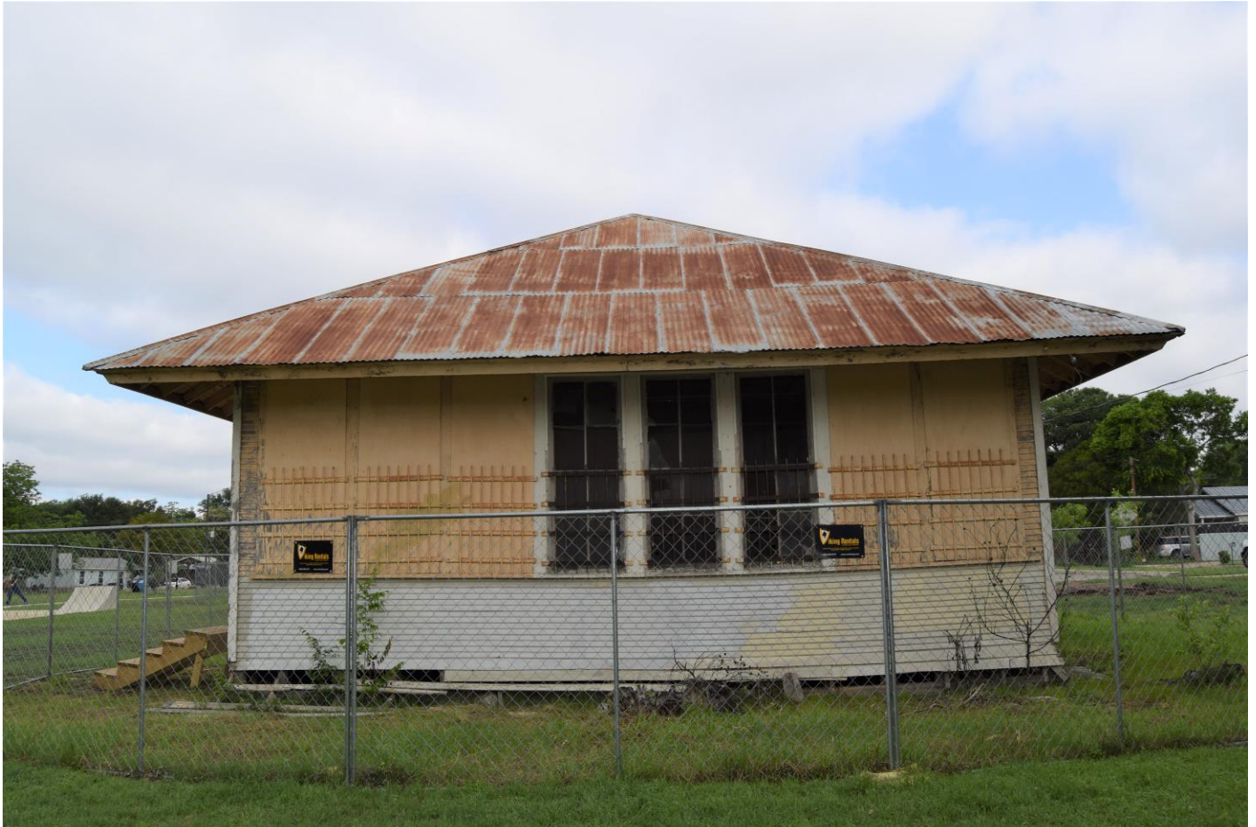
Photograph 4. Southeast exterior façade, view facing northwest.
