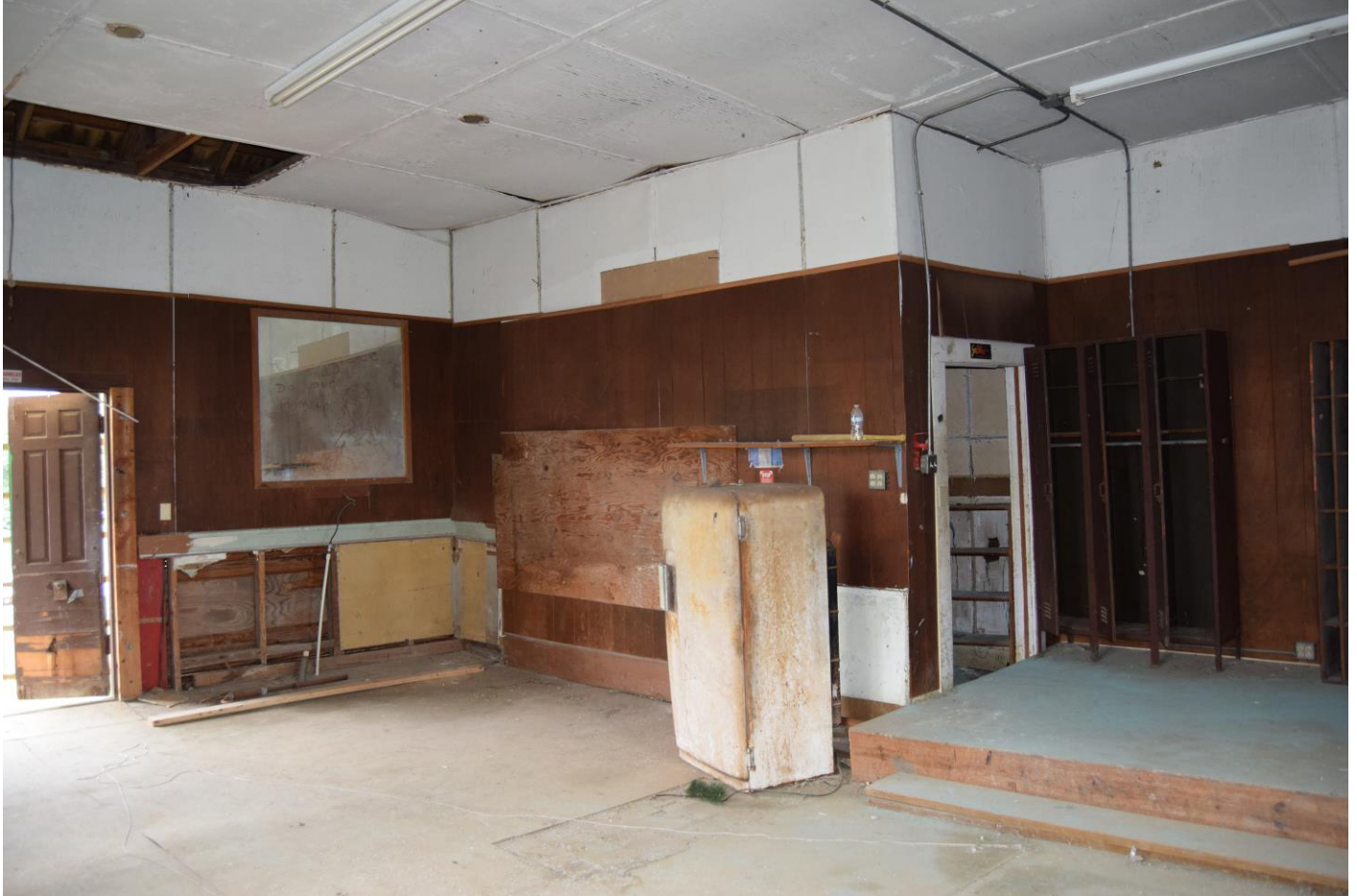
Photograph 10. Northwest and southwest interior walls, view facing west.
