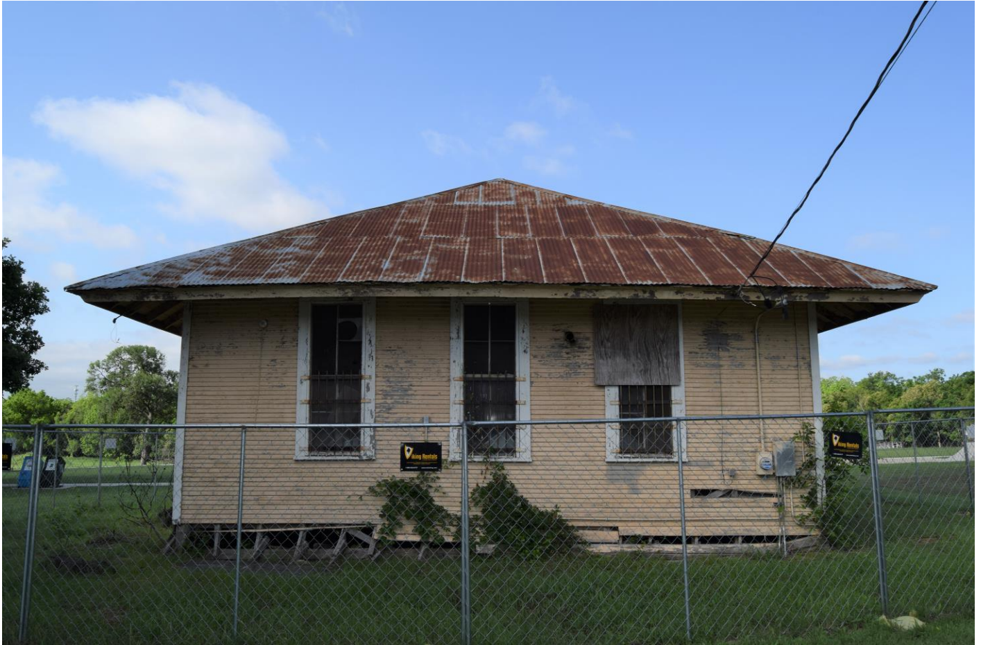
Photograph 6. Northeast exterior façade, view facing southwest.
