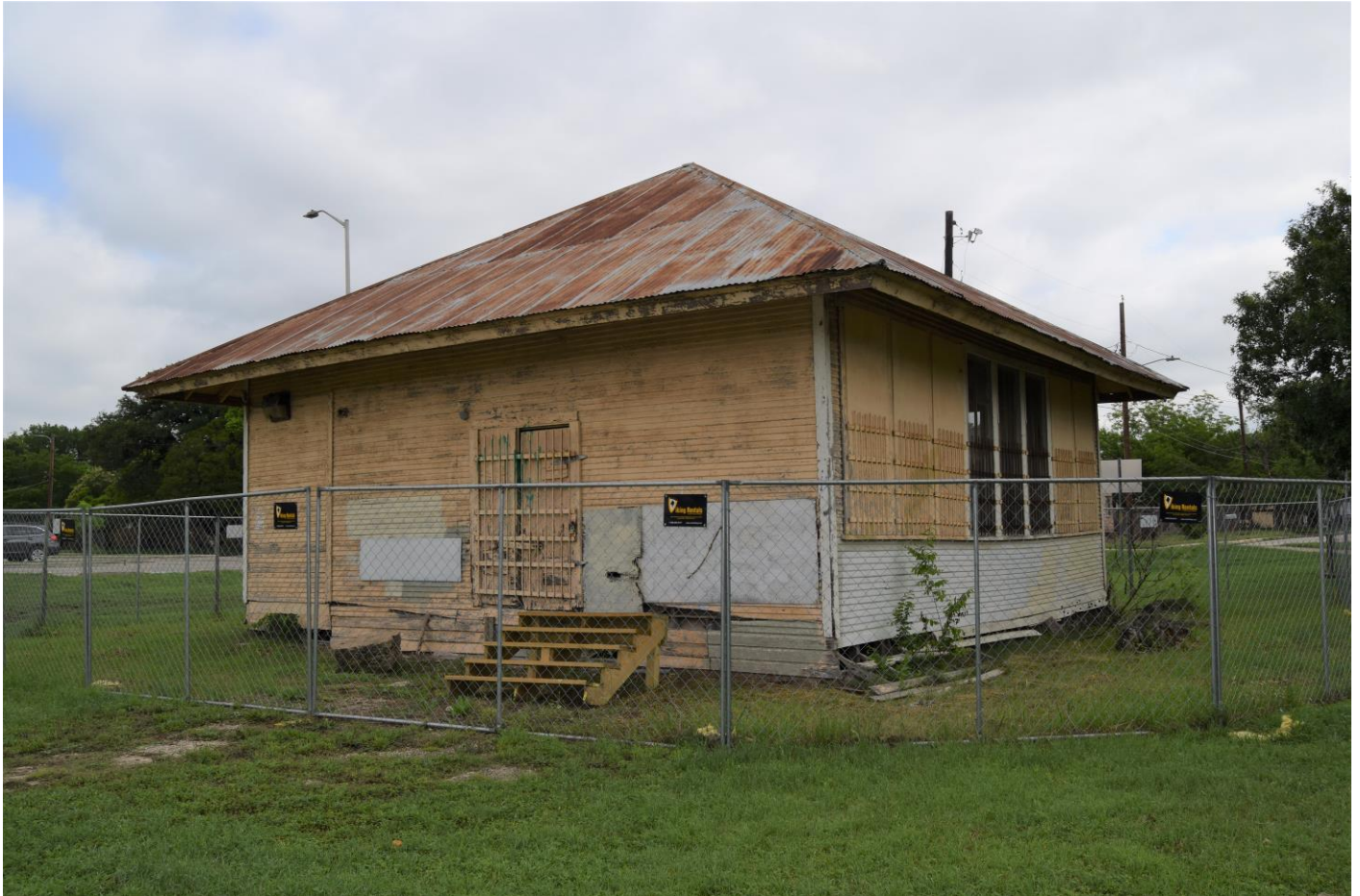
Photograph 3. South exterior oblique, view facing north.
