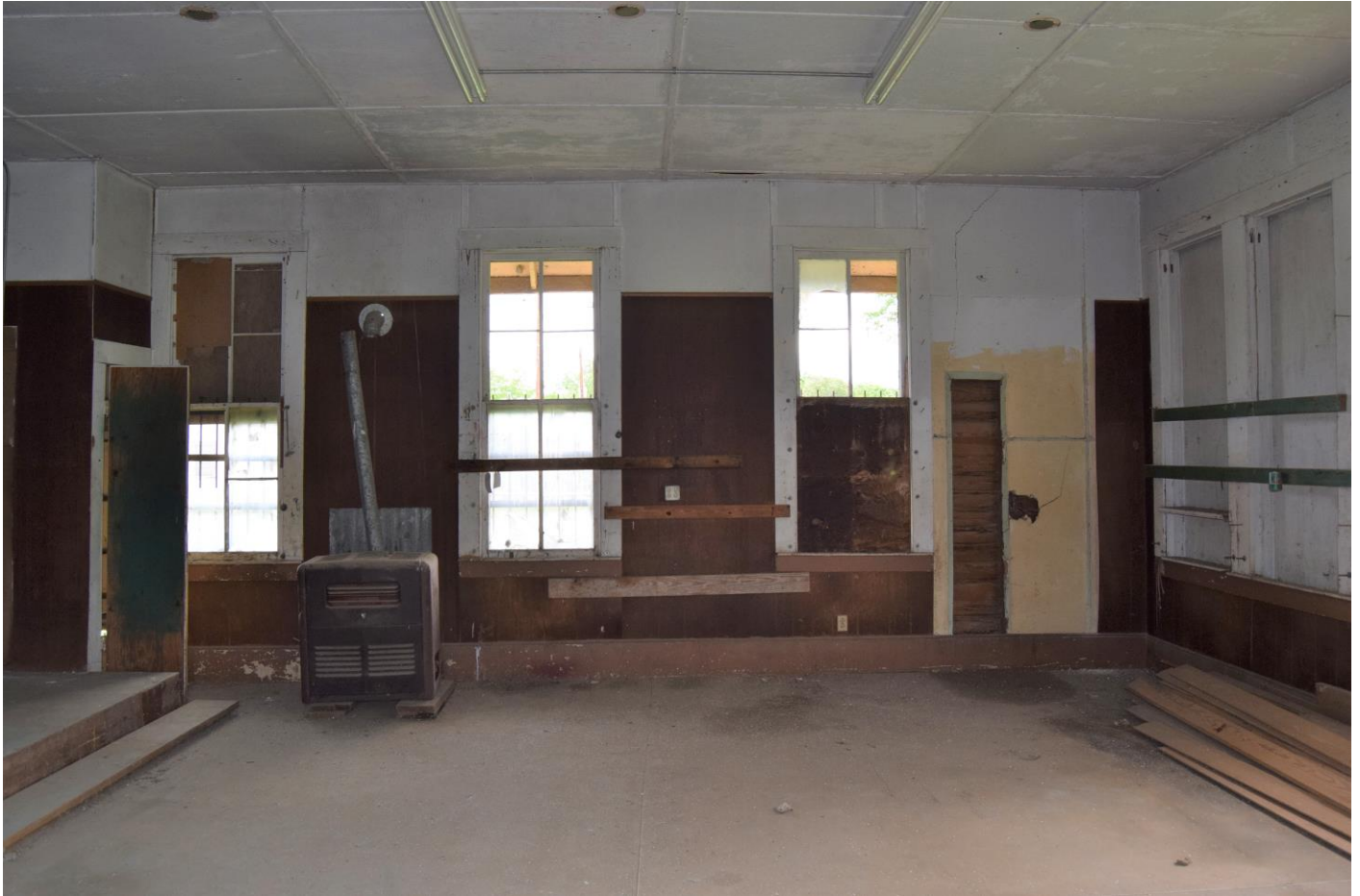
Photograph 8. Northeast wall of interior, view facing northeast.
