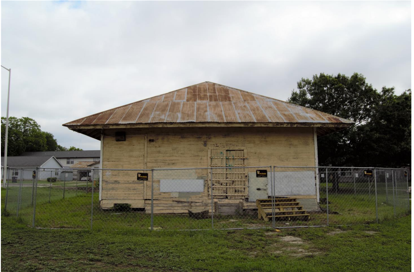
Photograph 2. Primary (southwest) exterior façade, view facing northeast.
