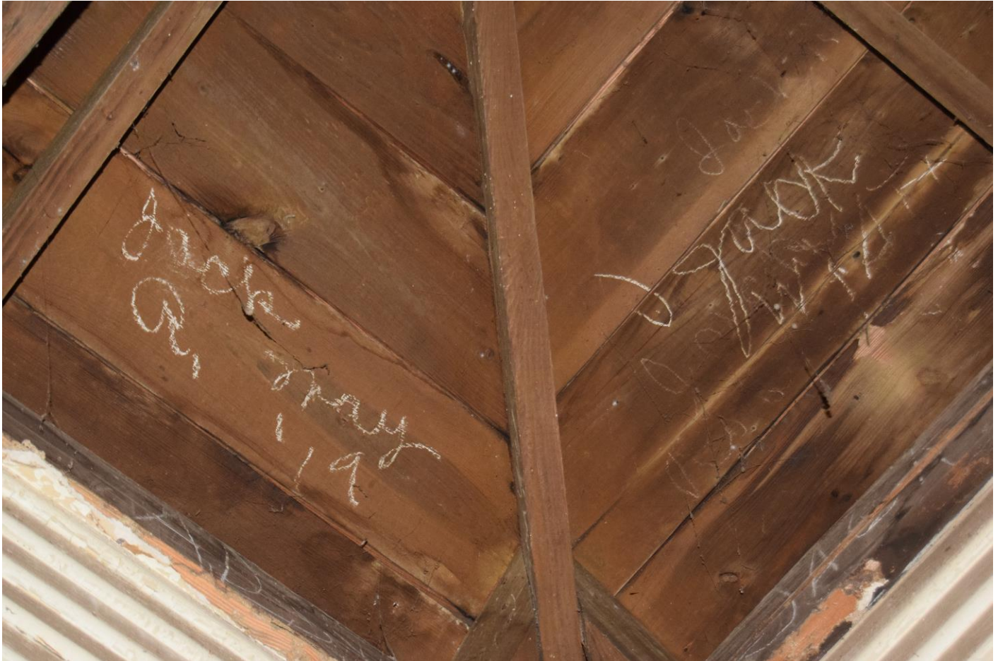
Photograph 17. Roof structure on interior of closet at south end of northwest wall, view facing southwest.
