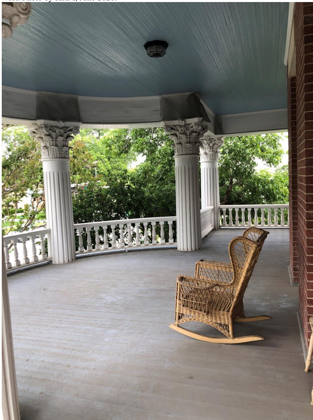
Figure 23. View of the rounded front gallery space on the second story of the Faust-Frueholz House, camera facing west. Photo by HHM, June 2021.
