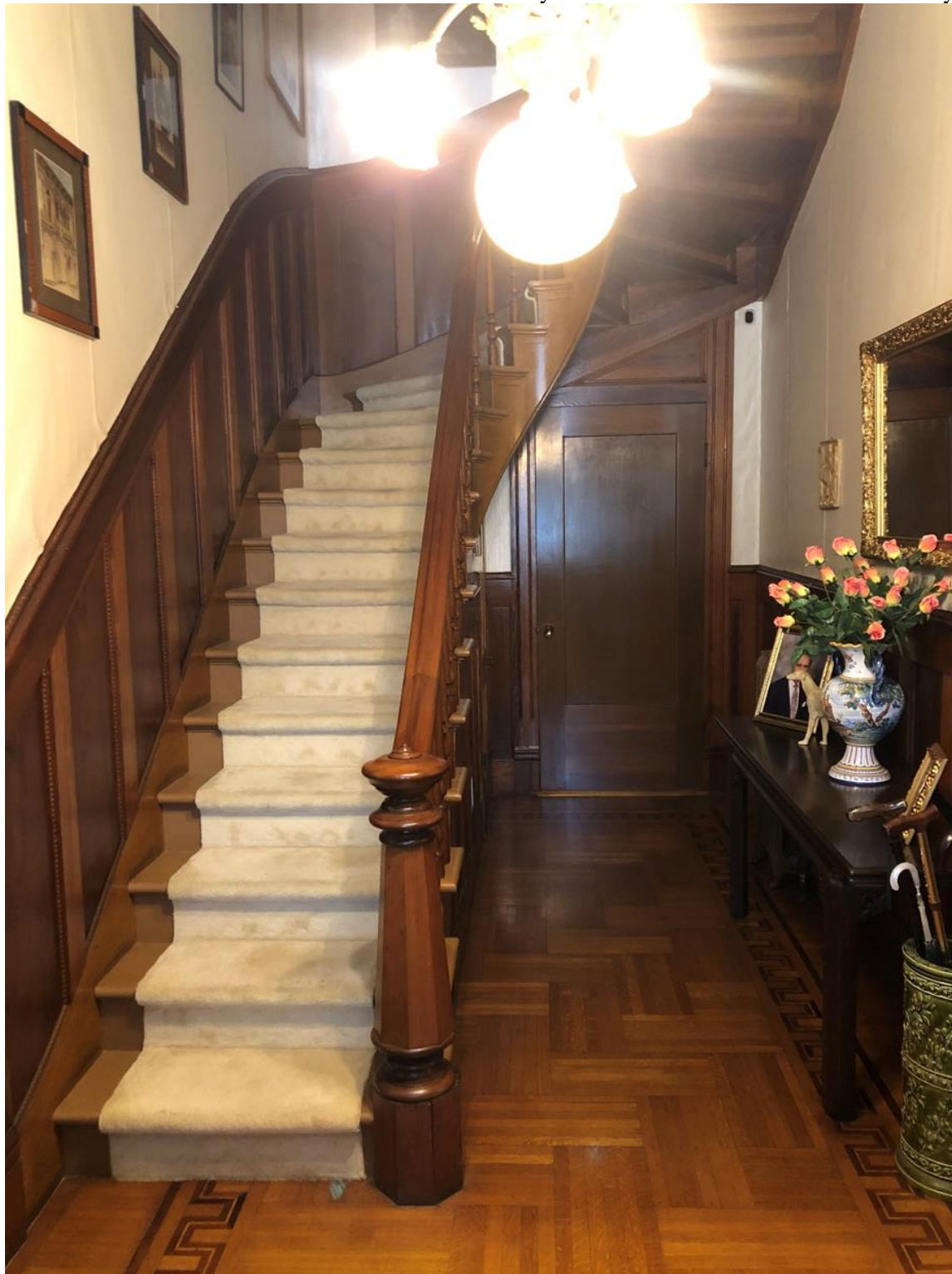
Photo 13. View of cantilevered staircase in the front foyer of the Faust-Frueholz House. Photo by HHM, June 2021.
