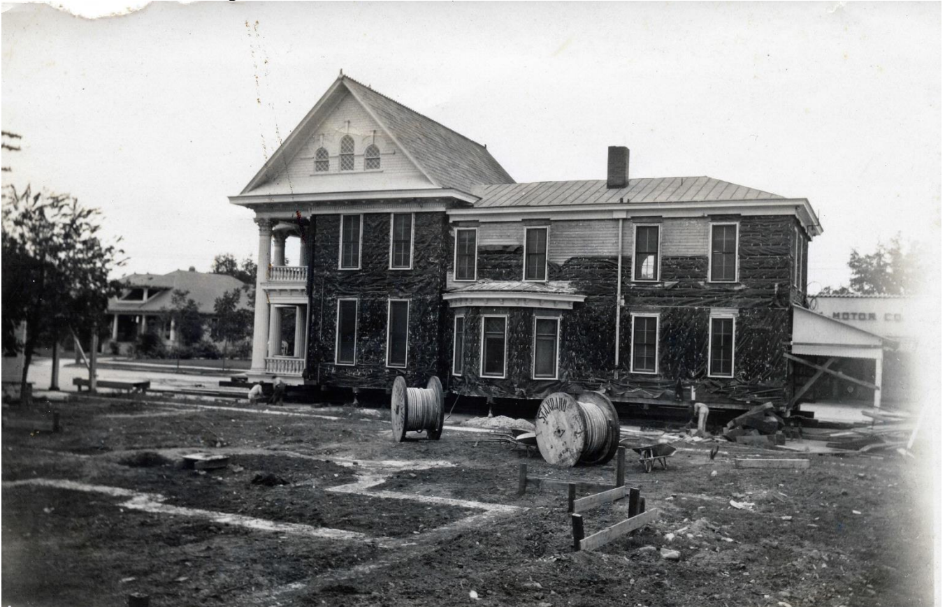
Figure 17. Photograph showing the Joseph Faust House near its final destination on the Frueholz property. Note the house's position in the middle of Coll Street. The stonework in the foreground was laid by Dr. Frueholz, Sr. as part of the new foundation for the relocated edifice. The exterior walls lack bricks, which were removed to lighten the load during the relocation process and later reinstalled. April 1929. Source: Joe Tays, current owner of the Frueholz House and Medical Building.
