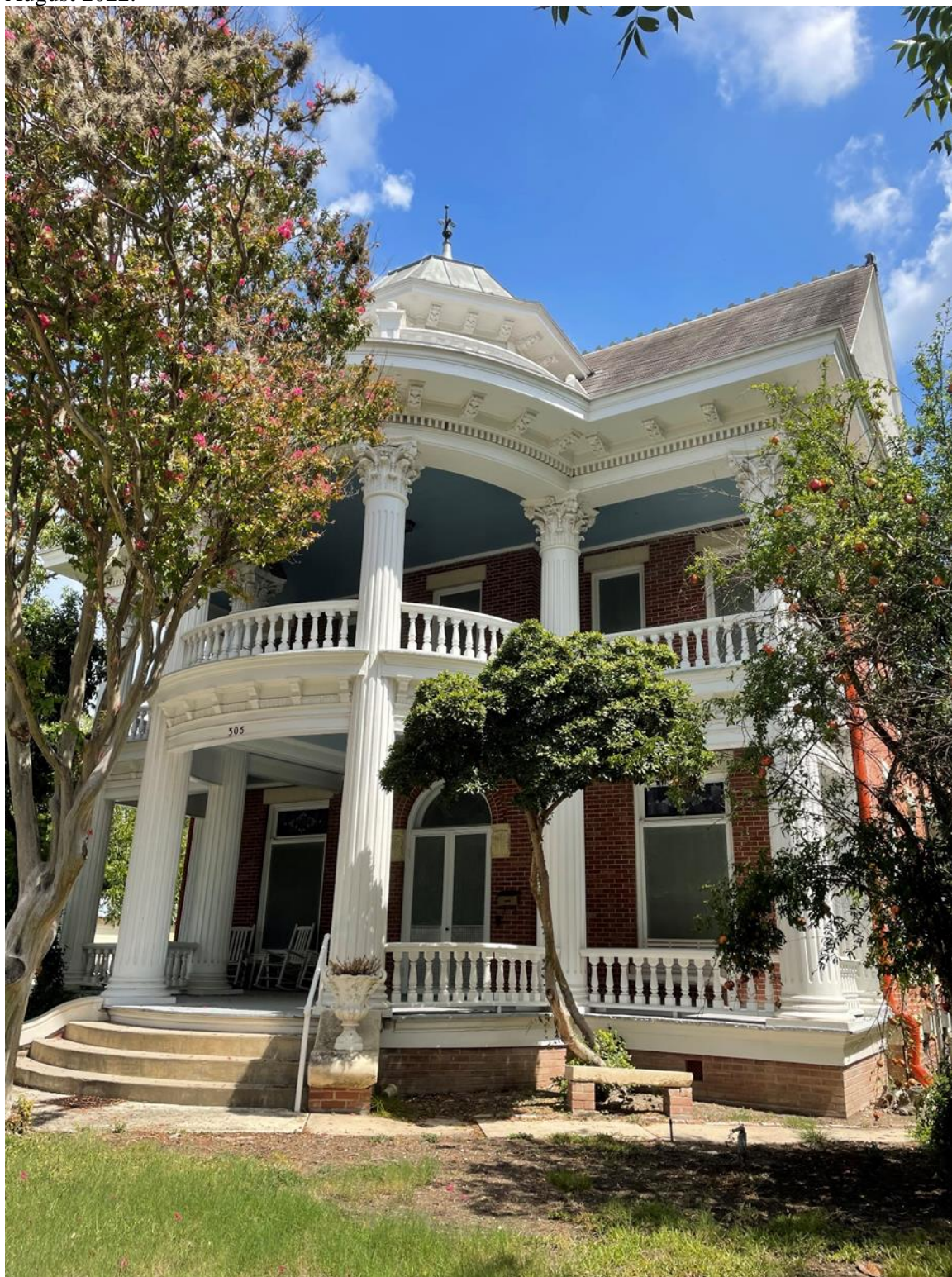
Photo 3. Oblique view of the front façade of the Faust-Frueholz House, camera facing north. Photo by HHM, August 2022.
