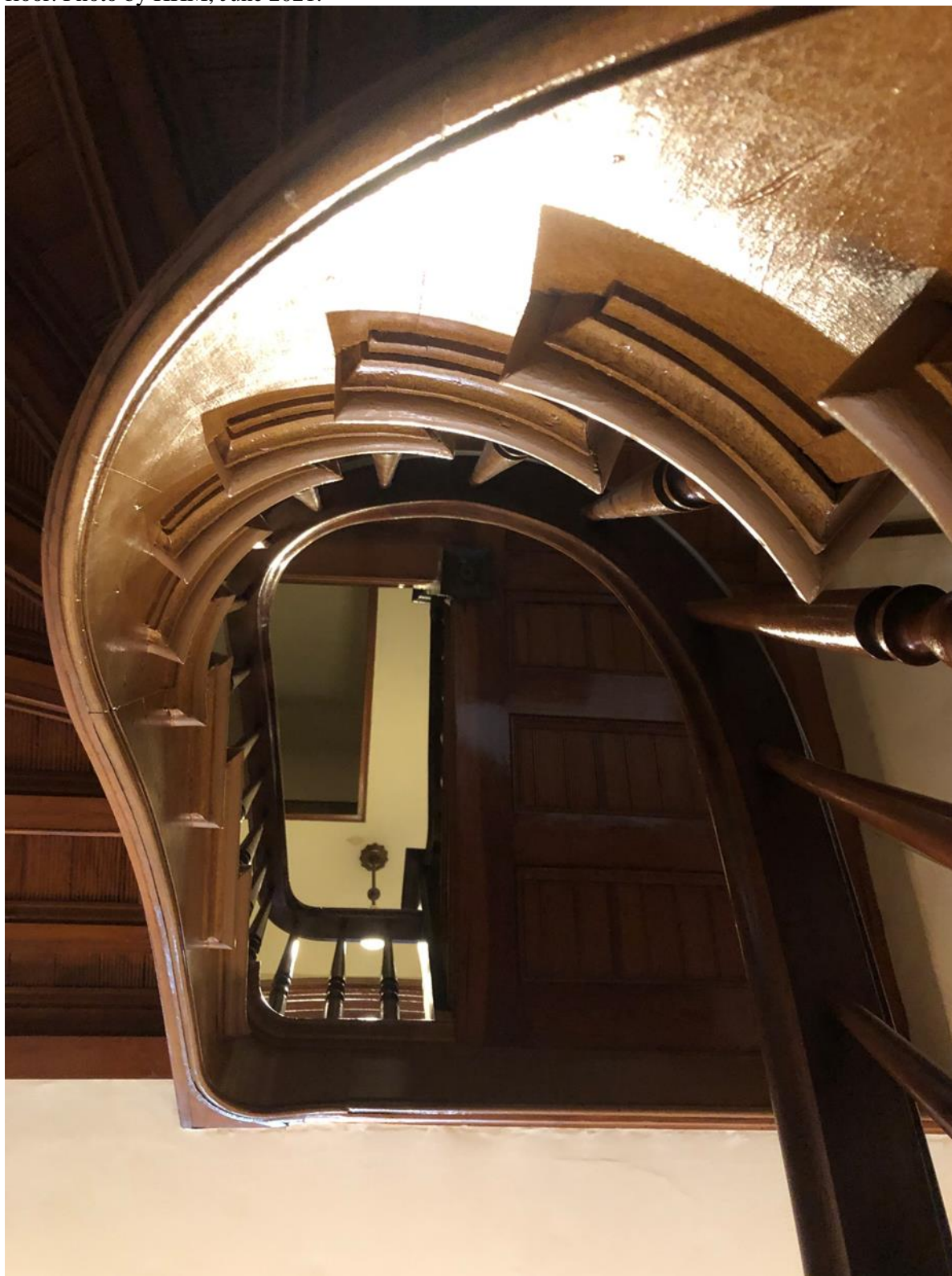
Photo 14. View of cantilevered staircase in the front foyer of the Frueholz House, looking upward from the ground floor. Photo by HHM, June 2021.
