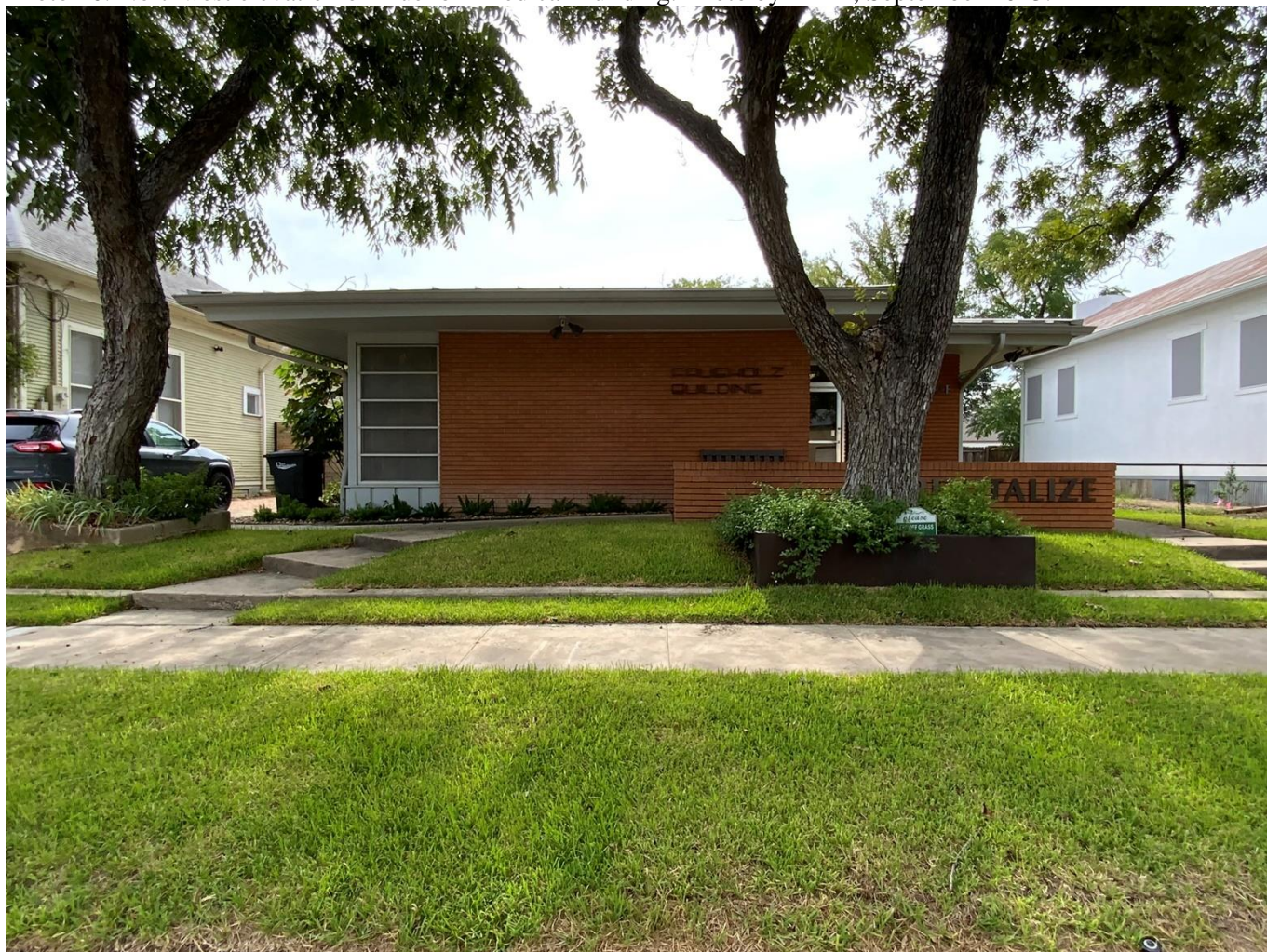
Photo 10. Northwest elevation of Frueholz Medical Building. Photo by HHM, September 2023.
