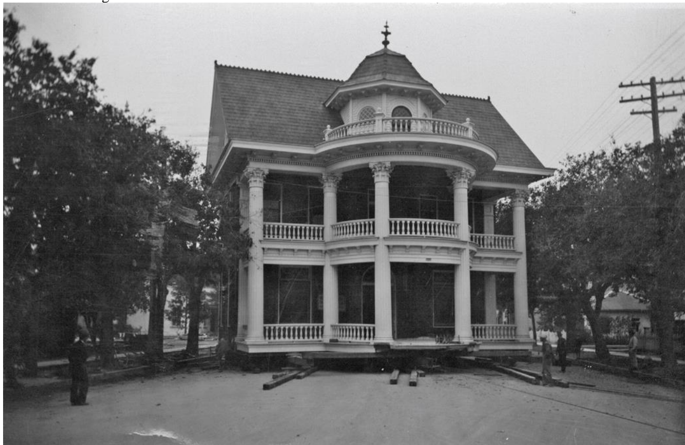
Figure 15. Photograph of the Joseph Faust House being hoisted onto rollers at its original location (where the Faust Hotel was later built and remains today). April 1929. Source: Joe Tays, current owner of the Frueholz House and Medical Building.
