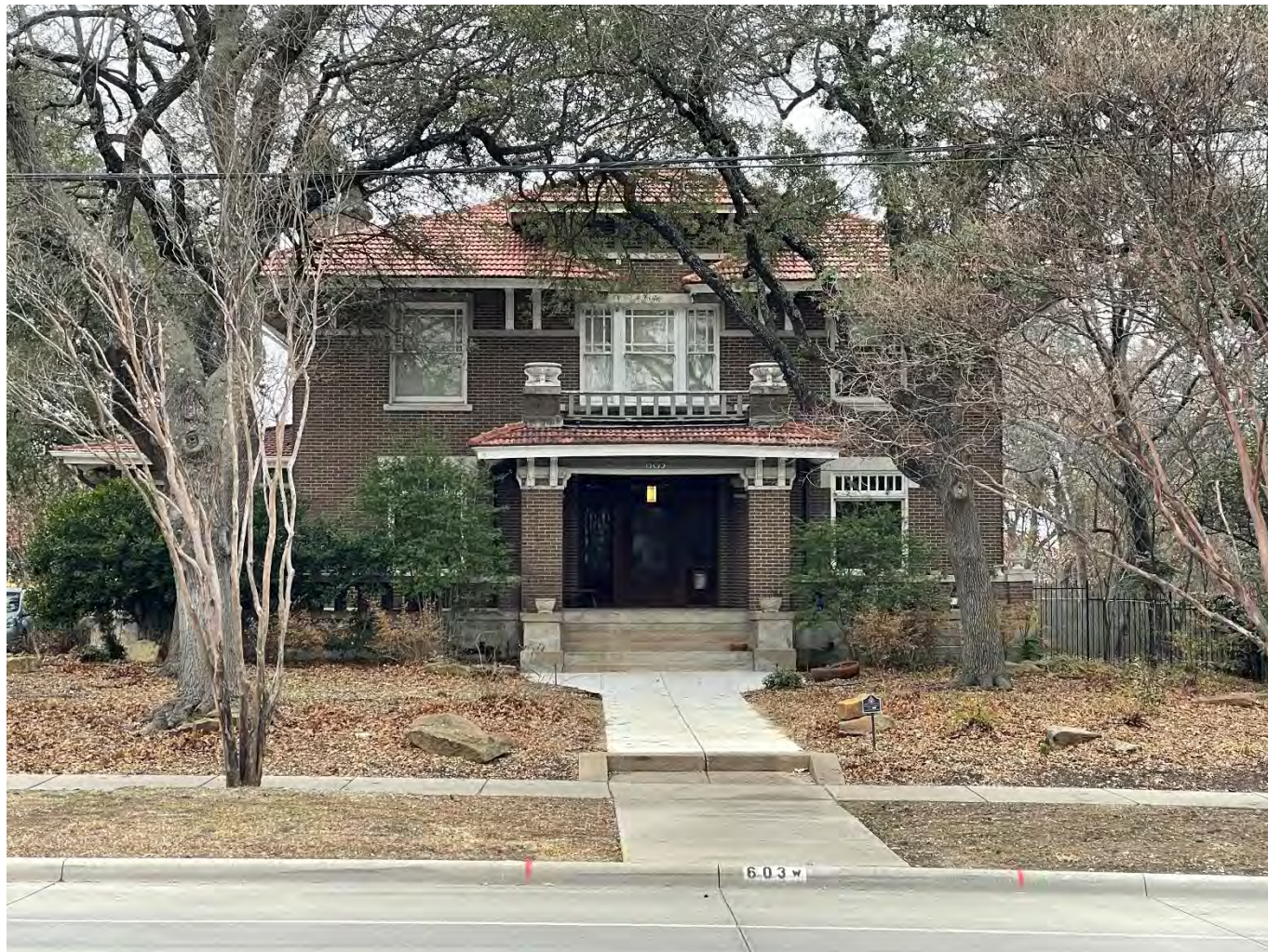
Photo 23. Frontal view of the McCartney House , 603 West Marvin Avenue A (Resource 24). Camera facing southwest.
