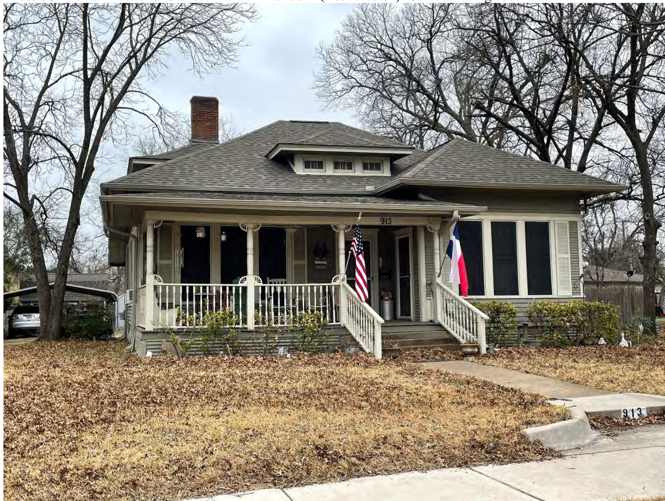
Photo 38. Frontal view of 913 West Marvin Avenue A (Resource 62). Camera facing southwest.
