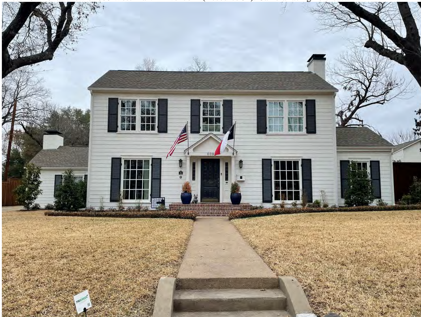
Photo 25. Frontal view of 608 West Marvin Avenue A (Resource 31). Camera facing northeast.
