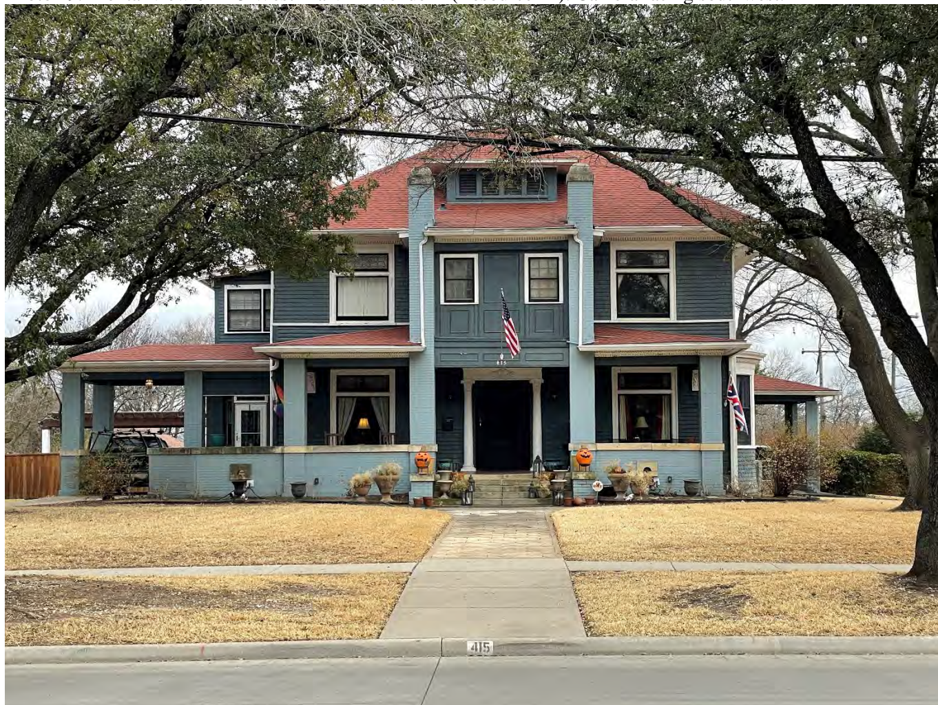
Photo 19. Frontal view of 415 West Marvin Avenue A (Resource 11). Camera facing southwest.
