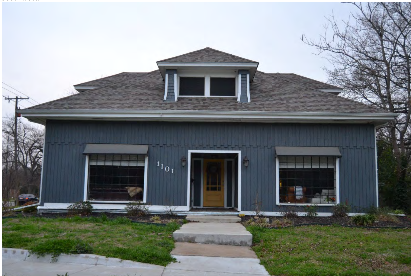
Photo 46. Frontal view of noncontributing resource at 1101 West Marvin Avenue A (Resource 73). Camera facing southwest.
