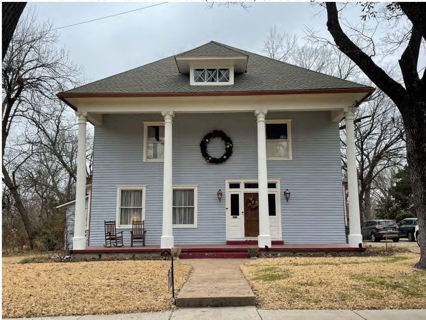
Photo 32. Frontal view of 901 West Marvin Avenue A (Resource 51). Camera facing southwest.
