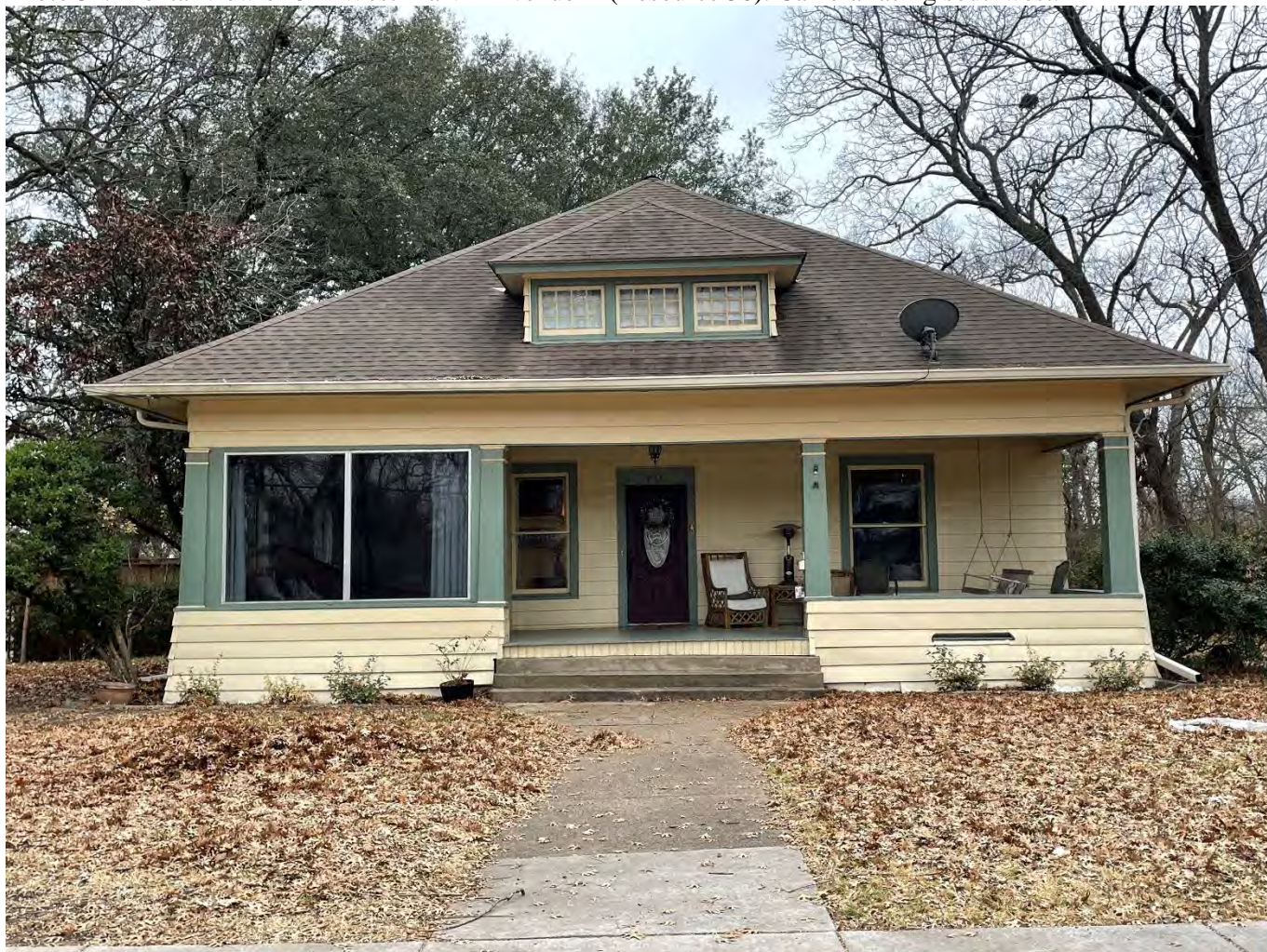
Photo 31. Frontal view of 811 West Marvin Avenue A (Resource 50). Camera facing southwest.
