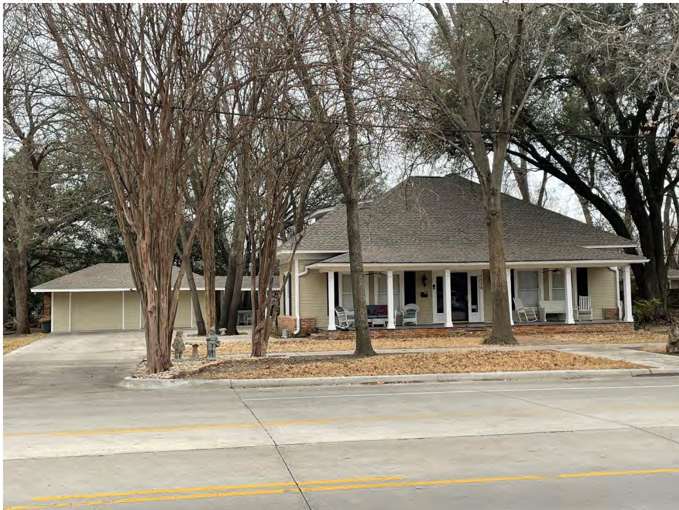
Photo 43. Frontal view of 1115 West Marvin Avenue A (Resource 77). Camera facing southwest.
