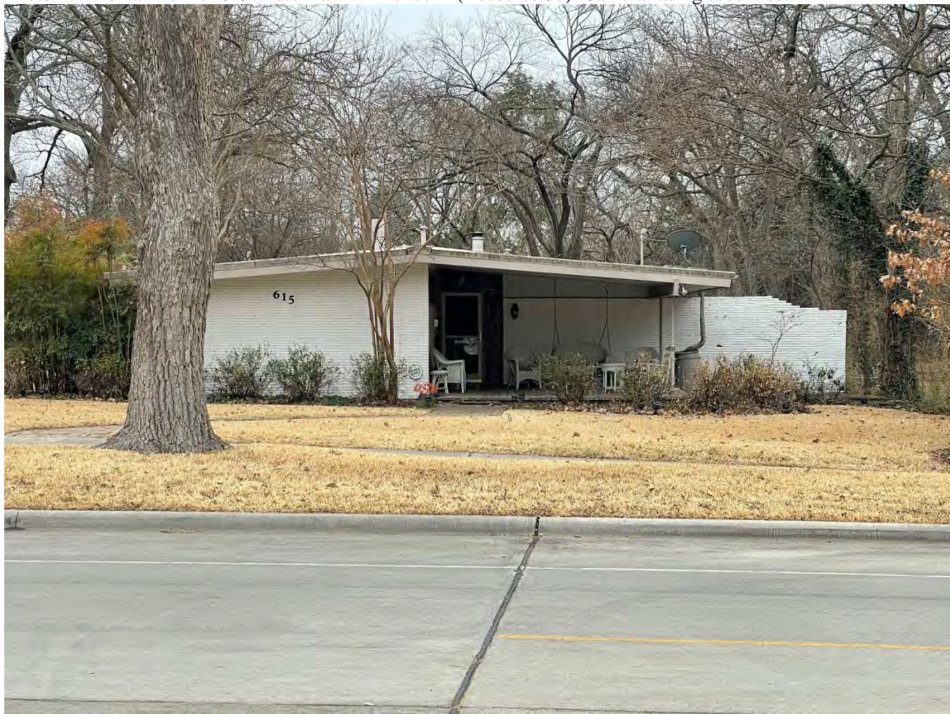
Photo 27. Frontal view of 615 West Marvin Avenue A (Resource 37). Camera facing southwest.
