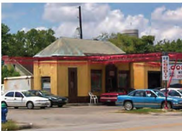
E. 2101 Washington Ave. Formerly Humble Oil & Refining Co. 1930, Single-Story, <3,000 SF
