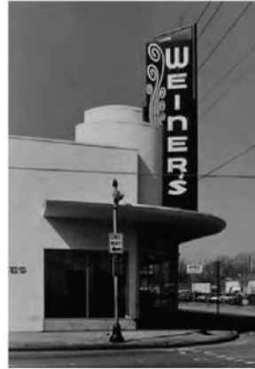
7. 4901 Washington Ave, Formerly Weiner's Dry Goods Store 1946. Photo by Yolita Schmidt.
