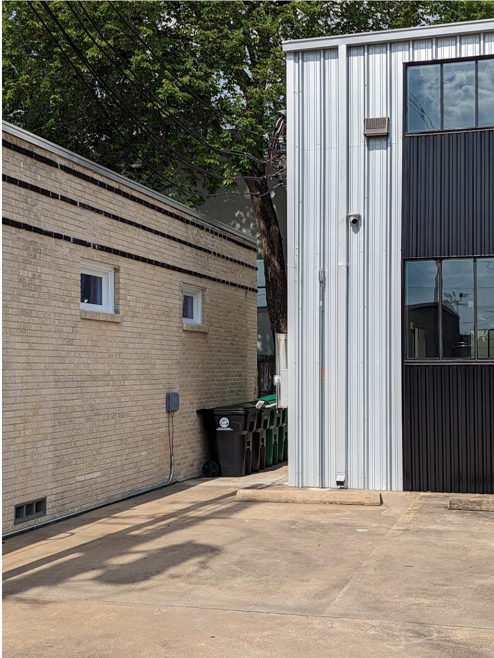
Photo 8: South elevation showing previous connection to adjacent building. June 8, 2023.
