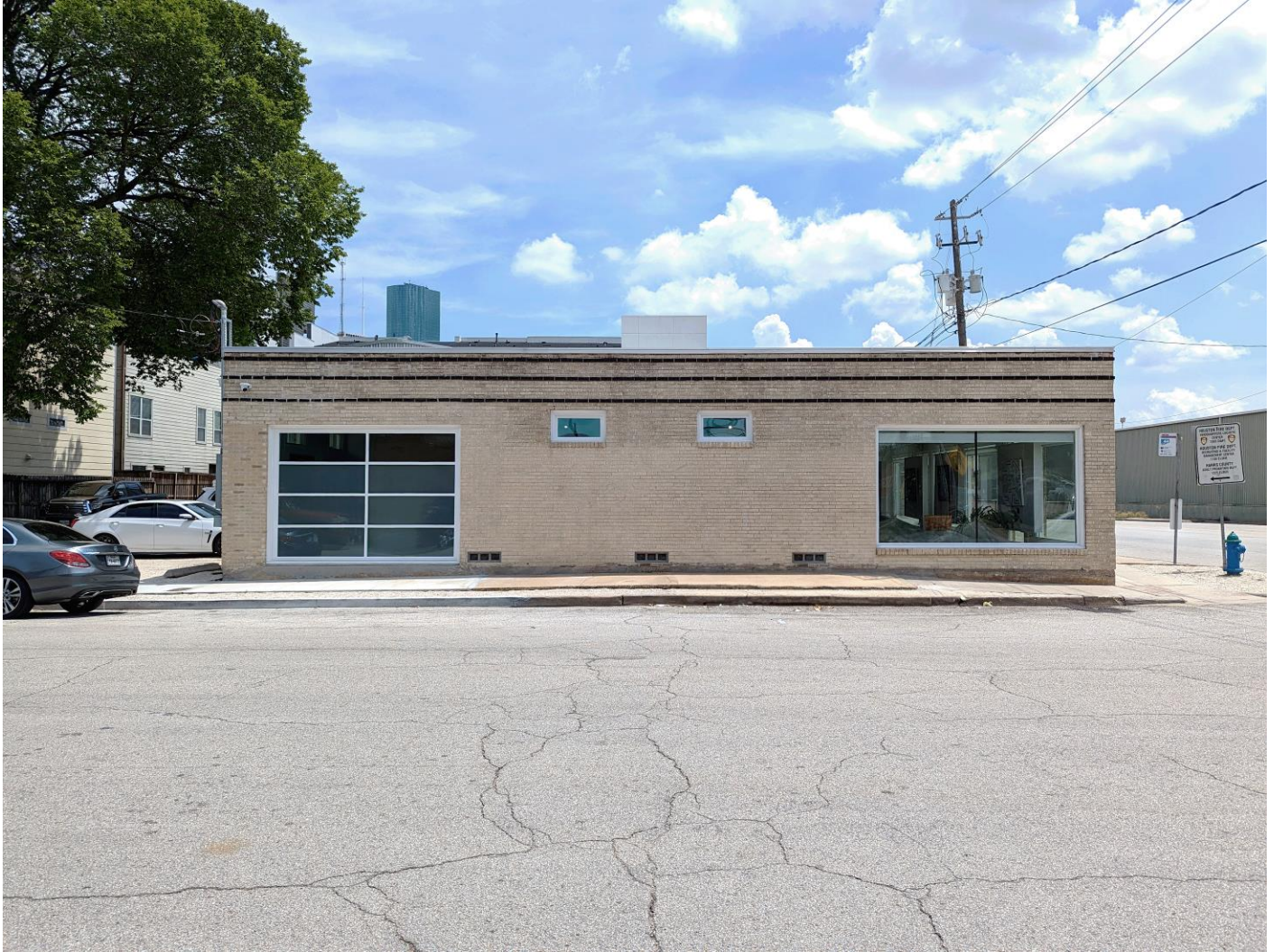
Photo 4: North elevation facing Dart Street. June 8, 2023.
