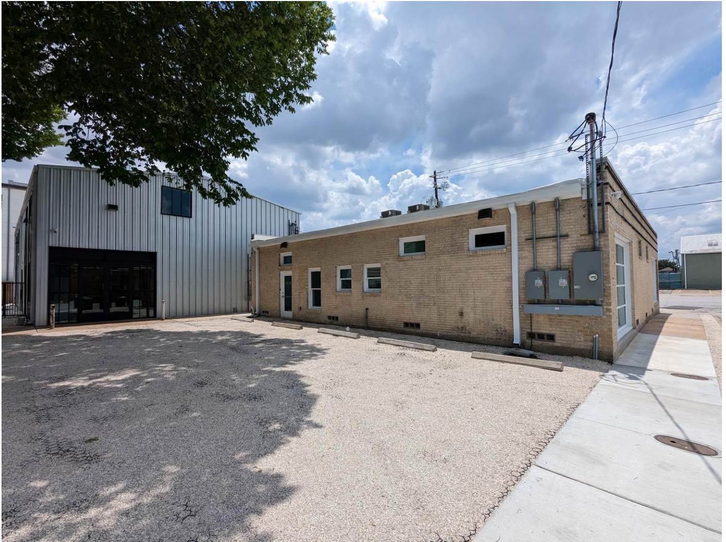
Photo 5: Rear (east) elevation with adjacent building at 1224 Houston Avenue at left. June 11, 2023.
