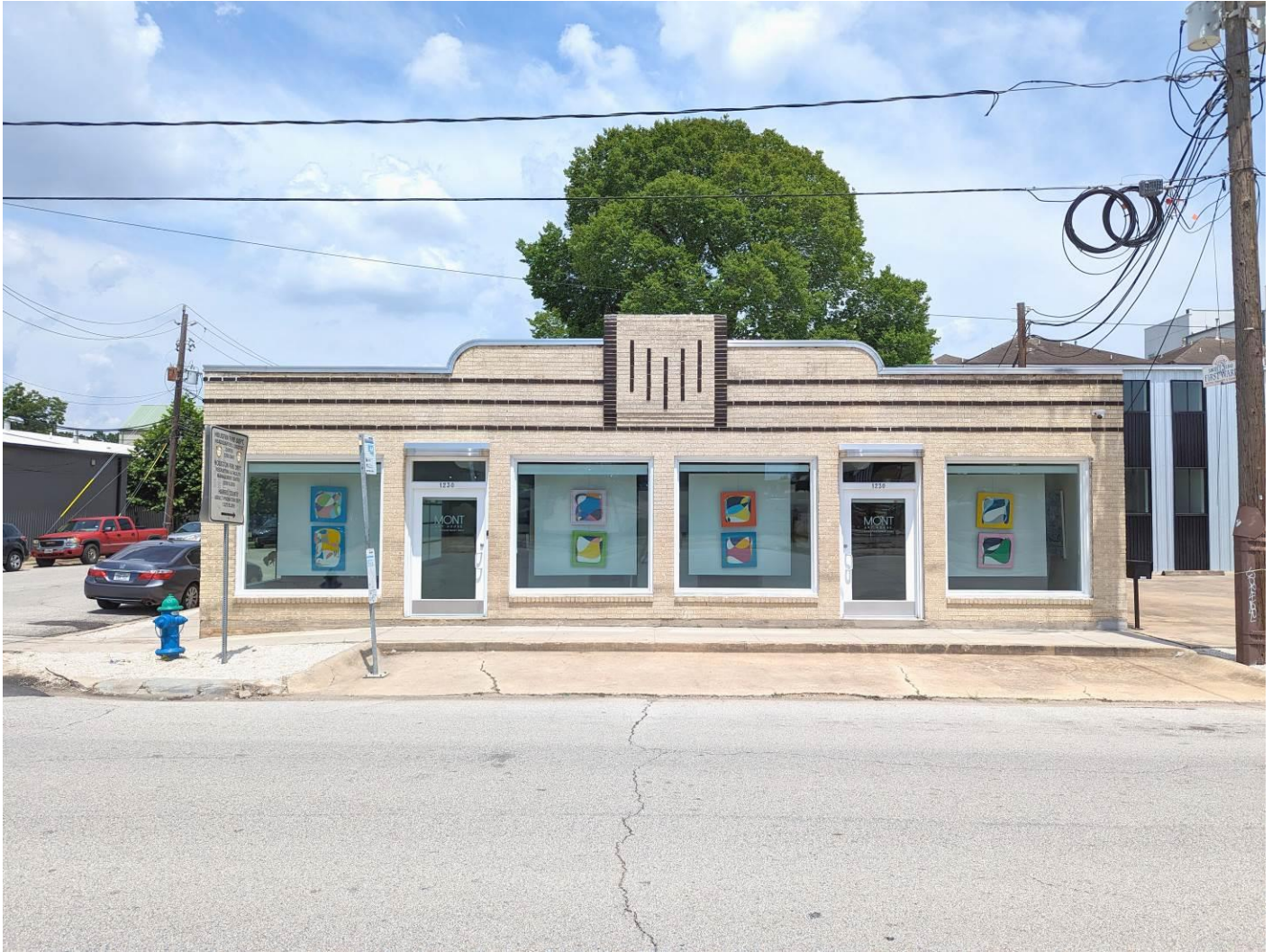
Photo 1: Primary (west) elevation facing Houston Avenue. June 8, 2023.
