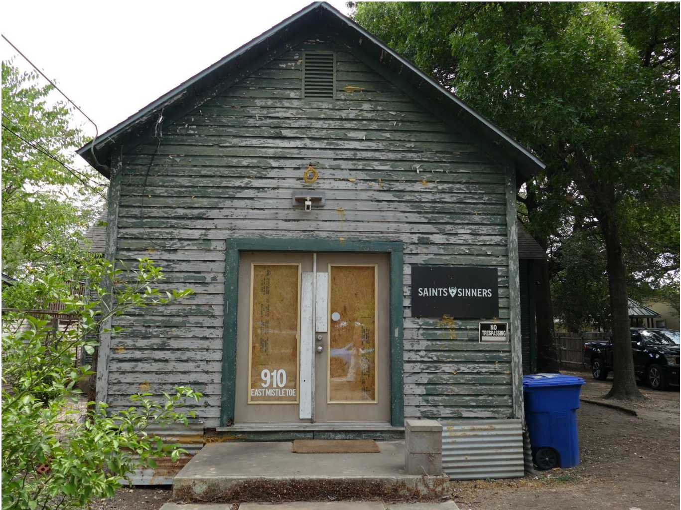
Photo 3: Primary (North) Elevation. View South.
