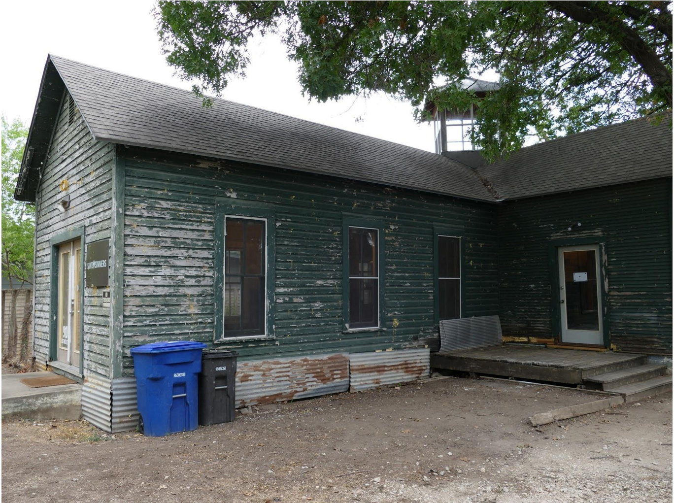
Photo 4: Oblique. Primary (North) and West Elevations. View Southeast.
