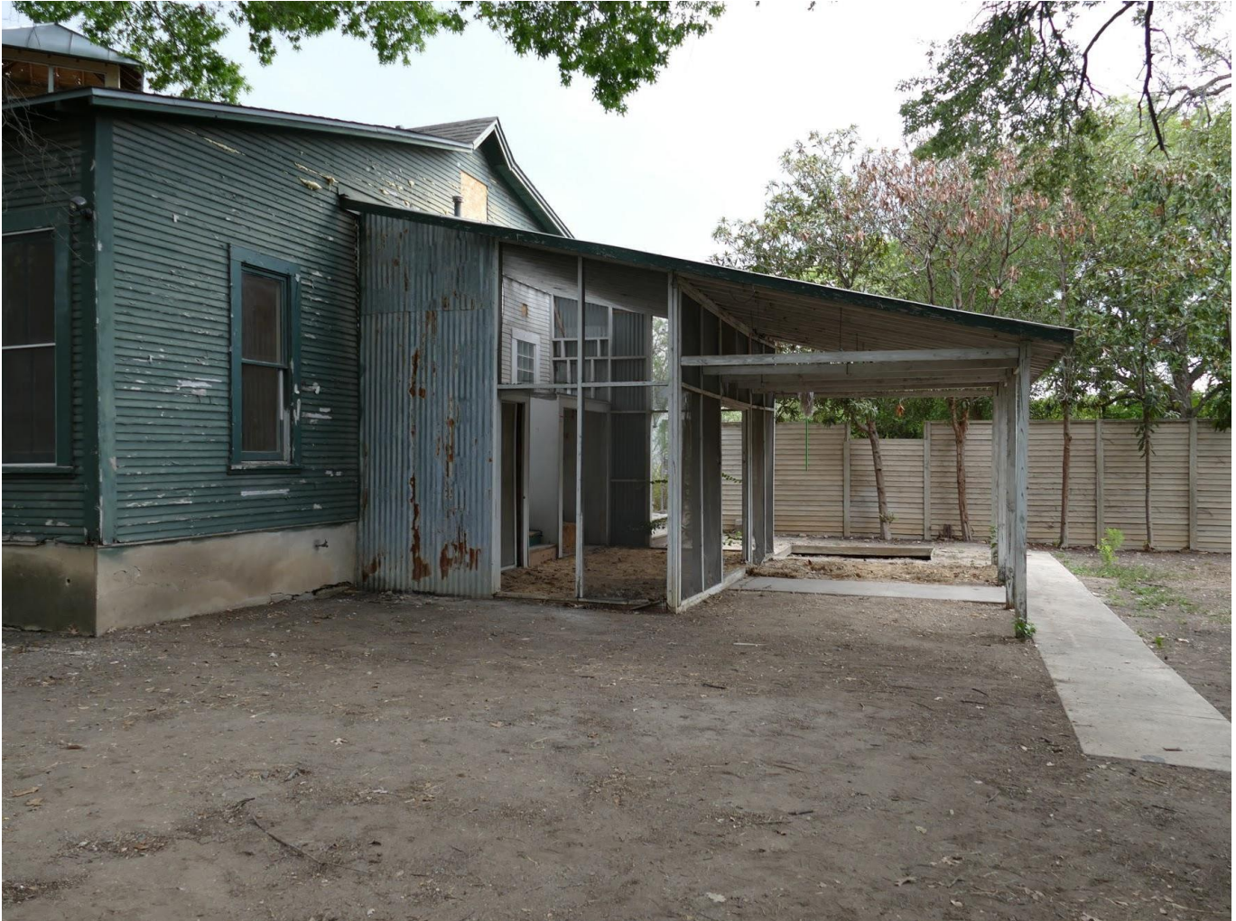
Photo 6: South Elevation, View East.
