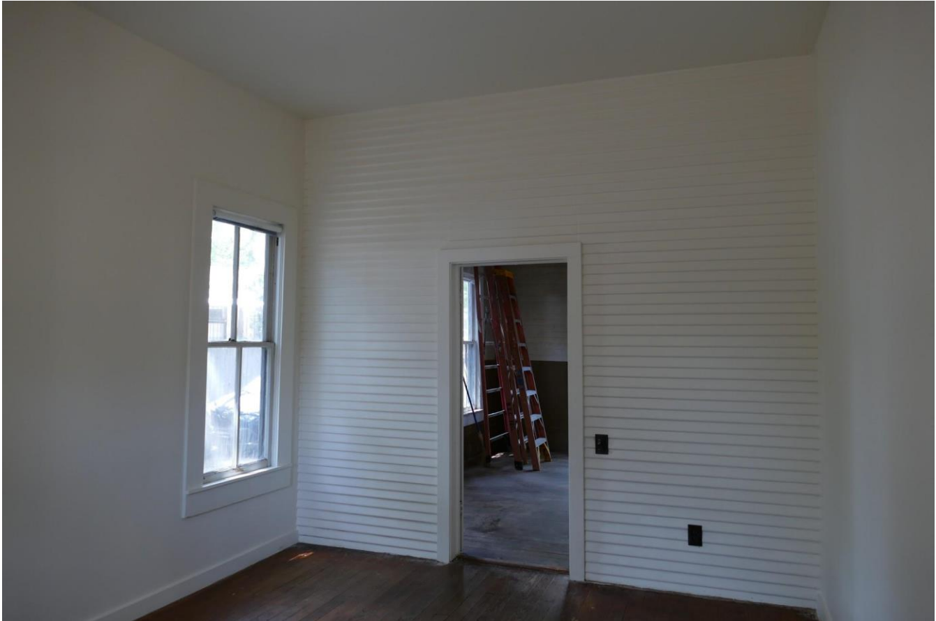
Photo 26: West room in rear addition. View North.
