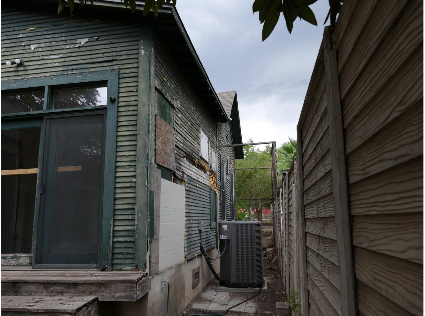
Photo 10: South and East Elevations. View North.
