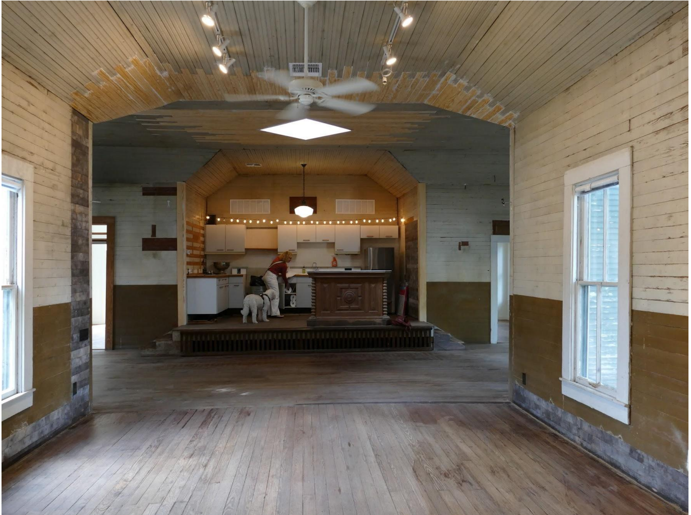
Photo 19: View of apse from nave. View South.
