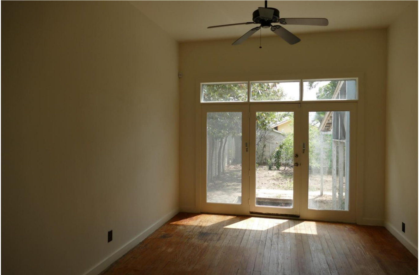
Photo 22: East room in rear addition. View South.
