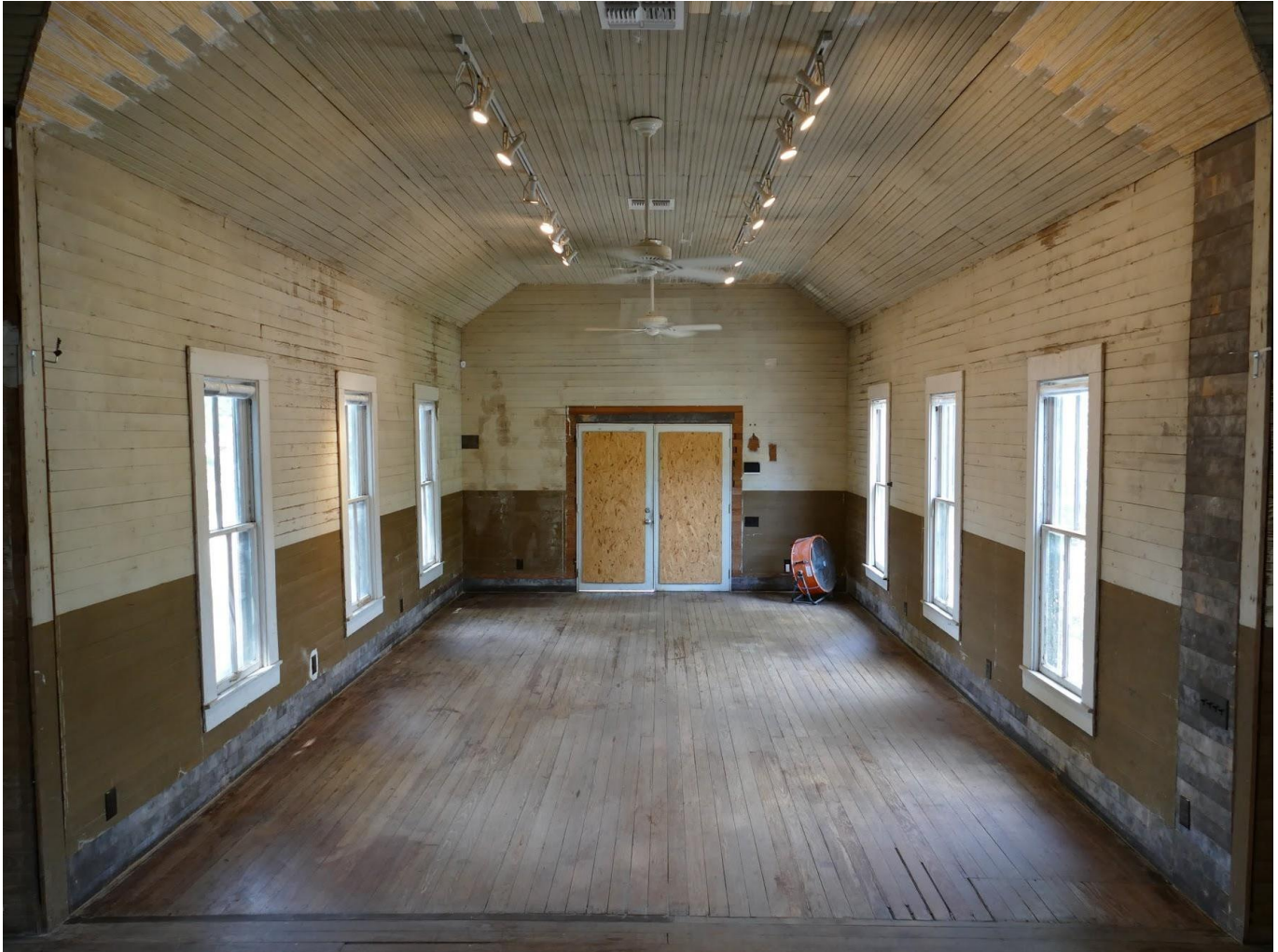
Photo 13: Nave facing main entrance. View North.
