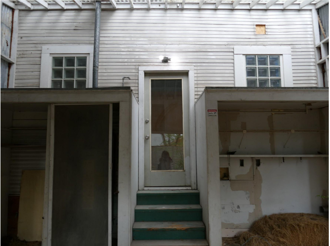
Photo 8: South Elevation beneath Shed. View North.
