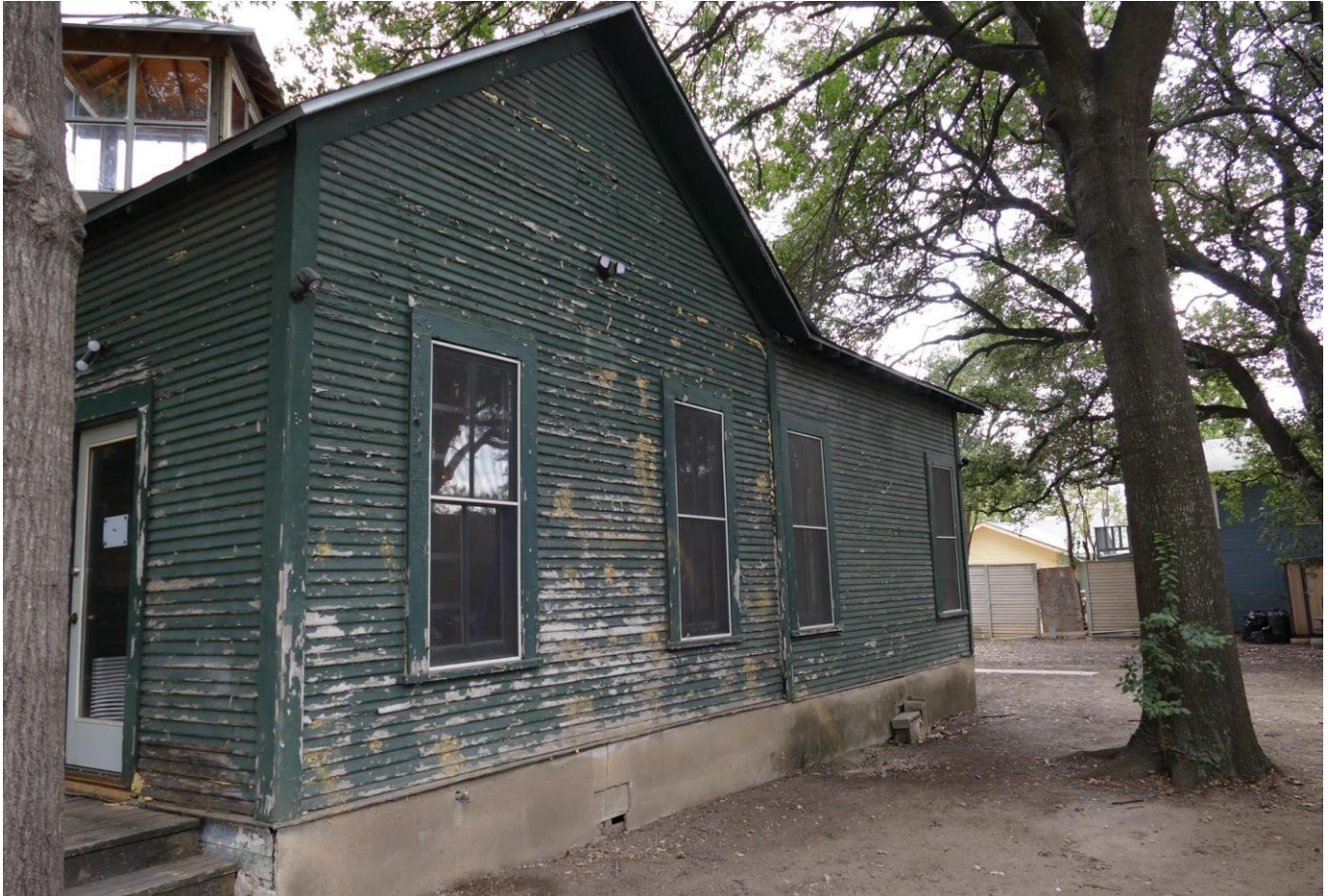
Photo 5: West Elevation. View Southeast.
