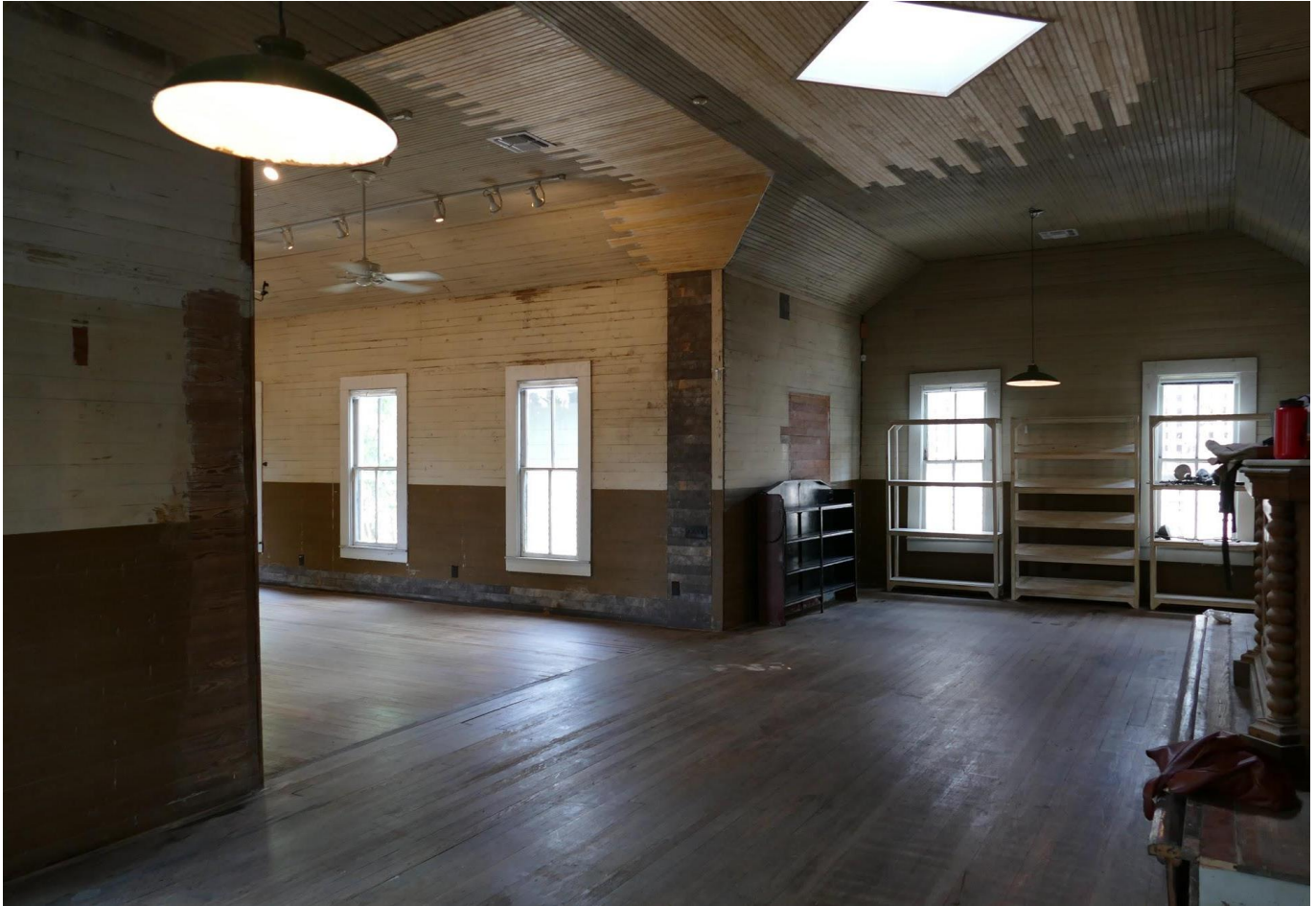
Photo 16: View from transept into nave. View Northeast.
