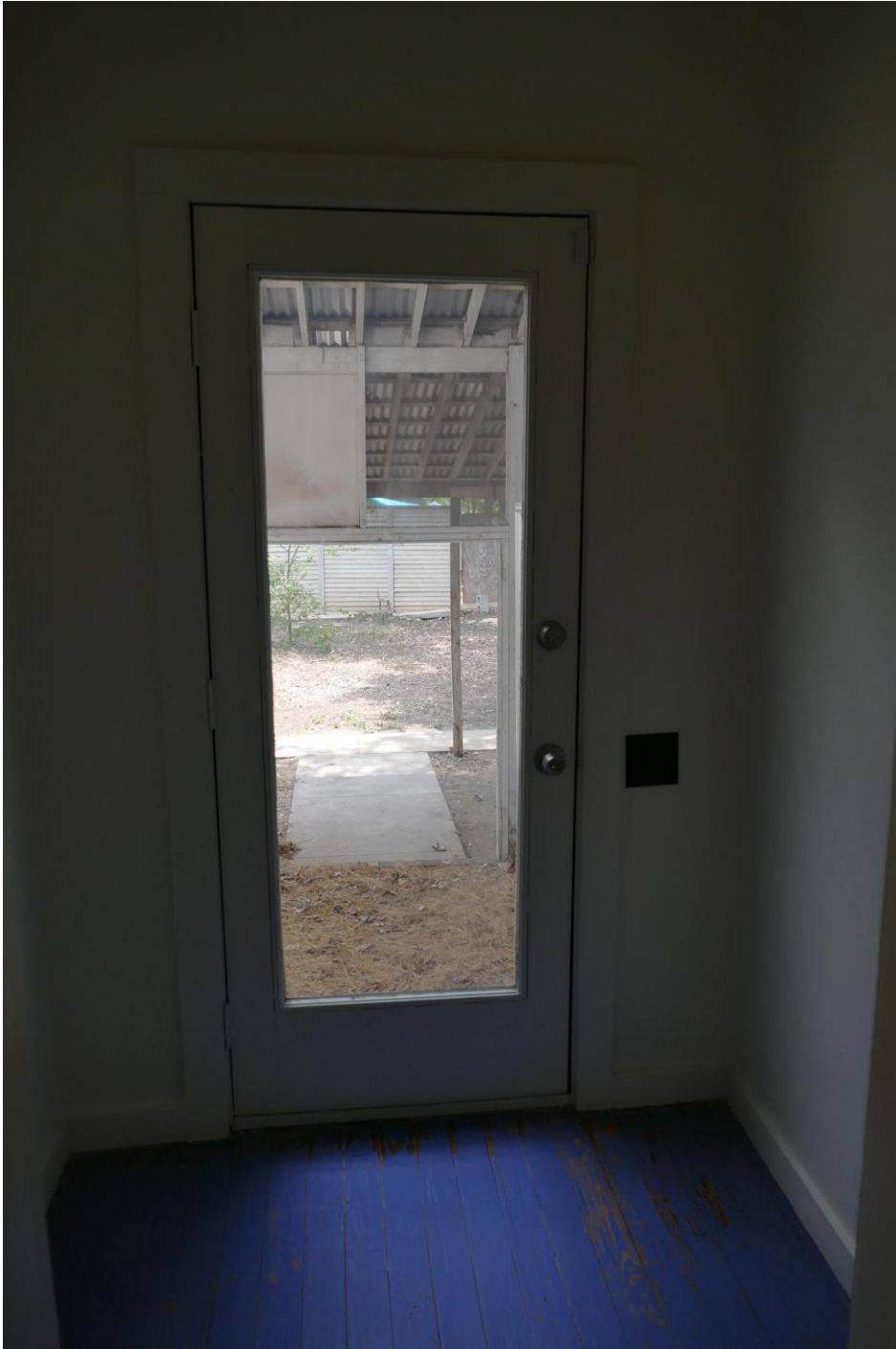
Photo 25: Rear hall with exterior door. View South.
