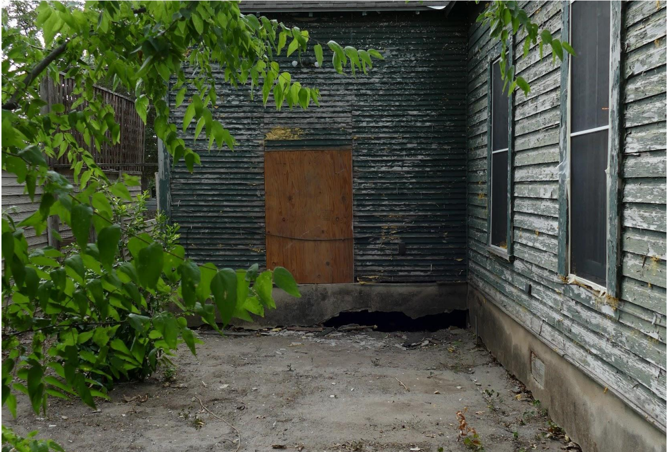
Photo 11: East wing North Elevation. View South.
