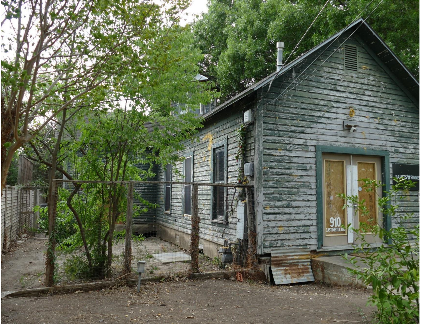
Photo 12: North and East Elevations. View Southwest.
