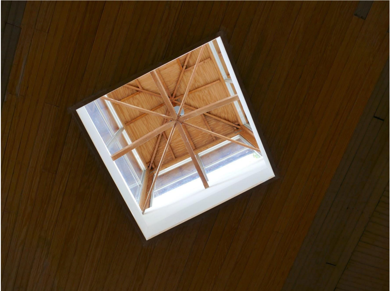
Photo 18: View of cupola above transept.
