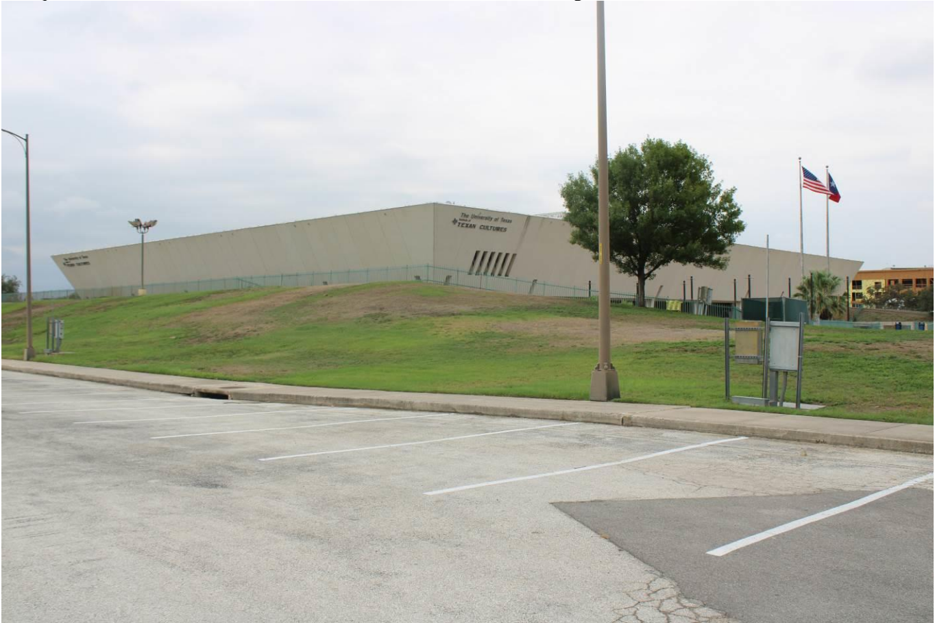
Oblique of ITC northwestern and northeastern elevations, camera facing south
