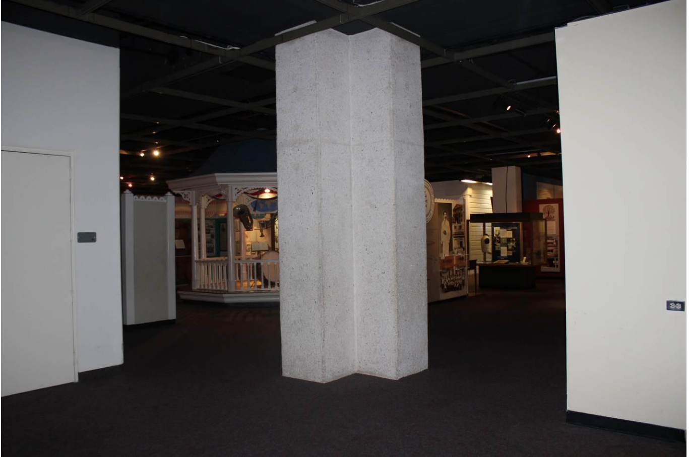
Photo 20 Interior limestone aggregate concrete pier
