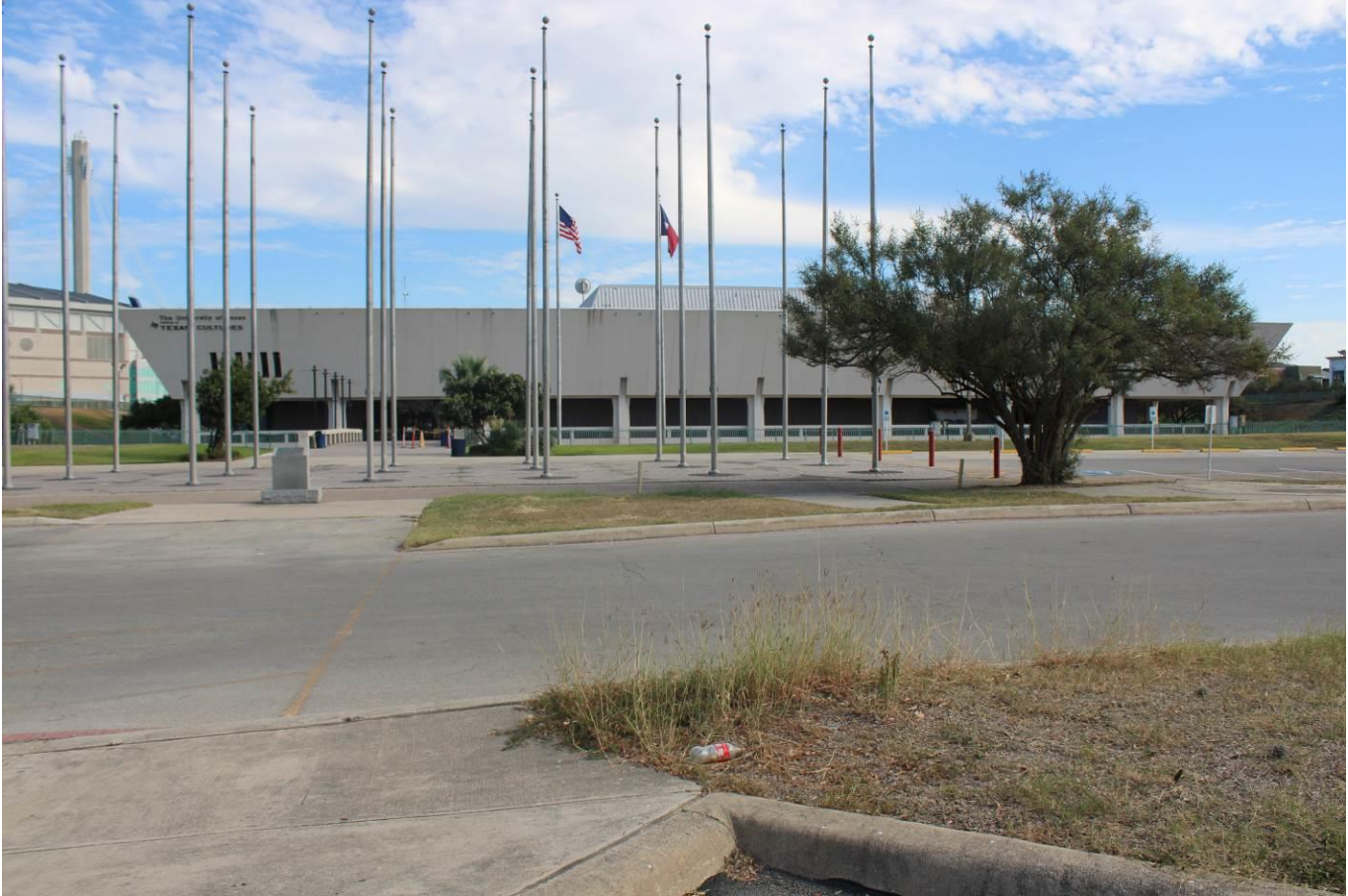
Photo 6 ITC facade with berms on both sides, camera facing southeast
