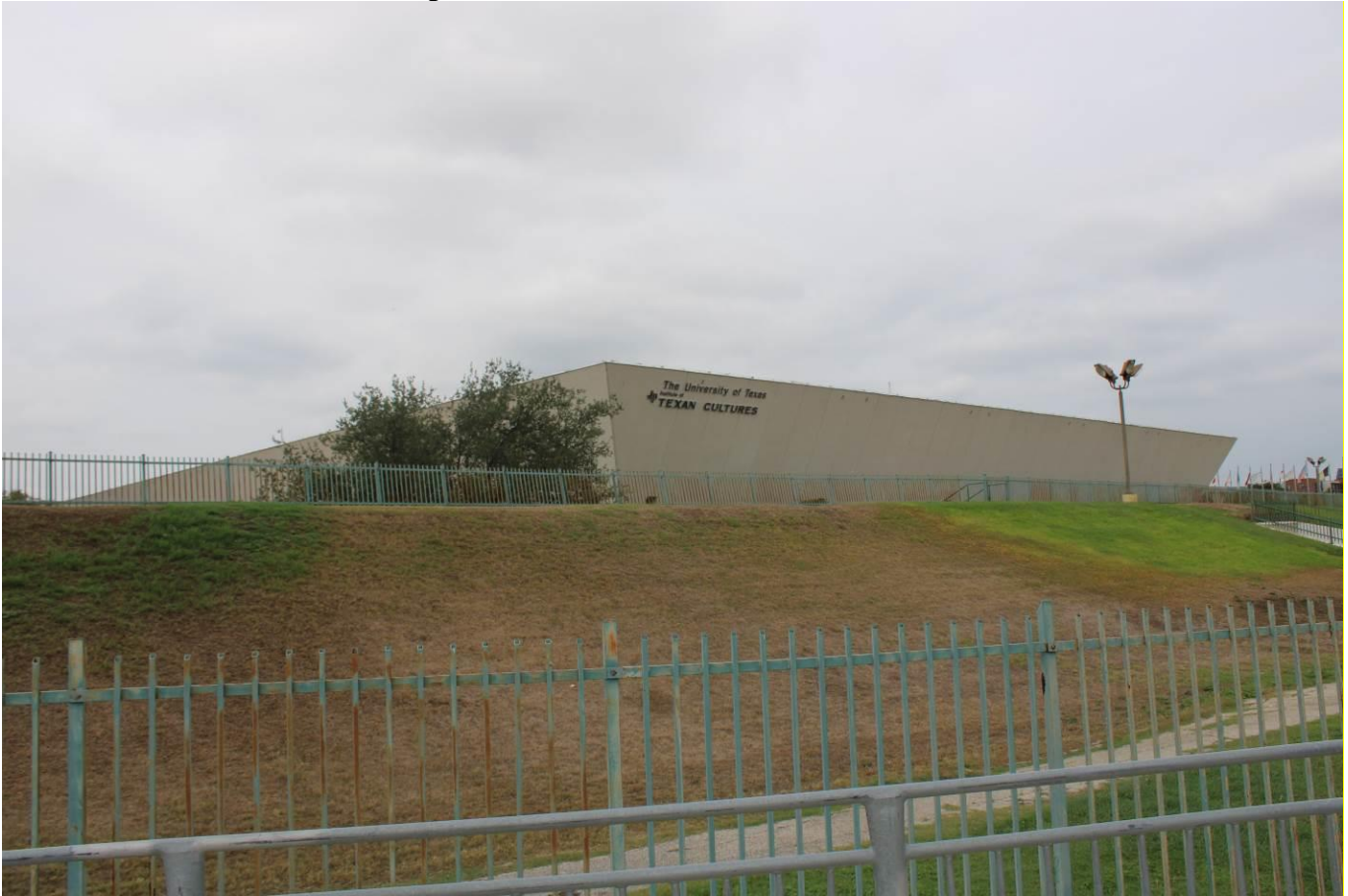
Photo 10 Northeastern elevation, camera facing southeast
