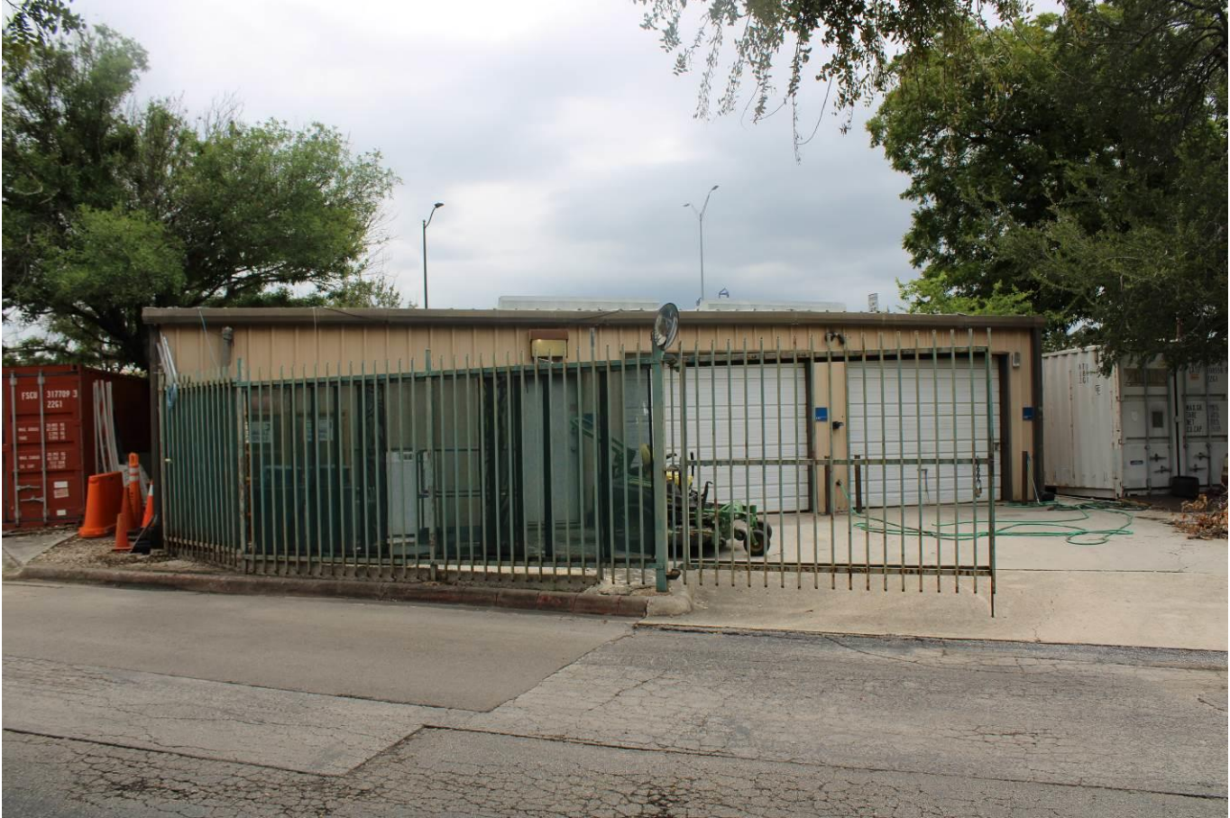
Photo 35 Storage building, camera facing east
