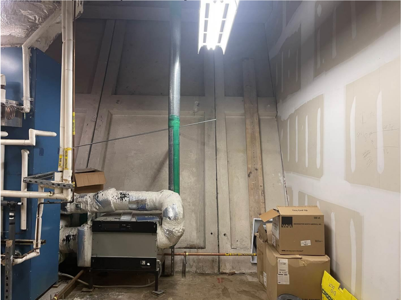
Photo 23 Third floor interior space between panels and building frame.
