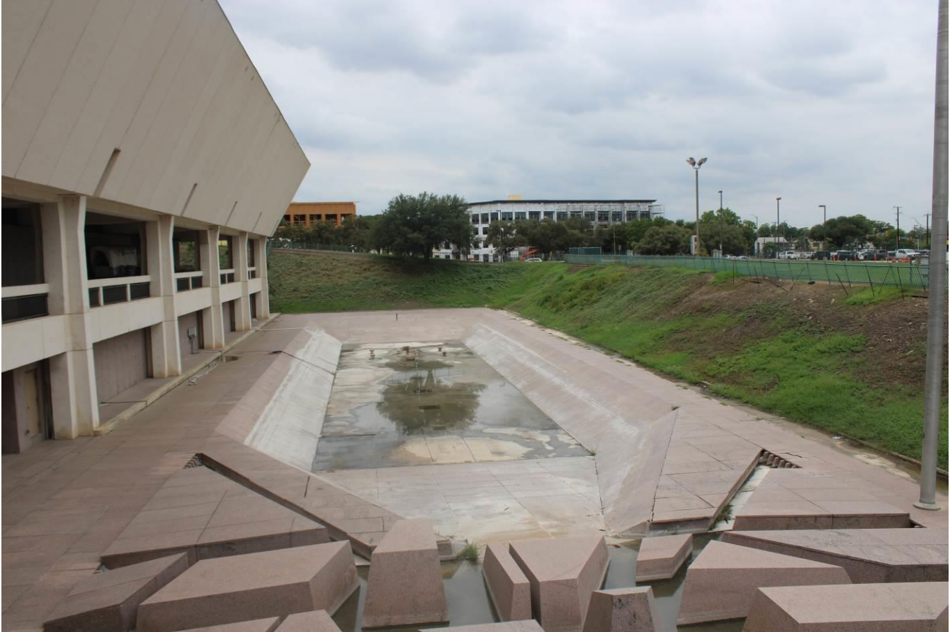
Photo 26 Fountain, camera facing southwest
