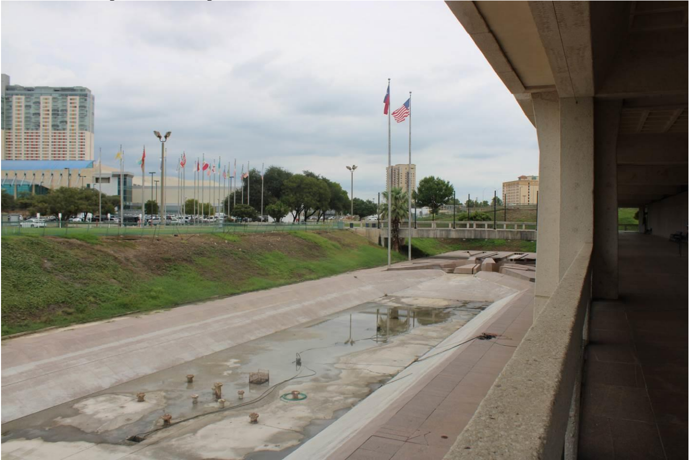
Photo 7 Fountain and Bridge, camera facing north
