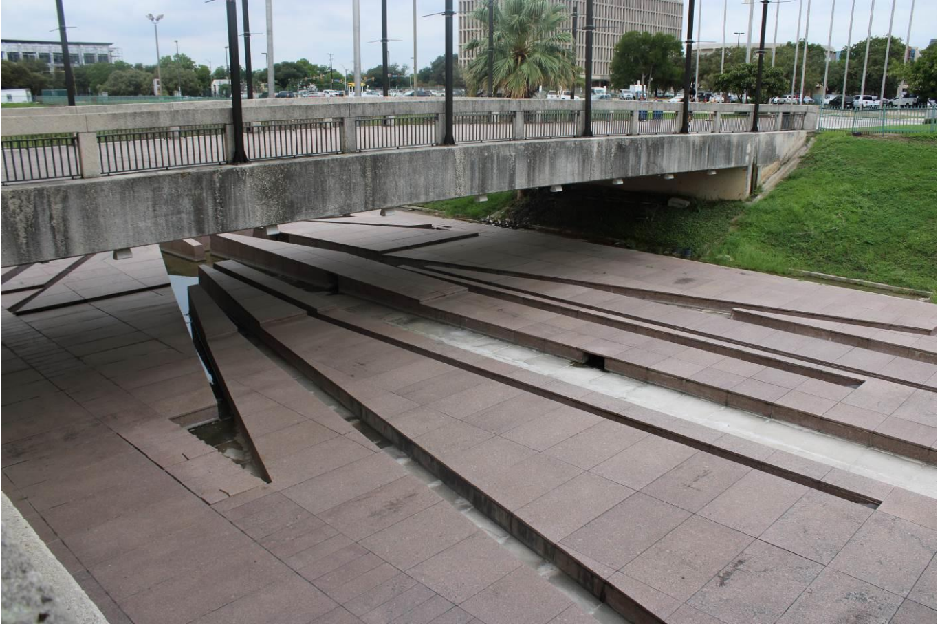
Photo 8 Bridge and water feature, camera facing southeast
