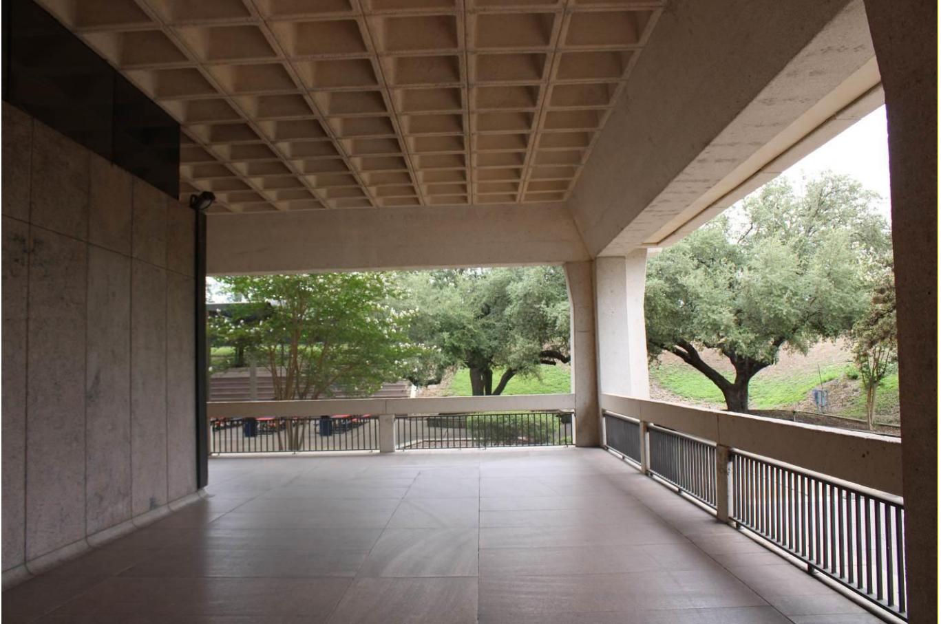
Photo 9 Waffle slab under third story, camera facing southwest
