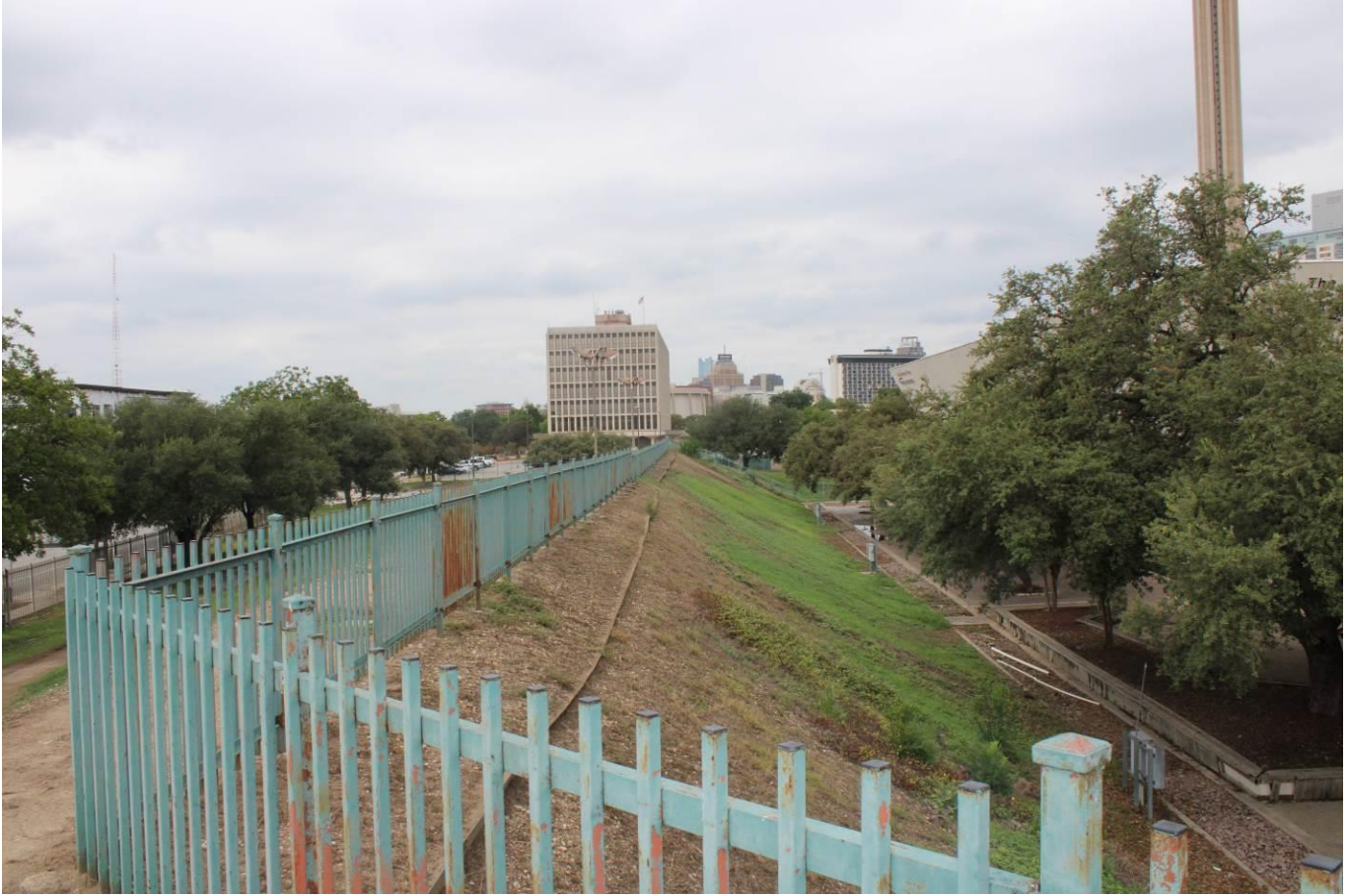
Photo 24 Fence on southwest berm, camera facing west
