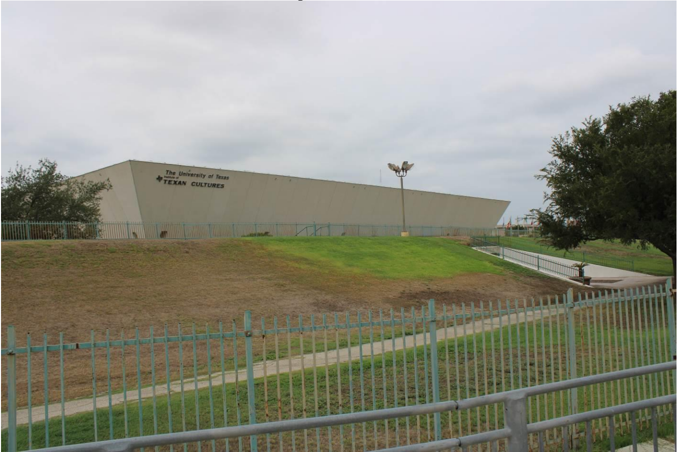
Photo 4 ITC northeastern elevation and berm, camera facing southwest
