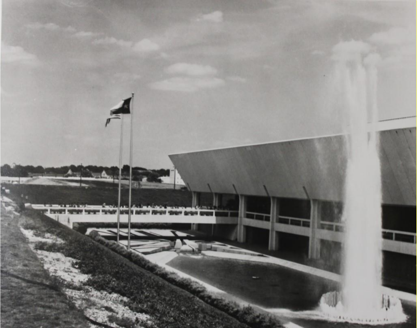
Figure 7. ITC facade showing fountain and pool, sometime before 1976. Source: Institute of Texan Cultures, Special Collections, University of Texas San Antonio
