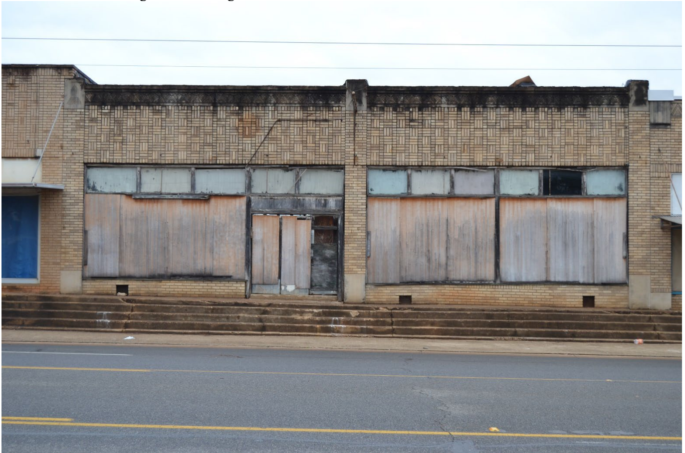
Photo 10. Camera facing north showing Resource 4 at 3717 West Marshall Avenue.
