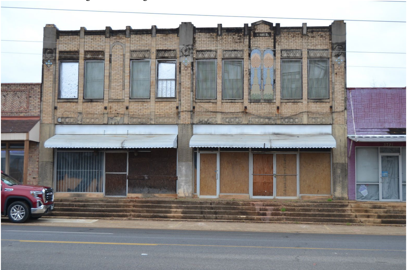
Photo 6. Camera facing north showing Resource 1 at 3725 West Marshall Avenue.
