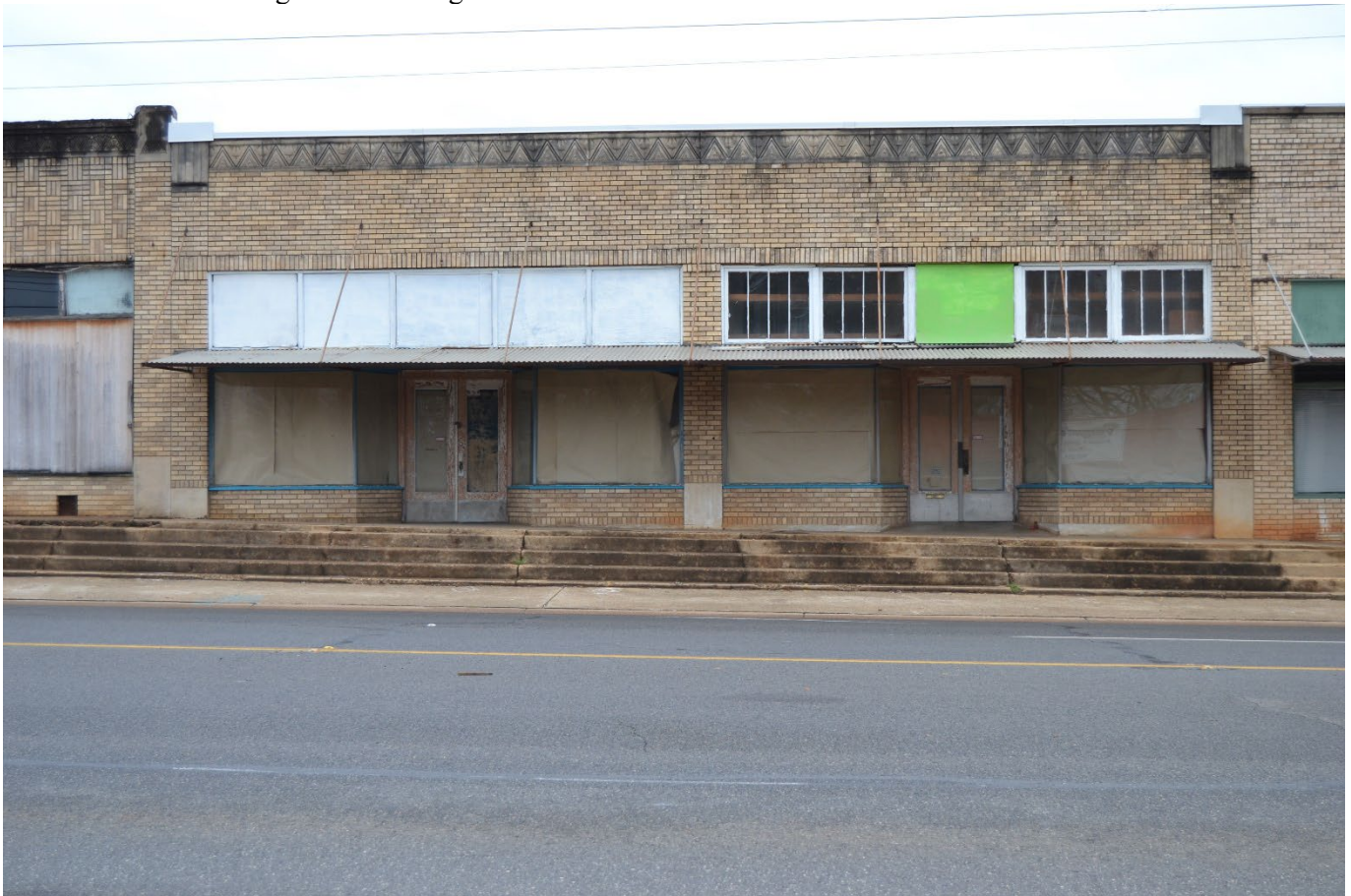
Photo 11. Camera facing north showing Resource 5 at 3713 West Marshall Avenue.
