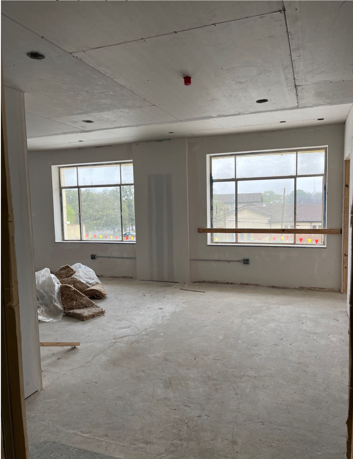
Photo 11: Montgomery County Hospital, Third Floor Patient Room, 1954 Addition, View North.
