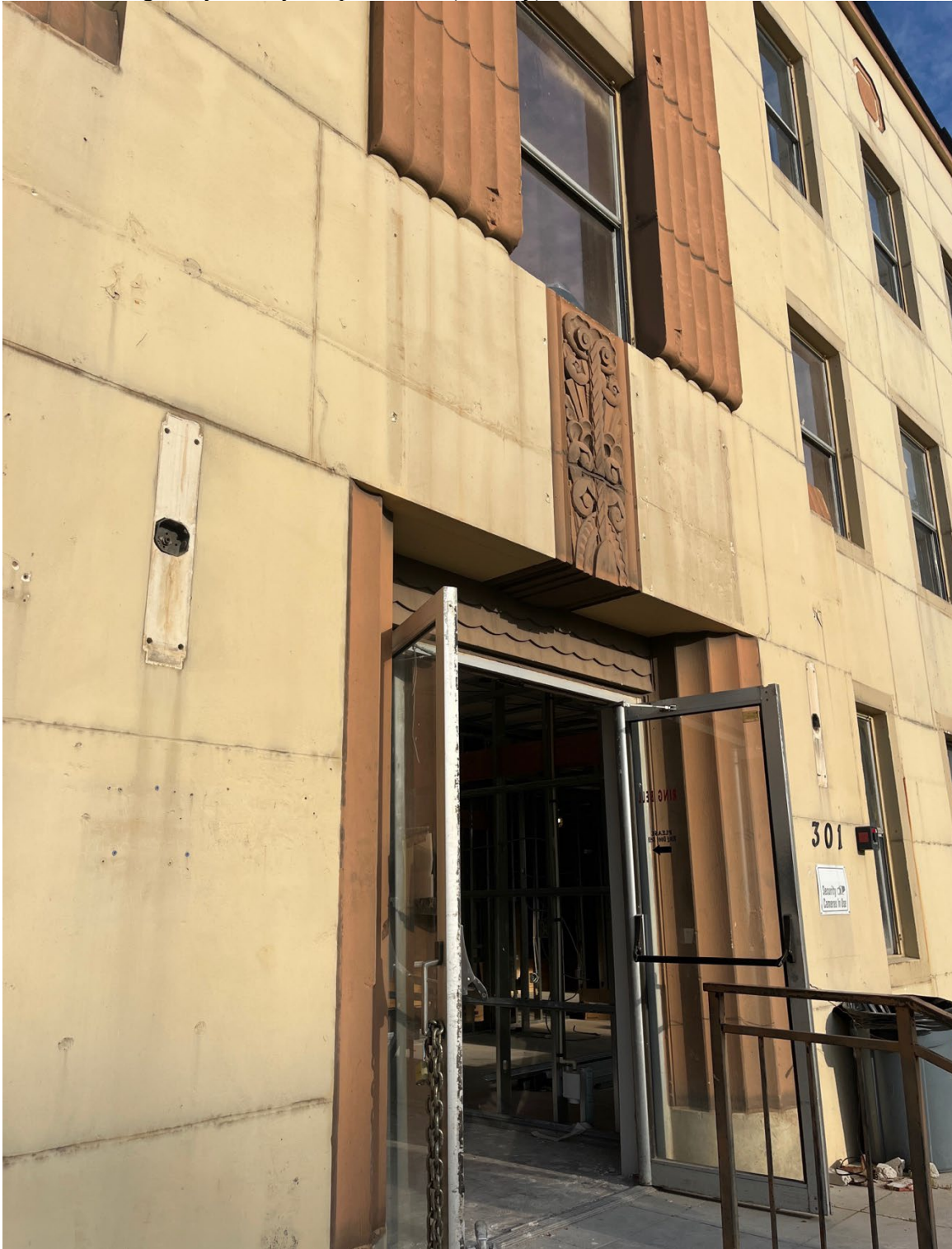
Photo 3: Montgomery County Hospital, West (Primary) Elevation entrance detail view.
