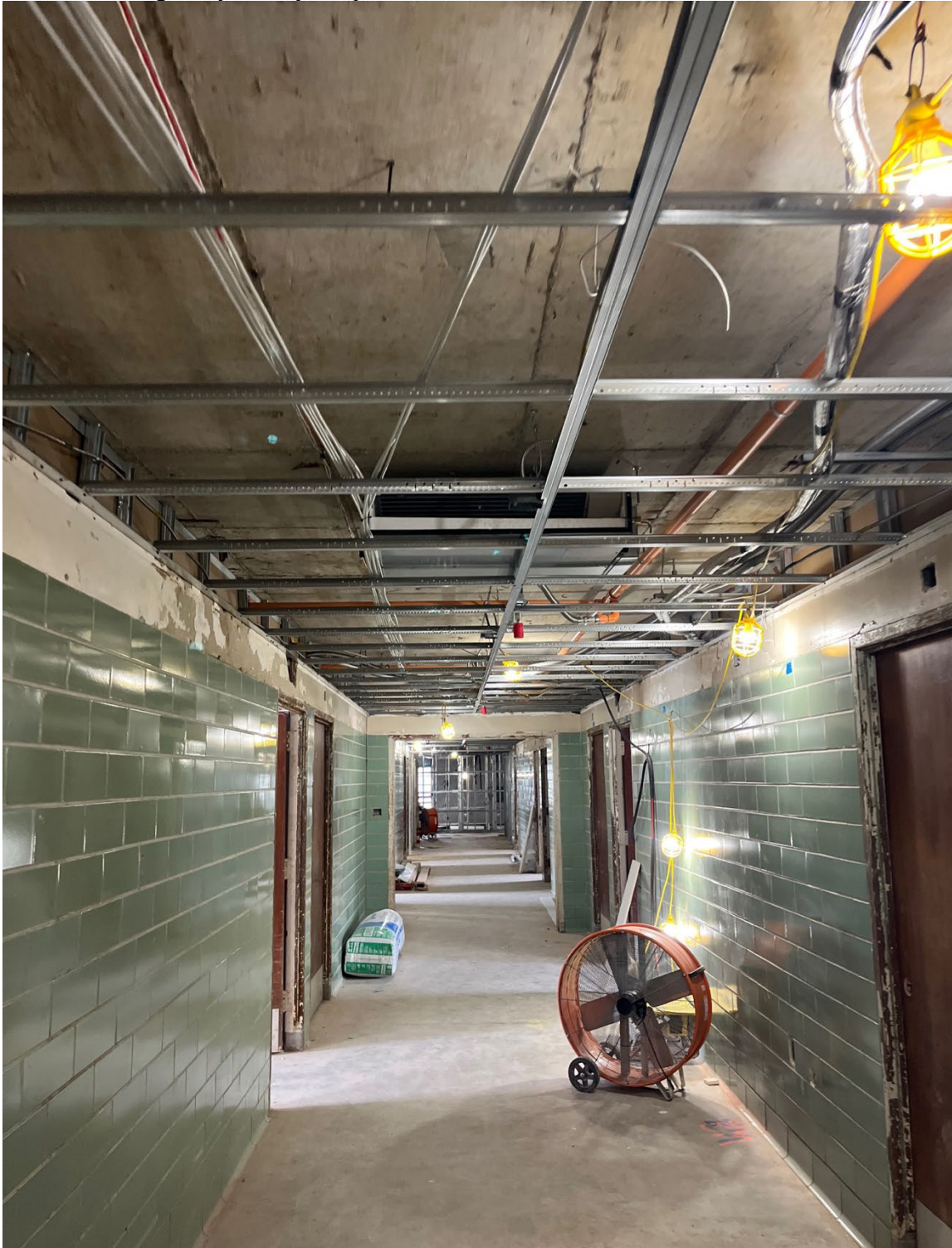
Photo 10: Montgomery County Hospital, Second Floor Corridor, 1954 Addition, View East.
