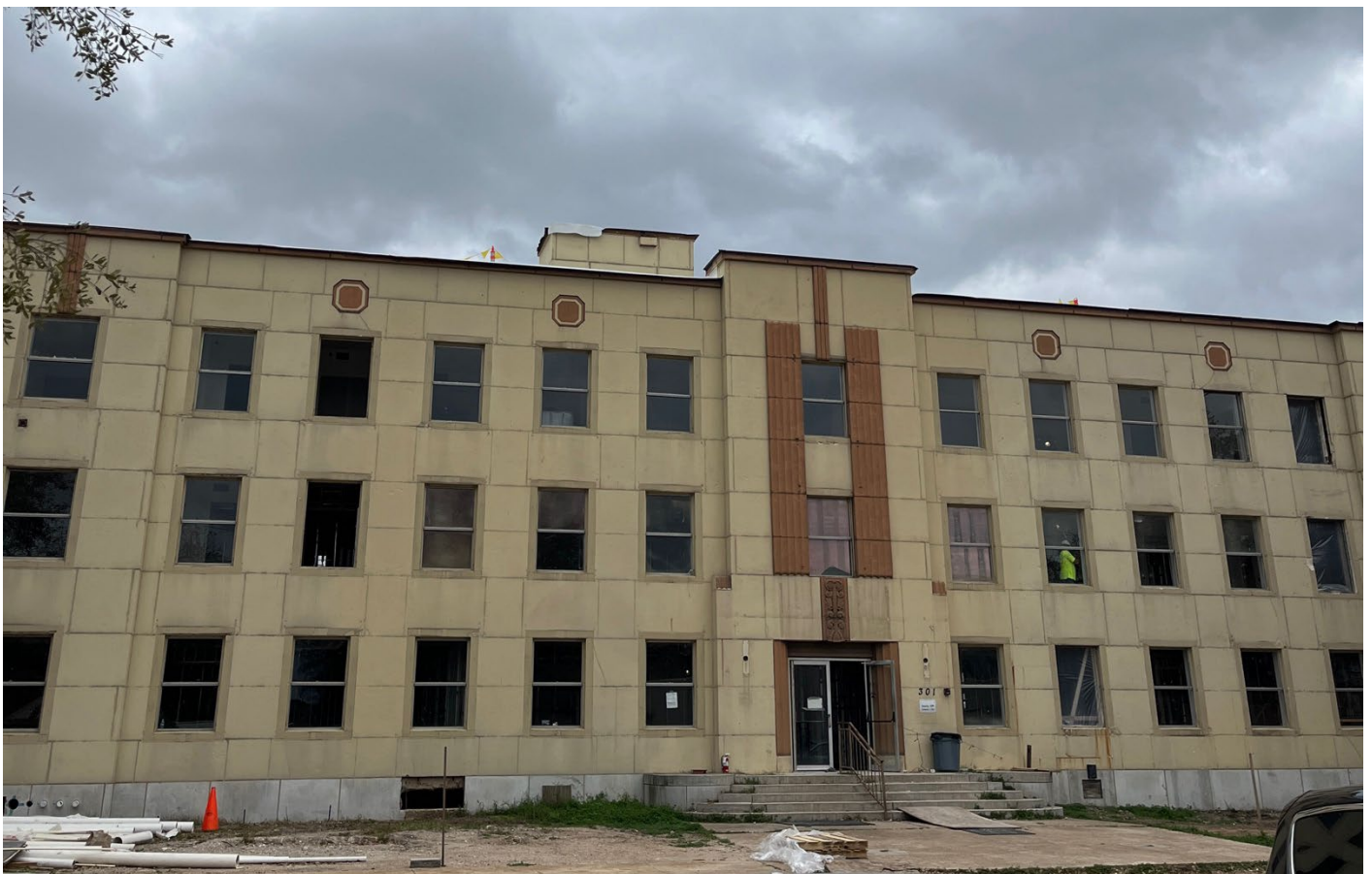
Photo 1: Montgomery County Hospital, Primary (West) Elevation. View East.
