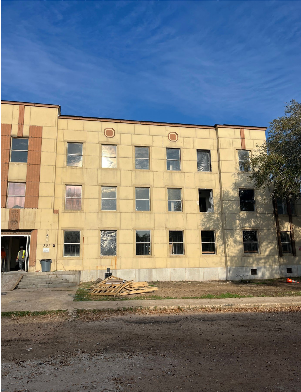
Photo 2: Montgomery County Hospital, West (Primary) Elevation, looking northeast.
