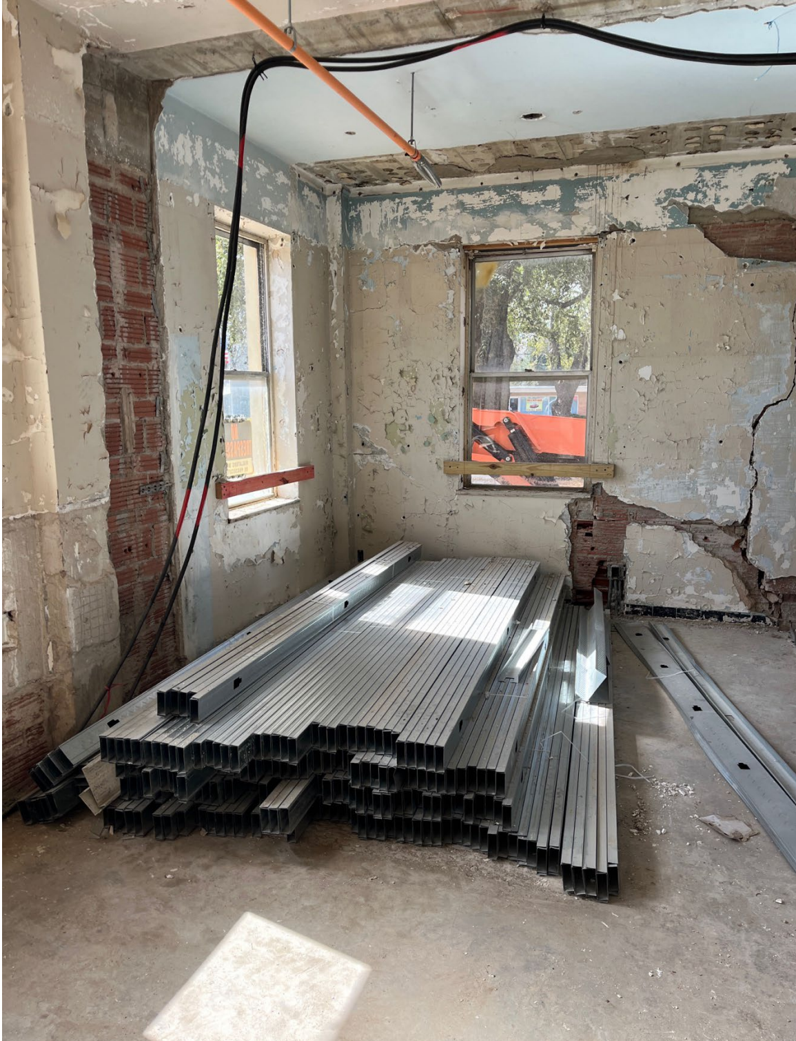
Photo 9: Montgomery County Hospital, First Floor Sunroom, 1938 wing, View West.
