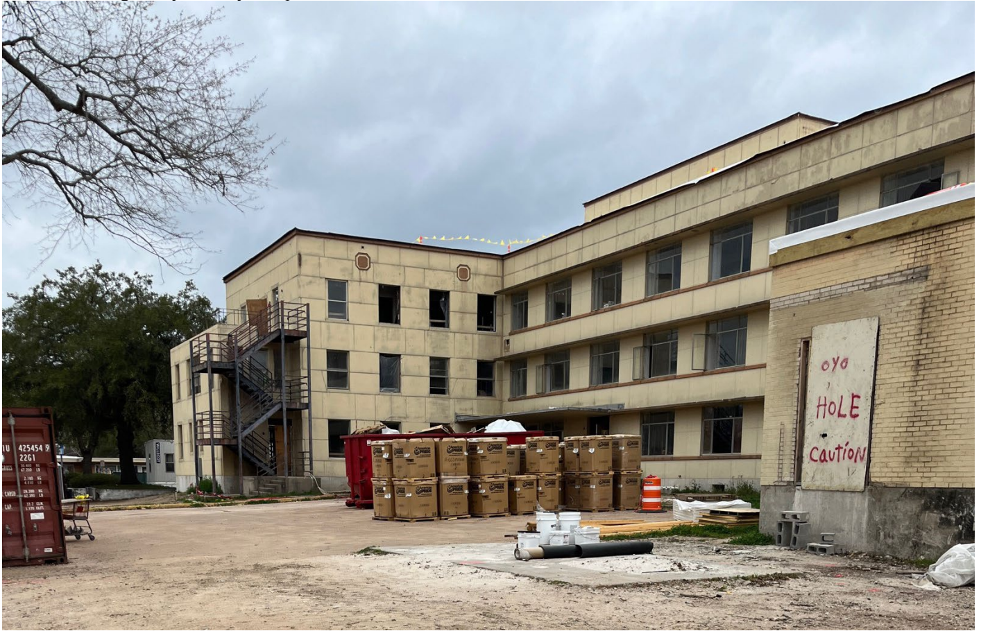
Photo 5: Montgomery County Hospital, South Elevation, View Northwest.
