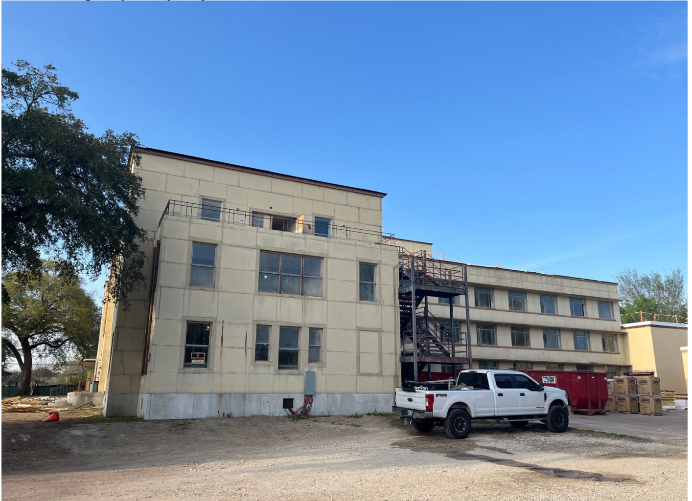
Photo 4: Montgomery County Hospital, South Elevation, View Northeast.
