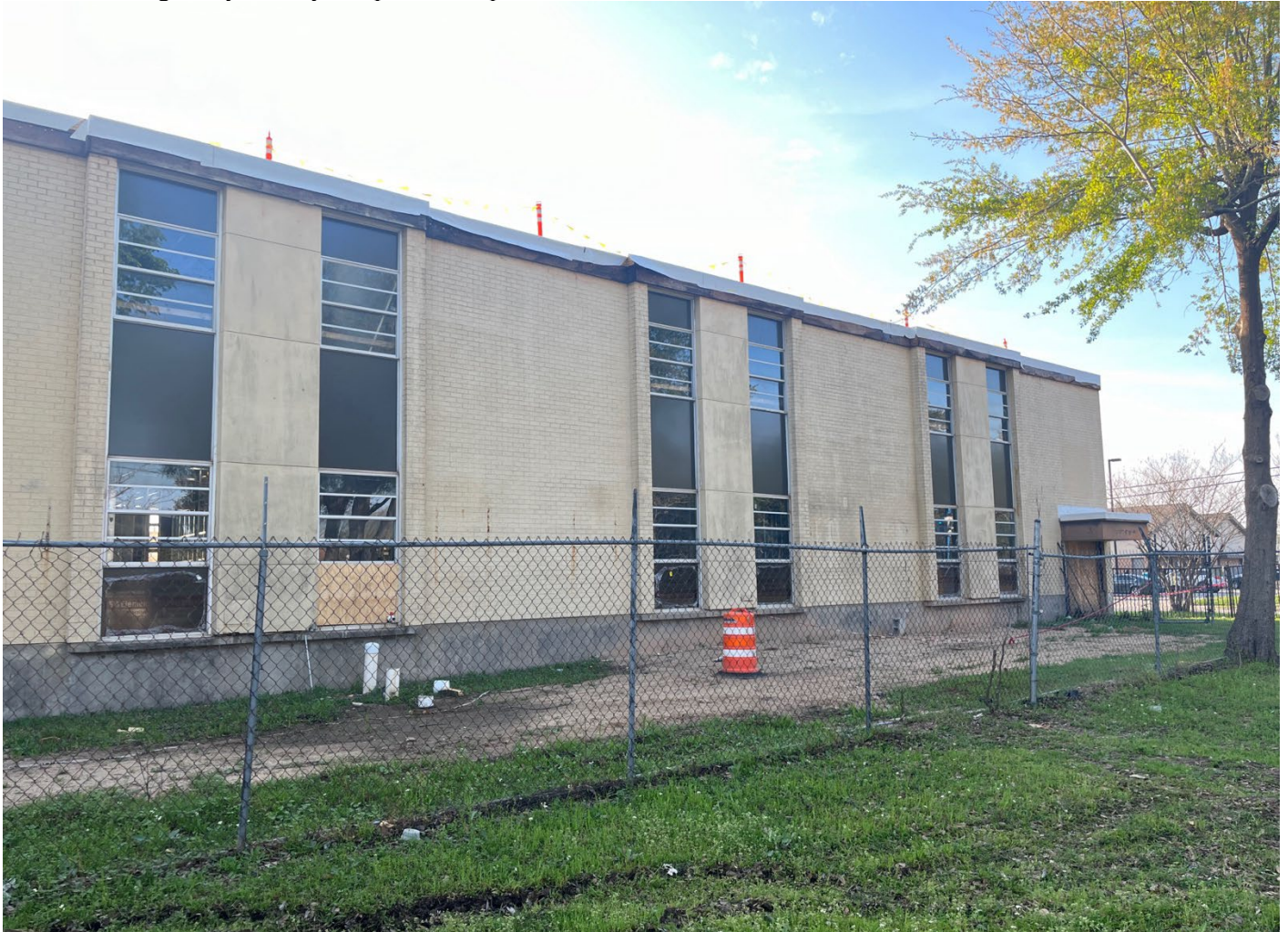
Photo 7: Montgomery County Hospital, Oblique, East Elevation. View Northwest.
