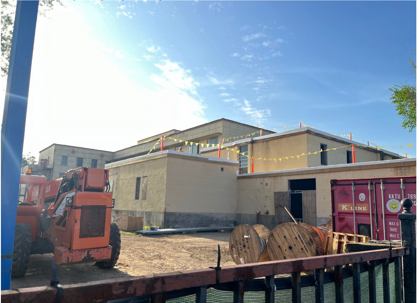
Photo 6: Montgomery County Hospital, Oblique, South and East Elevations. View Northwest.
