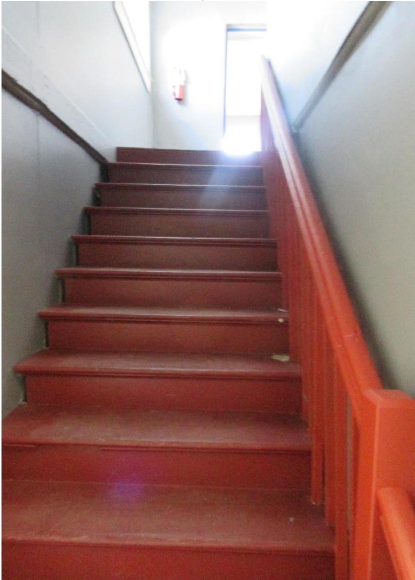
Photo 17: Staircase to second story, view southeast.
