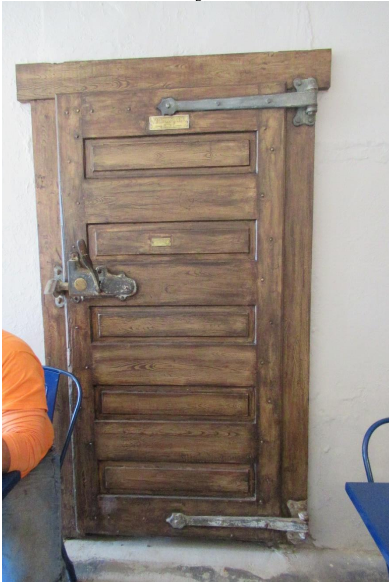
Photo 16: Detail of restored refrigerated door in 1925 Meat Market ground floor, view northwest.
