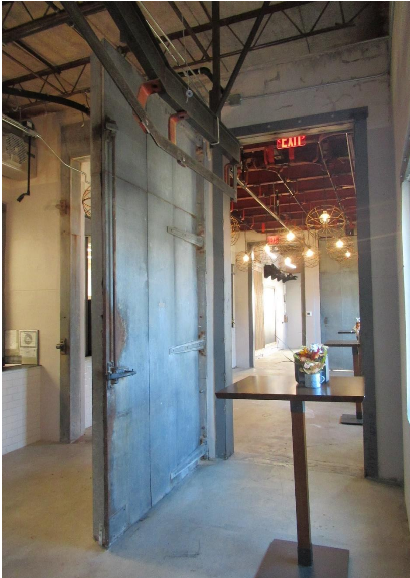
Photo 15: Interior view of c. 1970 meat processing addition showing retained refrigerator doors and overhead meat processing equipment. View northeast.
