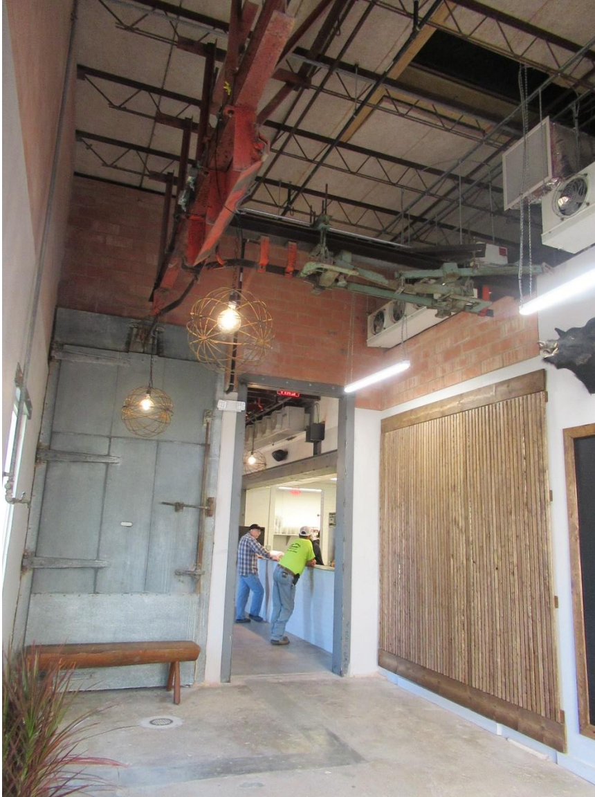
Photo 14: Interior view of c. 1970 meat processing addition showing retained refrigerator doors and overhead meat processing equipment. View west.
