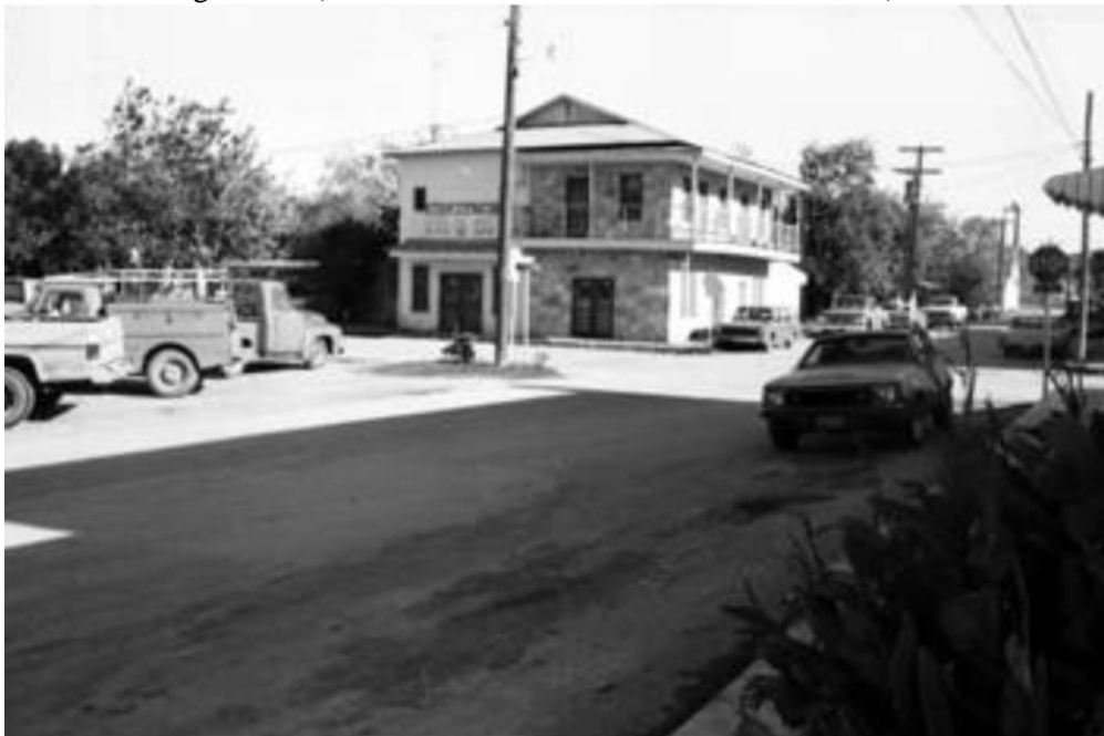
Figure 10: Southwest view from Paris Street across from Houston Square after roof was reconstructed with Dutch gable and central ridge, 1977 (Source: Castroville Chamber of Commerce).
