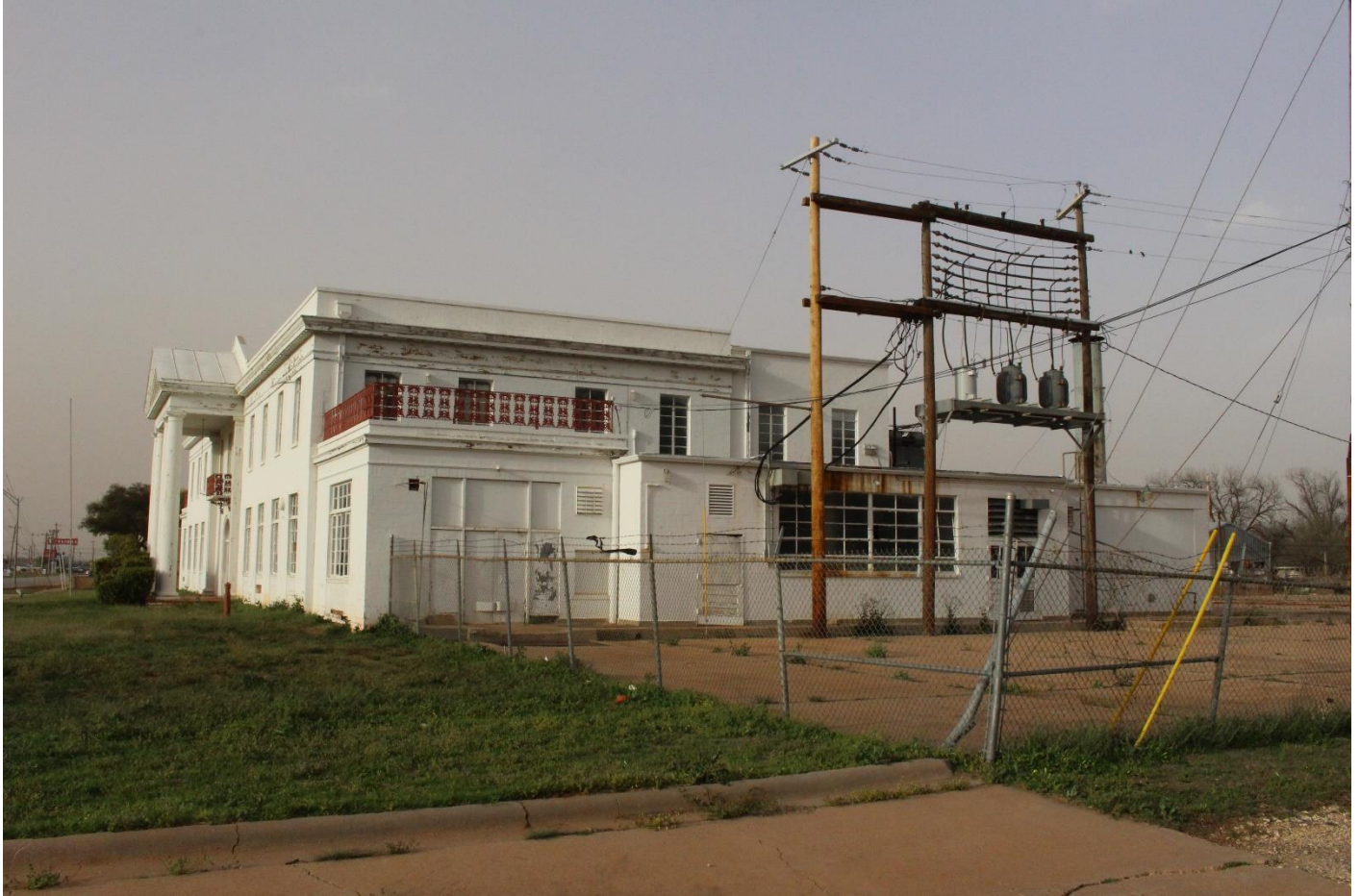
Photo 7. Borden Company south elevation, looking north.
