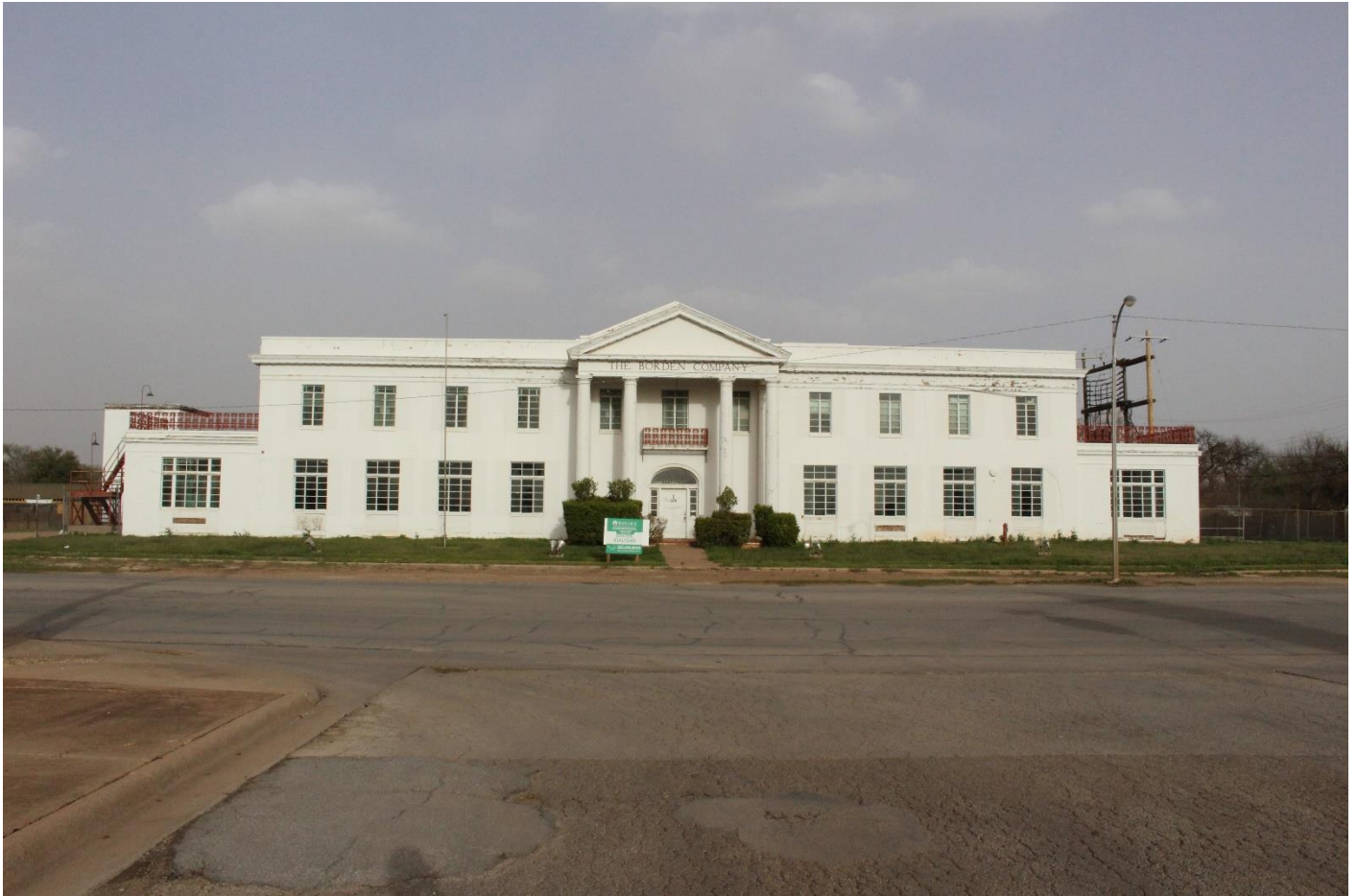
Photo 2. Borden Company façade (west elevation), looking east.
