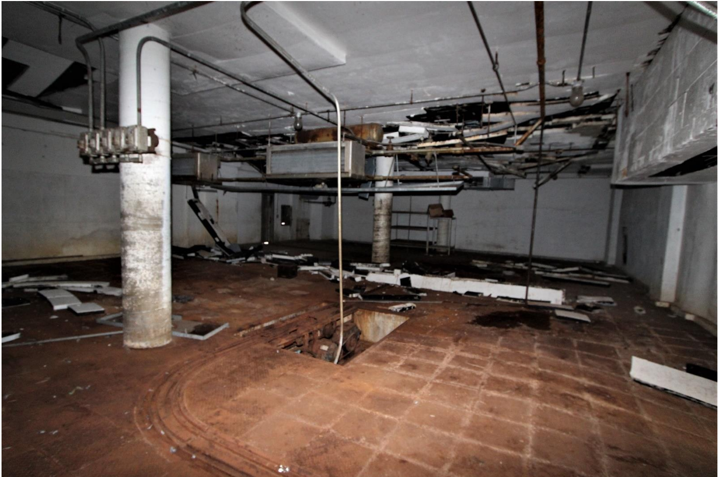
Photo 23. Borden Company, First Floor, Cold Storage Room, looking south.
