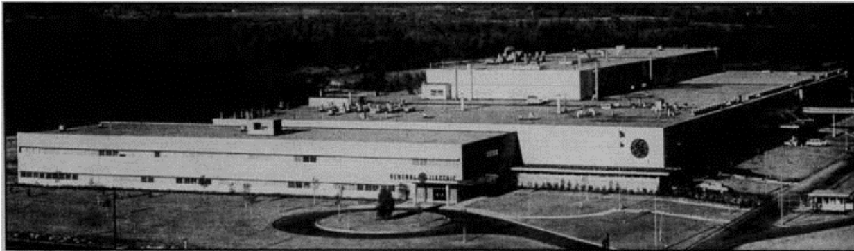
Figure 10: Texas Plants Designed by Walter Kidde. Top: General Electric, Tyler, Texas (GE Plant Heats Economy with Air-Conditioning Plant," Abilene Reporter-News , January 1, 2000, 104.) Bottom: Ethicon, San Angelo, Texas. ("Even More Things You Didn't Know About J&J," Kilmer House , accessed on June 1, 2023, https://www.kilmerhouse.com/2010/05/even-more-things-you-didnt-know-about-jj .)
