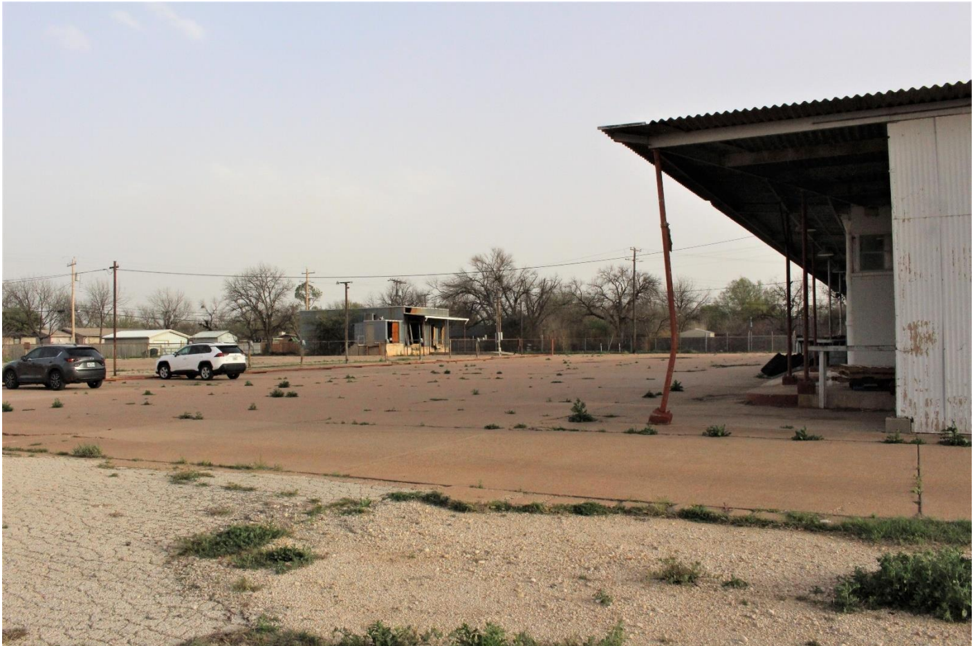
Photo 12. View of ca. 1973 cold storage building, looking southeast.
