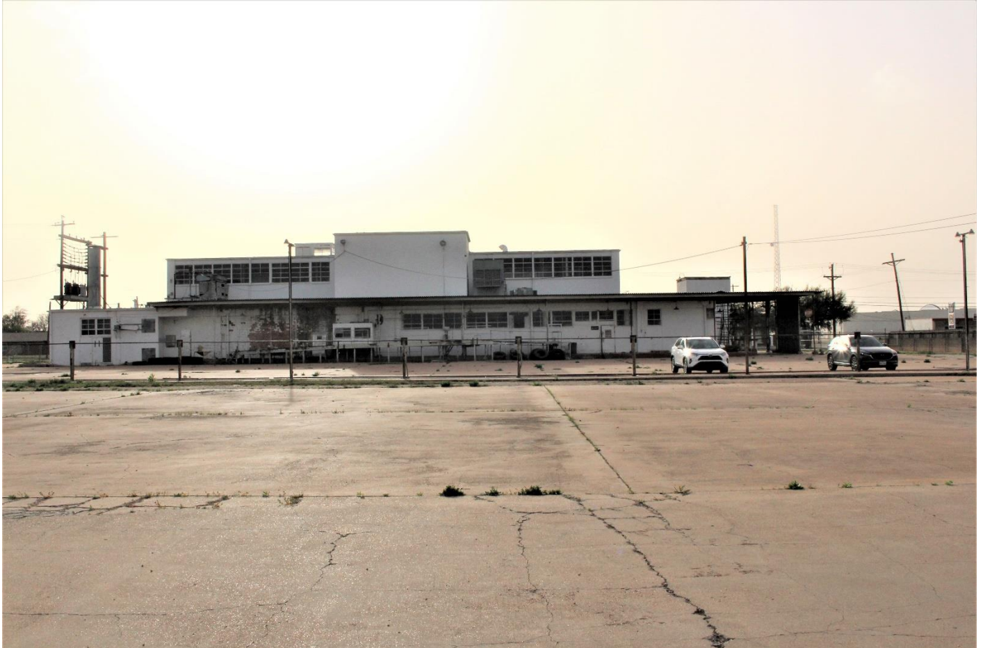
Photo 9. Borden Company rear elevation, looking west.
