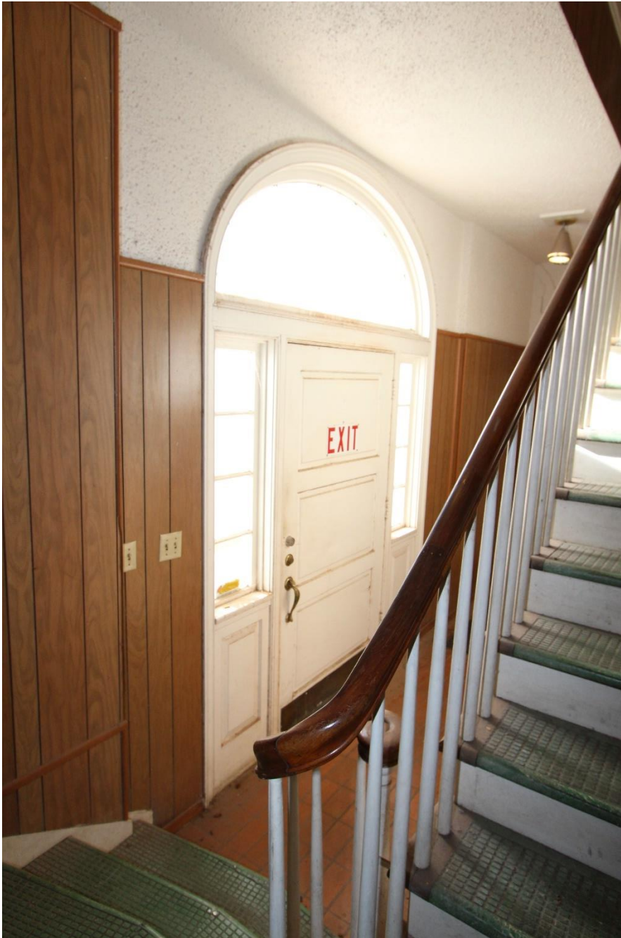
Photo 19. Borden Company, First Floor, Interior Front Staircase, looking northwest.
