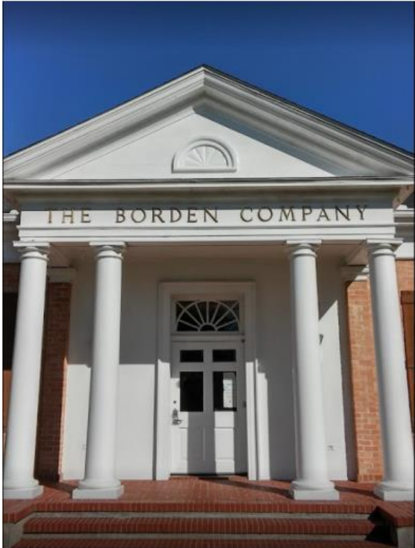
Figure 24: Borden Plant in Lafayette, LA. Built in 1966. (Google Maps, 2023.)
