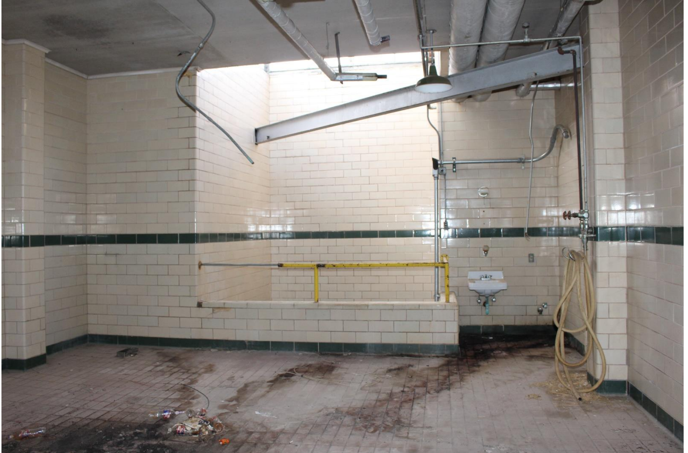
Photo 27. Borden Company, Second Floor, Milk Room, looking northeast.
