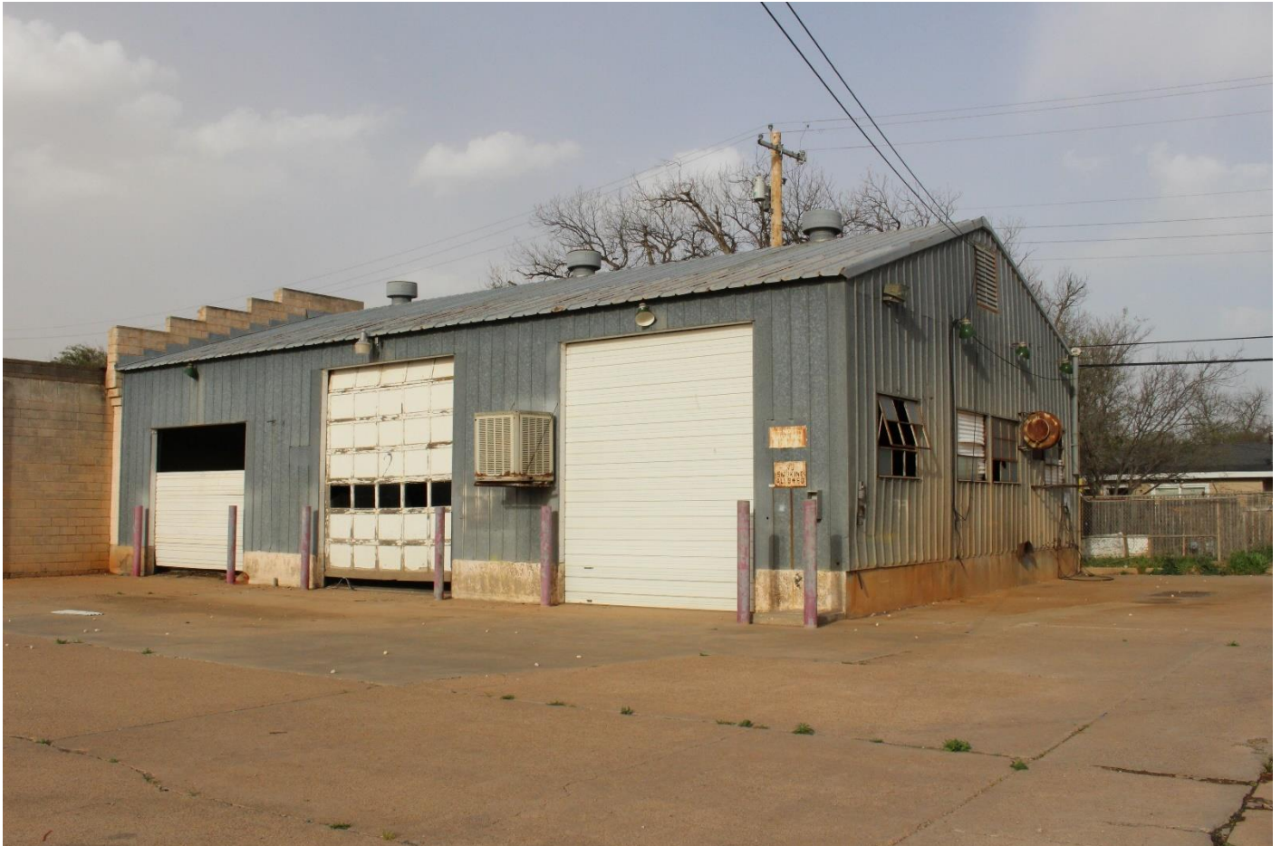
Photo 13. Garage facade, looking northeast.
