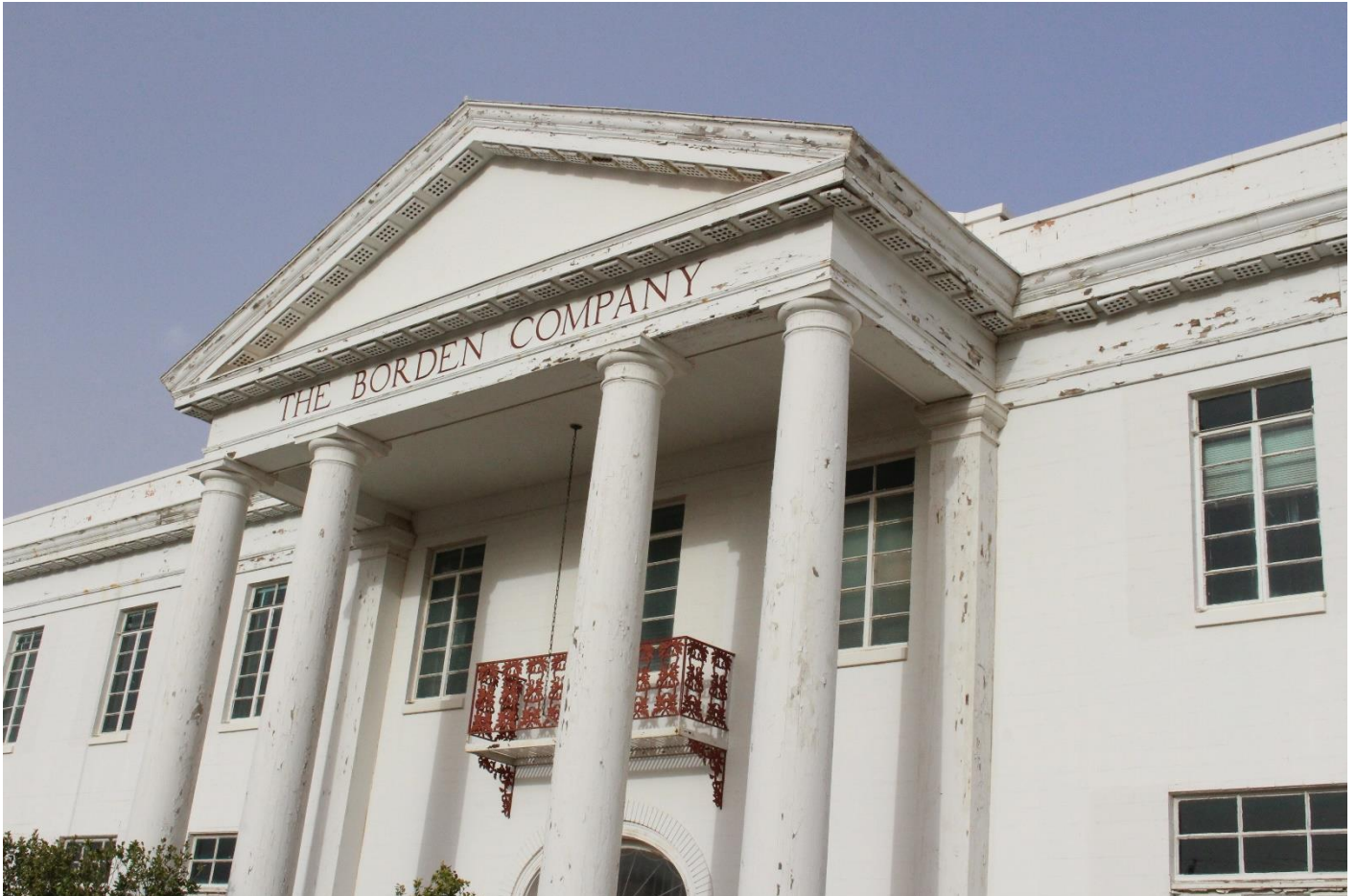
Photo 4. Borden Company façade (west elevation), looking northeast.
