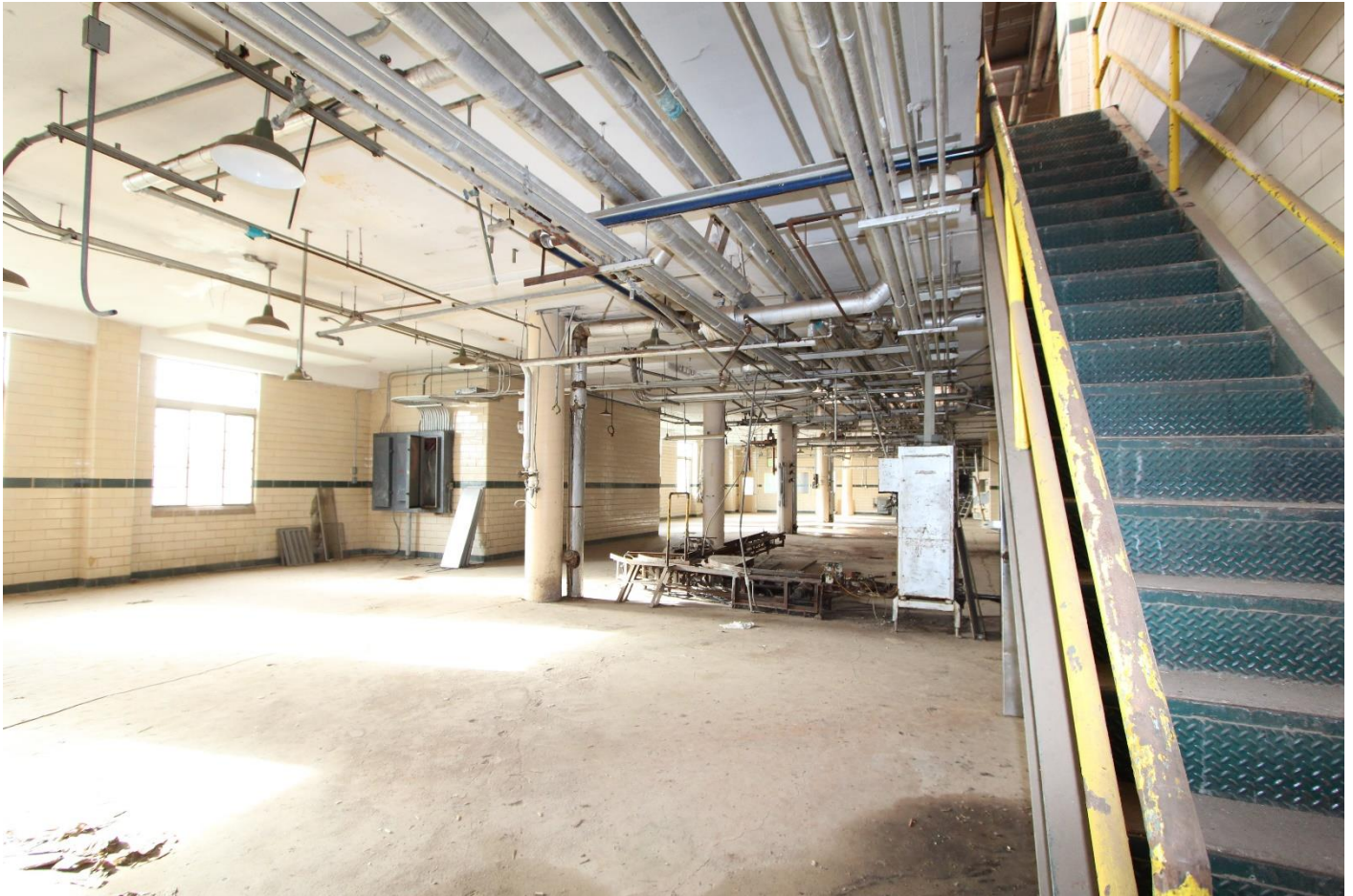
Photo 26. Borden Company, First Floor, Possible Bottle/Carton Room, looking north.
