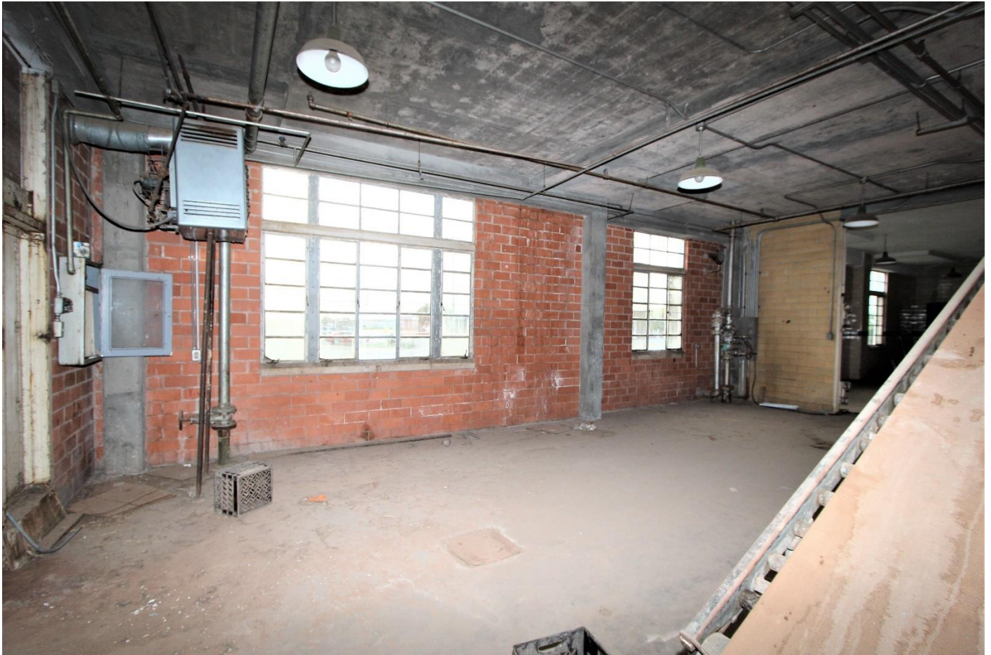
Photo 25. Borden Company, First Floor, Southwest Room, looking northwest.
