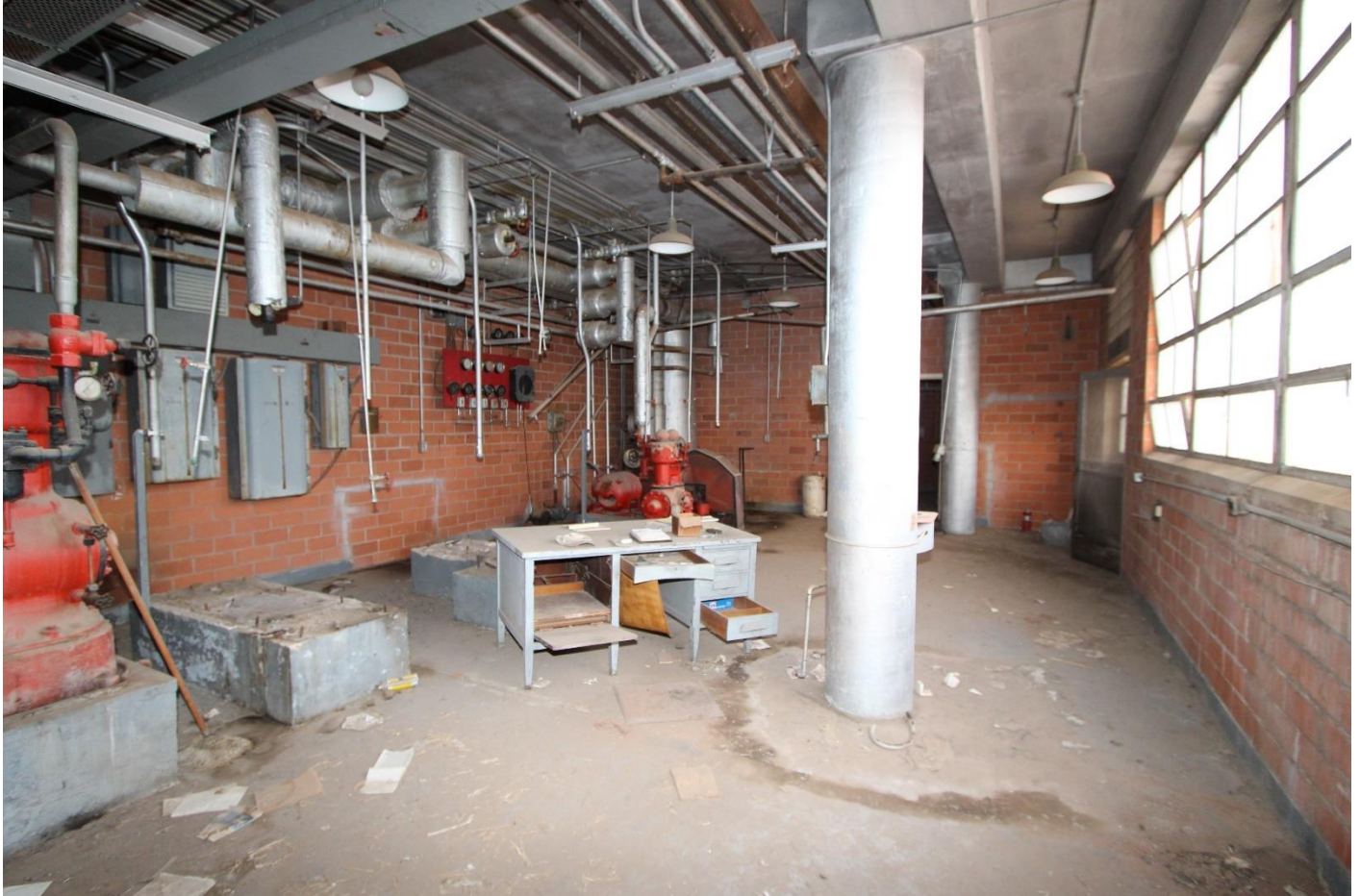
Photo 24. Borden Company, First Floor, Engine Room, looking east.
