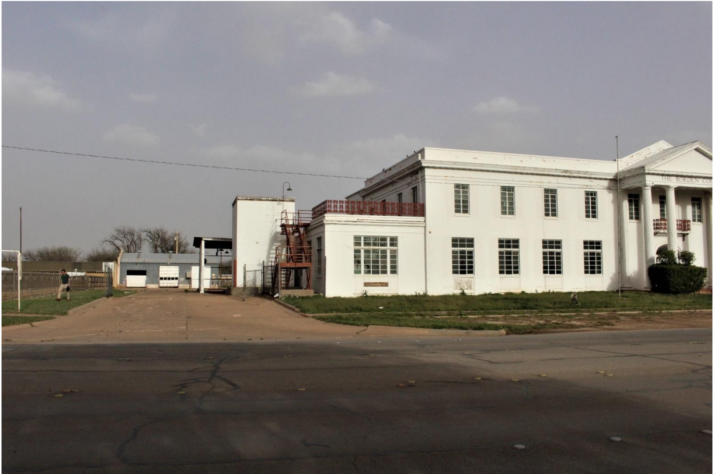
Photo 16. Borden Company façade (west elevation) and north elevation, looking east.
