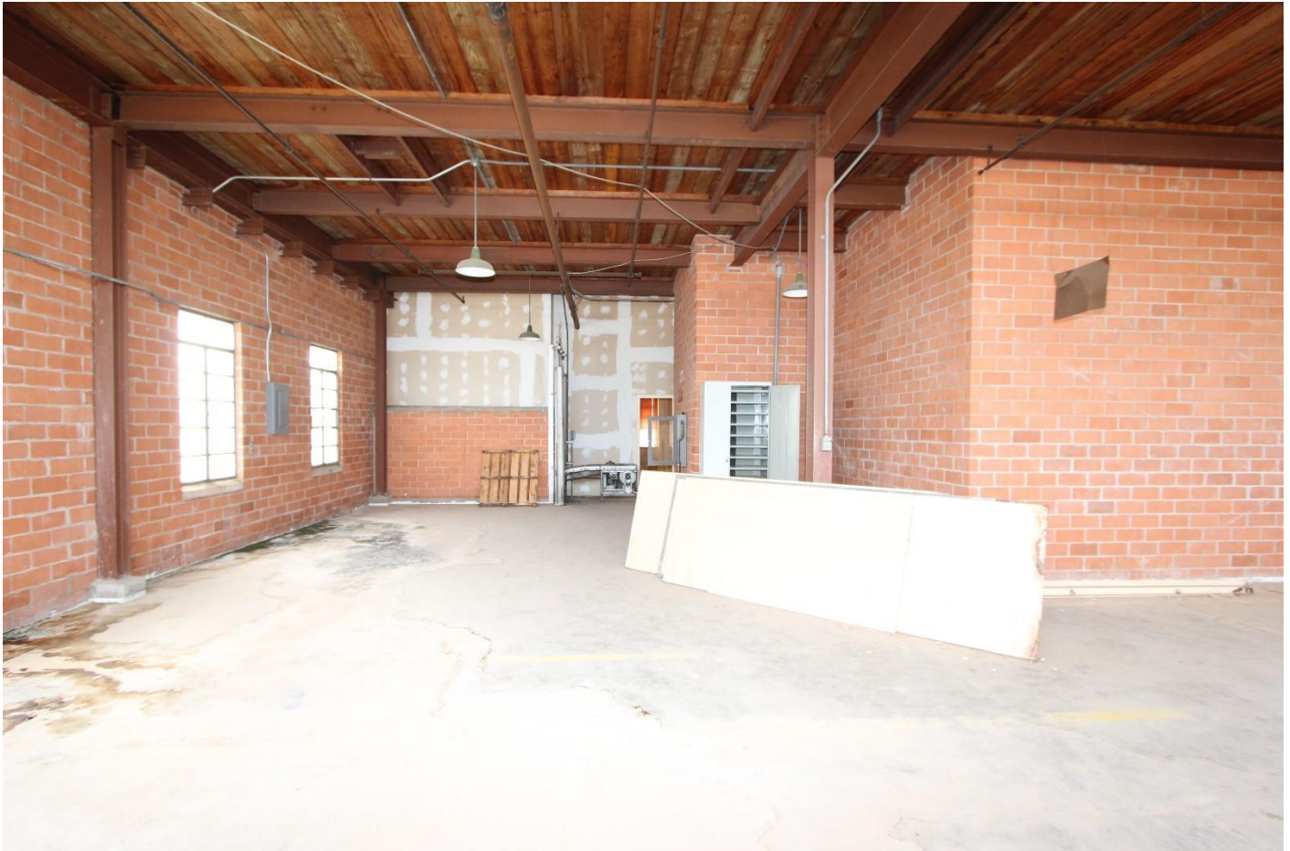
Photo 28. Borden Company, Second Floor, Southeast corner looking west.
