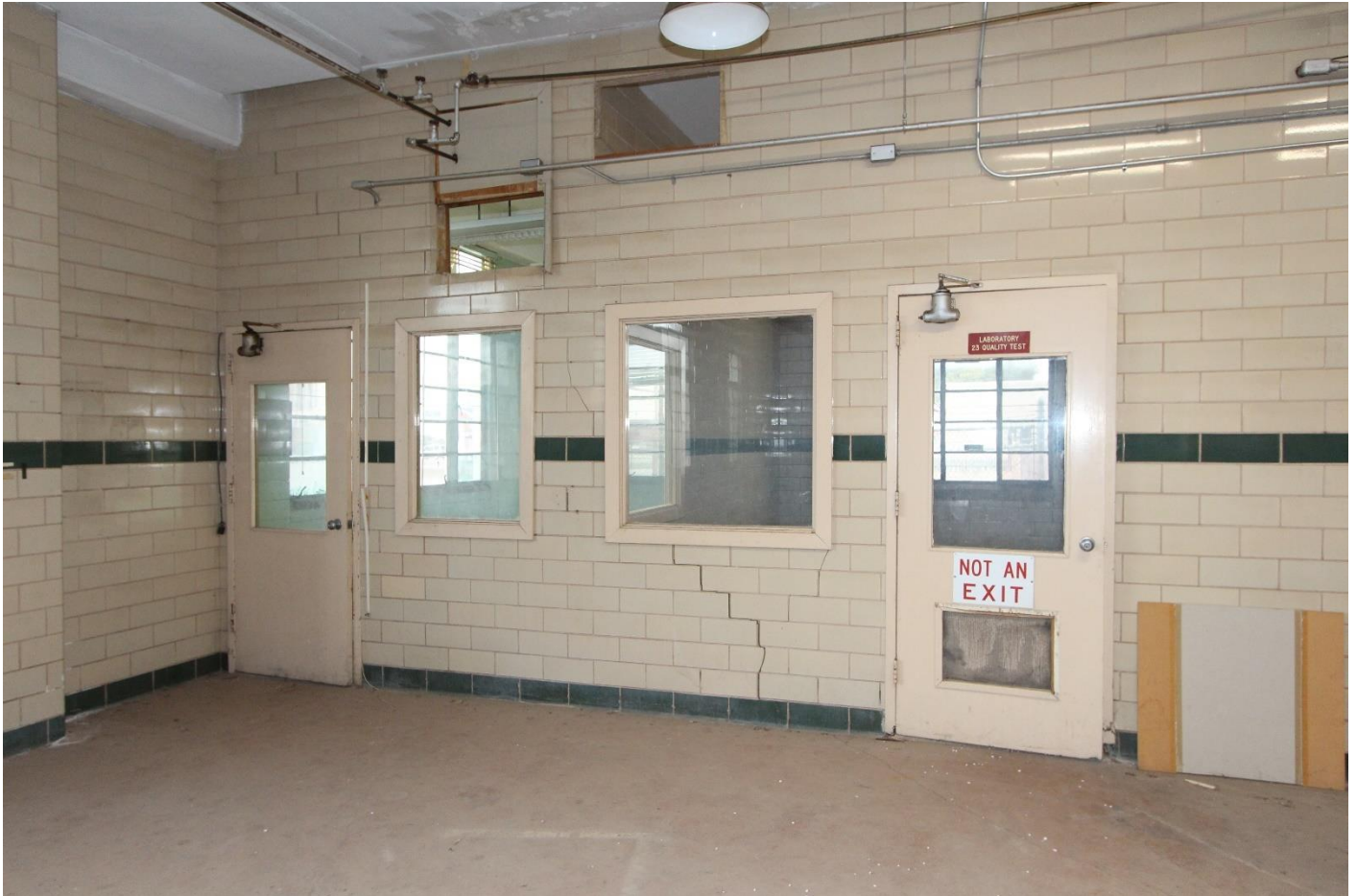
Photo 21. Borden Company, First Floor, Laboratory, looking north.
