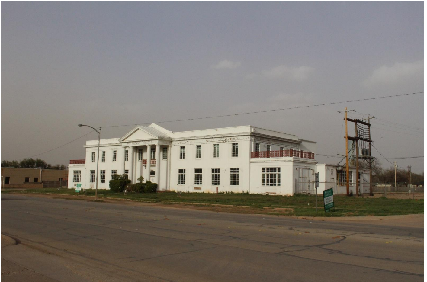
Photo 3. Borden Company façade (west elevation), looking northeast.
