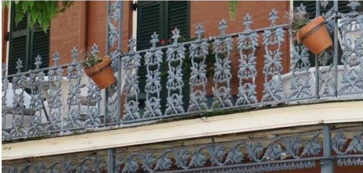
Figure 20: Historic Oak Leaf Patter Cast Iron. Top: LaBranche House, ca. 1840, New Orleans, LA. (Morgan Randall, "Discover the Hidden Histories Told by the French Quarter's Balconies," 2017, accessed 2023. https://www.atlasobscura.com/articles/ironwork-new-orleans-french-quarter-pontalba-adinkra . Bottom Left: Nominated Borden Plant in Abilene. (Deb Sheals, 2023.) Bottom Right: Railing on an 1800s house in Richmond, VA. (Richmond Iron, accessed 2023 https://richmondiron.com/1505-west-ave-cast-iron-porch-expansion/ )
