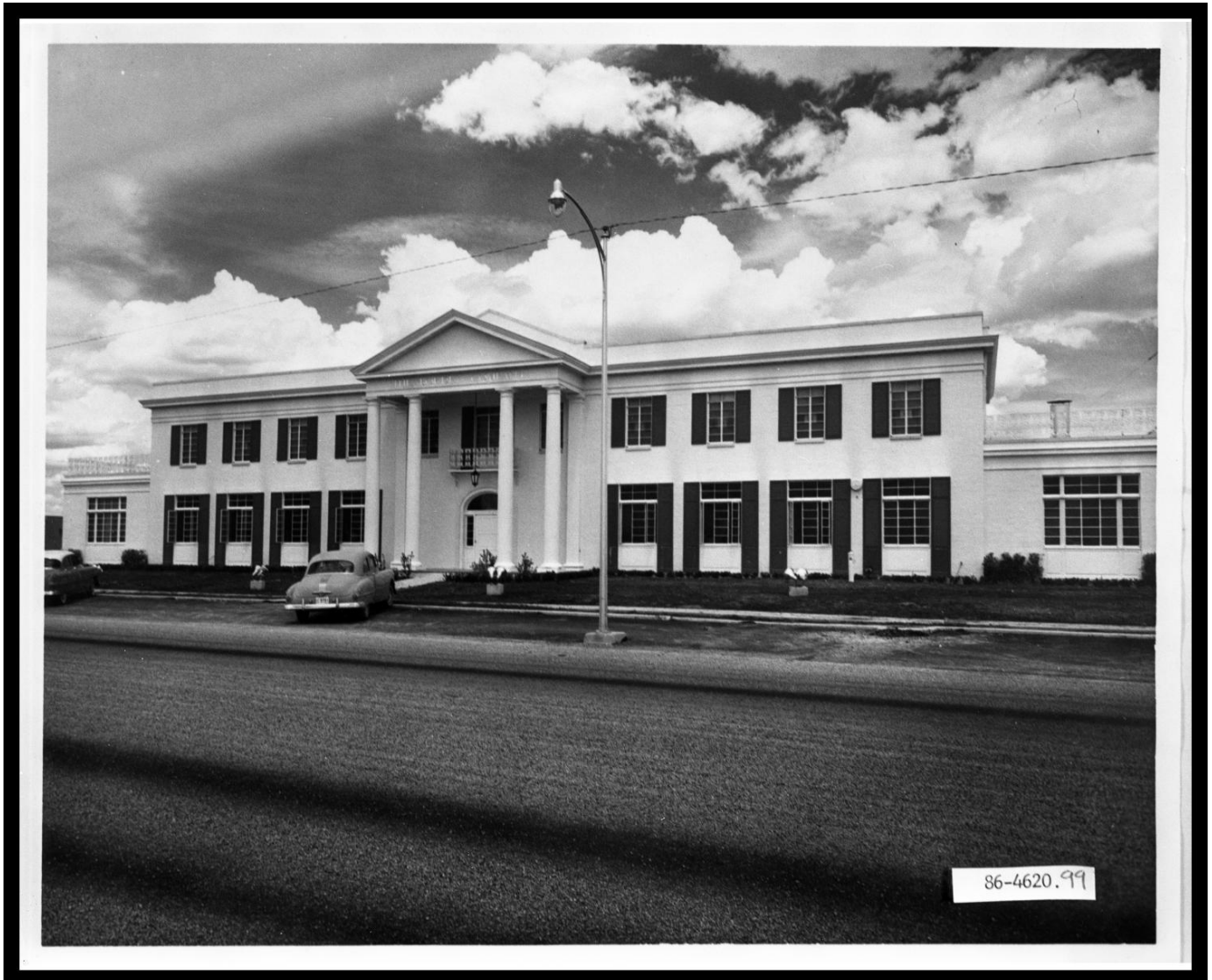
Figure 5: Borden Plant in Abilene, late 1950s or early 1960s. ("Borden Building," The Portal to Texas History , Accessed December 6, 2022, https://texashistory.unt.edu/ark:/67531/metaph55215/?q=borden%20abilene . crediting Hardin-Simmons University Library.)
