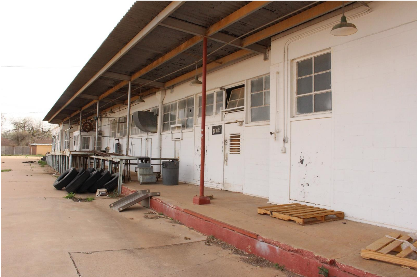
Photo 11. Borden Company rear elevation, looking southwest.
