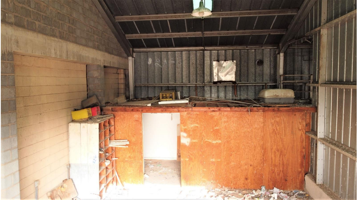
Photo 14. Garage interior, looking northeast.
