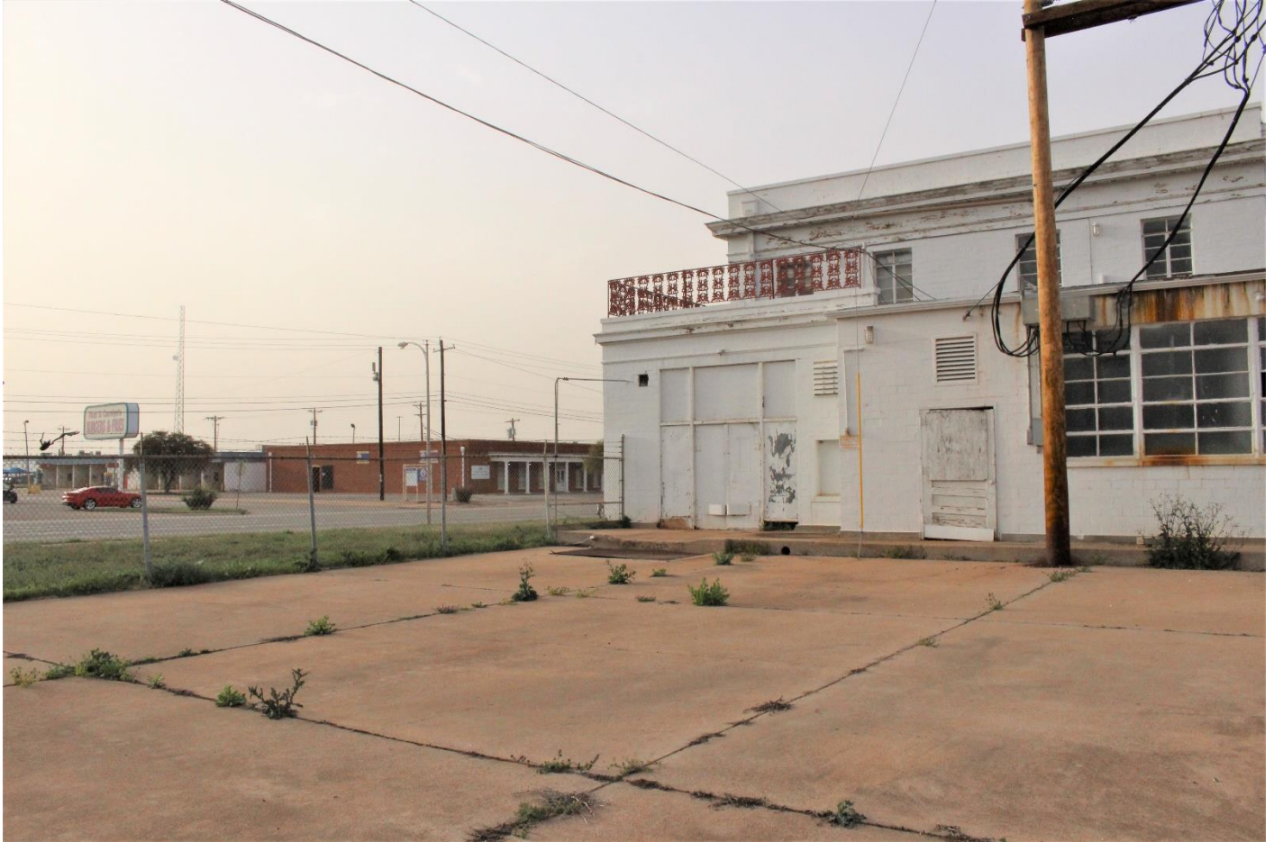
Photo 6. Borden Company south elevation, looking northwest.
