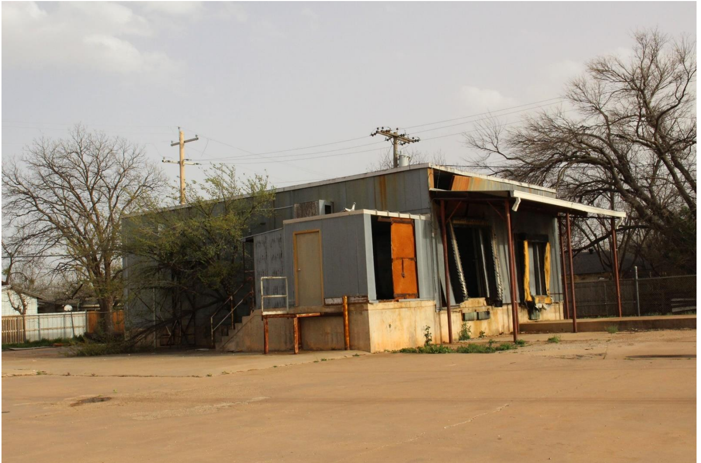
Photo 15. Cold Storage Building, looking southeast.
