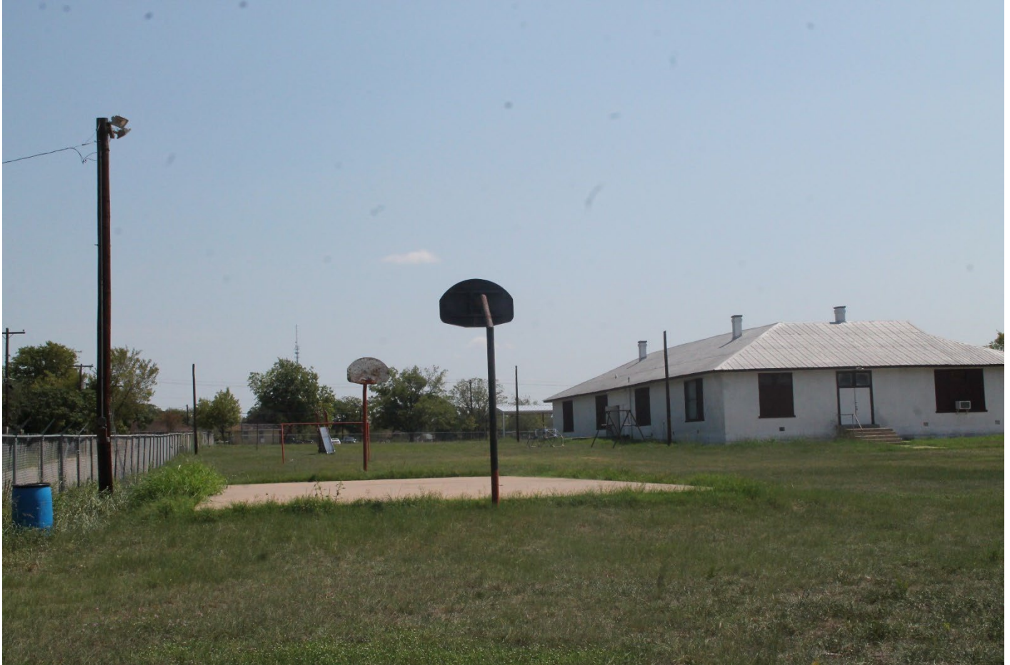
Photo 25: View of non-contributing basketball court, looking east, classroom building in background.
