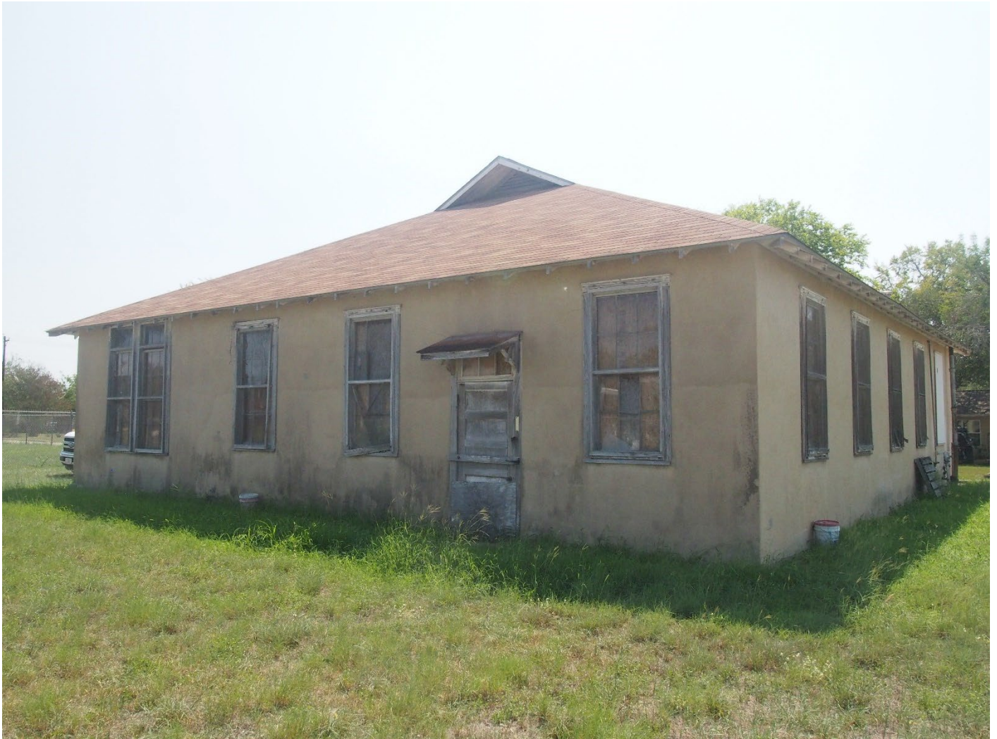
Photo 20: Vocational building, looking southeast.
