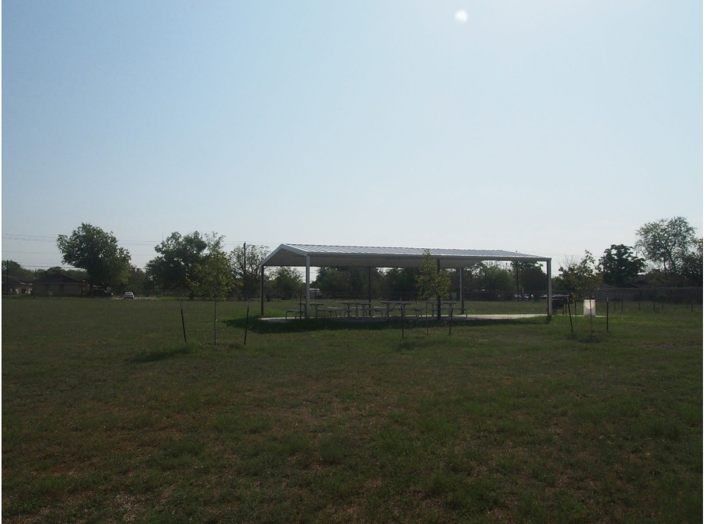
Photo 28: Non-contributing pavilion and picnic area to the east of the classroom building, looking east.
