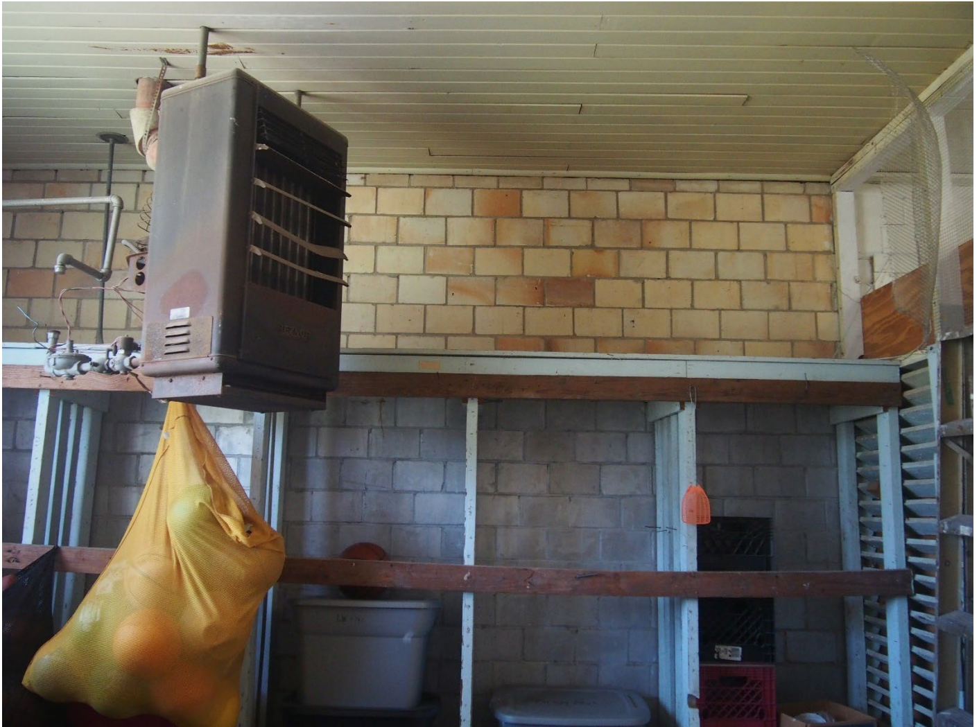
Photo 17: Gymnasium, men's locker room, looking east.
