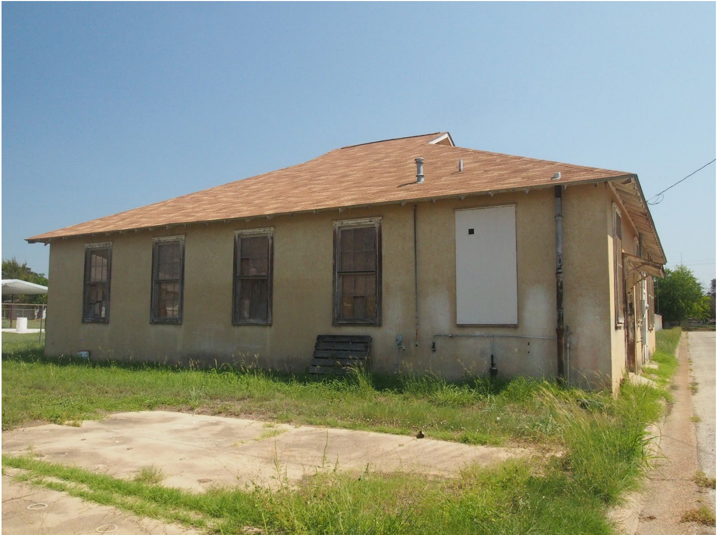
Photo 19: Vocational building, looking northeast.
