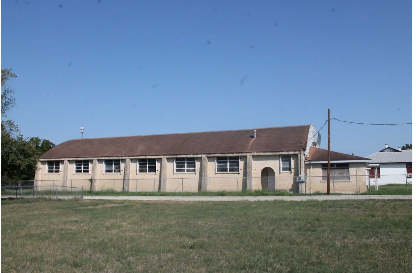
Photo 12: Gymnasium, looking northwest.
