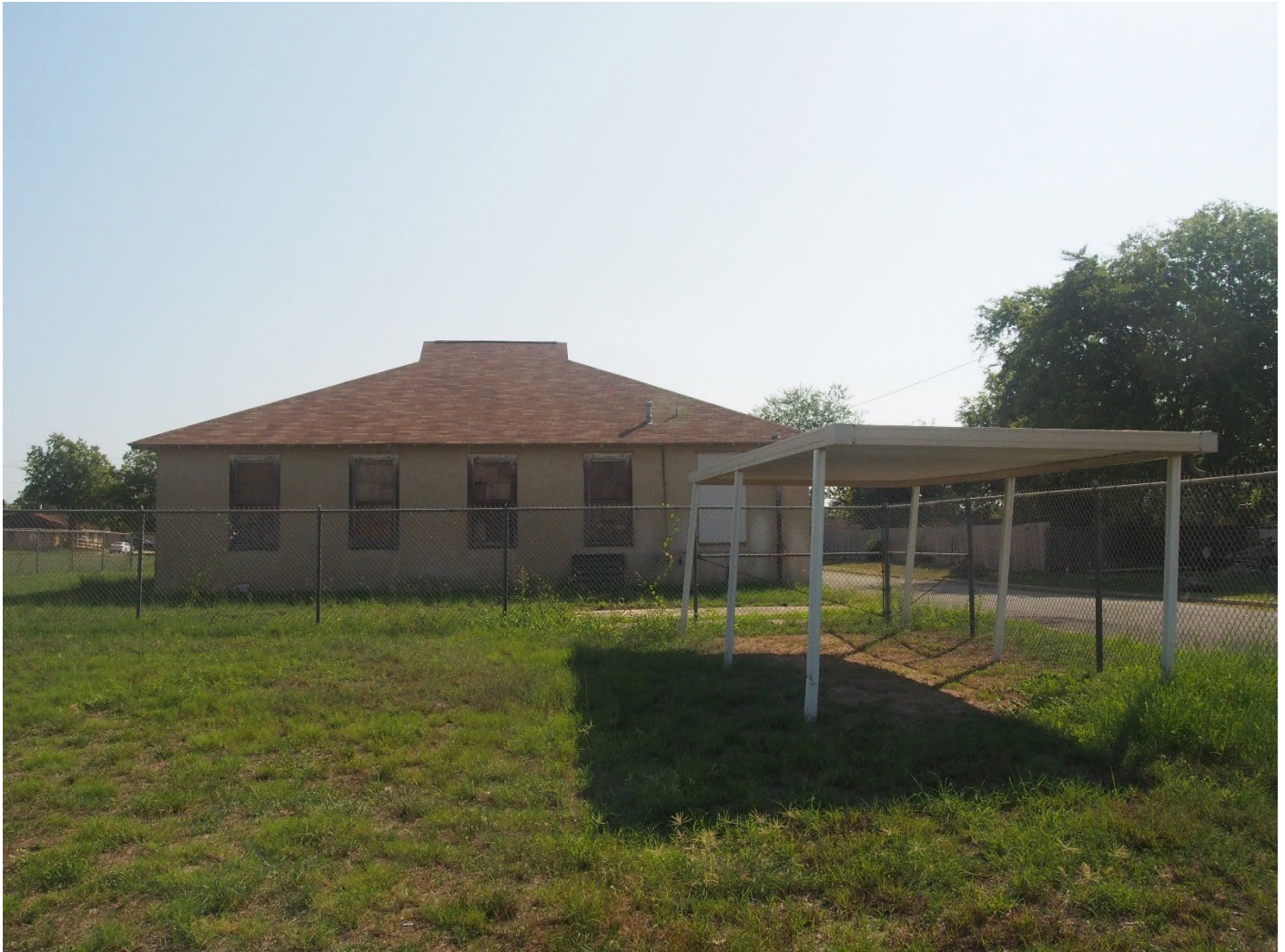
Photo 27: Non-contributing carport to the west of the vocational building, looking northeast, vocational building in background.
