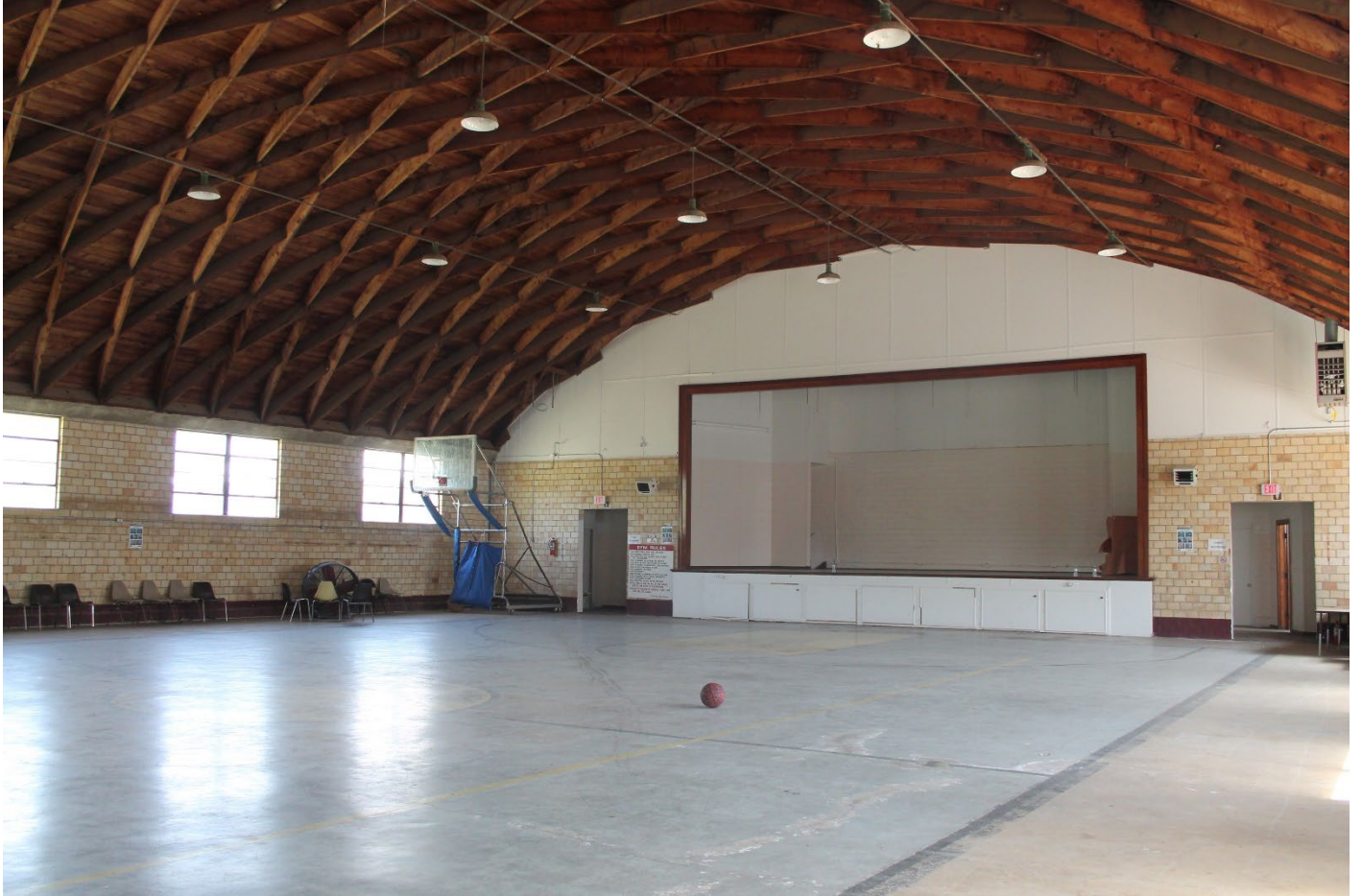
Photo 15: Gymnasium, view of stage, looking east.
