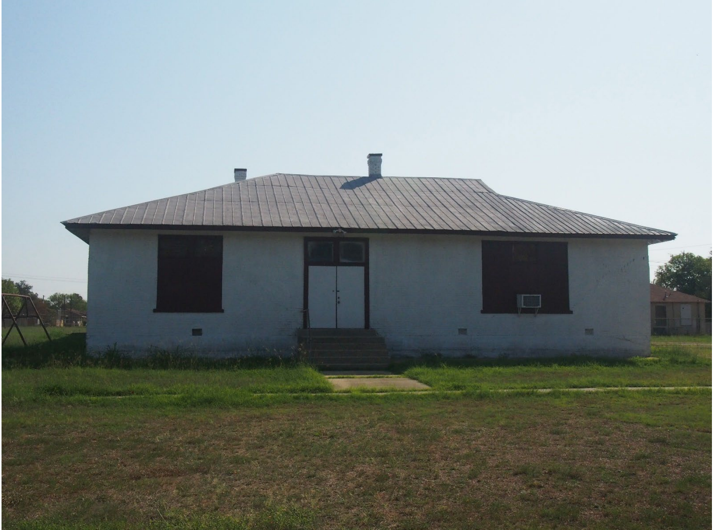
Photo 2: Main classroom building, looking northeast.
