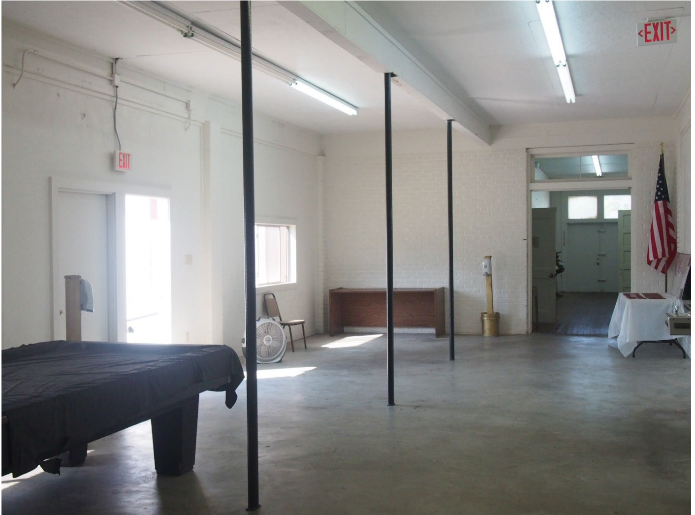
Photo 5: Main classroom building, foyer, looking southeast.
