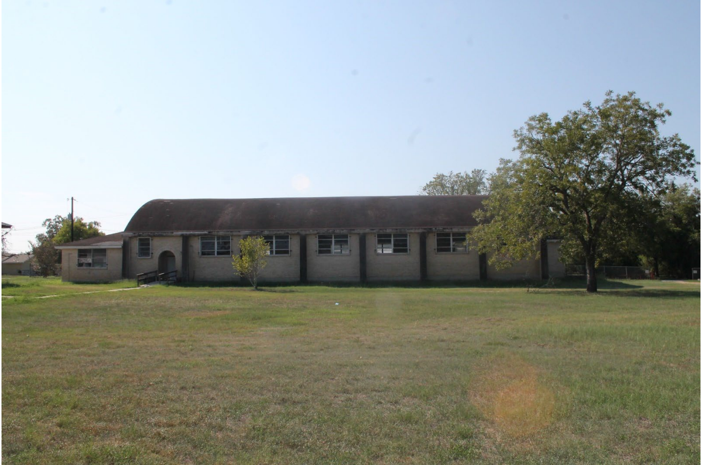
Photo 10: Gymnasium, looking southeast.
