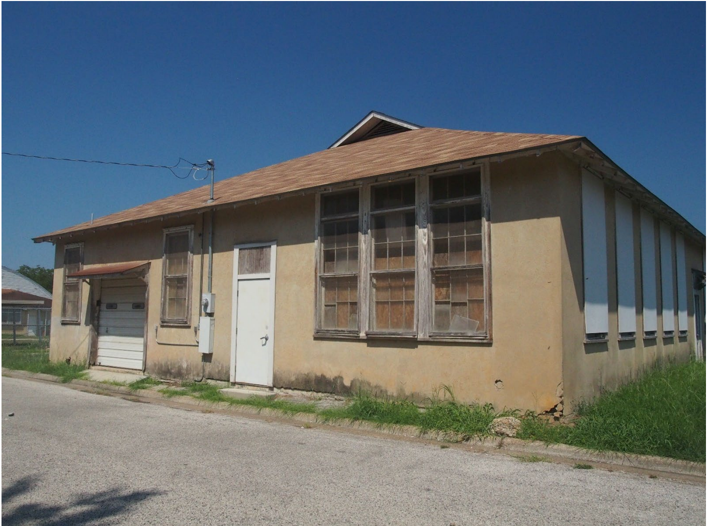
Photo 18: Vocational building, looking north.
