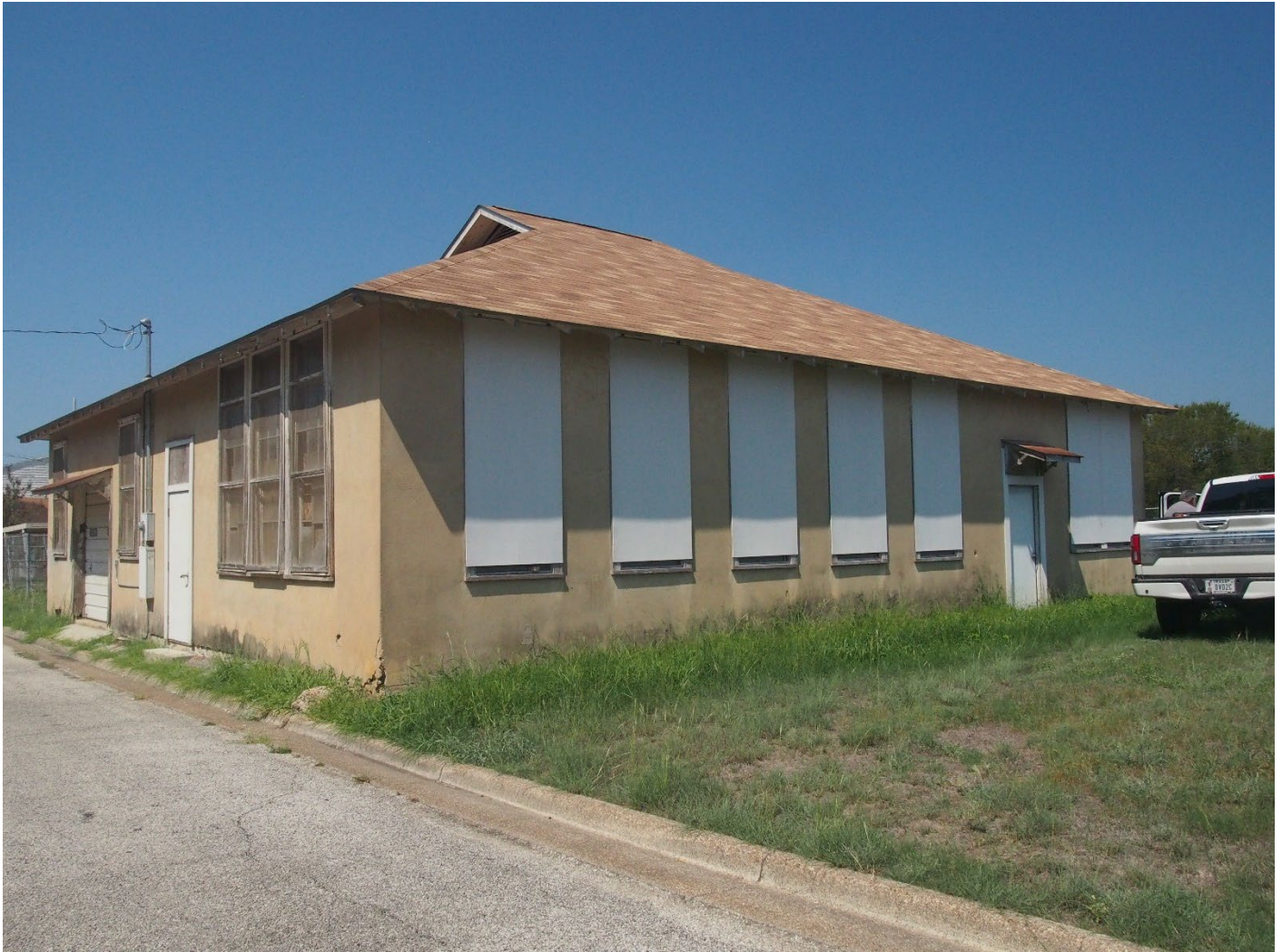
Photo 21: Vocational building, looking southwest.
