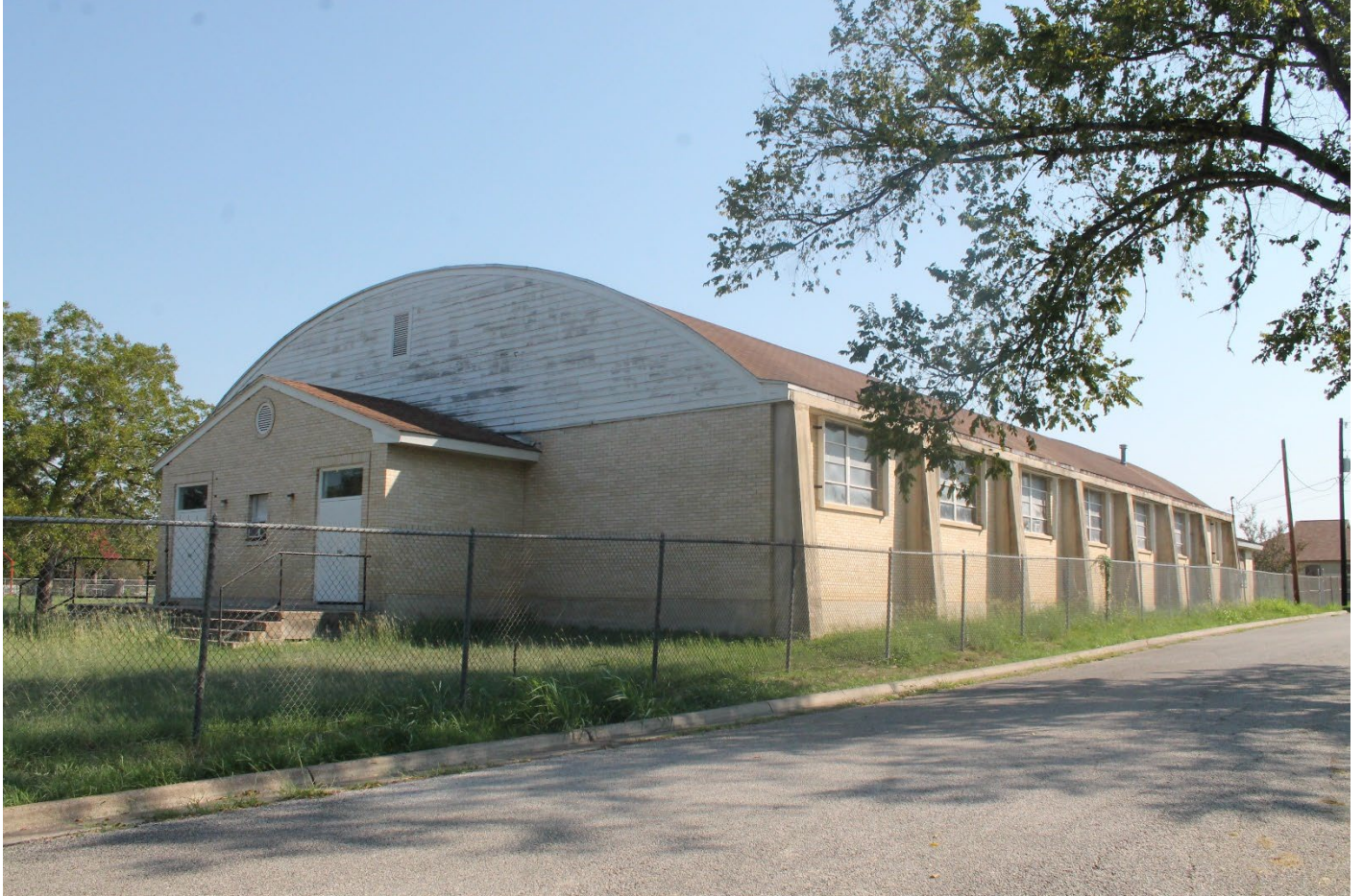
Photo 9: Gymnasium, looking north.
