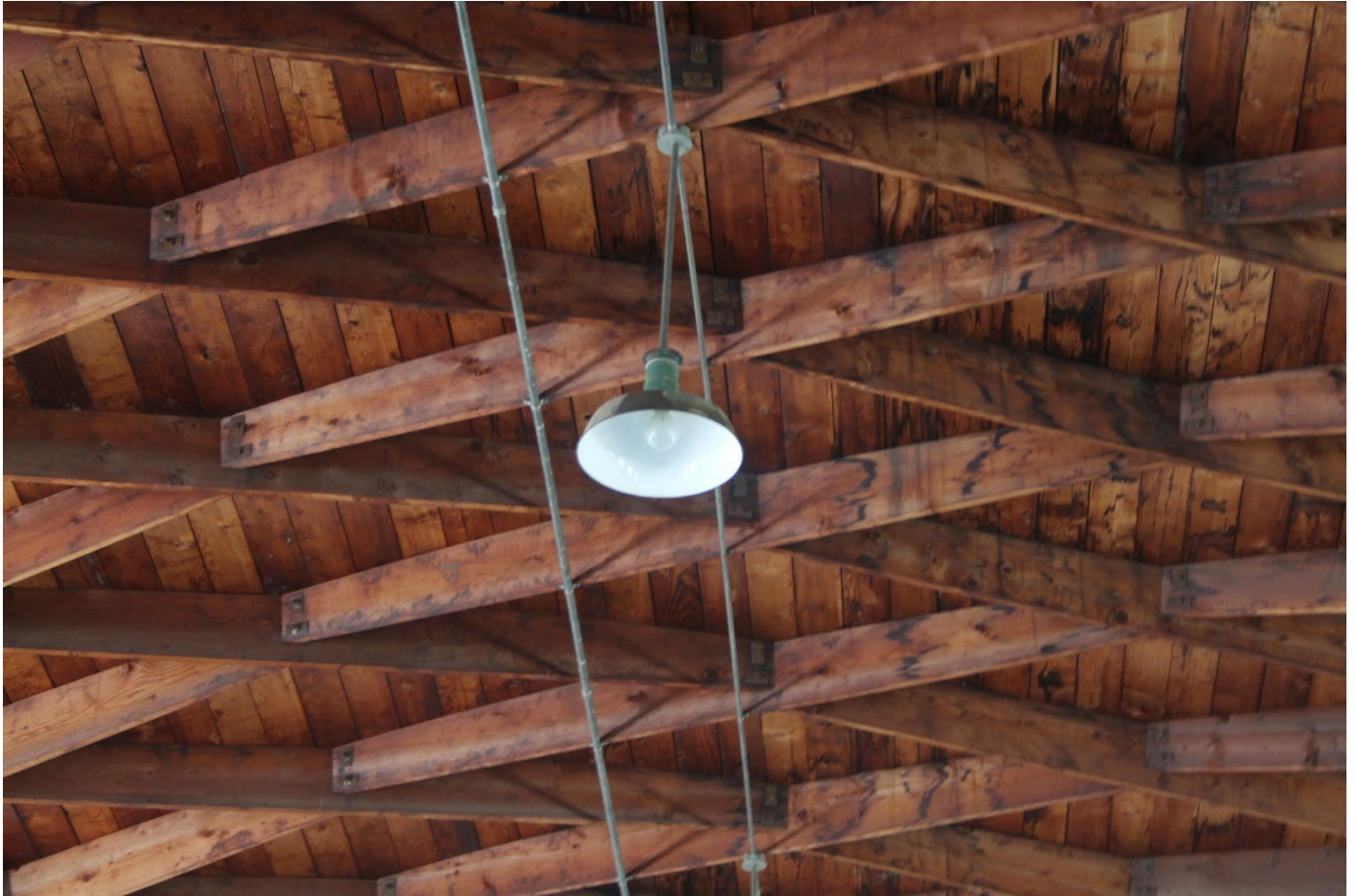
Photo 14: Gymnasium, detail view of lamella roofing.
