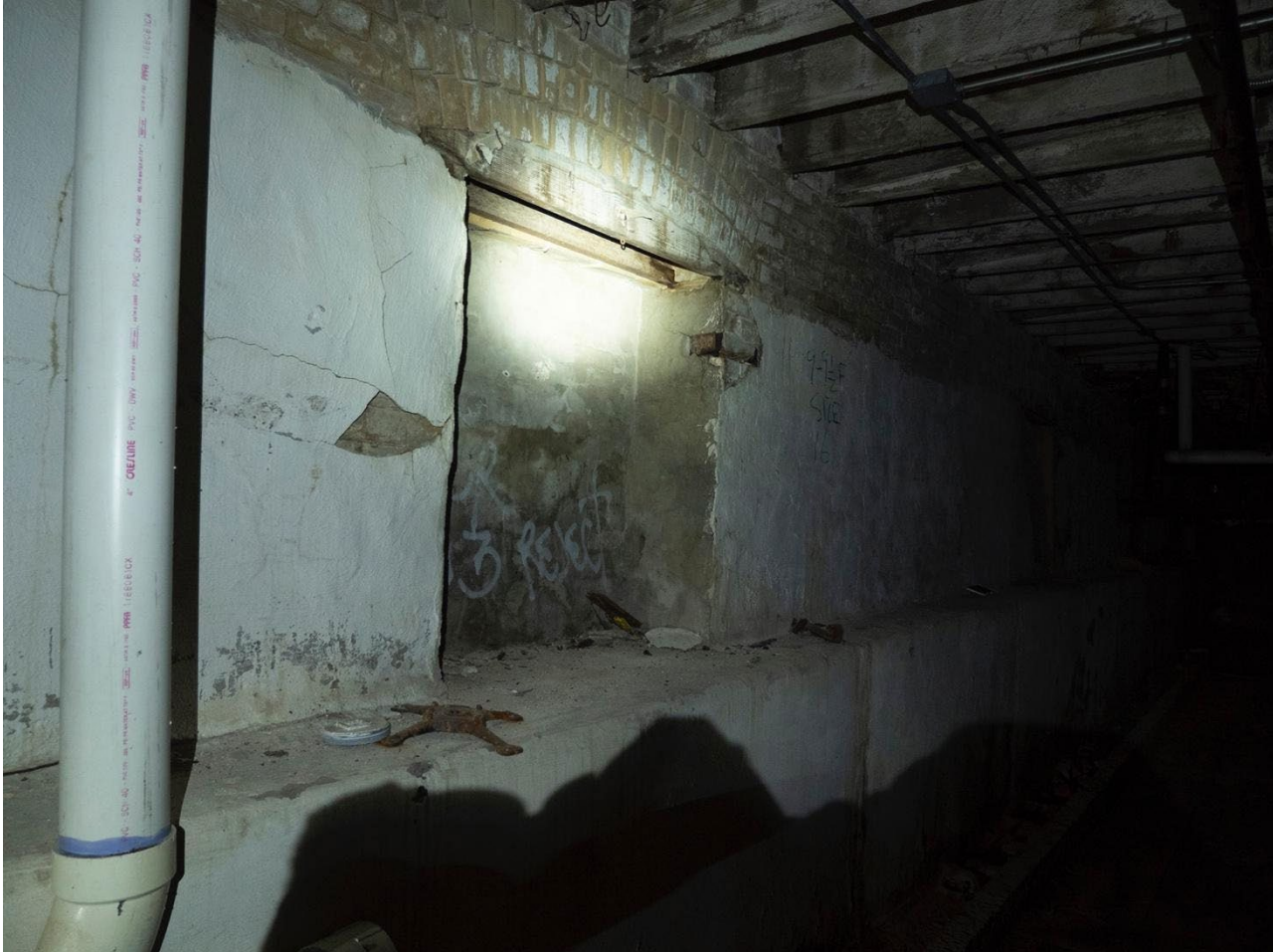
Photo 12: Hugo & Schmeltzer Company Building, Infilled Lightwell in Basement.
