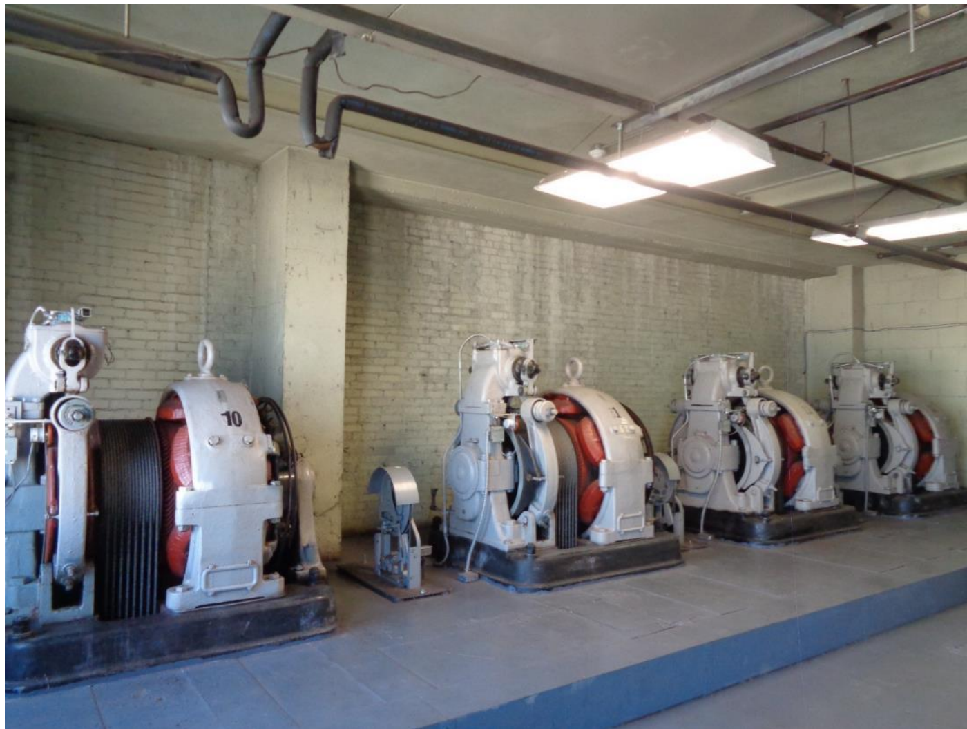
Photo 18: Elevator hoists, penthouse. View southeast.
