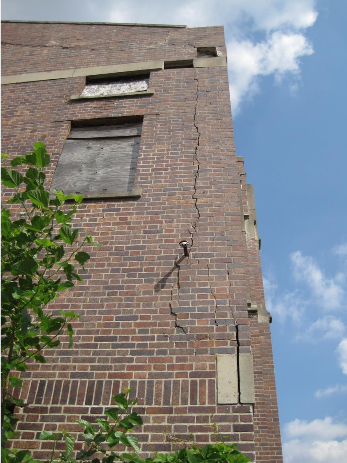
Figure 10. Brick separating at the rear (northwest) façade in 2010. Source: Texas Historical Commission.
