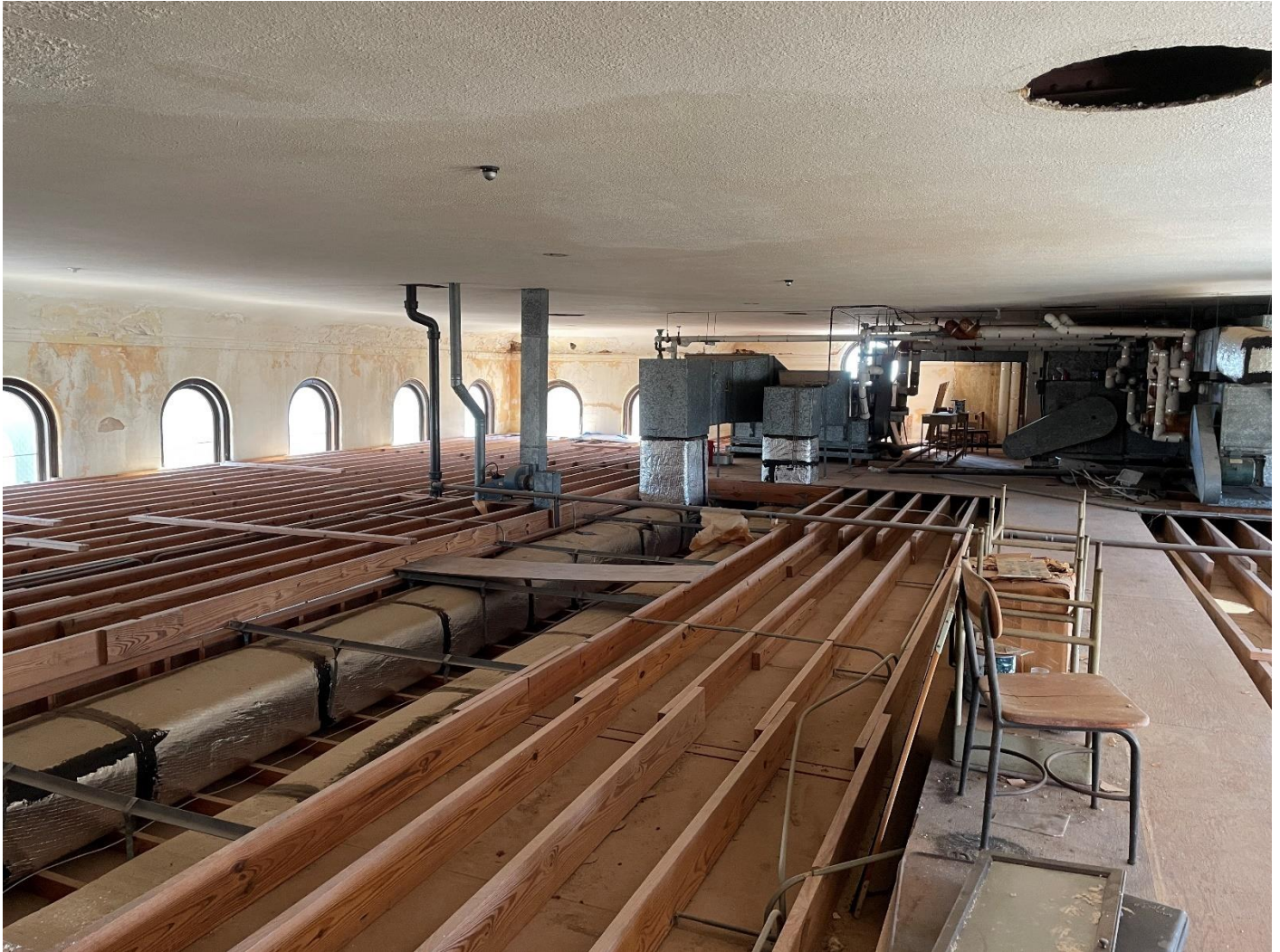
Photo 30. HVAC/mechanical (added at balcony level of former Sanctuary in 1963), looking southeast.
