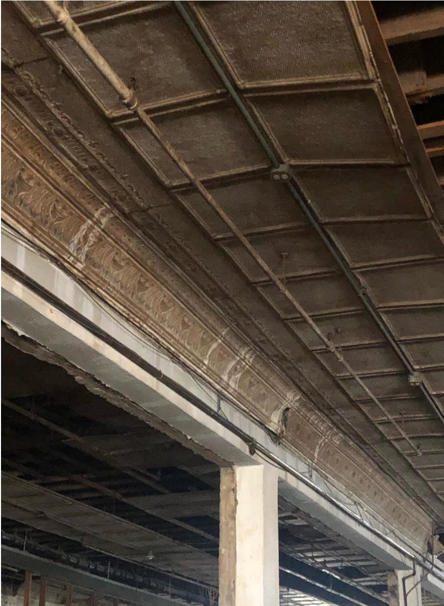
Photo 7: Fulwiler Building (159 Walnut St), First Floor Ceiling Detail. March 24, 2021.
