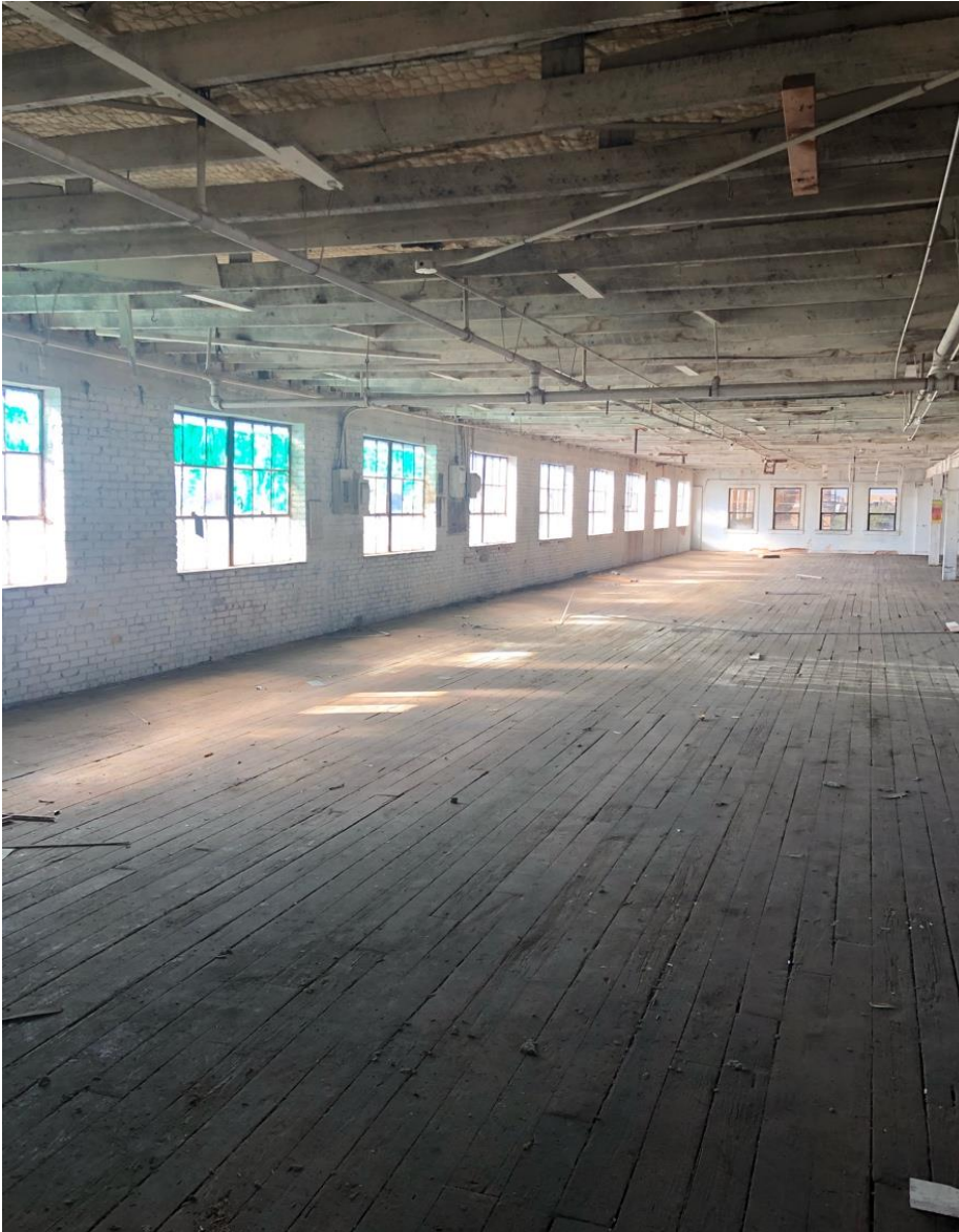
Photo 9: Fulwiler Building (159 Walnut St), Third Floor. View Southwest. March 24, 2021.
