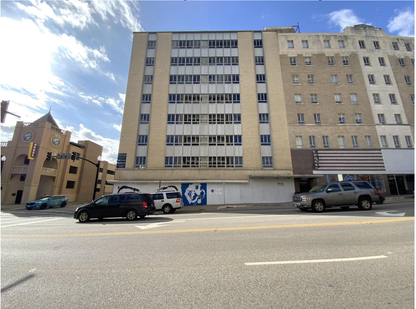
Photo No. 40. View of the 1954 S.A. Lindsey Building/Fair Petroleum Building (Resource 99), located at 115 South Broadway Avenue. The building adjoins the Fair Foundation Building (Resource 96) to the south. Camera facing west.
