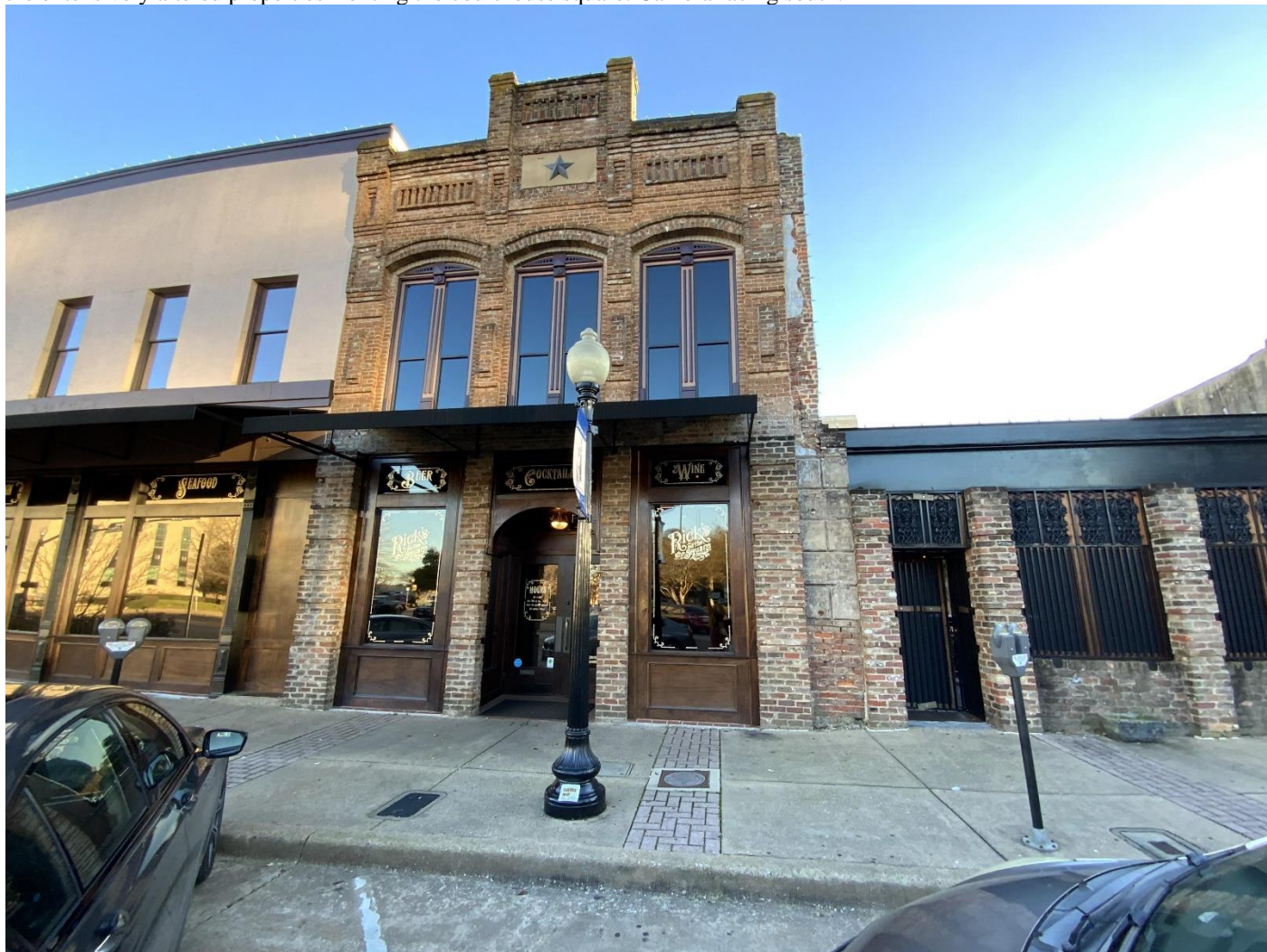
Photo No. 52. View of the two-part commercial block building (Resource 76) located at 110 West Erwin Street, an example of one of the extensively altered properties fronting the courthouse square. Camera facing south.
