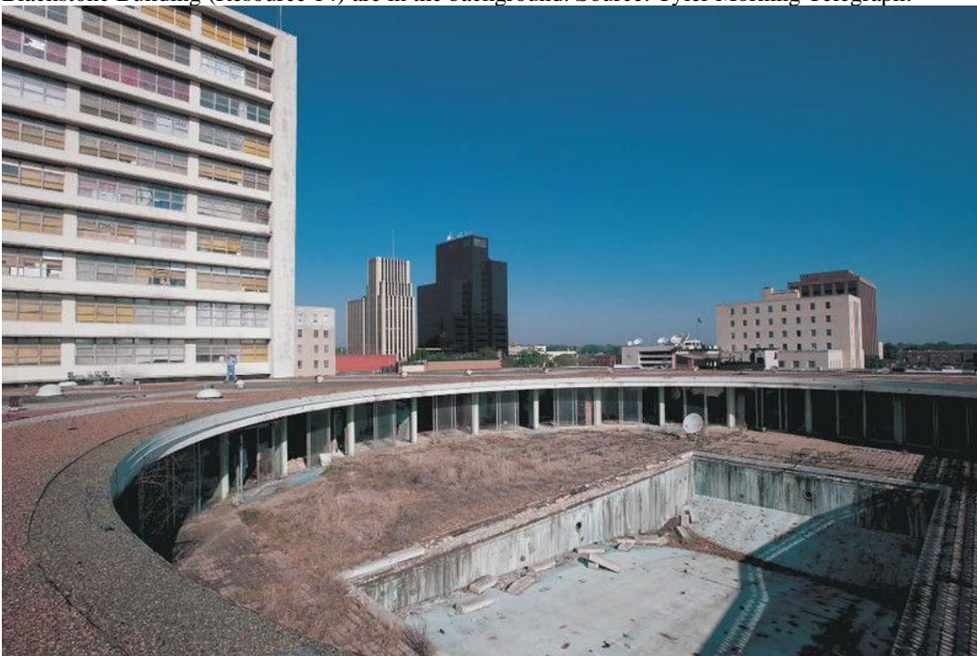
Figure 21. Current view of the swimming pool at the Carlton Hotel (Resource 100), sitting vacant and in disrepair. Efforts are underway to revitalize the hotel. The Fair Foundation Building (Resource 96), People's National Bank (Resource 60), and the Blackstone Building (Resource 14) are in the background. Source: Tyler Morning Telegraph.
