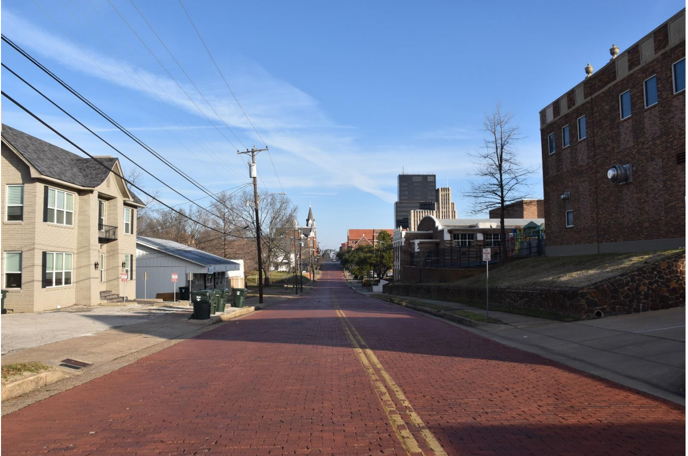
Photo No. 11. Contextual view looking north on South College Street. Camera facing north.
