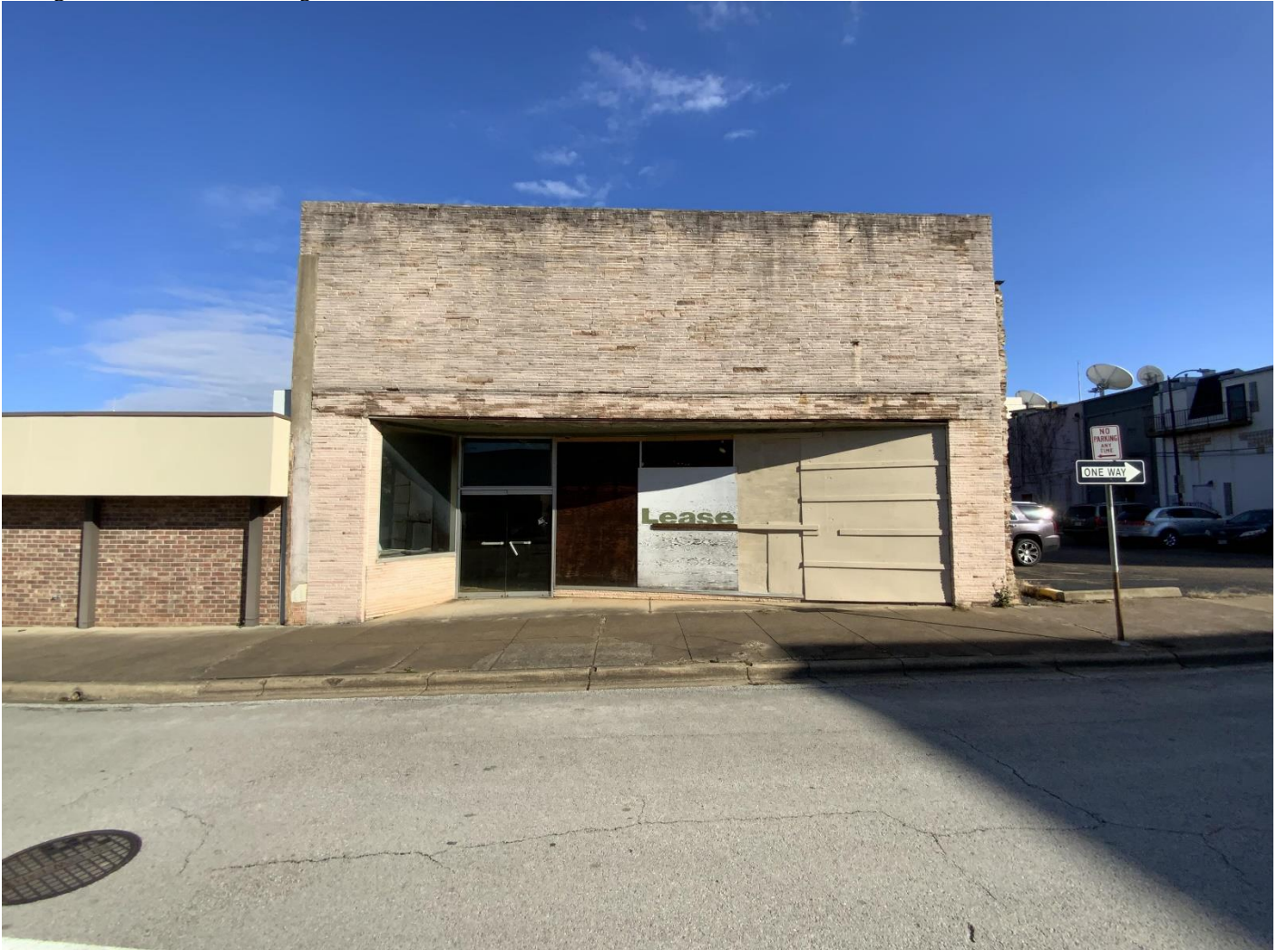
Photo No. 51. View of a brick one-part commercial block building (Resource 32) with an angled storefront, located at 207 North College Avenue. Camera facing east.
