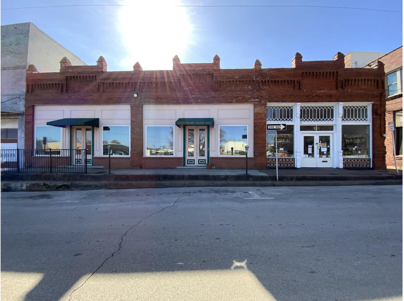
Photo No. 16. Frontal view of the Kamel Building (Resource 50), located at 211-215 East Ferguson Street. Camera facing northwest.
