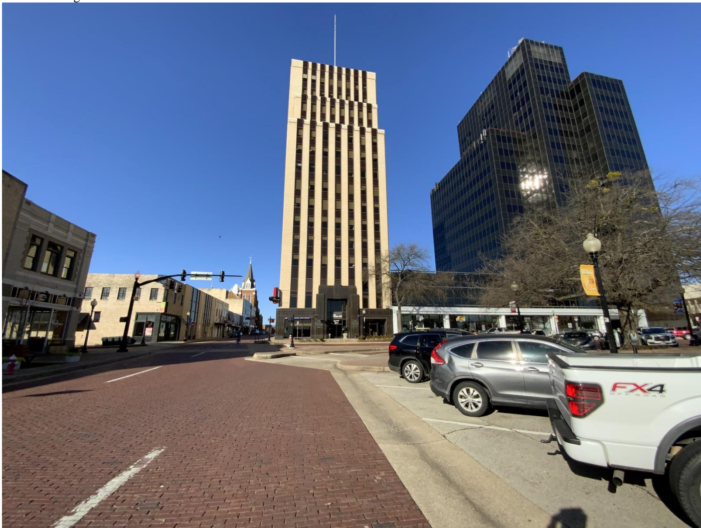
Photo No. 30. Contextual view looking westward on East Erwin Street of People's National Bank (Resource 60), the 15-story Art Deco highrise office building constructed on the northwest corner of North College Avenue and West Erwin Street in 1932. Camera facing west.
