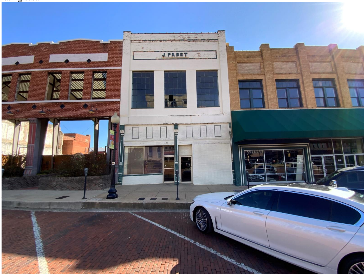
Photo No. 12. Front view of the J. Pabst Building, located at 109 North Spring Street (Resource 53). Camera facing east.
