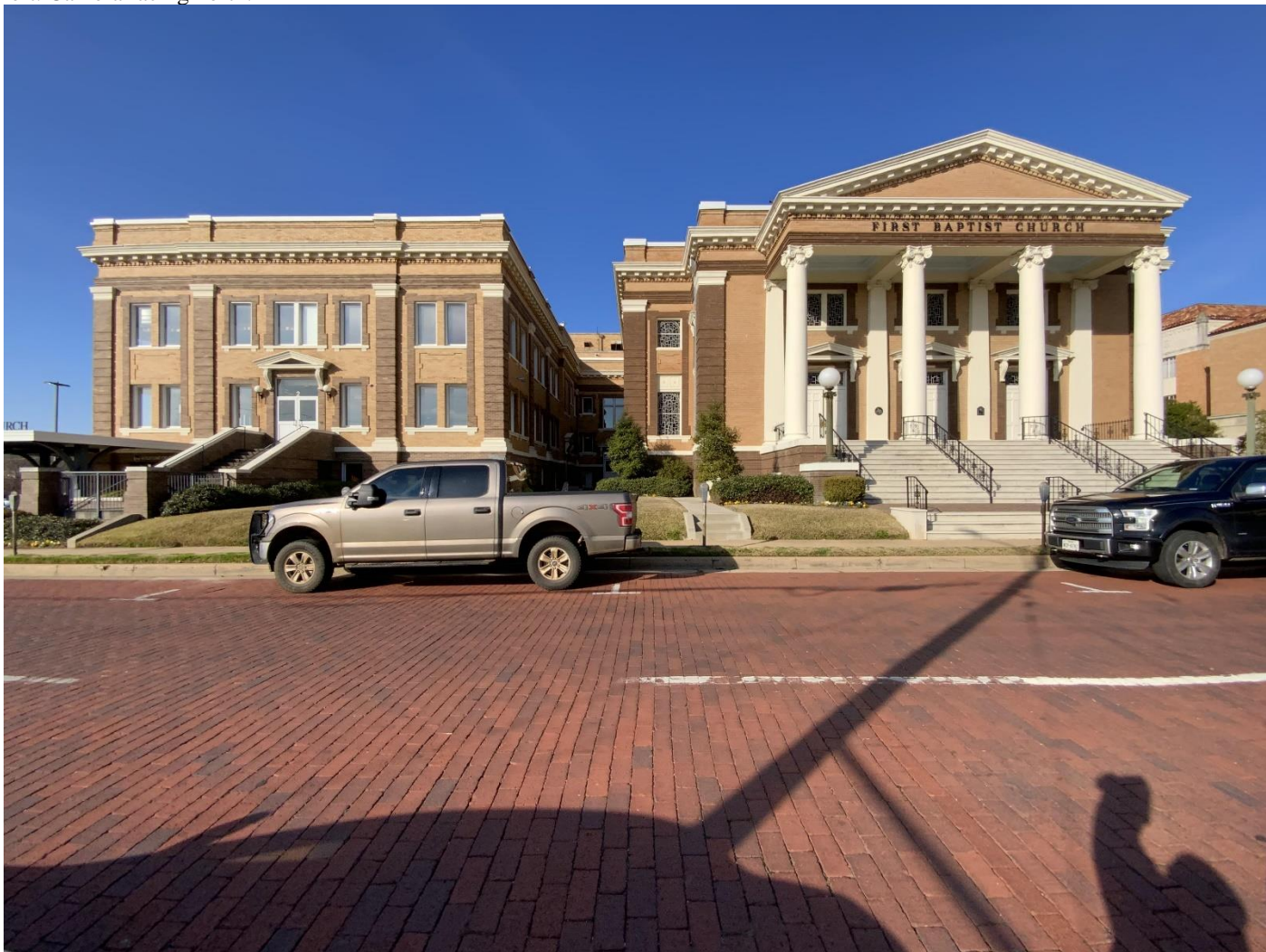
Photo No. 23. View of First Baptist Church (Resource 35), right, and the Lillie Belle Wright Education Building (Resource 34), left. Camera facing north.
