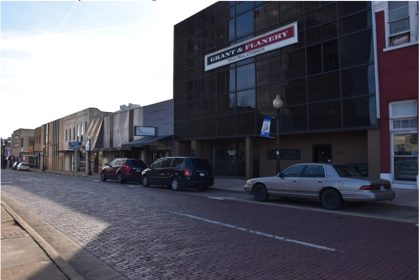
Photo No. 9. Contextual view of the north-facing commercial block buildings along the 200 block of West Erwin Street, many of which have been severely altered. Camera facing southeast.
