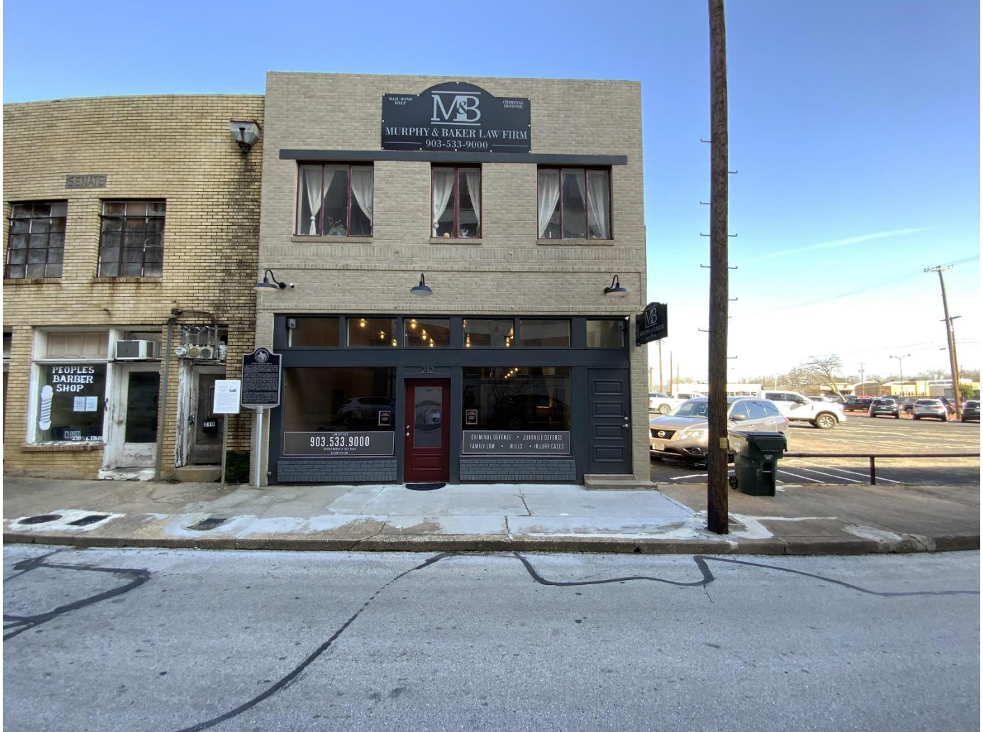
Photo No. 28. View of the two-part commercial block building located at 212 East Erwin Street (Resource 59). Clarence McDaniel, the son of a schoolteacher, ran People's Drug Store with his father-in-law Will Crawford out of this building. Later, in 1934, Henry Miller Morgan opened the first barber college for African Americans in the country, Tyler Barber College, in the edifice. Camera facing north.
