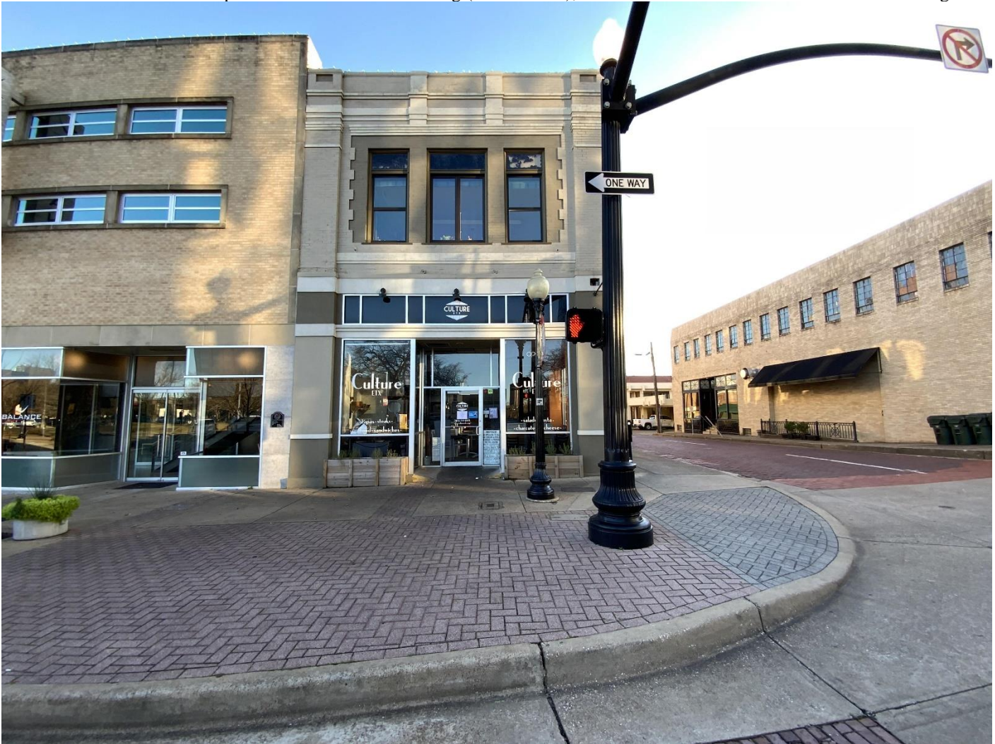
Photo No. 48. View of a two-part commercial block building (Resource 71), located at 110 West Erwin Street. Camera facing south.
