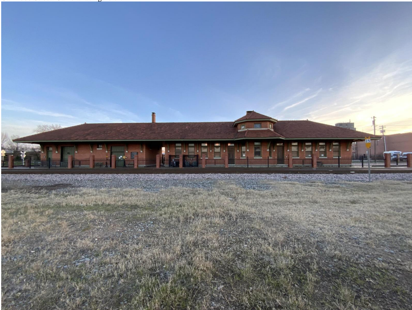
Photo No. 18. View of the St. Louis Southwestern Railway (Cotton Belt) Passenger Depot (Resource 2), located at 210 East Oakwood Street. Camera facing north.
