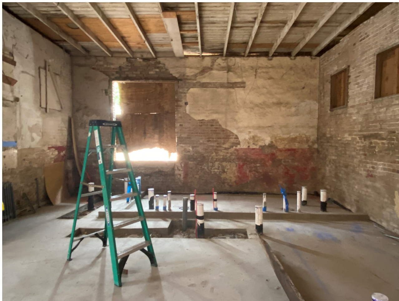
Photo 13: Interior view of rear addition during rehabilitation, facing north.
