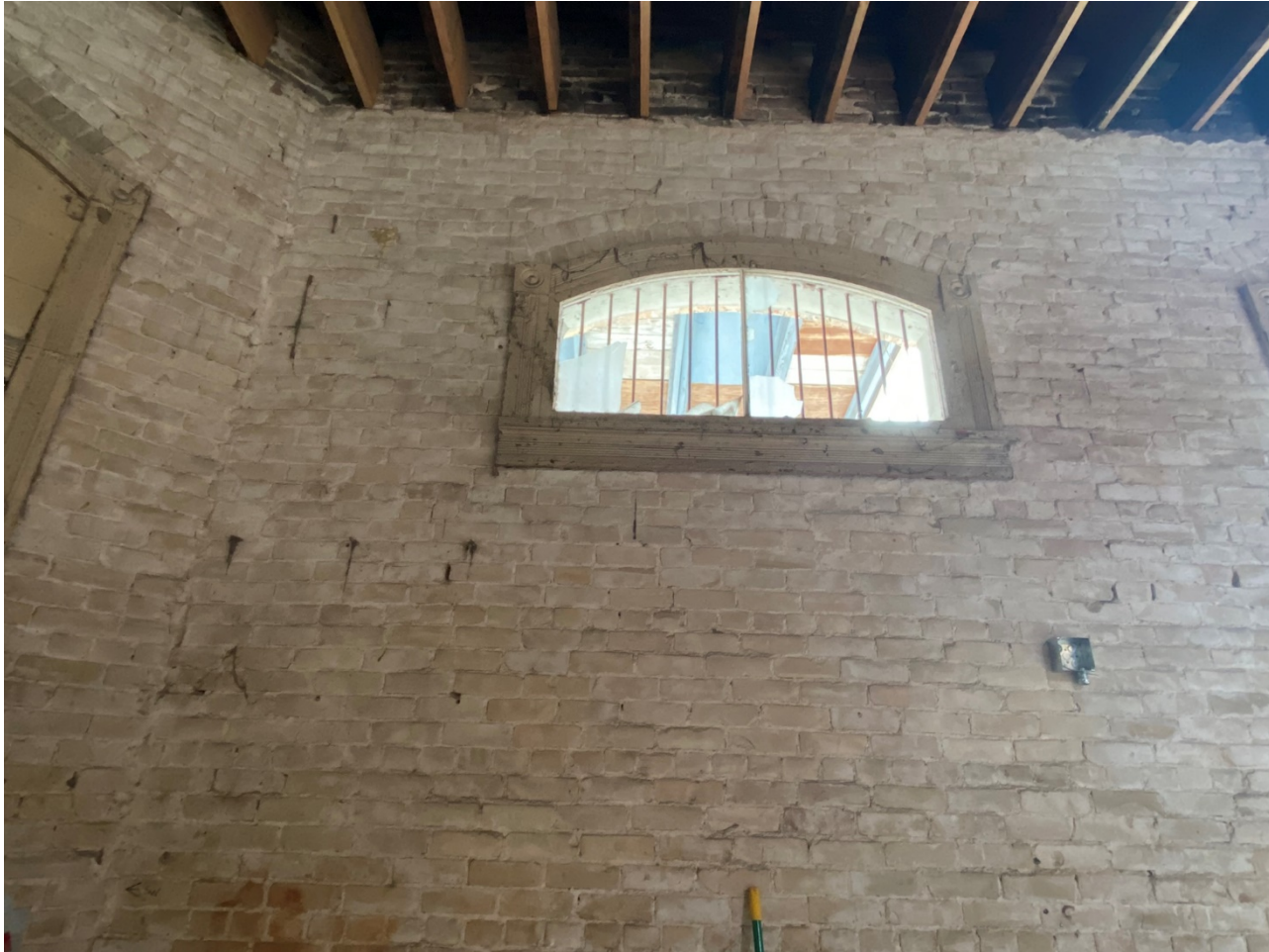
Photo 14: Interior view of window on west wall, facing west.
