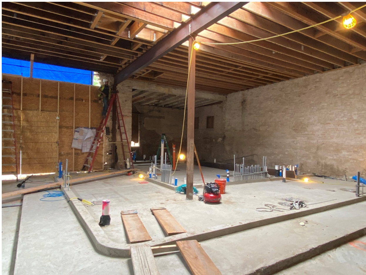
Photo 11: Interior view of building during rehabilitation, facing northeast.
