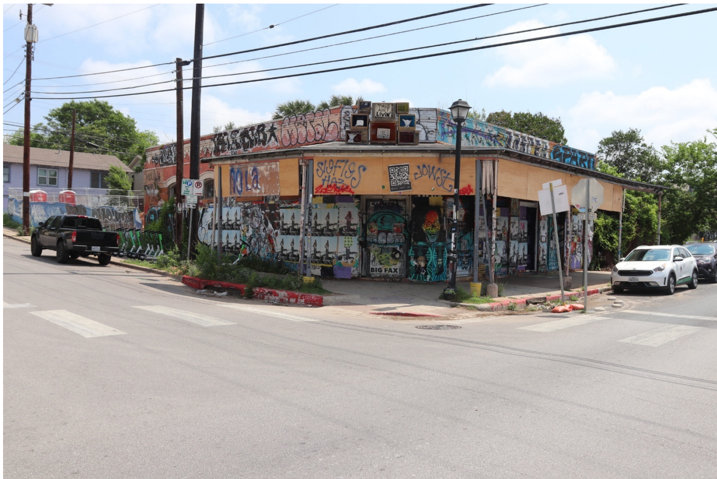
Photo 2: Southwest oblique showing chamfered corner entrance, facing northeast.
