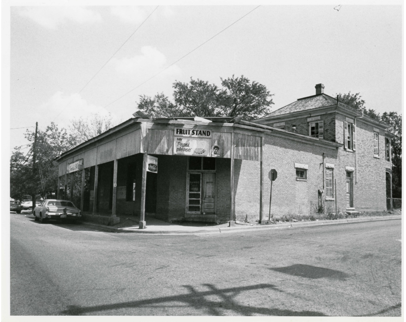
Figure 20. The NR-listed Haehnel Building at 1101 E. 11th Street, 1984. Note the similarity in the building's footprint, chamfered corner entrance, canopy, and front exterior to the nominated building at 1200 E. 6th Street. Source: Martha Doty and Joe Freeman, "Historic Resources of East Austin/East Austin MRA." National Register of Historic Places Inventory/Nomination Form, Texas Historical Commission, September 17, 1985, https://atlas.thc.texas.gov/NR/pdfs/85002295/85002295.pdf .
