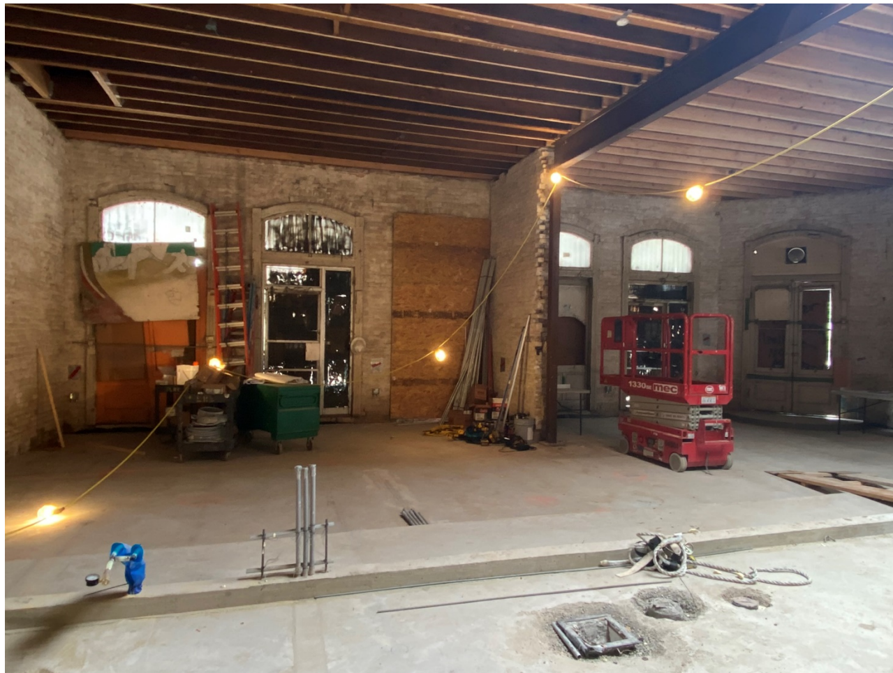
Photo 12: Interior view of building, facing southeast.
