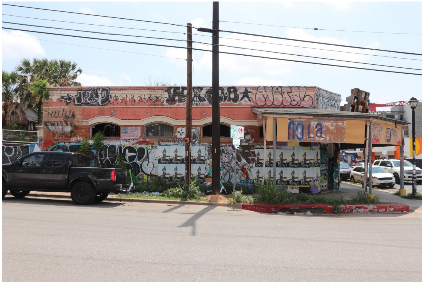
Photo 3: West elevation, facing east.
