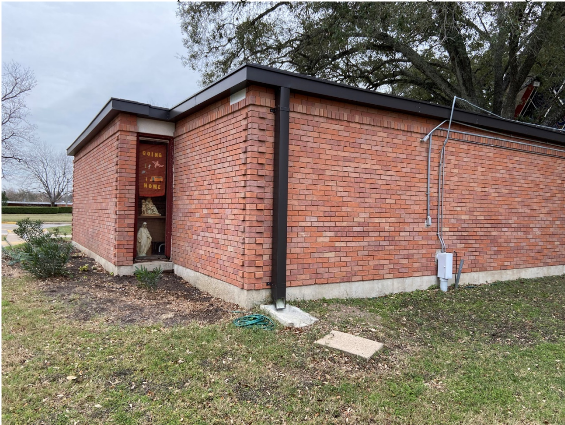
Photo 4: North elevation oblique showing reentrant corners and corbeling, camera looking southeast.
