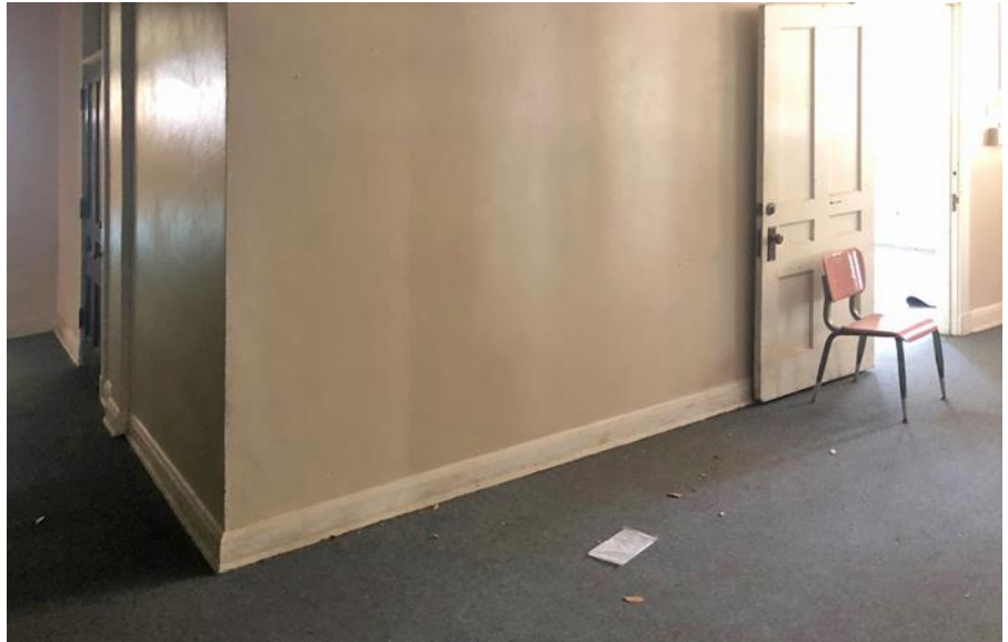
FIGURE 32: 2020 SFA Elementary, interior entry hall looking southwest, original doors and trim, base matched Giesecke & Harris typical detail
