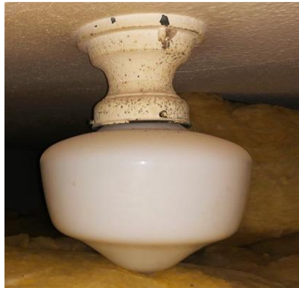
FIGURE 46: 2020 SFA Elementary, original north classroom corridor exterior light fixture and stucco ceiling concealed above drop-ceiling
