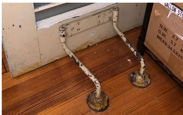
FIGURE 51: 2019 Zavala Elem. Austin, TX, Giesecke & Harris, closet door pivot hardware
