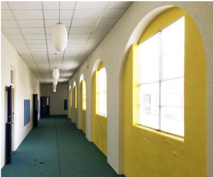
FIGURE 45: 2019 SFA Elementary, south classroom corridor, looking west, originally covered open-air corridors, infilled arches (right) opened to courtyard, entrance to classrooms (left)
