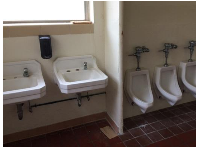
FIGURE 42: 2019 SFA Elementary, boys' restroom, original plaster walls, tile base, sinks remain
