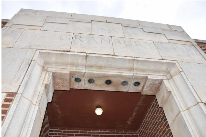
Photo 6: Inside east entryway looking up, camera facing west. May 15, 2018.
