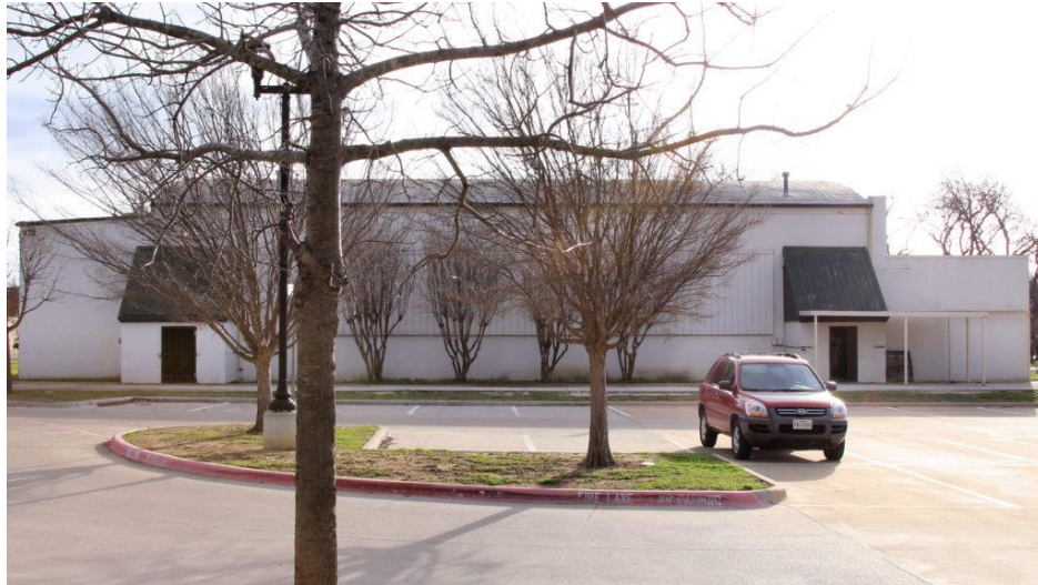
Figure 11: Burlleson Gymnasium, designed by architect C.M. Love and constructed in 1935. From Living New Deal, https://livingnewdeal.org/projects/burleson-gymnasium-tx/ .
