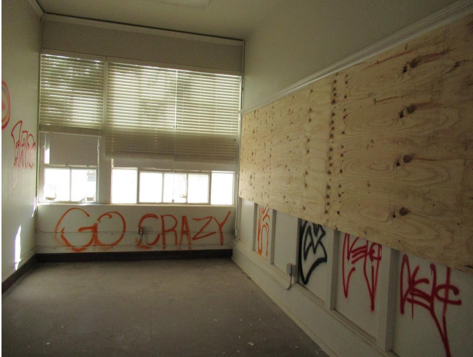
Photo 19: Second Floor Office
