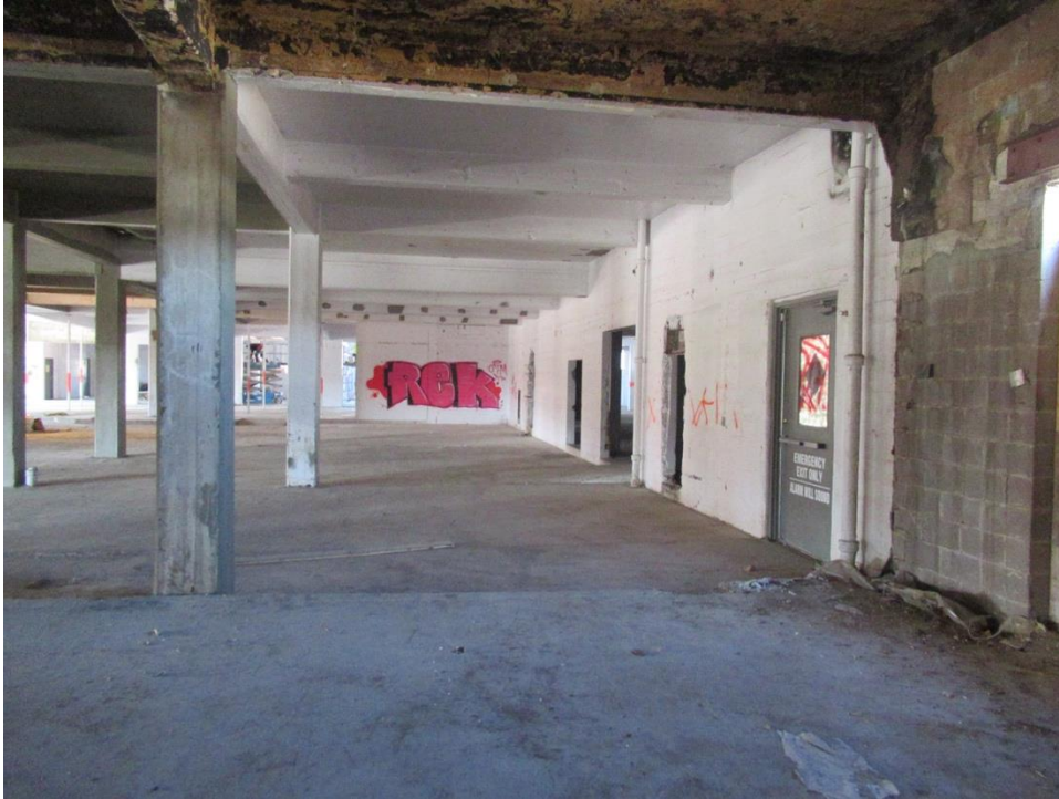
Photo 13: First Floor Central Space
