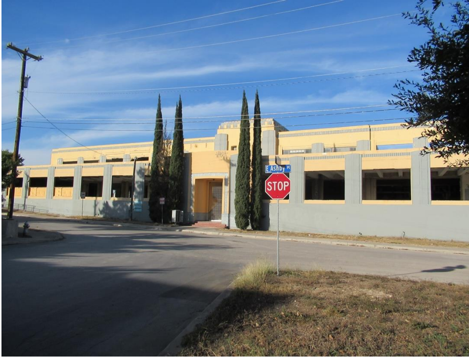
Photo 1: Primary (Southwest) Elevation, View Northwest.
