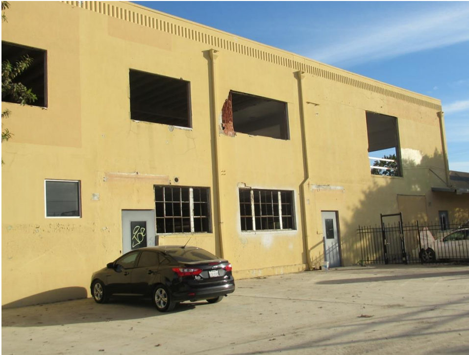
Photo 5: Northwest Elevation, View East.
