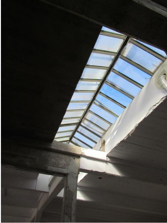
Photo 9: Second Floor Skylight Detail
