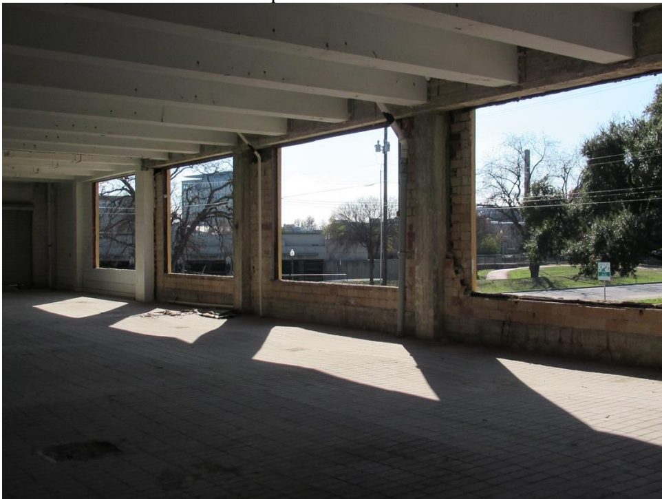
Photo 12: First Floor Southeast Space
