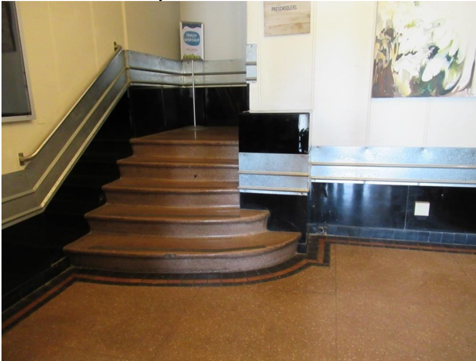
Photo 11: First Floor Lobby
