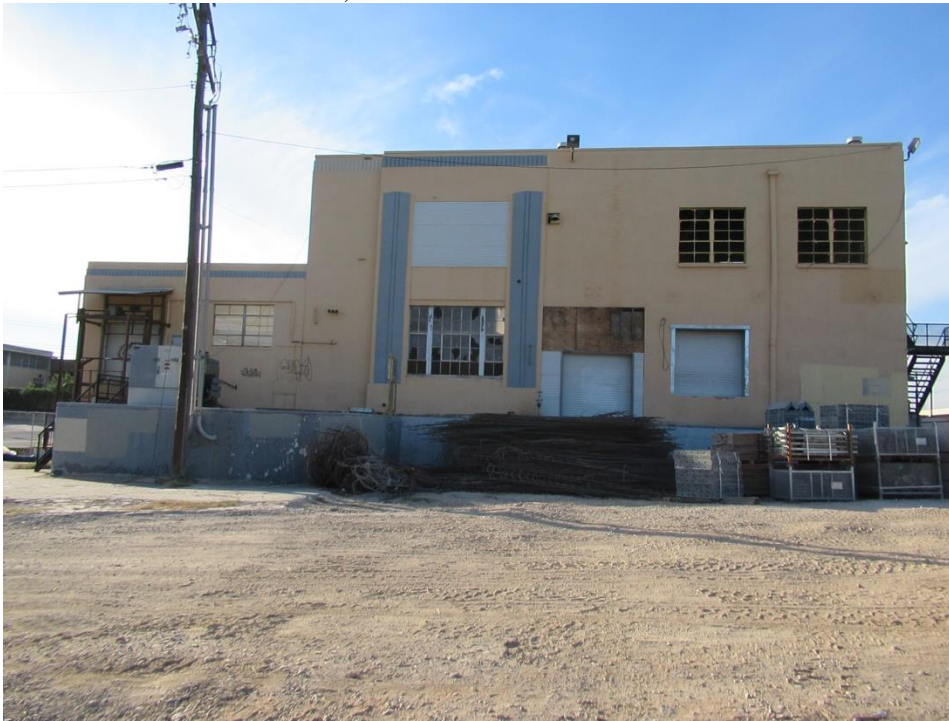
Photo 2: Southeast Elevation, View West.
