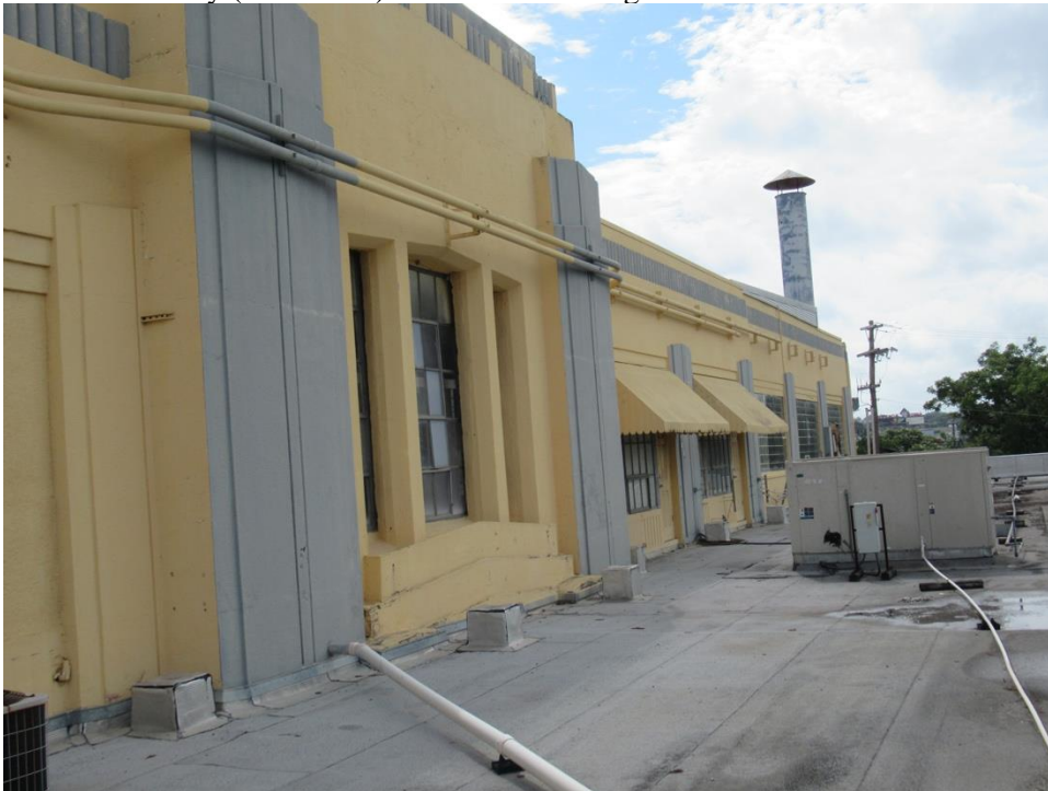
Photo 6: Primary (Southwest) Elevation Showing Second Floor Exterior from Roof, View East
