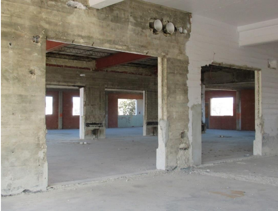
Photo 15: Second Floor Northwest Space
