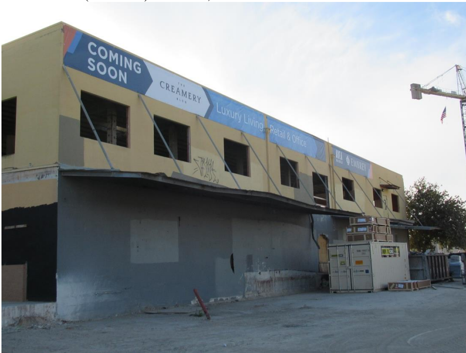
Photo 4: Rear (Northeast) Elevation, View South
