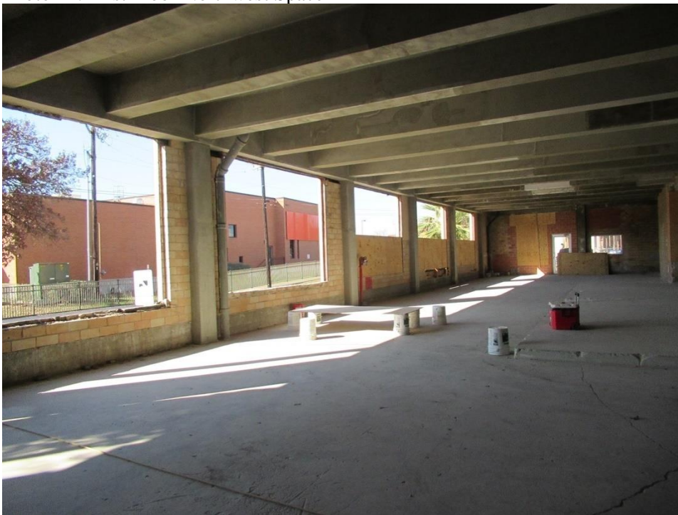
Photo 14: First Floor Northwest Space
