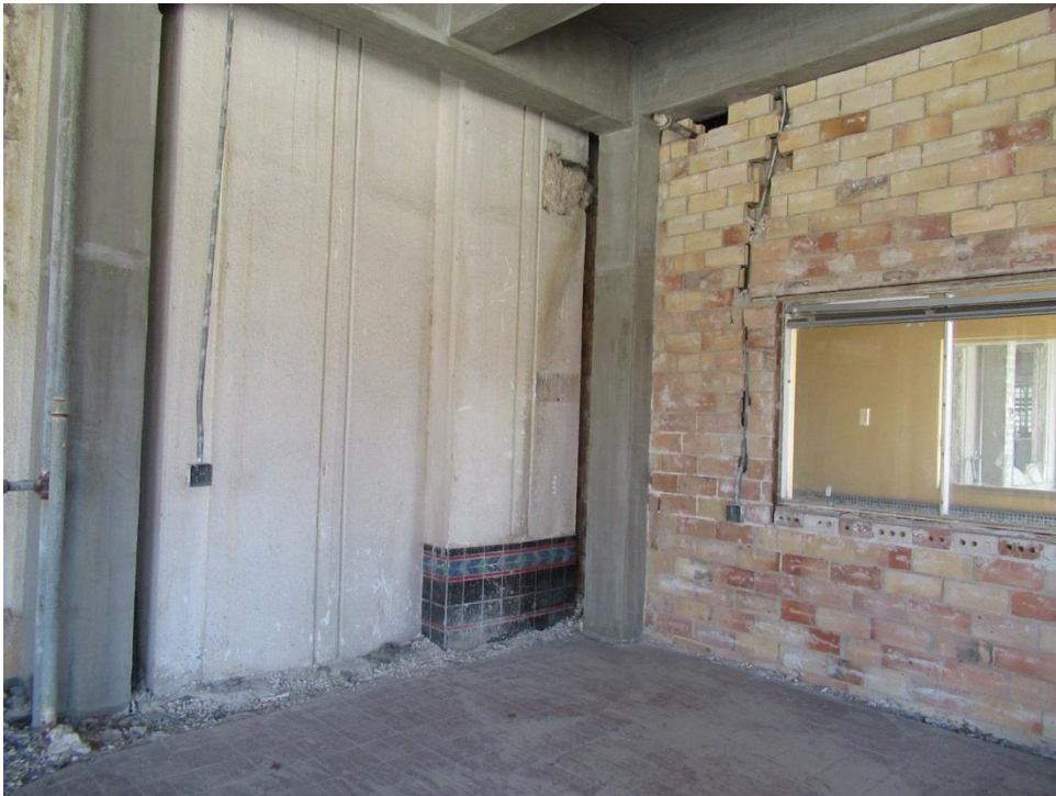
Photo 10: First Floor Entrance Vestibule
