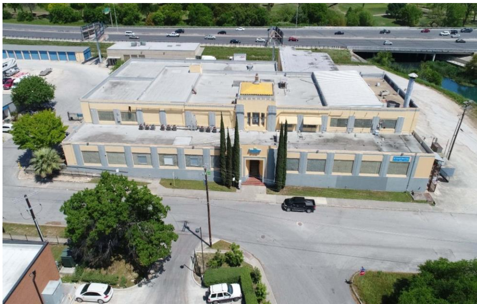
Figure 30: Primary (Southwest) Elevation, View Northeast. Taken November 2019, prior to partial demolition. Non-historic additions and window infill have been removed.
