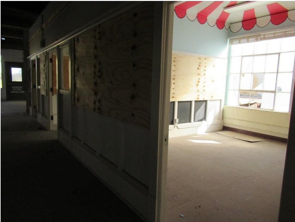
Photo 18: Second Floor Corridor
