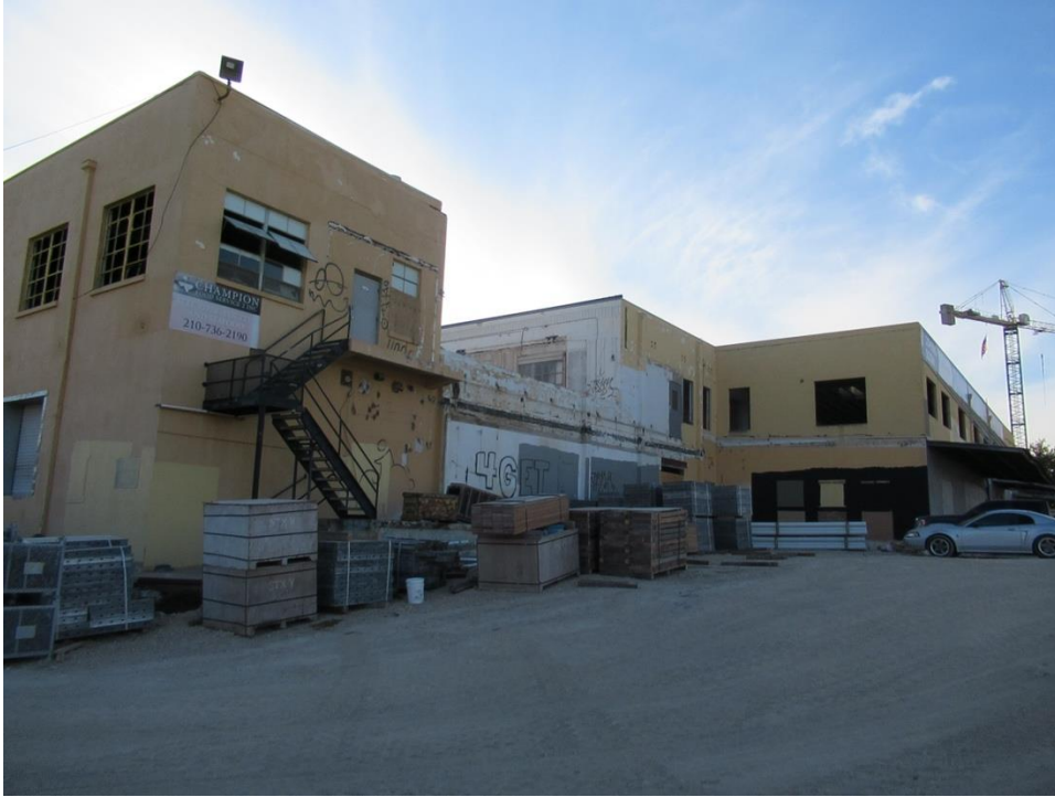
Photo 3: Rear (Northeast) Elevation, View West.
