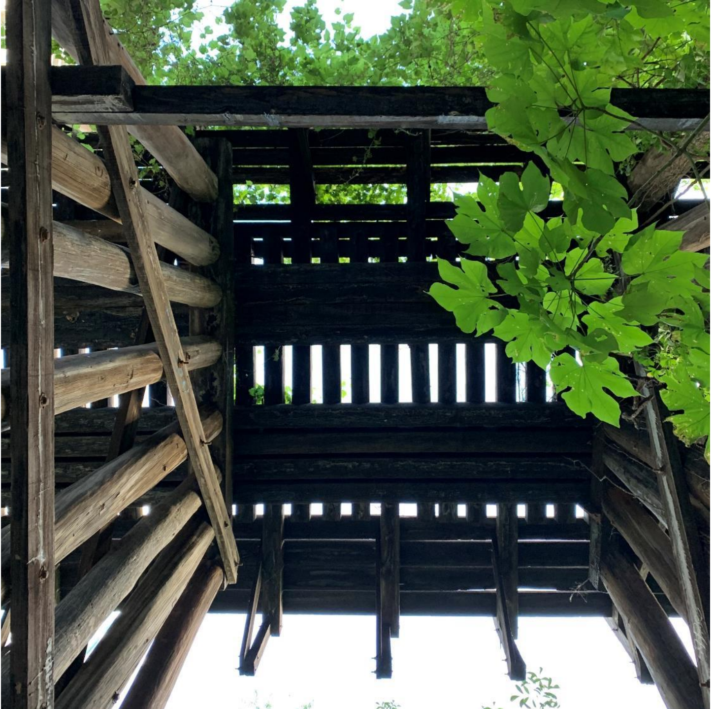
Photo 10: View from beneath Third Street Railroad Trestle. Photo by Andrew Boudreaux.
