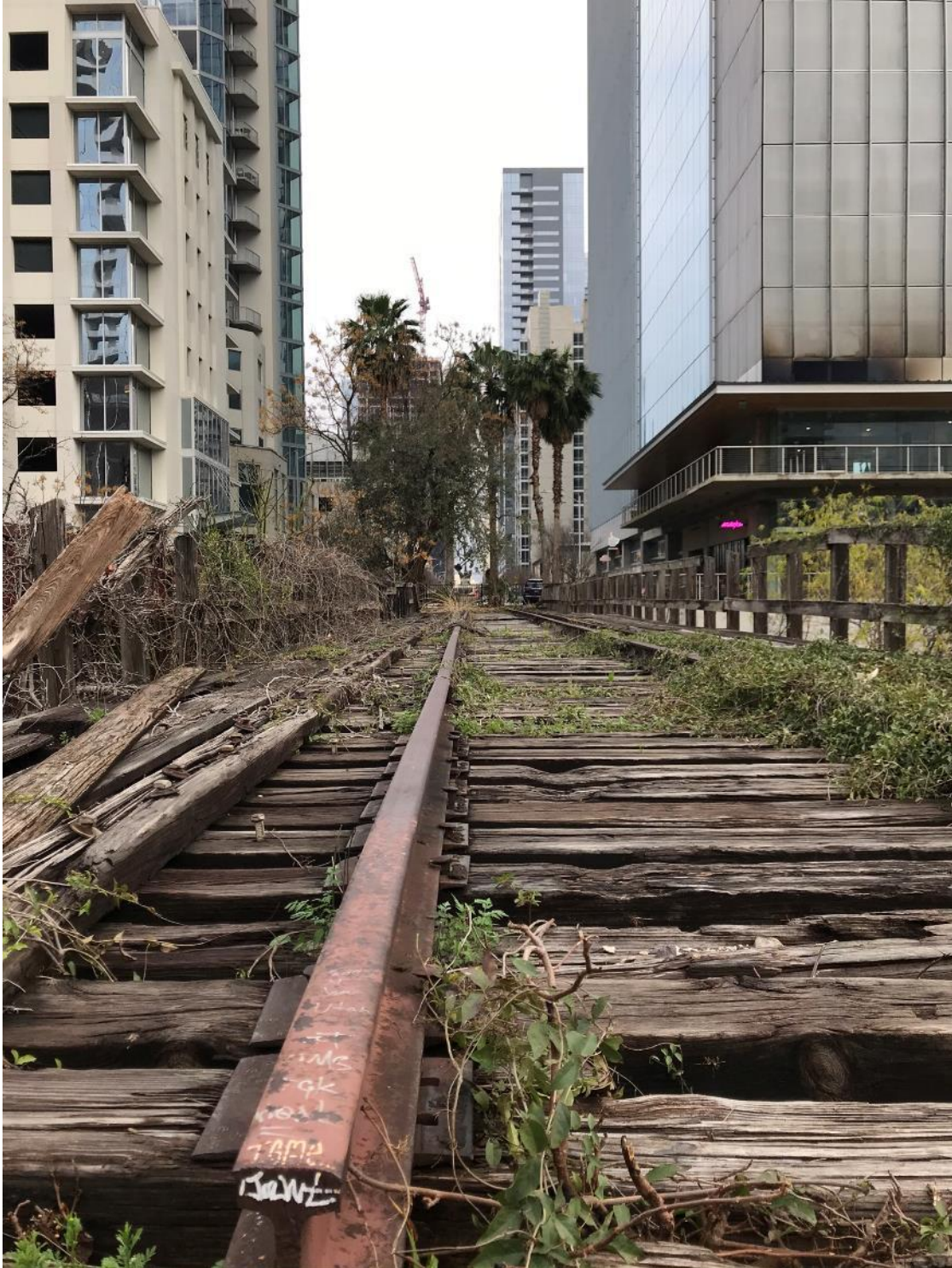
Photo 3: Third Street Railroad Trestle surface detail, camera facing east. Photo by Joemy Buschur.
