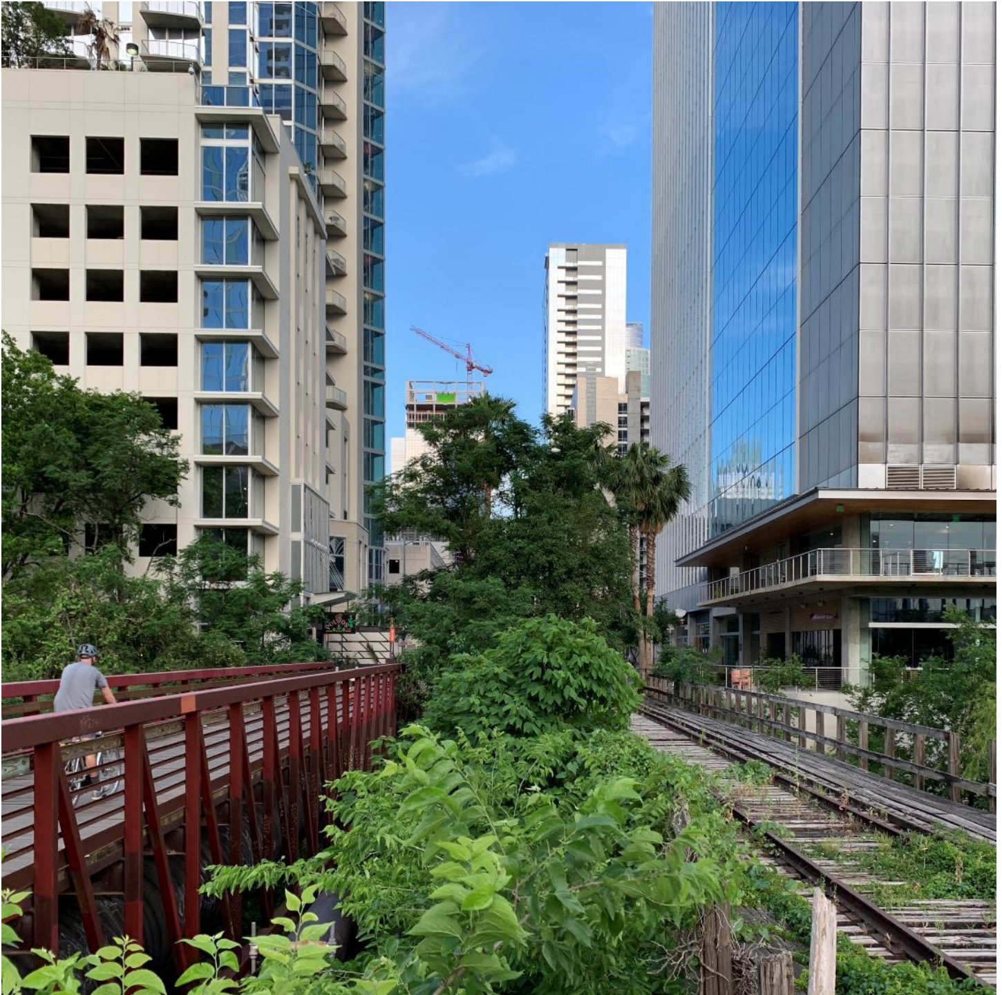
Photo 7: View of Shoal Creek Trail Bridge and Third Street Railroad Trestle, camera facing east. Photo by Andre Boudreaux.
