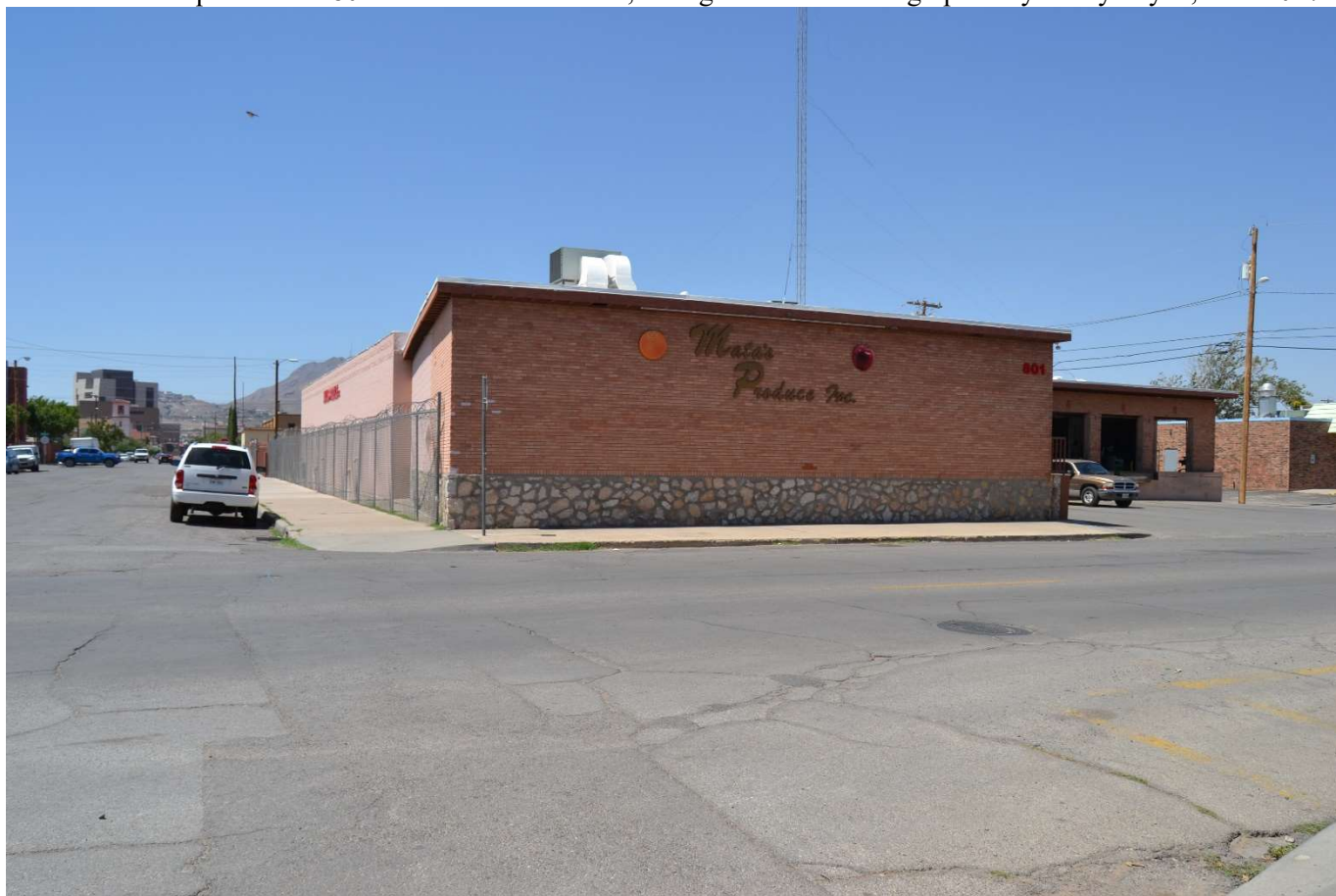
Photo 44. Oblique view of 801 East Seventh Avenue, facing northeast. Photographed by Emily Payne, June 2017.
