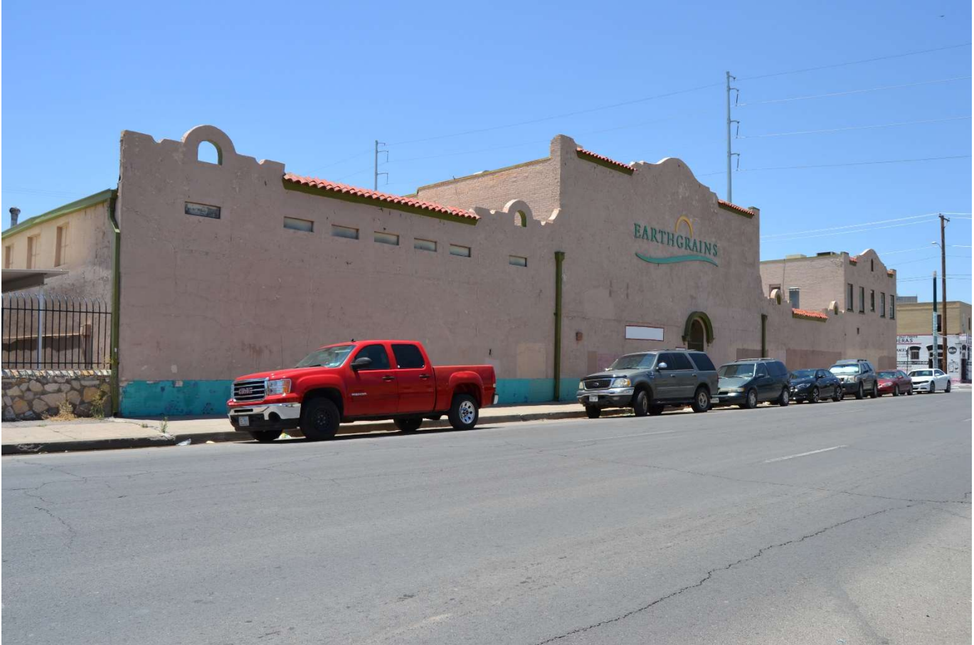
Photo 43. Oblique view of the Purity Baking Company (later the Rainbow Baking Company, now Earth Grains), 701 South Kansas Street, facing northwest. Photographed by Emily Payne, June 2017.
