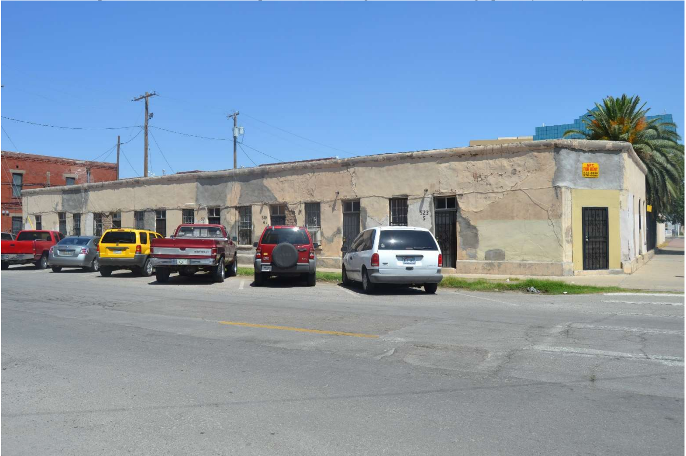
Photo 52. Oblique view of 415 South Campbell Street, facing northwest. Photographed by Erin Tyson, June 2017.
