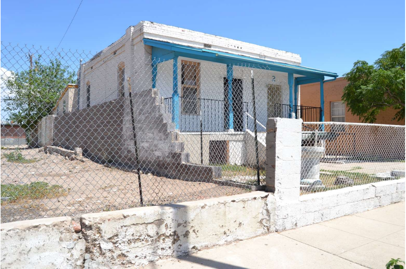
Photo 55. Oblique view of 710 South St. Vrain Street, facing southeast. Photographed by Kristina Kupferschmid, June 2017.
