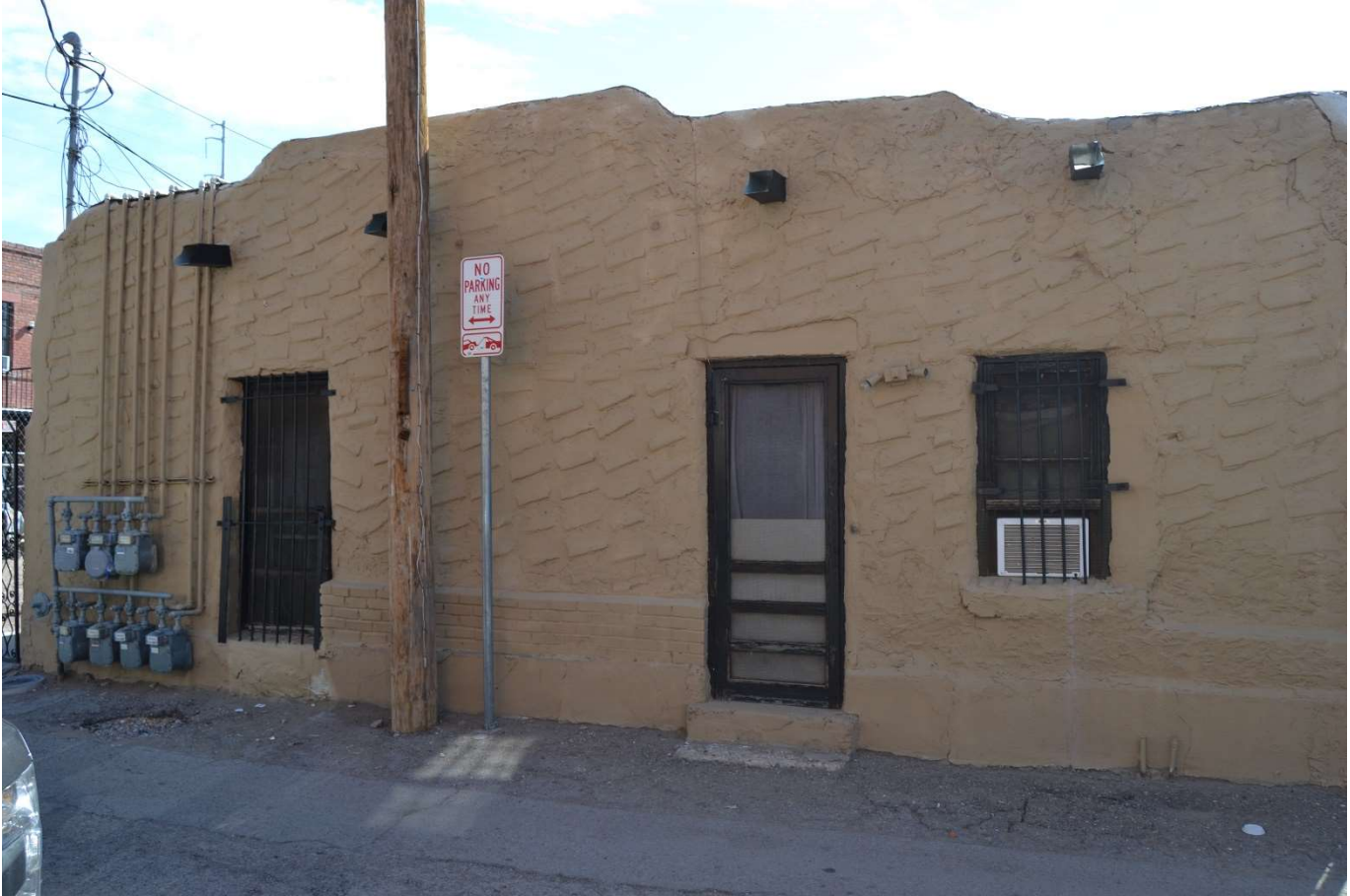
Photo 11. Oblique view of the alley dwelling at the rear of 715 South Oregon Street (fronting Alley E), facing east-northeast. Photographed by Shonda Mace, August 2017.
