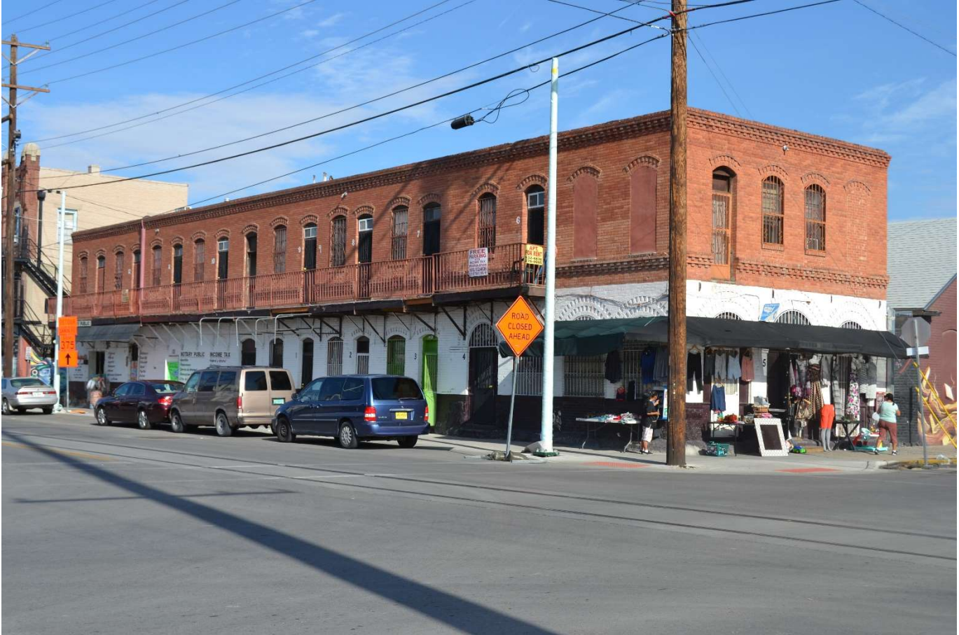
Photo 57. Oblique view of 621 South Oregon Street, facing northwest. Note post-railroad brick detailing at window cornices and parapet reflecting Territorial Revival stylistic influences. Photographed by Shonda Mace, July 2017.
