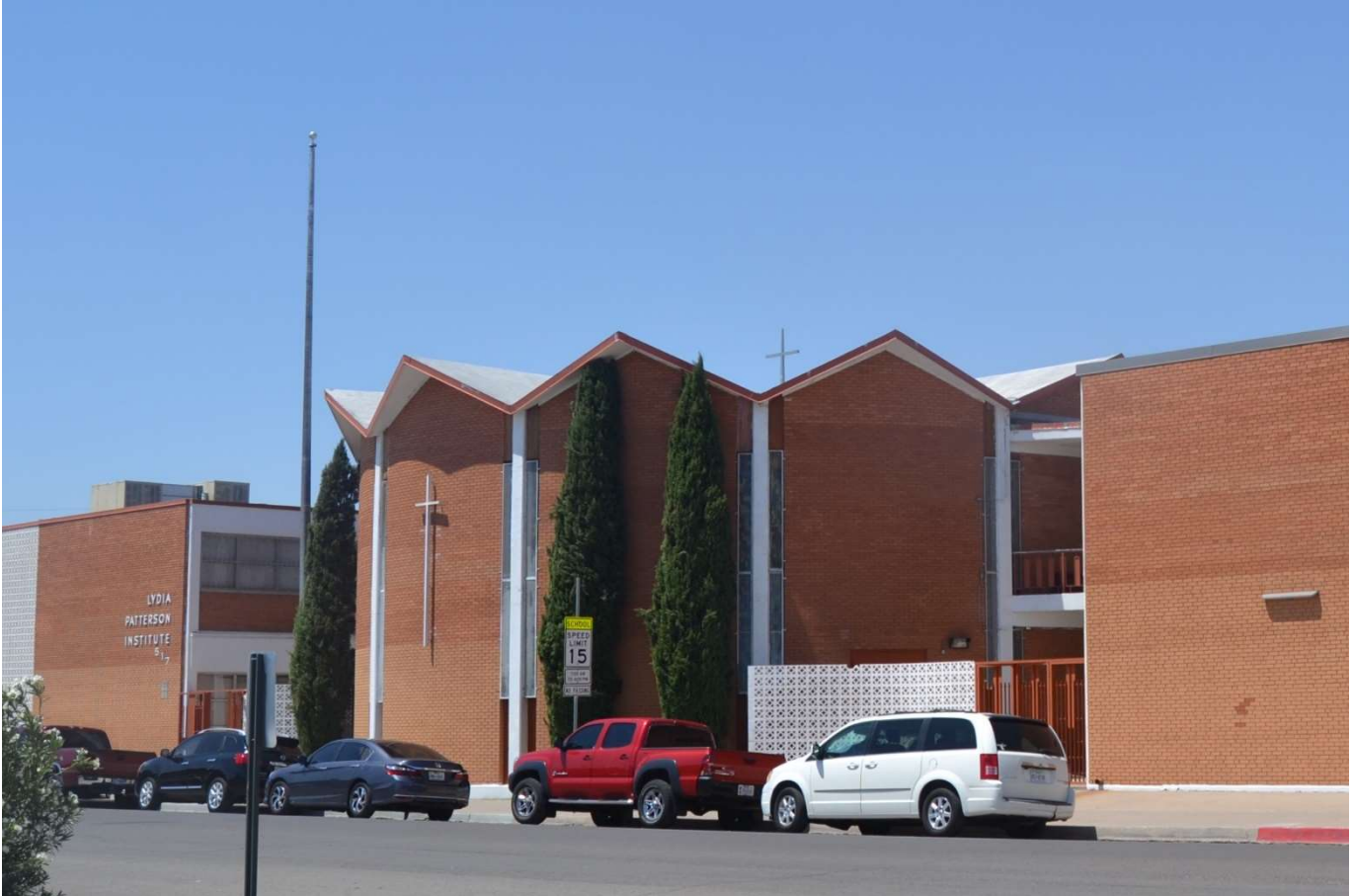
Photo 16. Oblique view of the Lydia Patterson Institute, 517 South Florence Street, facing southwest. Photographed by Erin Tyson, June 2017.
