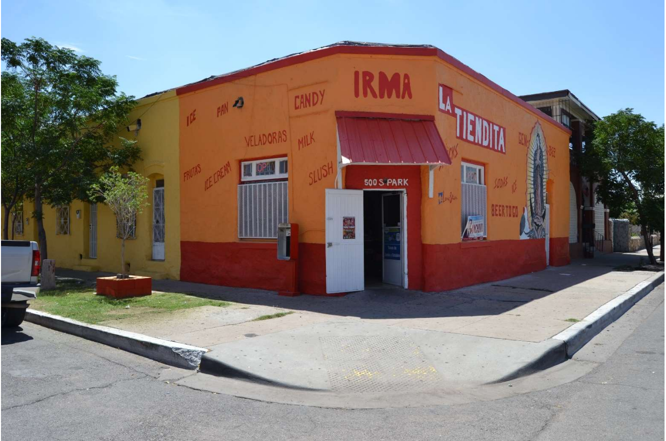
Photo 33. Oblique view of 1310 East Third Avenue, facing southeast. Photographed by Kristina Kupferschmid, July 2017.
