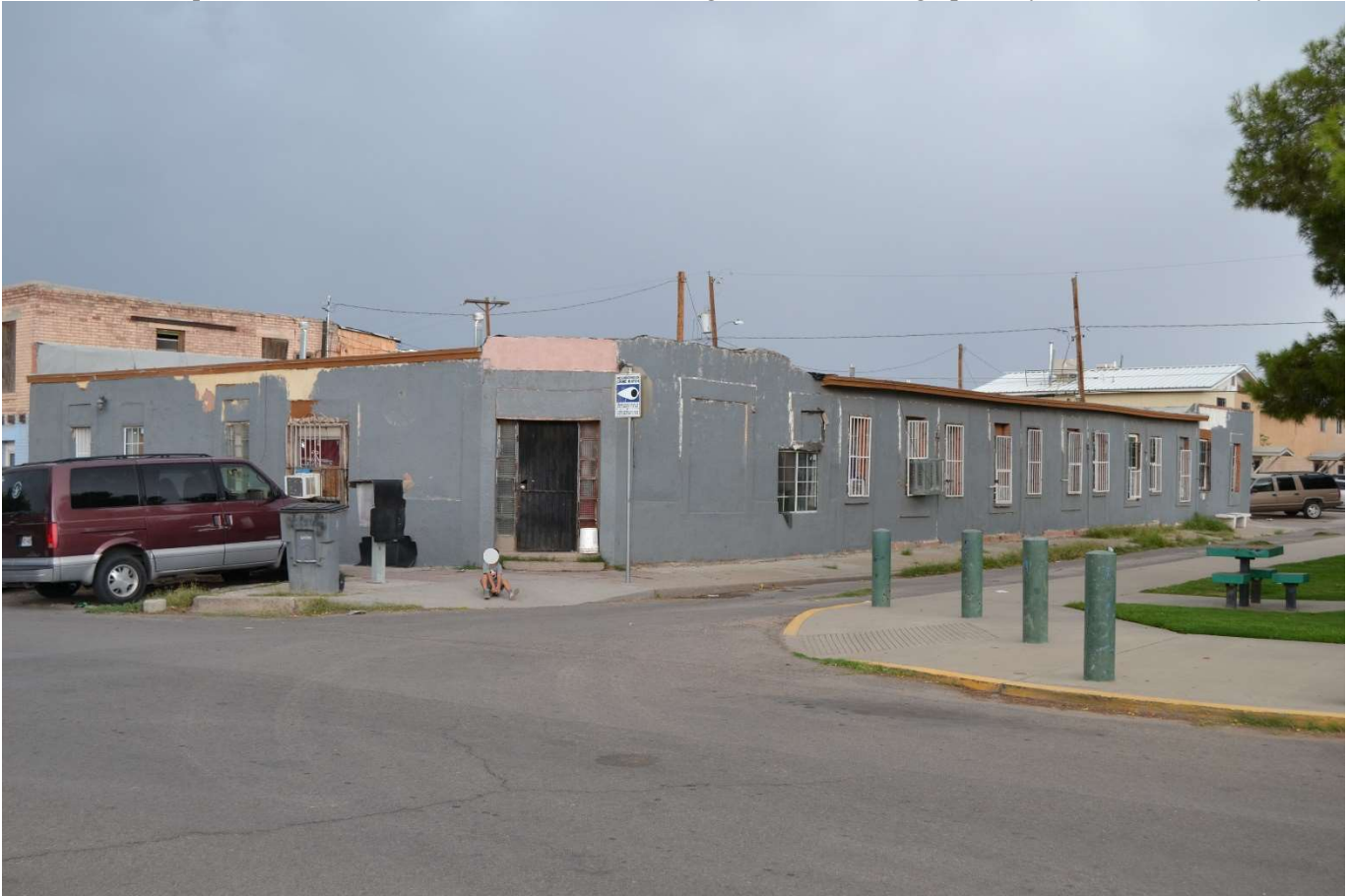
Photo 64. Oblique view of 918 South St. Vrain Street, facing northeast. Photographed by Shonda Mace, July 2017.
