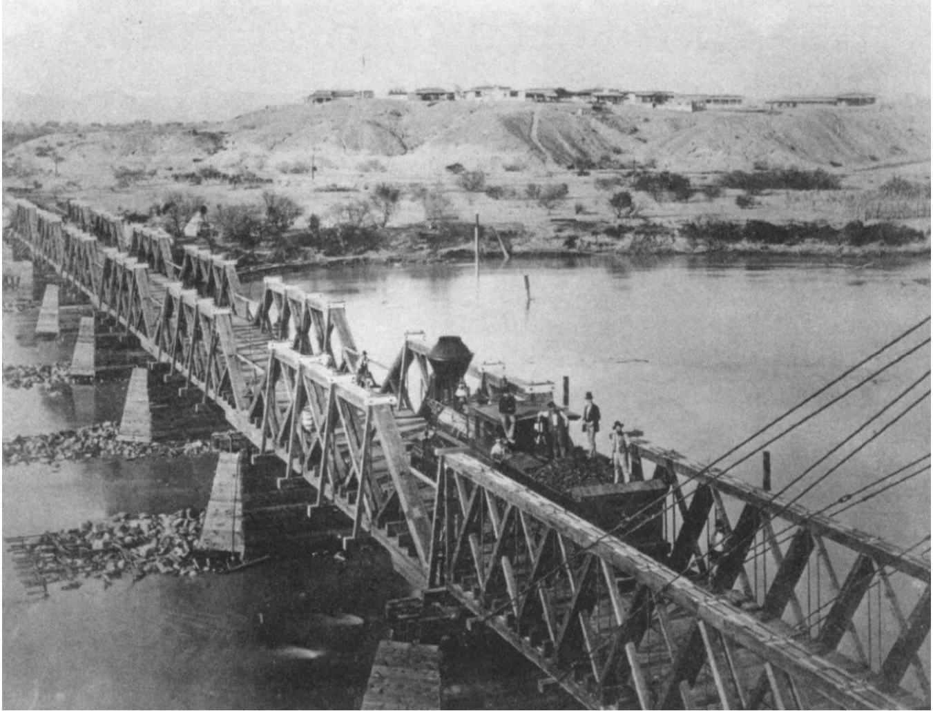
Figure 15. Photo of the international railroad bridge across the Rio Grande in 1881. Source: University of Texas at El Paso Library, special Collections Department, Laurence Stevens Papers, photo # MS1·14, reproduced in Hodges, "Bridges across the Borderline," 27.
