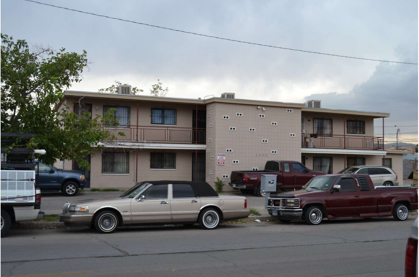
Photo 77. Oblique view of 1020 East Seventh Avenue, facing southwest. Photographed by Shonda Mace, July 2017.
