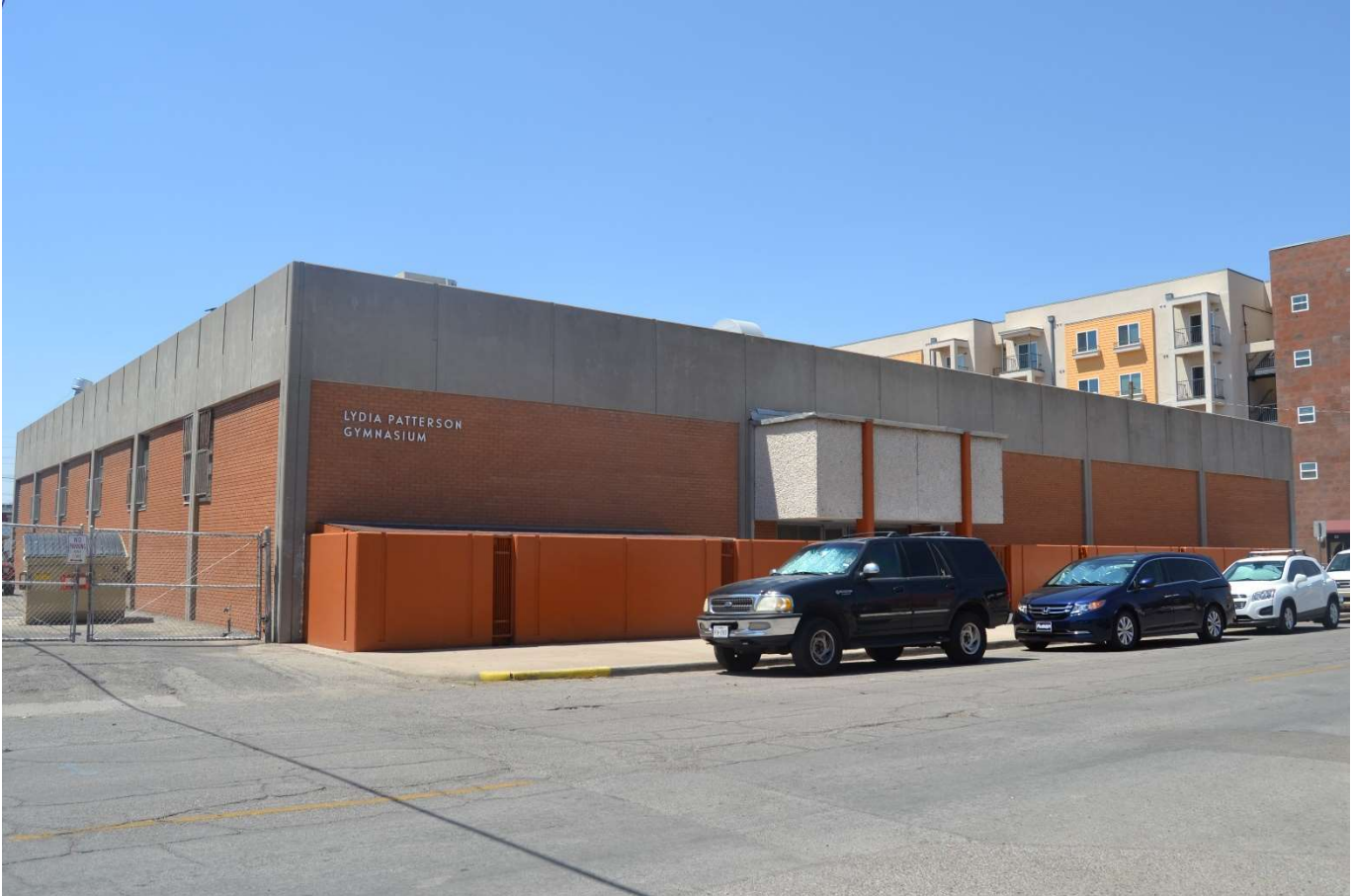
Photo 17. Oblique view of the Lydia Patterson Gymnasium, rear of 517 South Florence Street (fronting East Third Avenue), facing southeast. Photographed by Kristina Kupferschmid, September 2017.
