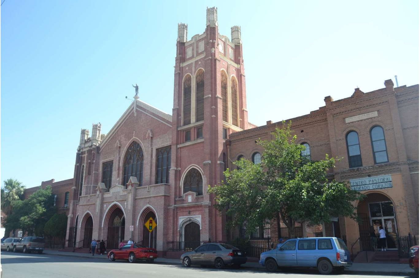
Photo 39. Oblique view of Sacred Heart Church sanctuary 1892 (altered 1923), 602 South Oregon Street, facing northeast. Photographed by Erin Tyson, June 2017.
