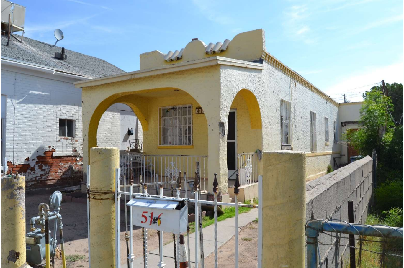
Photo 20. Oblique view of 516 Nino Aguilera Street, facing northeast. Photographed by Kristina Kupferschmid, July 2017.
