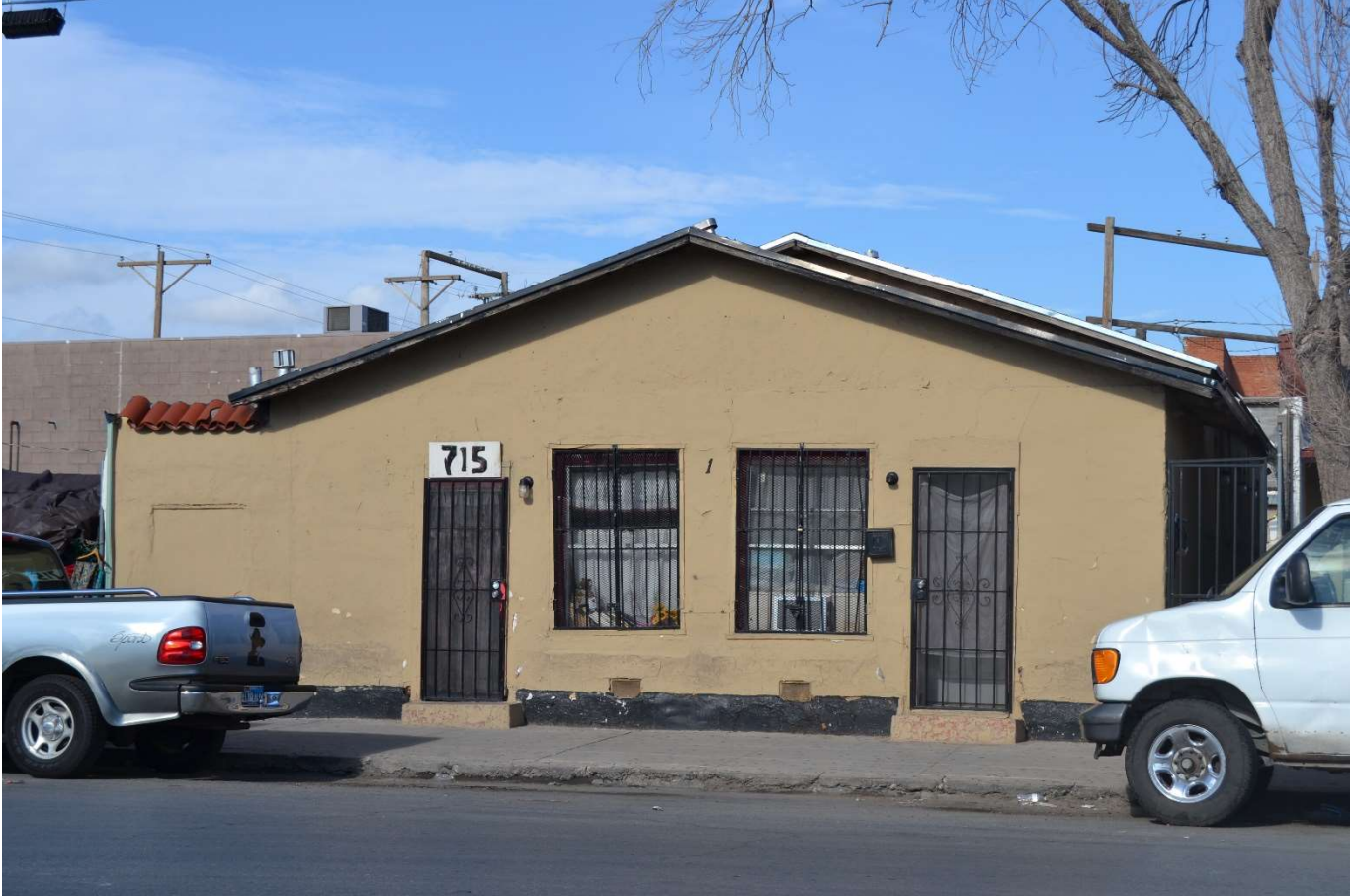
Photo 10. Oblique view of 715 South Oregon Street, facing southwest. Photographed by Shonda Mace, August 2017.
