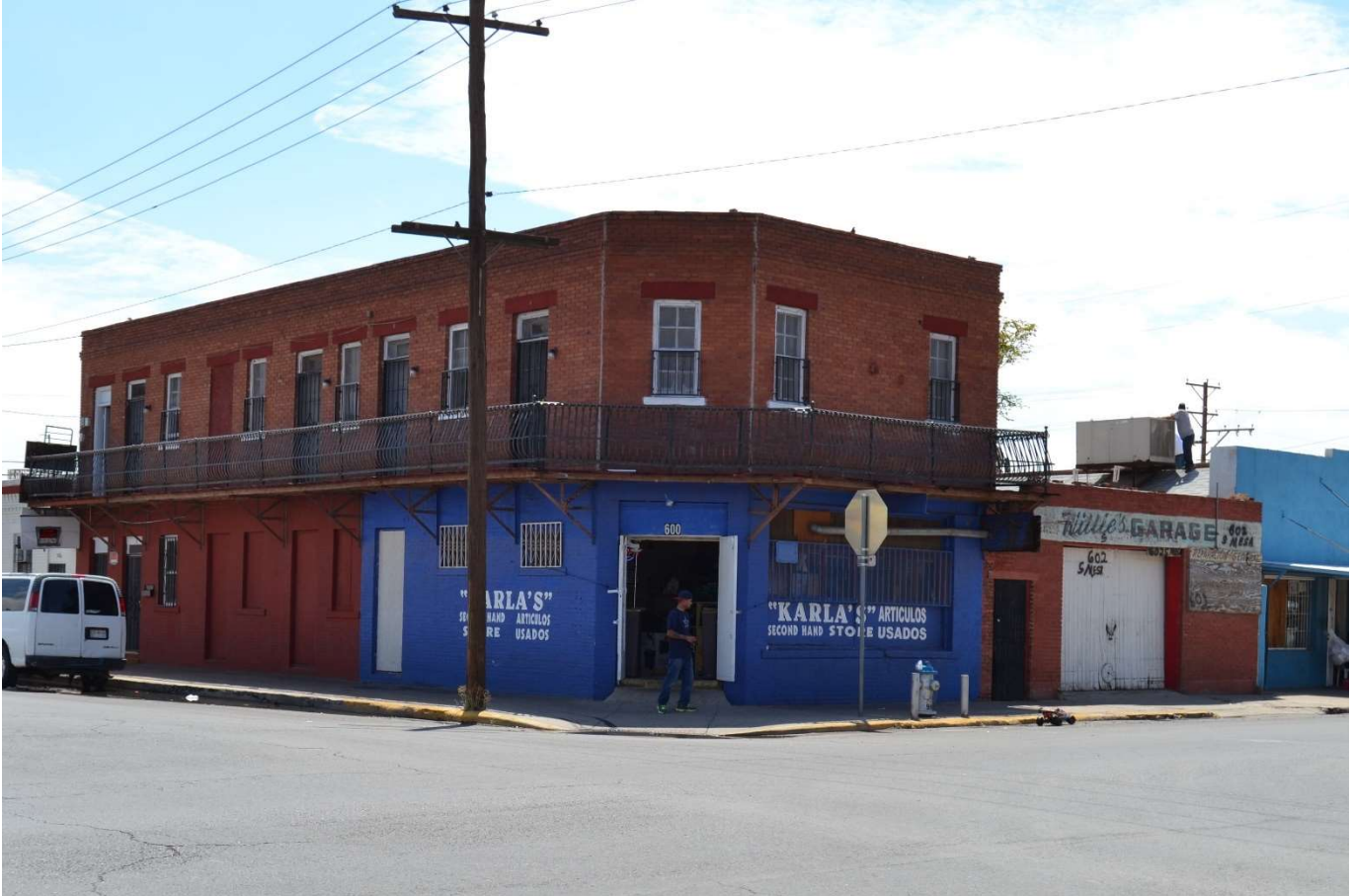
Photo 32. Oblique view of 600 South Mesa Street, facing southeast. Photographed by Kristina Kupferschmid, August 2017.
