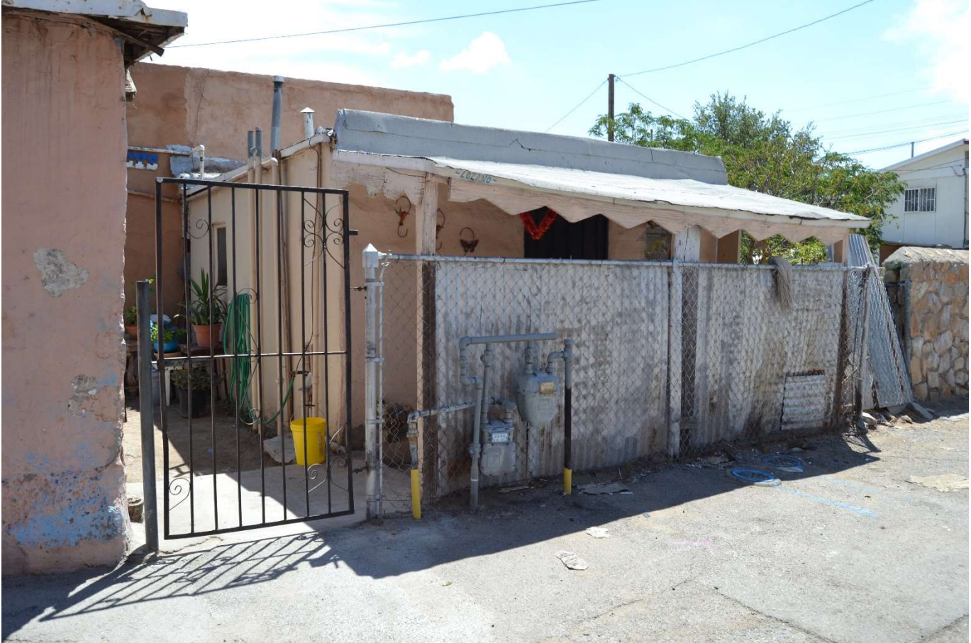
Photo 69. Oblique view of the one-room adobe rear dwelling at 607 South Ochoa Street (fronting the alley), facing southwest. Photographed by Kristina Kupferschmid, August 2017.
