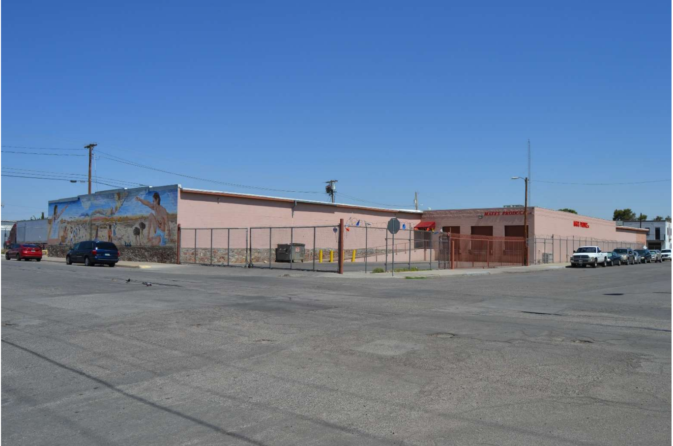
Photo 45. Oblique view of the rear of 801 East Seventh Avenue, facing southeast. Photographed by Emily Payne, June 2017.
