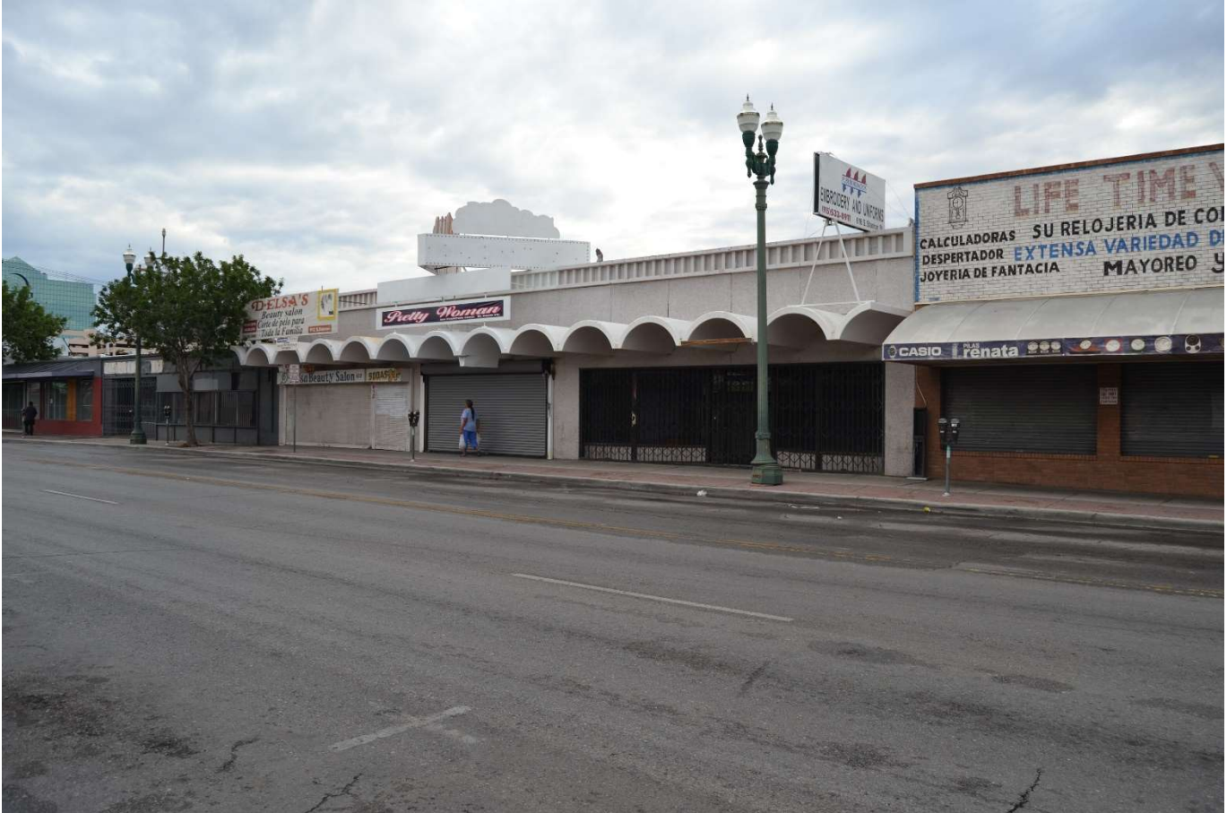
Photo 78. Oblique view of 612 South Stanton Street, facing northeast. Photographed by Kristina Kupferschmid, August 2017.
