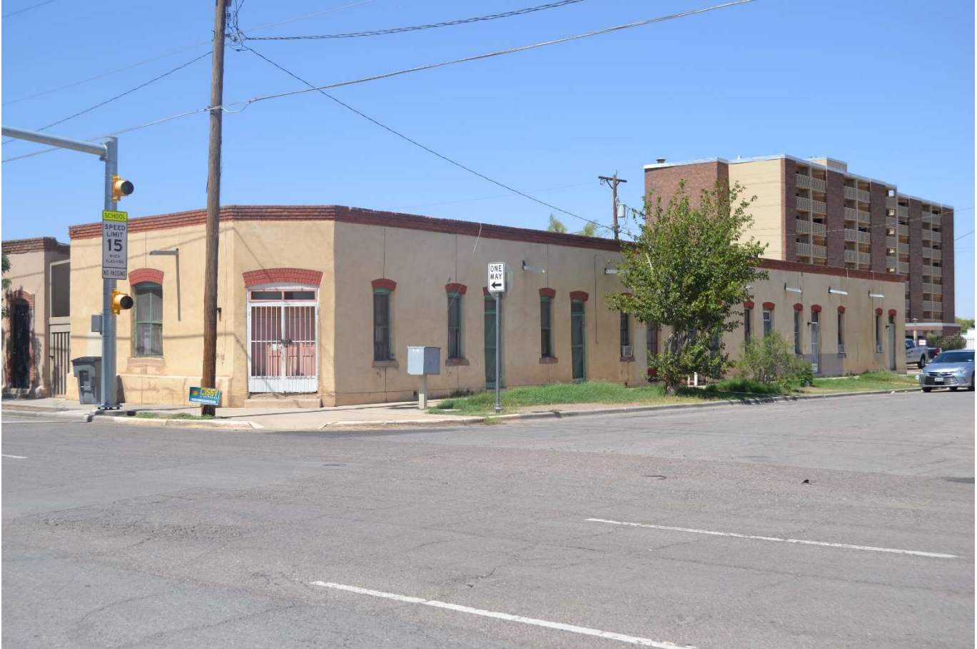
Photo 9. Oblique view of 1020 South Campbell Street, facing northeast. Photographed by Erin Tyson, June 2017.
