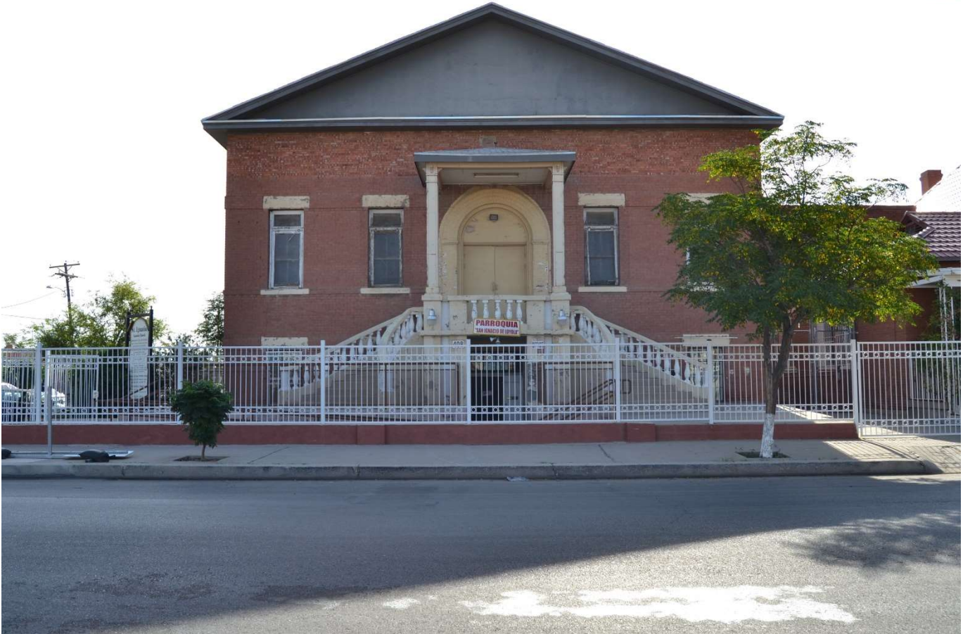
Photo 3. Façade view of St. Ignatius of Loyola Catholic Church and School (1905), 408 Park Street, facing east-northeast. Photographed by Kristina Kupferschmid, July 2017.
