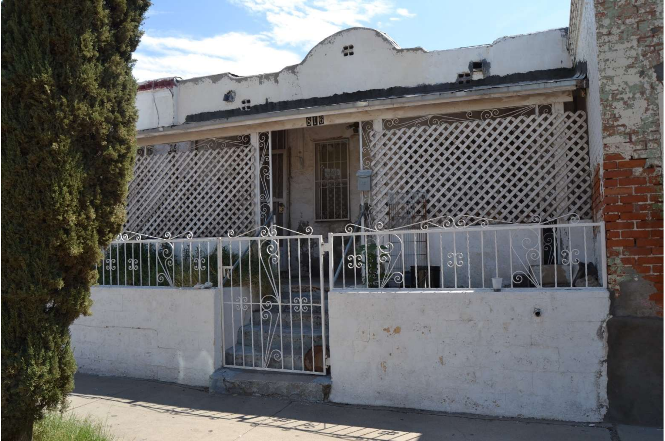
Photo 27. Oblique view of the residential unit at 818 South Hills Street, facing northeast. Photographed by Shonda Mace, July 2017.
