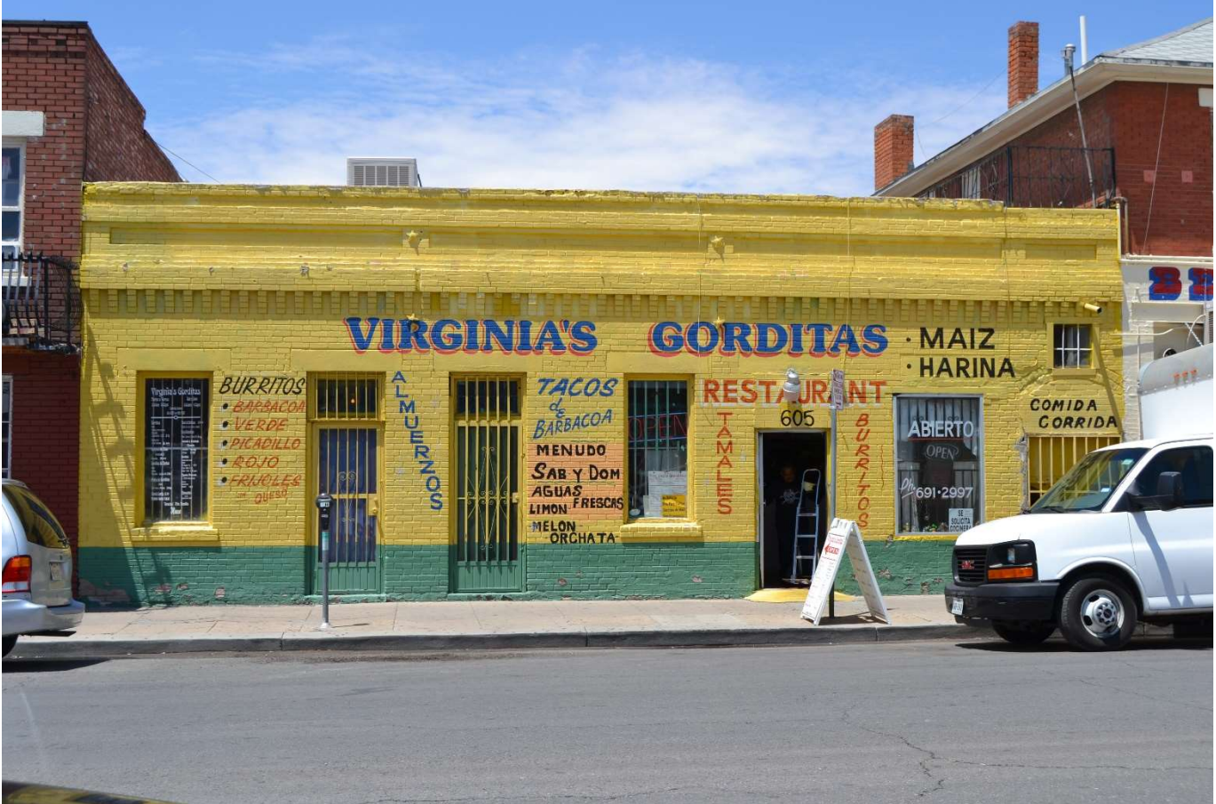
Photo 14. Façade view of 601 South Mesa Street (alternately addressed as 605 South Mesa Street), facing west-southwest. Photograph by Shonda Mace, August 2017.
