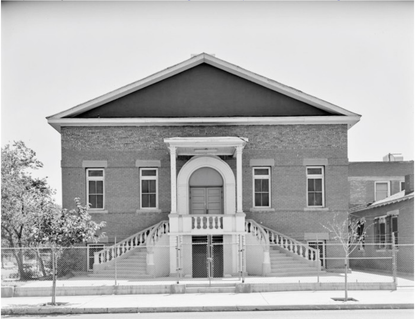
Figure 29. Photograph of the original portion of Saint Ignatius Catholic Church at 408 Park Street, constructed in 1904. Source: Texas Historical Commission, [Saint Ignatius], photograph, date unknown, The Portal to Texas History , crediting Texas Historical Commission, https://texashistory.unt.edu/ark:/67531/metaph680183/ .
