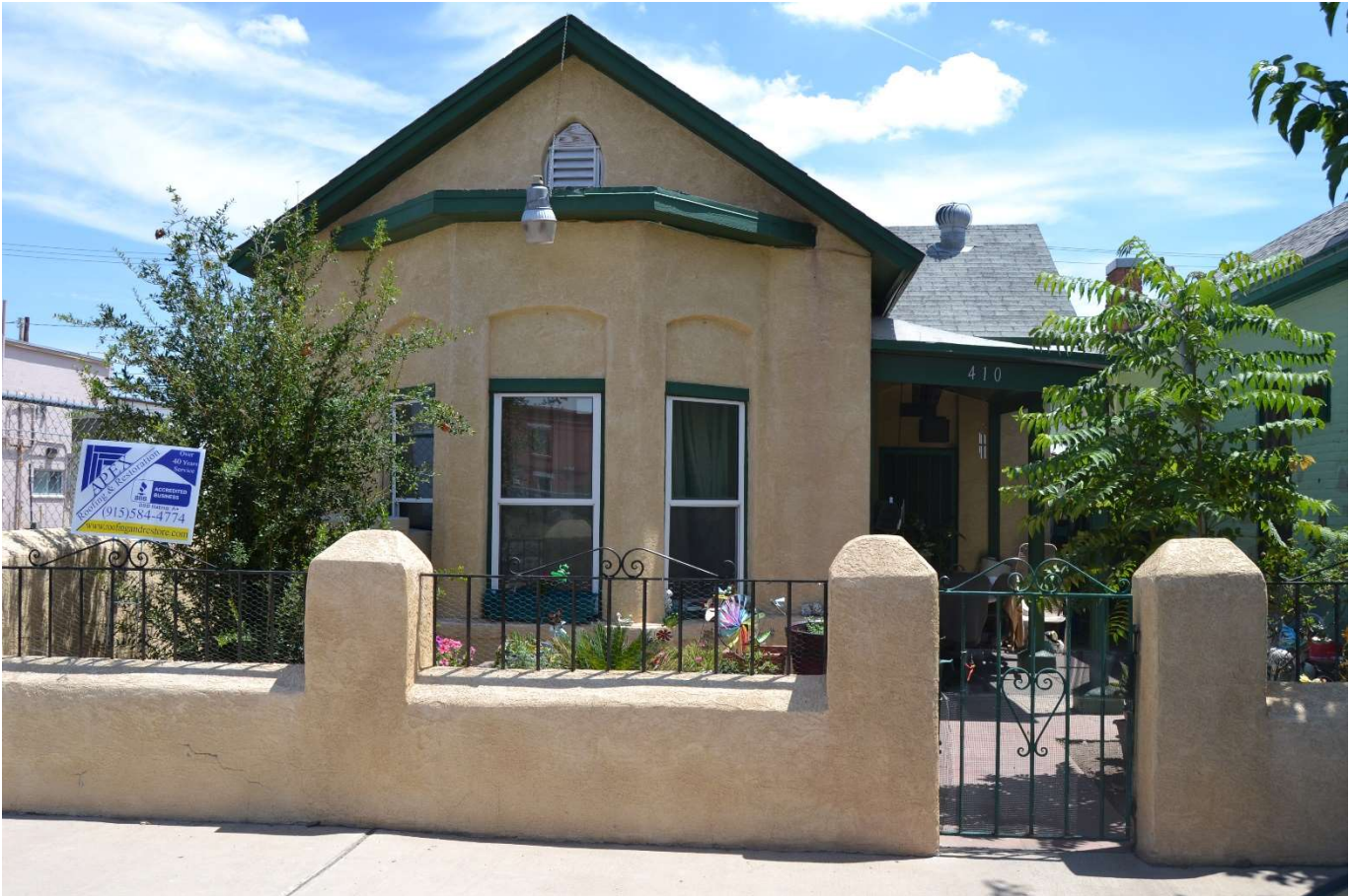
Photo 22. Façade view of 410 South Florence Street, facing east–northeast. Photographed by Emily Payne, June 2017.
