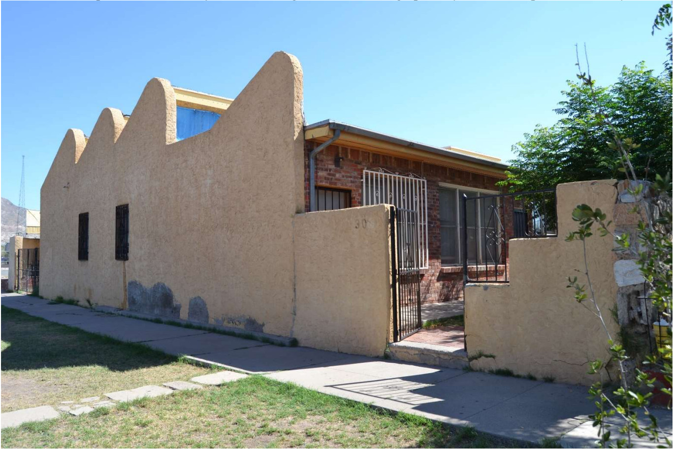
Photo 53. Oblique view of 306 Tays Street, facing northeast. Photographed by Kristina Kupferschmid, July 2017.
