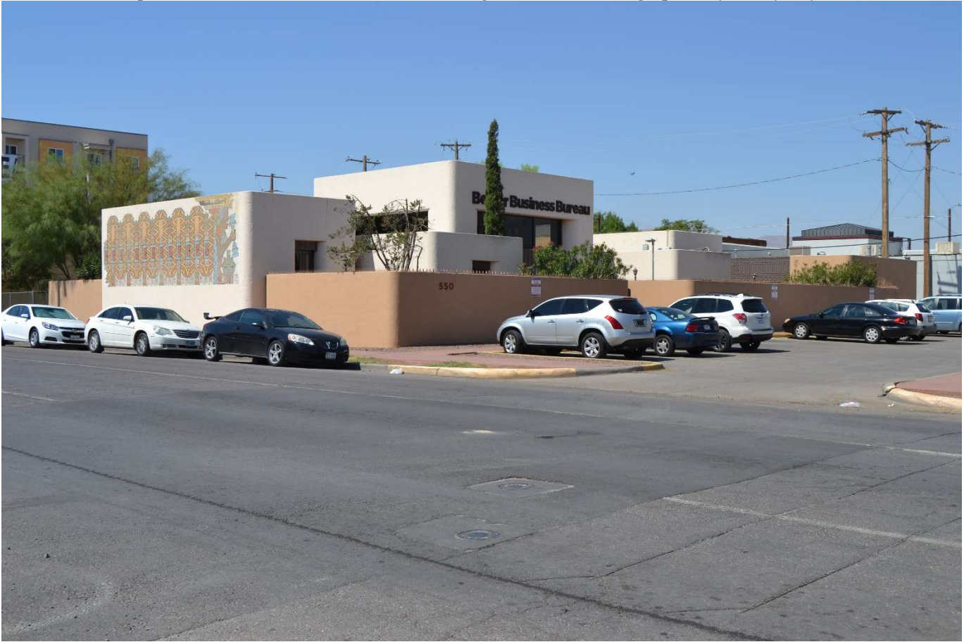
Photo 65. Oblique view of 550 East Paisano Drive, facing southwest. Photographed by Emily Payne, June 2017.
