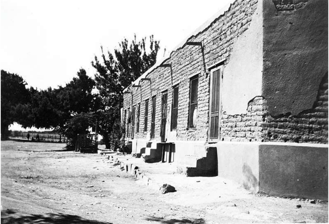
Figure 27. Photo of a typical adobe tenement in Segundo Barrio, no date (likely in the early twentieth century). Note that the precise location of this photo is not specified. Source: Palmore, "From Passage to Place."
