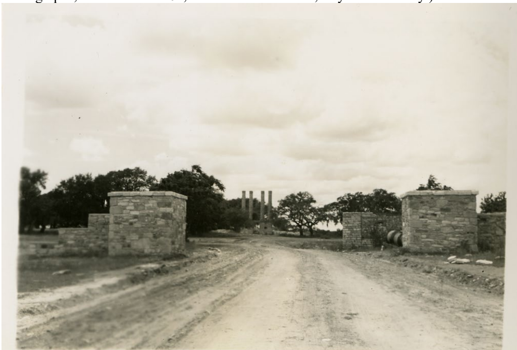
Figure 12: 1952 photograph of the east entrance of Academy Hill, the first floor of the boarding house ruin is located directly behind the right entrance gate and the academic building ruins are in the background. (BU Records: Photographs, Accession #22.01, The Texas Collection, Baylor University.)
