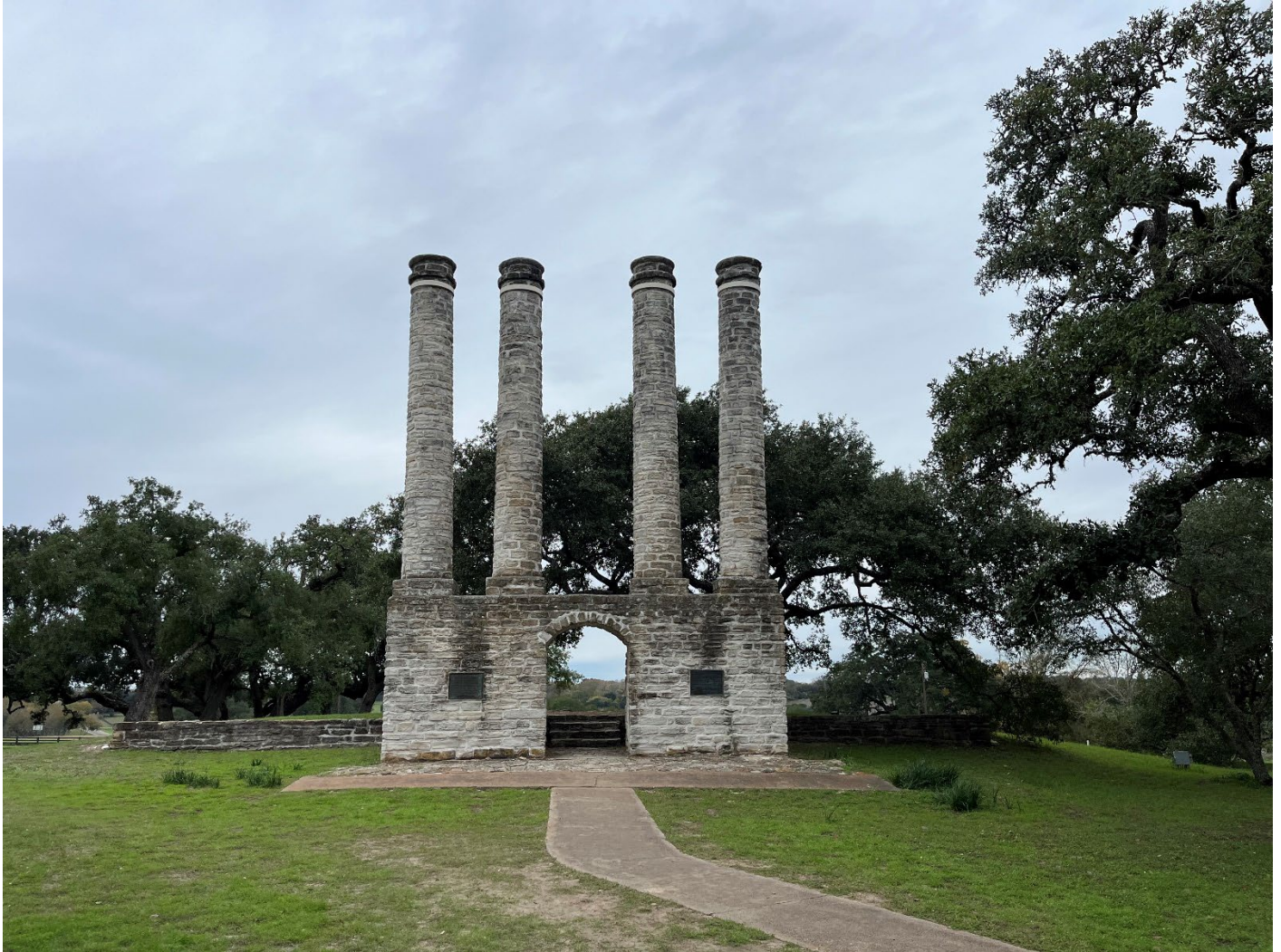
Photo 1: Academic building ruins (Contributing Resource 1, Feature A) frontal view facing west.
