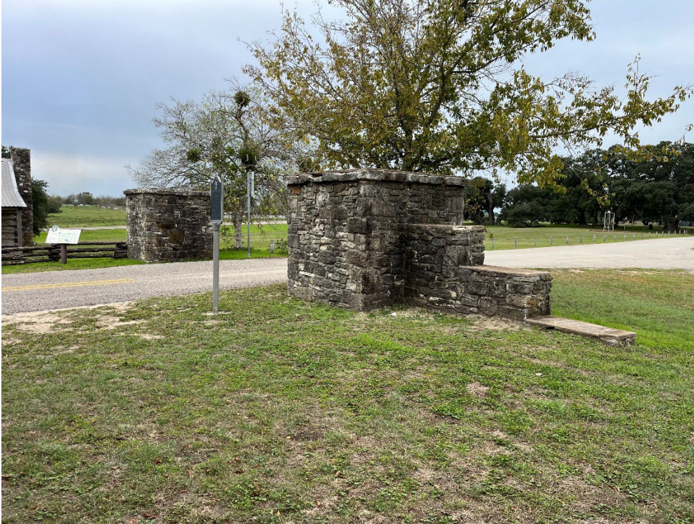
Photo 7: Entrance gate pillars (Non-Contributing Object, Resource 2), looking southwest.
