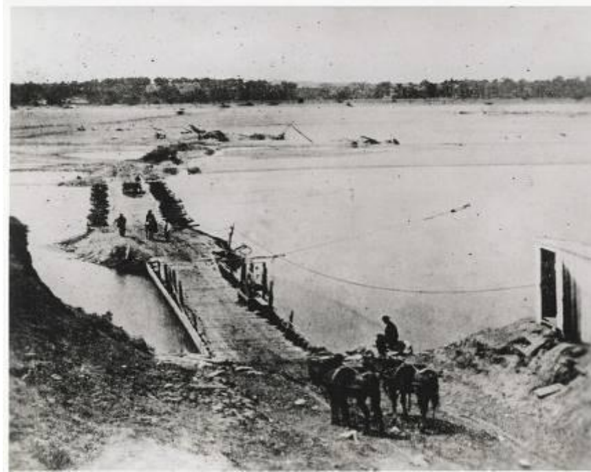
Figure 4: The first pontoon bridge was built in 1869 but they washed away with every flood. (Source: McGraw Marburger & Associates, 2002)
