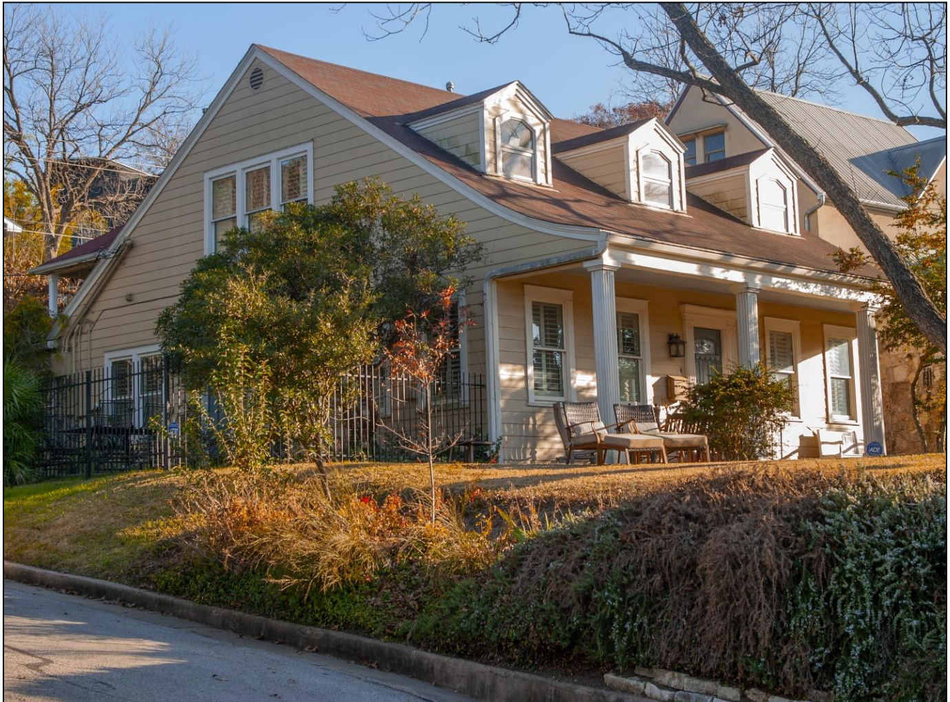
Photo 21: 1801 Alameda Drive – Contributing Building Colonial Revival: Side-Gabled Roof (Cape Cod) Oblique: West and north elevations, camera facing southeast Photographer: Melanie Martinez, January 9, 2020
