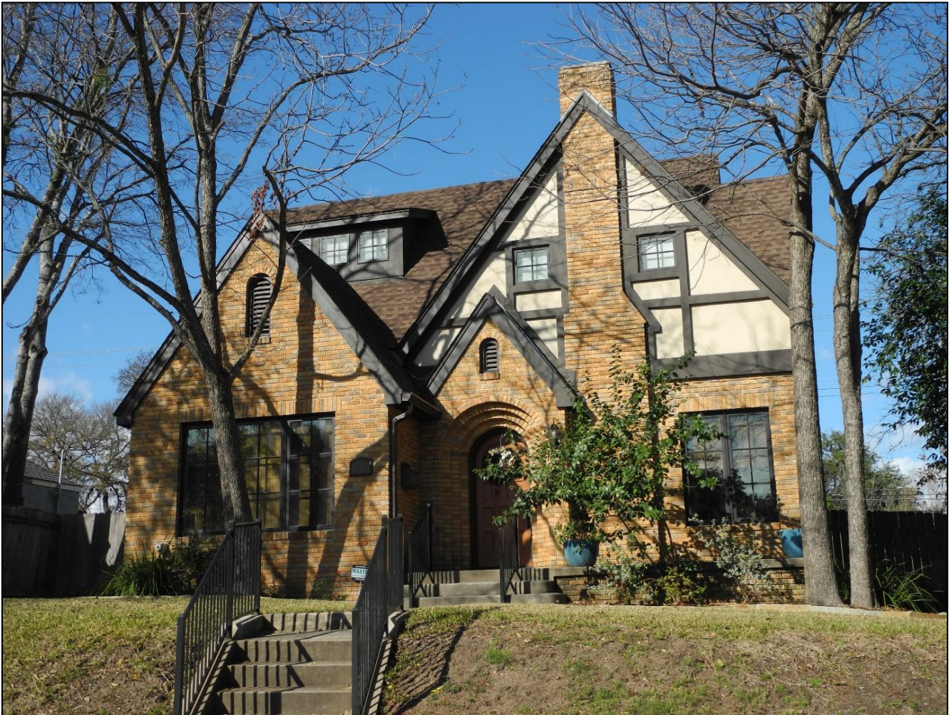
Photo 42: 1608 Travis Heights Blvd. – Noncontributing Building: Due to Alterations (Compatible) Tudor Revival: Multiple Façade Gables East elevation, camera facing west Photographer: Terri Myers, January 4, 2020
