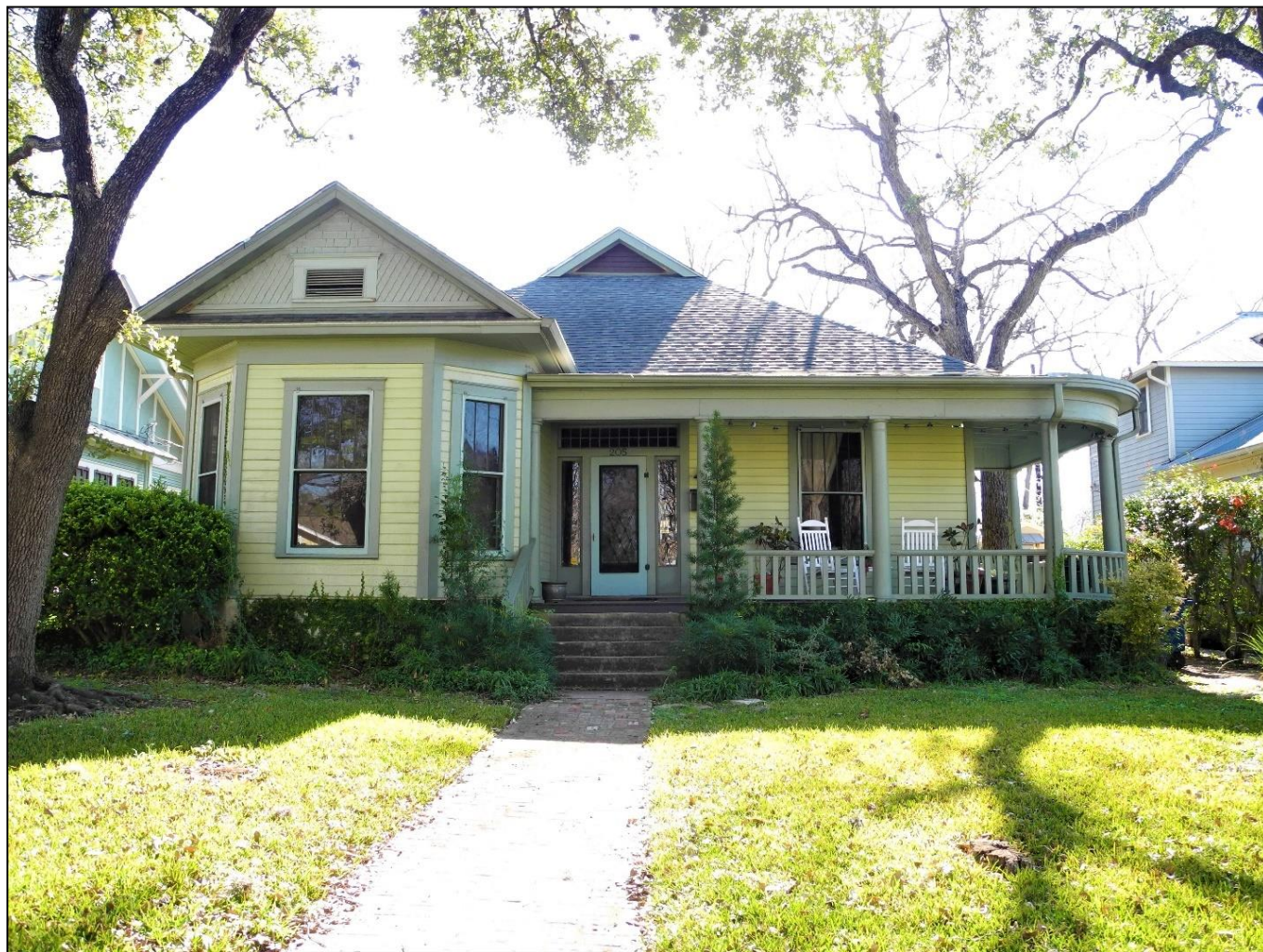
Photo 3: 205 E. Milton Street (Weyerman House) – Contributing Building Queen Anne: Free Classic North elevation, camera facing south Photographer: Terri Myers, January 24, 2020
