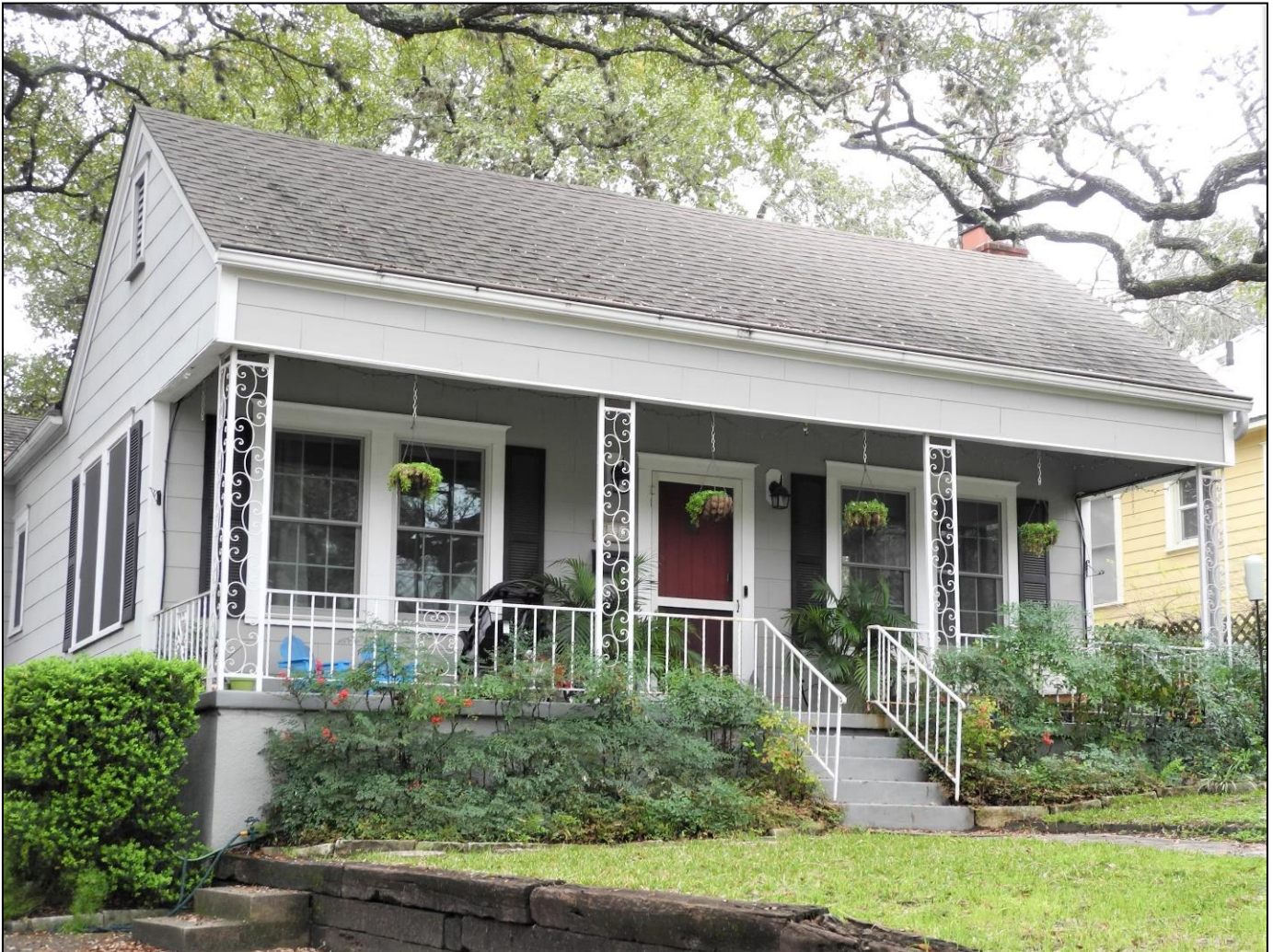
Photo 24: 517 E. Annie Street – Contributing Building Minimal Traditional: Side-Gabled Roof Oblique: North and east elevations, camera facing southwest Photographer: Terri Myers, March 10, 2020
