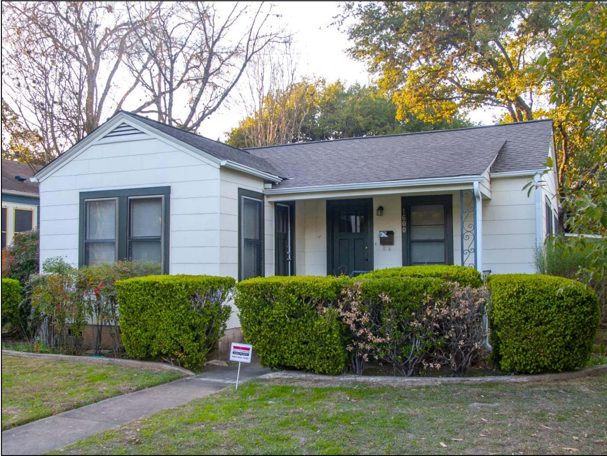
Photo 26: 1600 Travis Heights Blvd. – Contributing Building Minimal Traditional: Gable-and-Wing Roof Oblique: East and north elevations, camera facing southwest Photographer: Melanie Martinez, January 9, 2020
