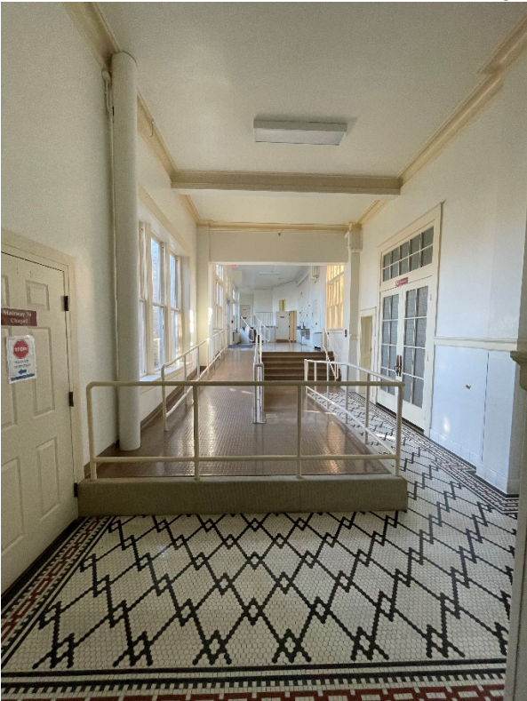
Photo 24: Ground level of south corridor looking south to convent entrance. Double doors (right) open to the auditorium.
