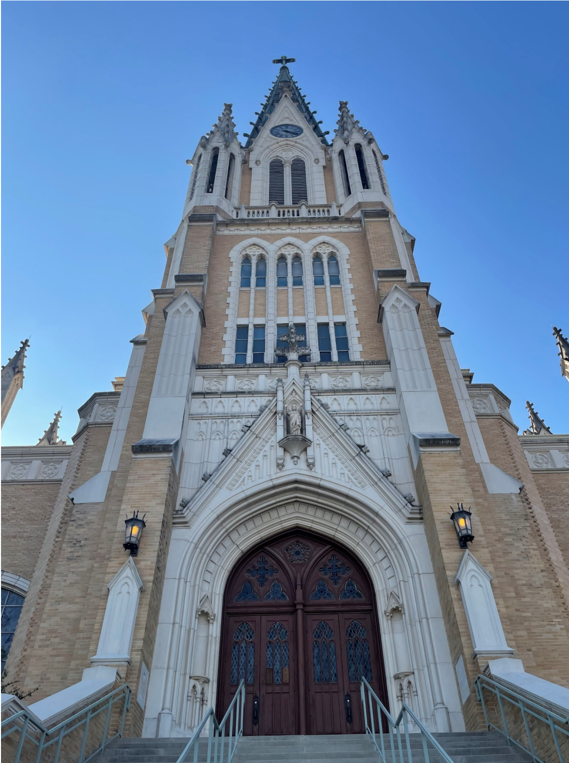
Photo 3: Chapel entrance detail, looking west.
