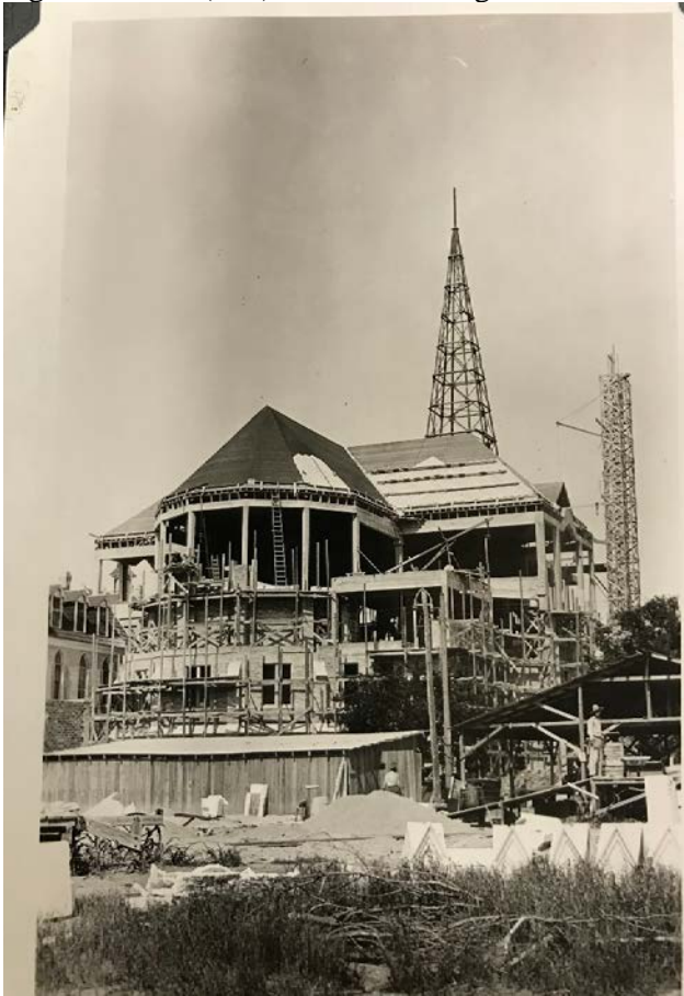
Figure 5: West (rear) elevation during construction. Source: Dielmann Papers, Col. 883.
