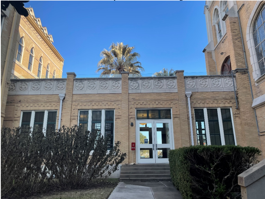
Photo 5: North corridor between Chapel and Main Building. View west.
