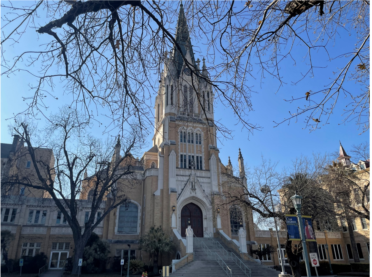
Photo 2: Sacred Heart Conventual Chapel. East (front) elevation, looking west.
