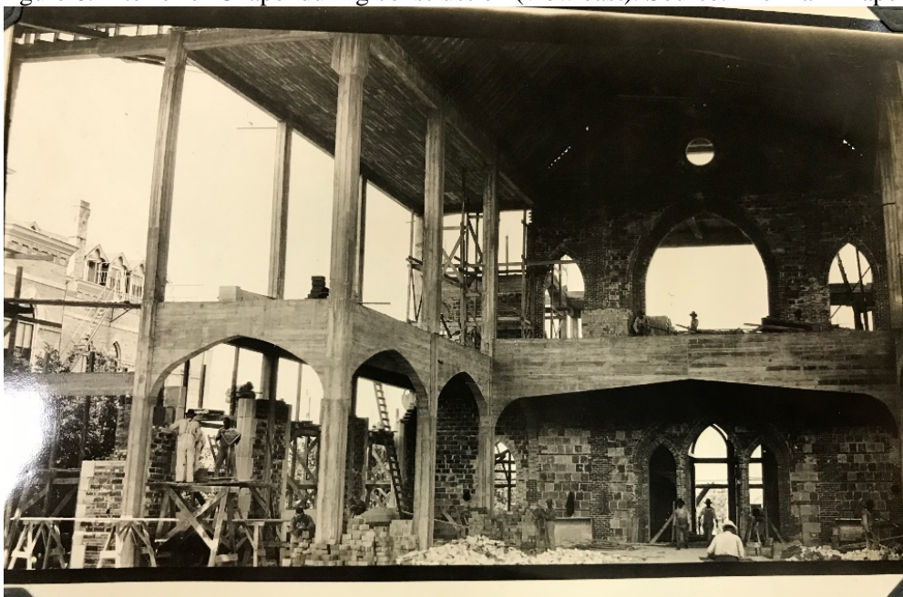
Figure 6: Interior of Chapel during construction (view east). Source: Dielmann Papers, Col. 883.
