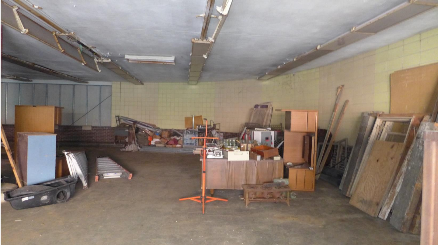
Photo 22 Motor bank entrance, camera facing south February 2021
