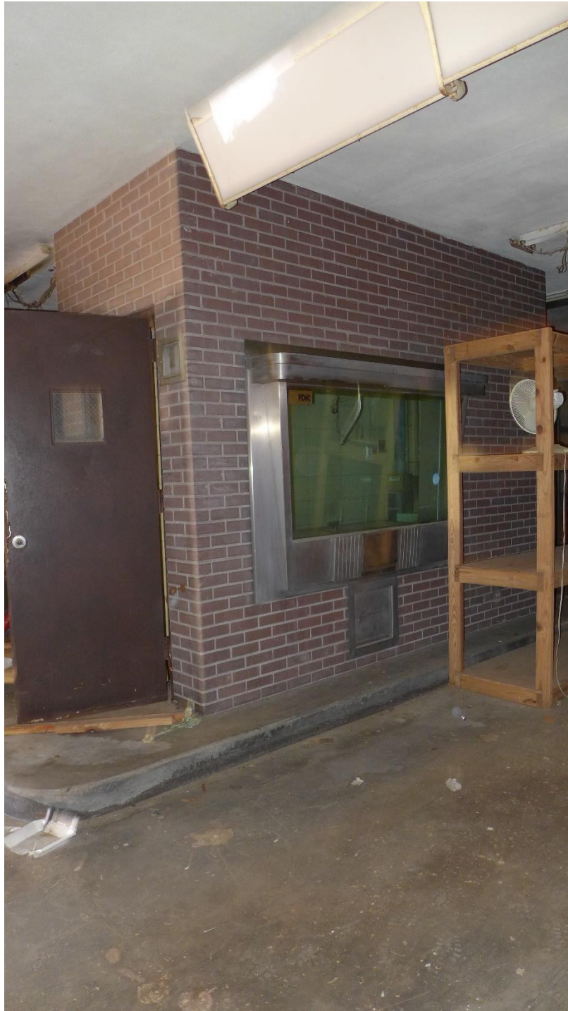
Photo 24 Drive-up teller window, camera facing northeast February 2021
