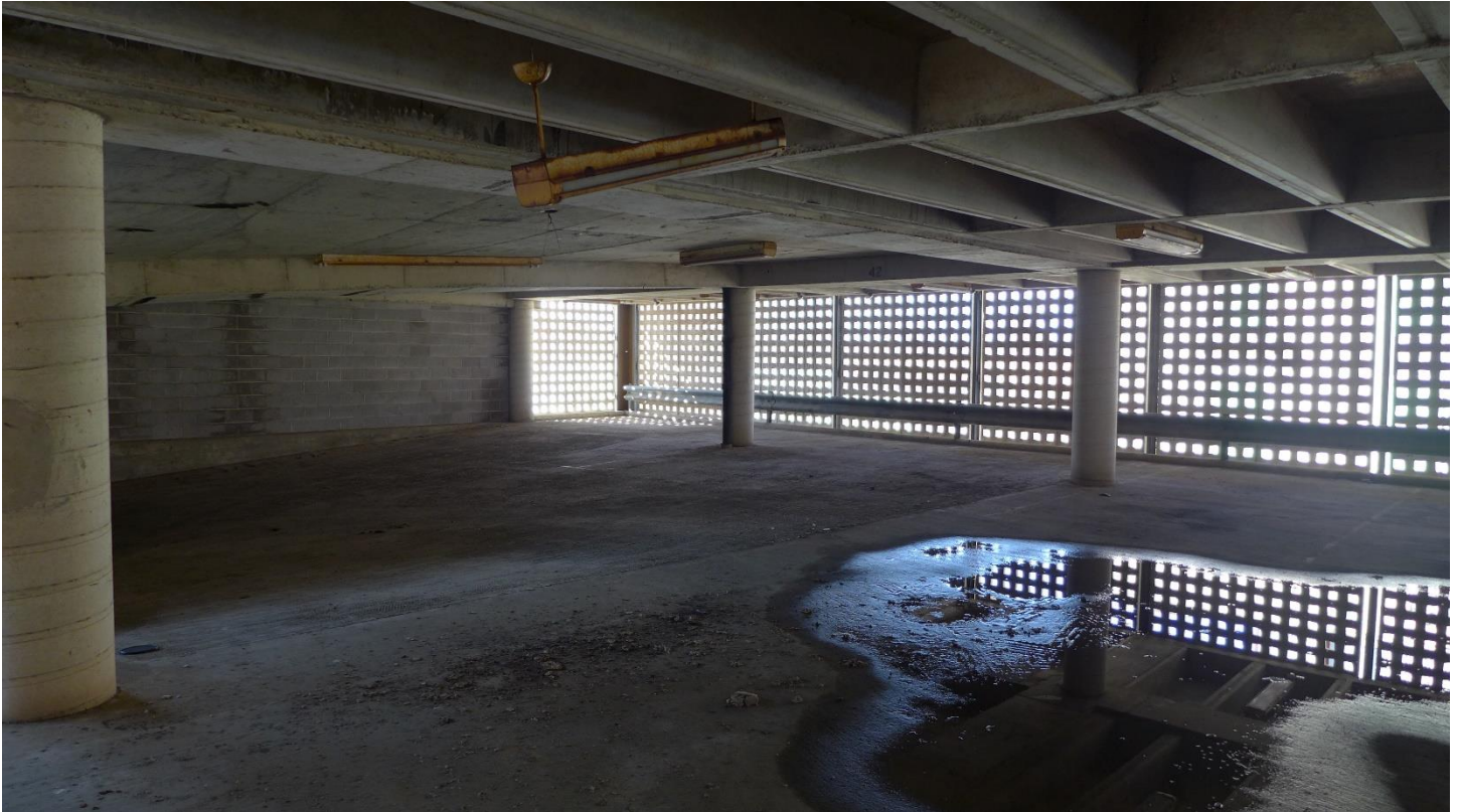
Photo 14 Typical garage upper level, camera facing northwest February 2021
