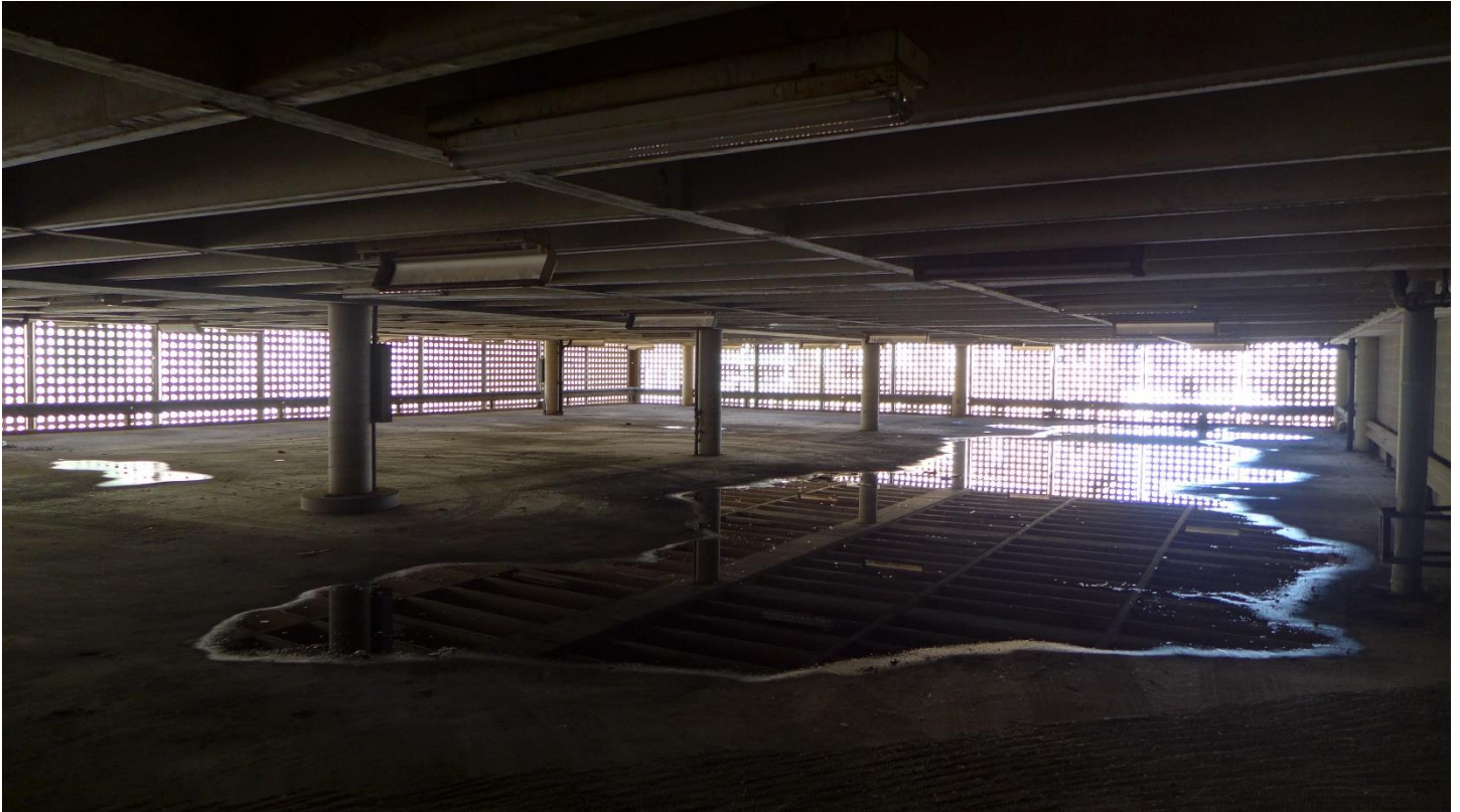
Photo 15 Typical garage upper level, camera facing northeast February 2021
