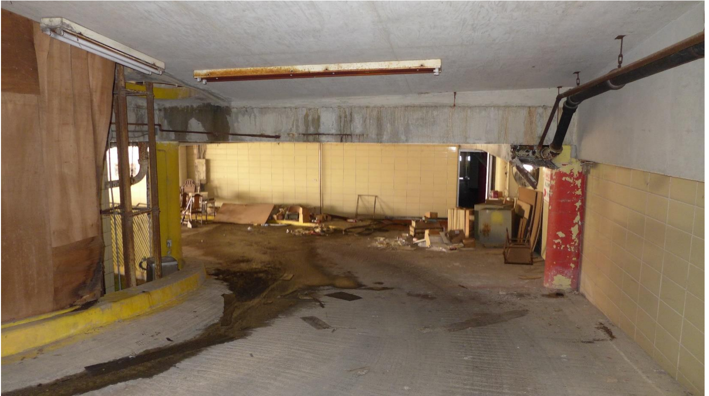
Photo 25 Garage entrance/exit bay, looking down ramp, camera facing north February 2021
