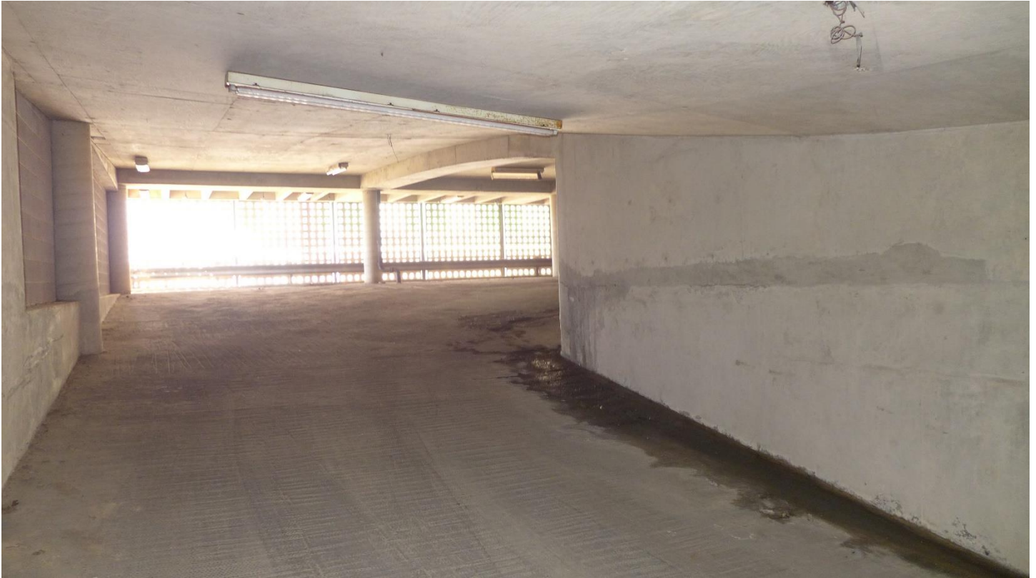
Photo 13 Parking garage ramp, level two, camera facing north September 2020
