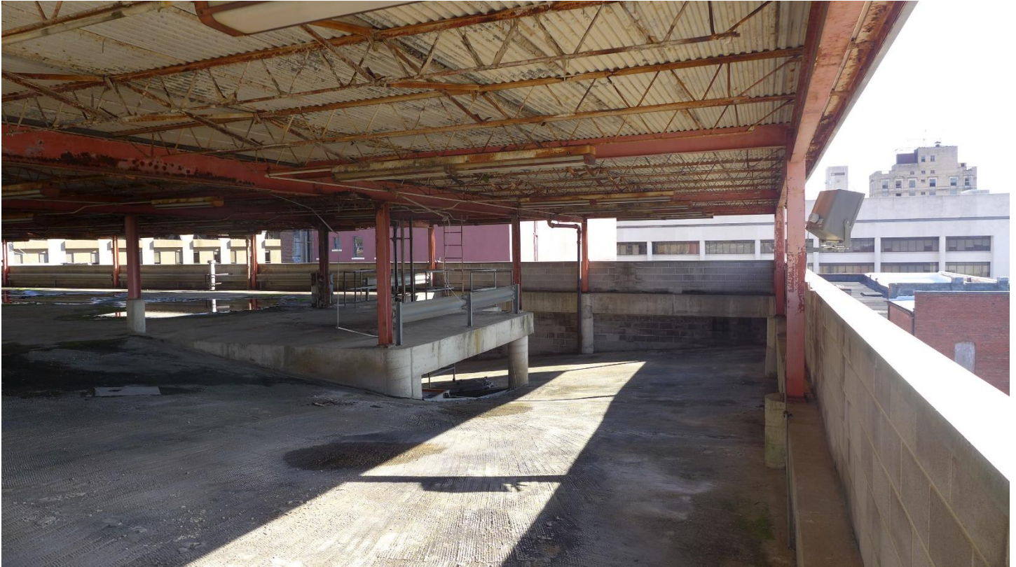
Photo 16 Garage top level, camera facing south February 2021
