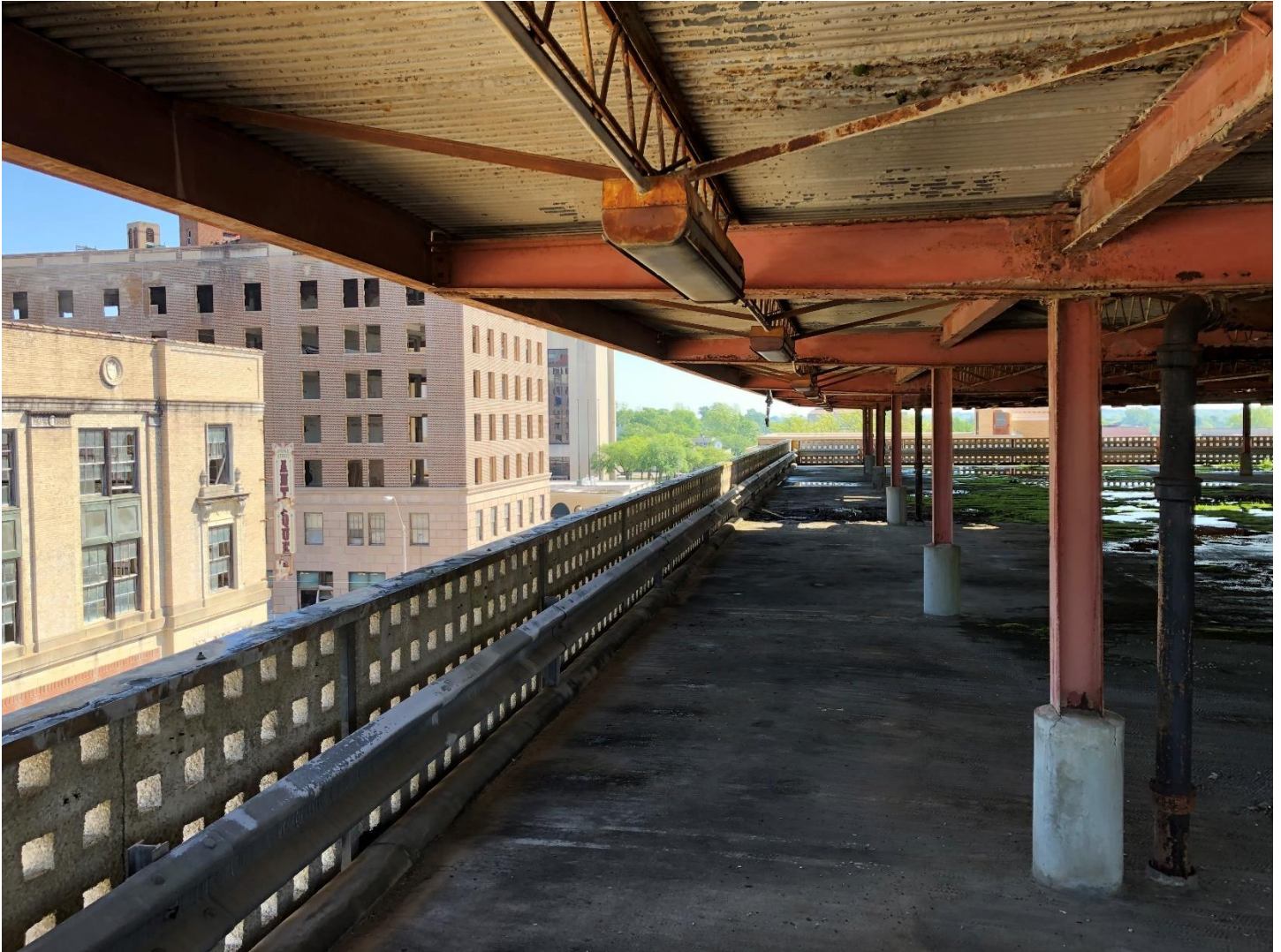
Photo 18 Garage top level, camera facing northeast February 2021
