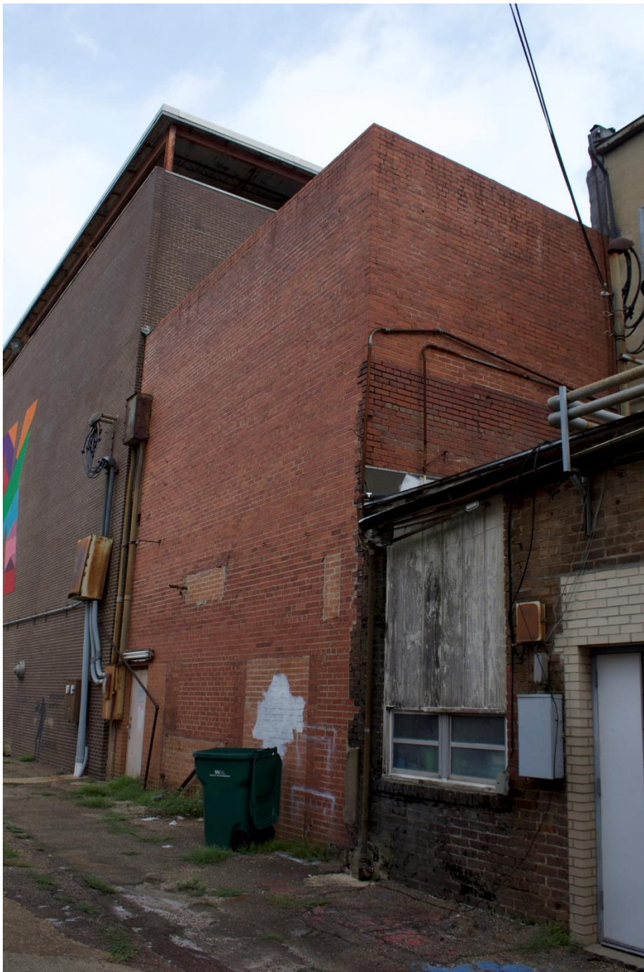
Photo 27 West Elevation of the 1962 Office Annex, camera facing northeast March 2021
