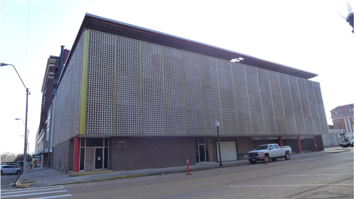
Photo 3 North elevation camera facing south January 2021
