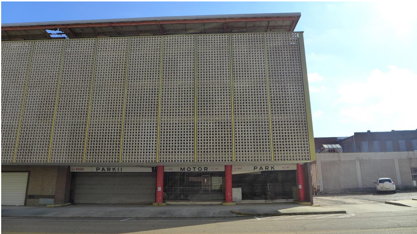
Photo 6 North elevation (west half), camera facing south February 2021
