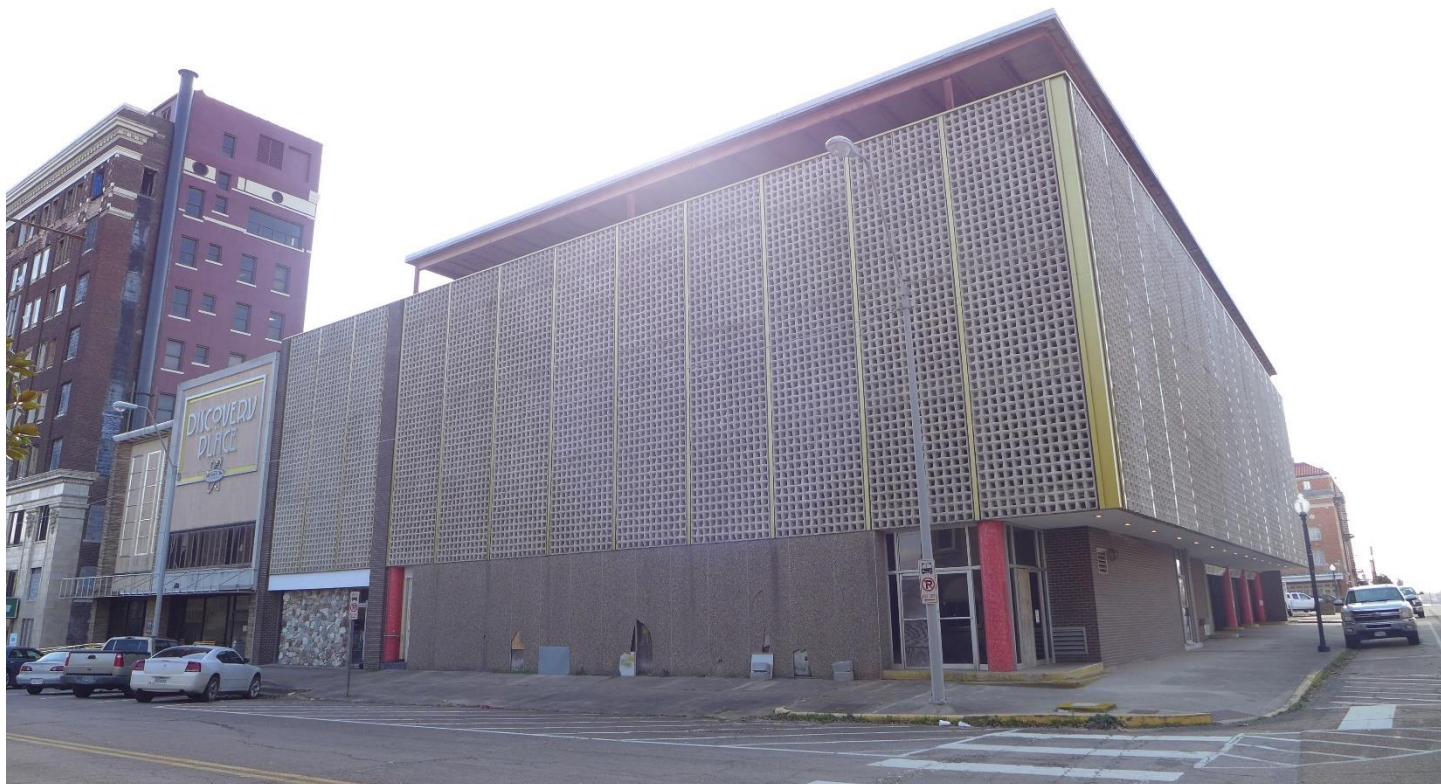
Photo 4 East elevation, camera facing southwest February 2021
