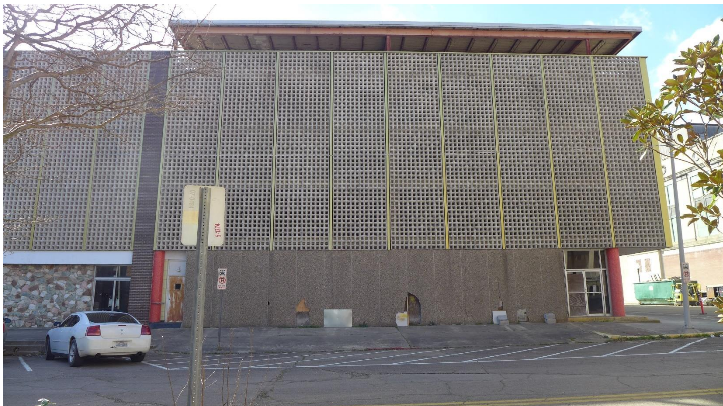
Photo 5 East elevation, camera facing west February 2021
