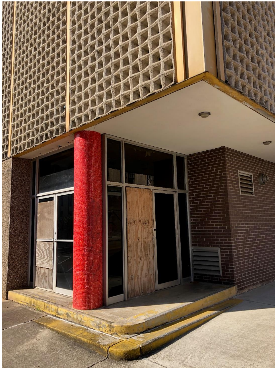
Photo 10 Street level corner entrance, camera facing southwest September 2020
