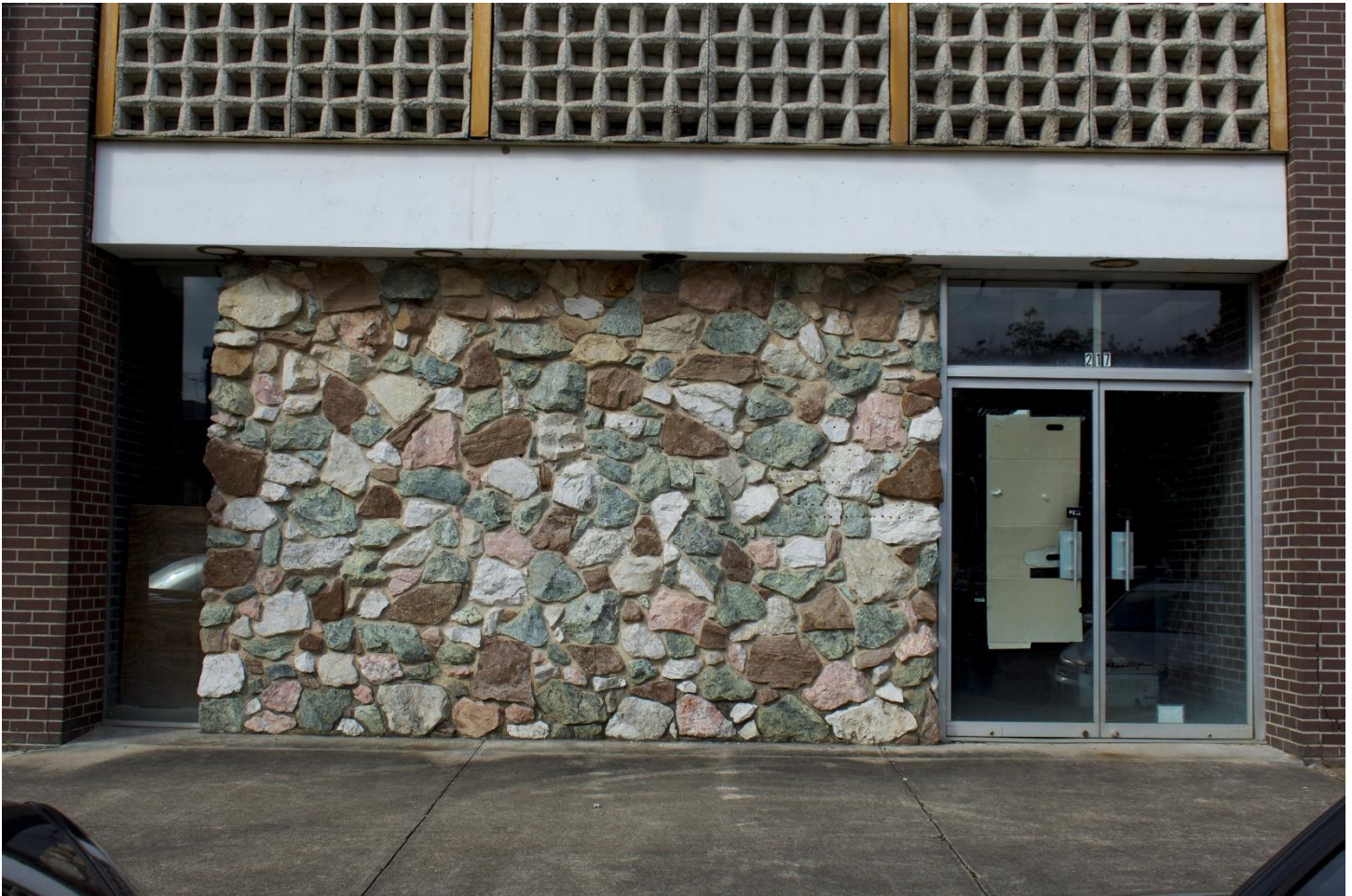
Photo 26 Pine Street entrance to the 1962 Office Annex, camera facing west September 2020
