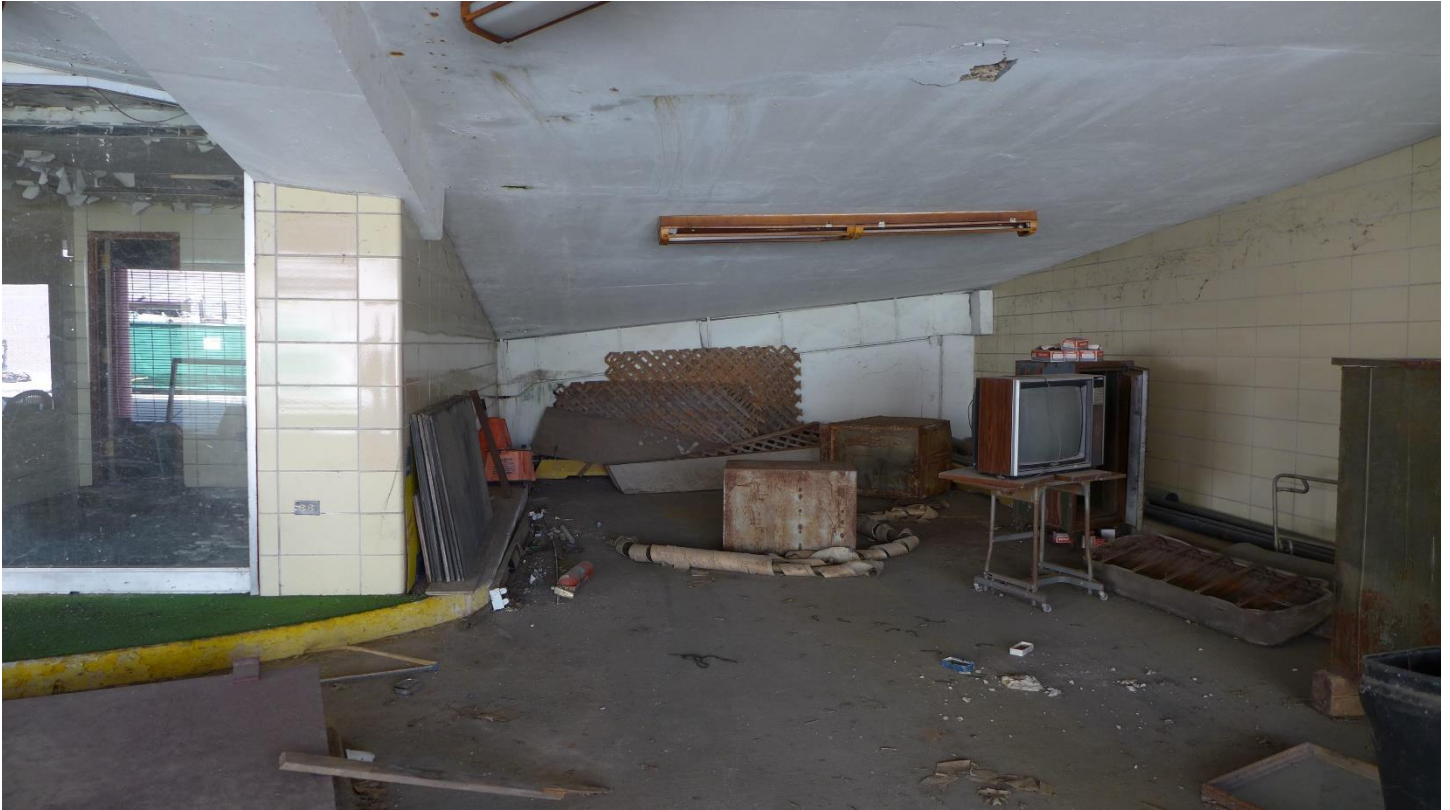
Photo 23 Garage entrance/exit bay, camera facing west February 2021
