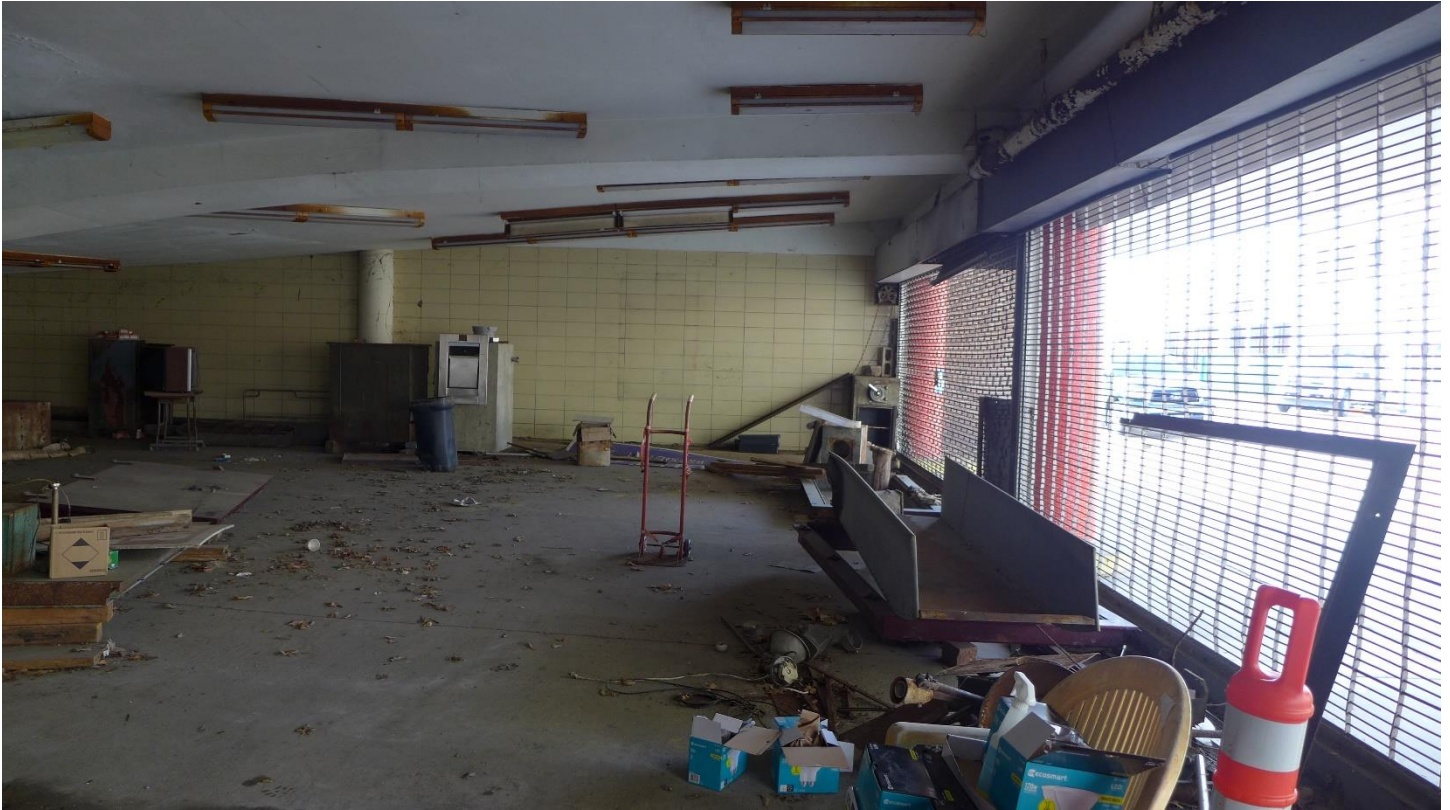
Photo 21 Garage entrance/exit bay, camera facing west January 2021
