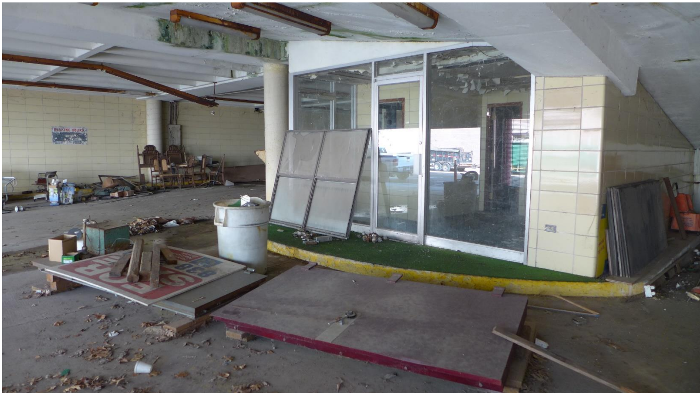
Photo 19 Garage entrance/exit bay, camera facing southeast February 2021
