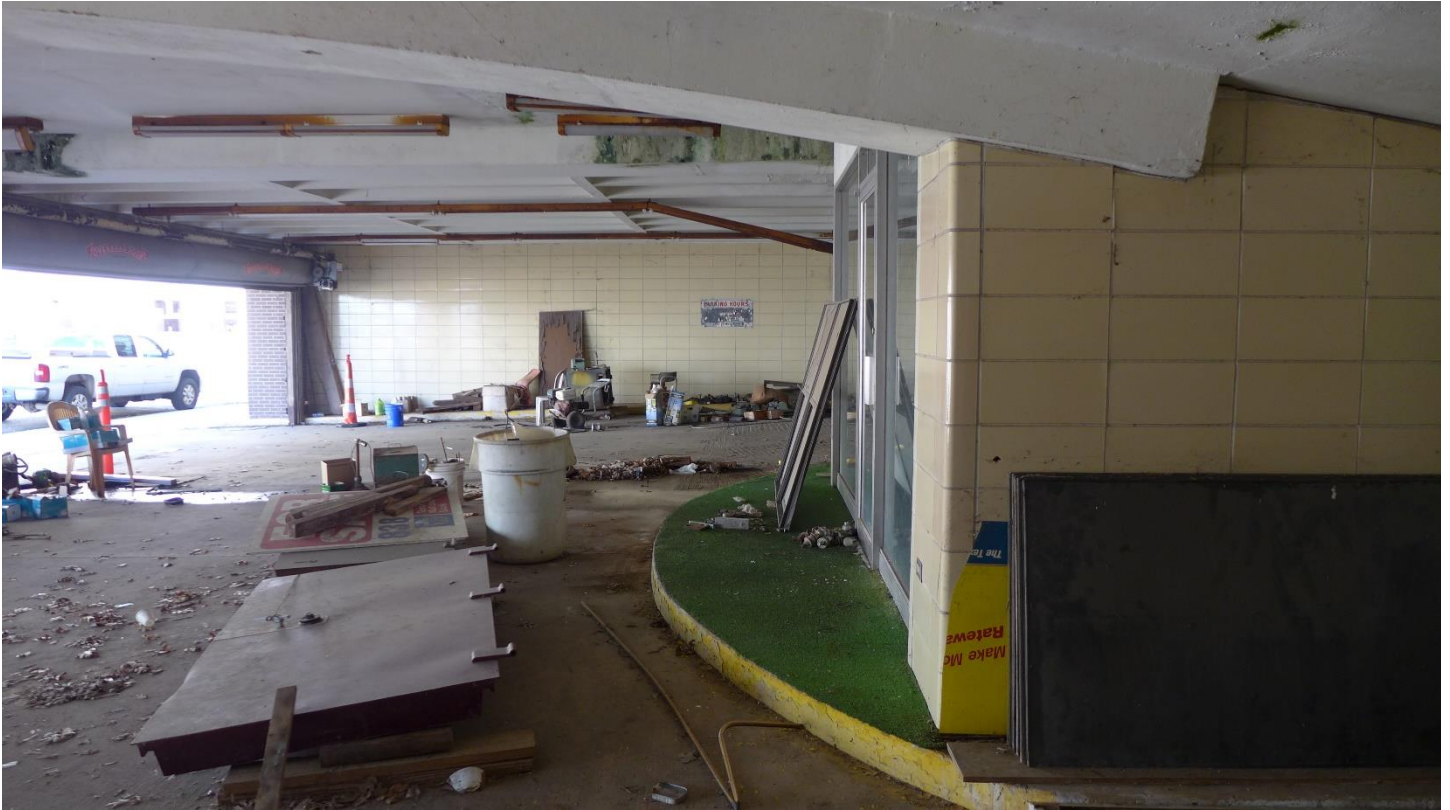
Photo 20 Garage entrance/exit bay, camera facing east February 2021
