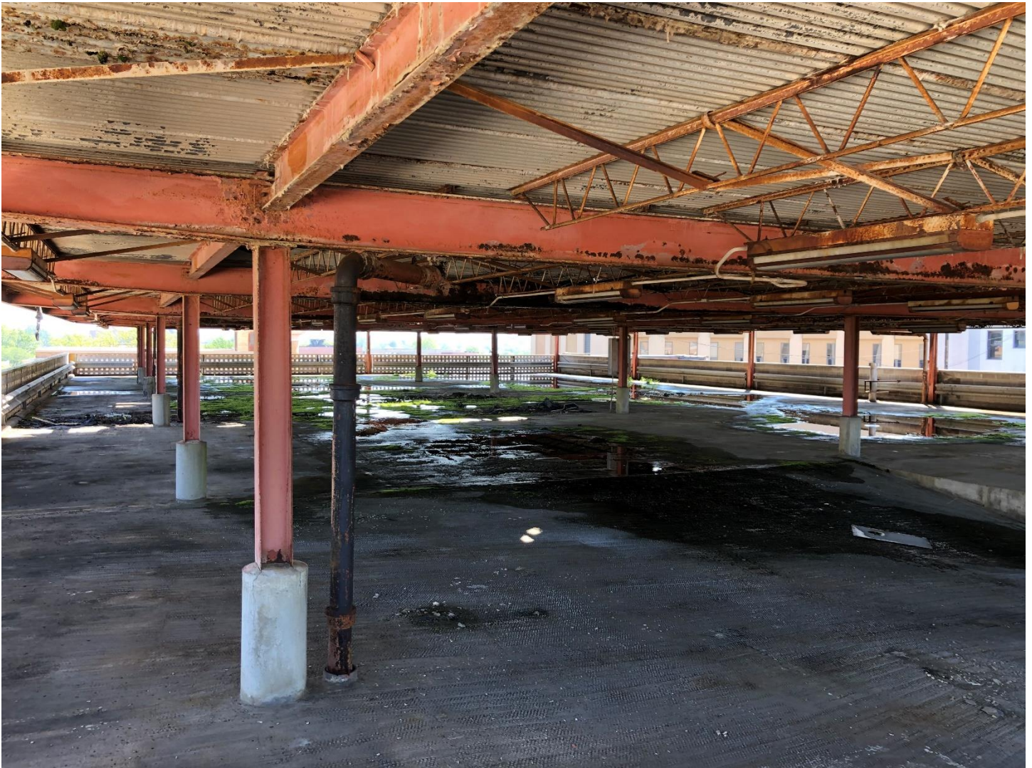
Photo 17 Garage top level, camera facing east February 2021
