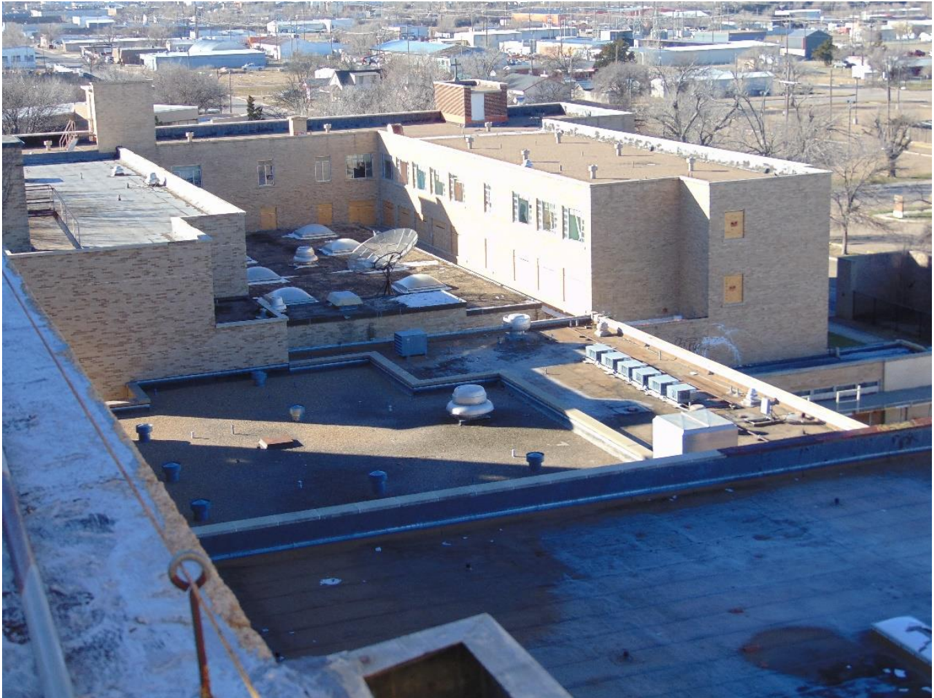
Rooftop view of the School of Nursing and kitchen and dining expansion, view south
