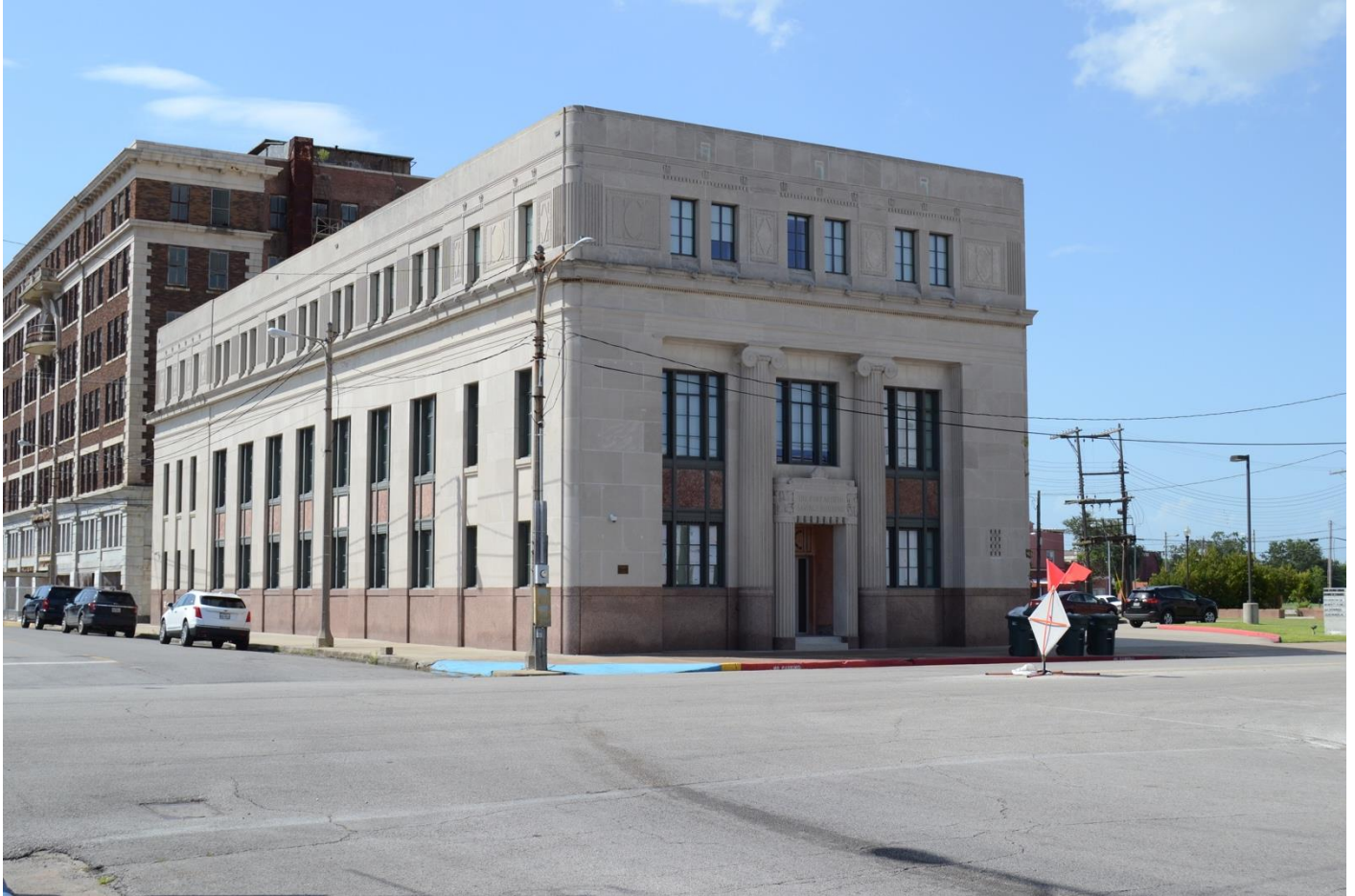
Photo 31. Oblique view of the First National Bank of Port Arthur Building (Resource 9), facing north-northwest.
