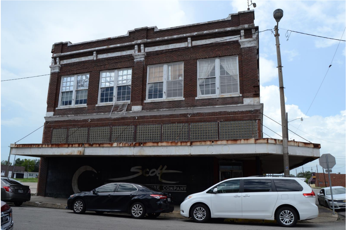
Photo 27. Façade of the John R. Adams & Co. Building (Resource 5), facing northwest.
