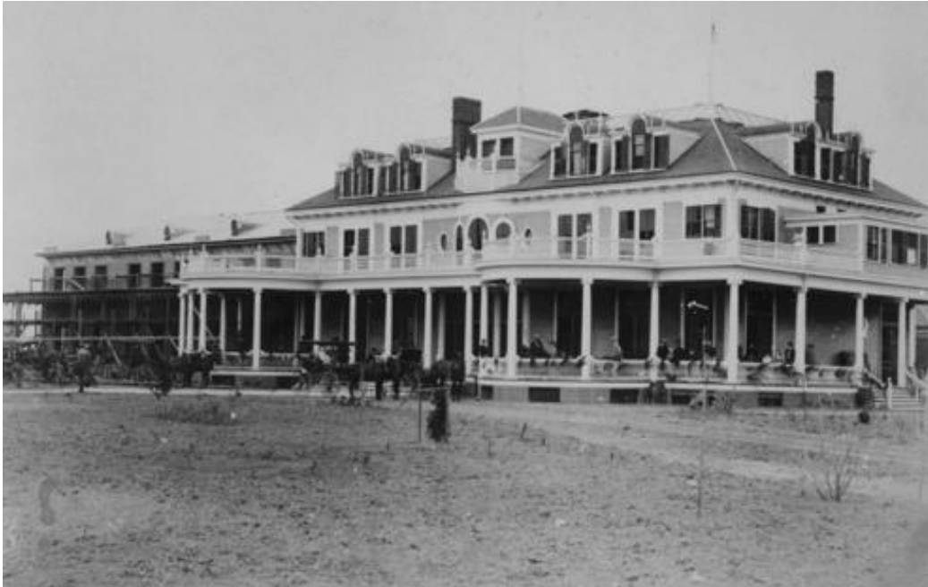
Figure 3. View of the Hotel Sabine, constructed by the Kansas City, Pittsburg & Gulf Railroad in 1896 to attract businessmen and settlers to Port Arthur. The spacious three-story hotel featured 70 rooms and surrounding tropical gardens. The hotel occupied the lakeshore where the present-day Jefferson County Office now stands. Source: The Portal to Texas History.
