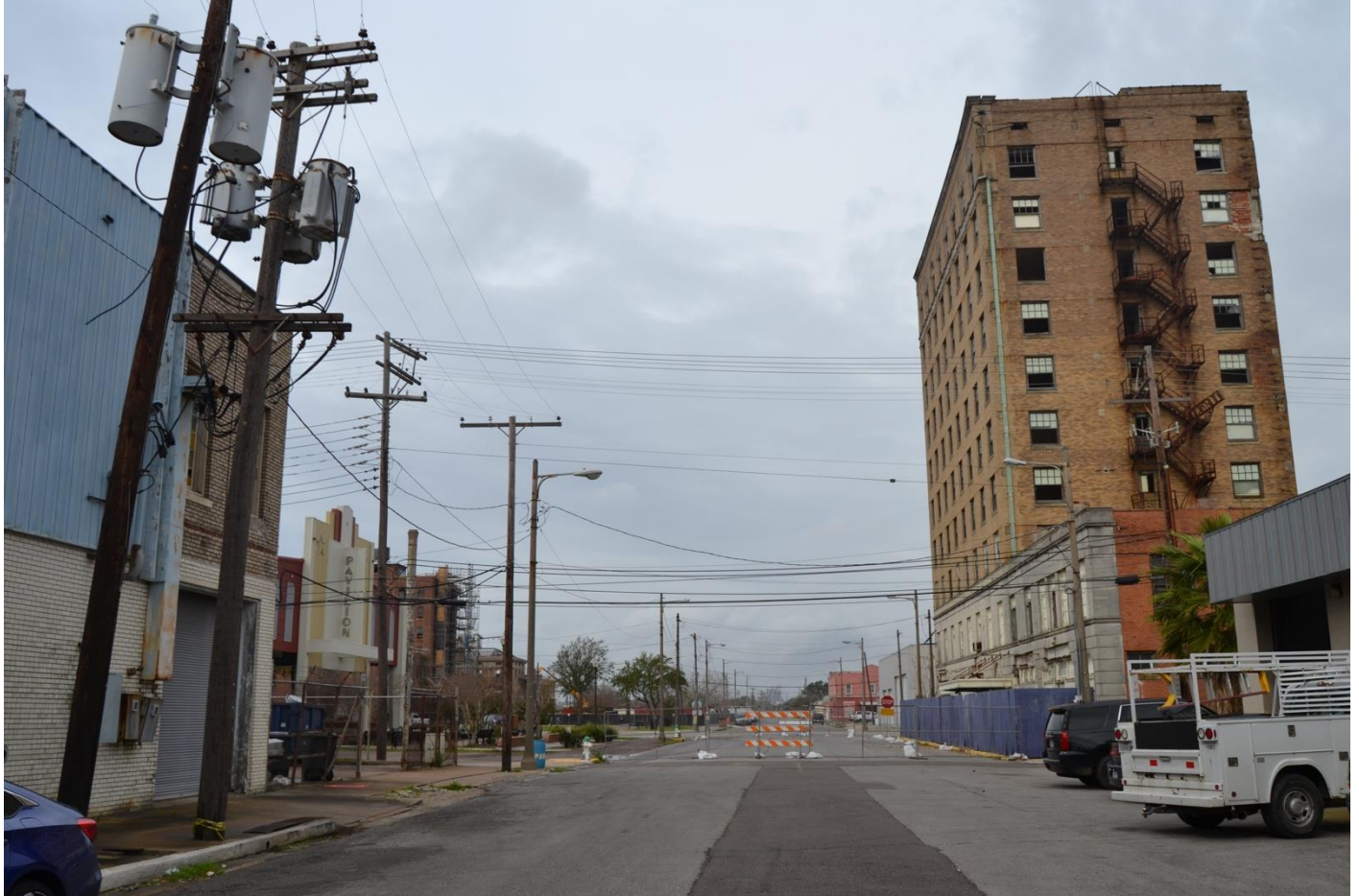
Photo 17. Contextual view of the 300 block of Waco Avenue, facing northwest.
