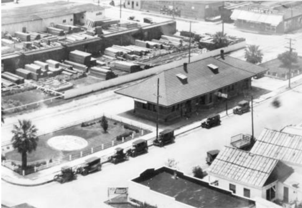
Figure 8. Photograph showing an early bird's-eye view of the Texas & New Orleans Railroad depot (Resource 1) on Austin Avenue. Date unknown. Source: The Portal to Texas History.
