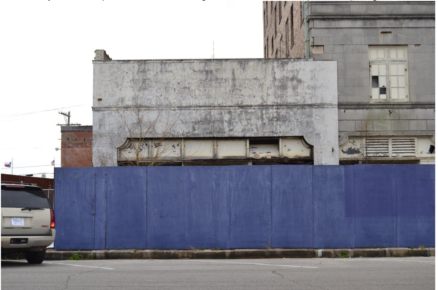
Photo 34. Façade of the one-part commercial block building located at 608 Procter Street (Resource 12), facing southeast.
