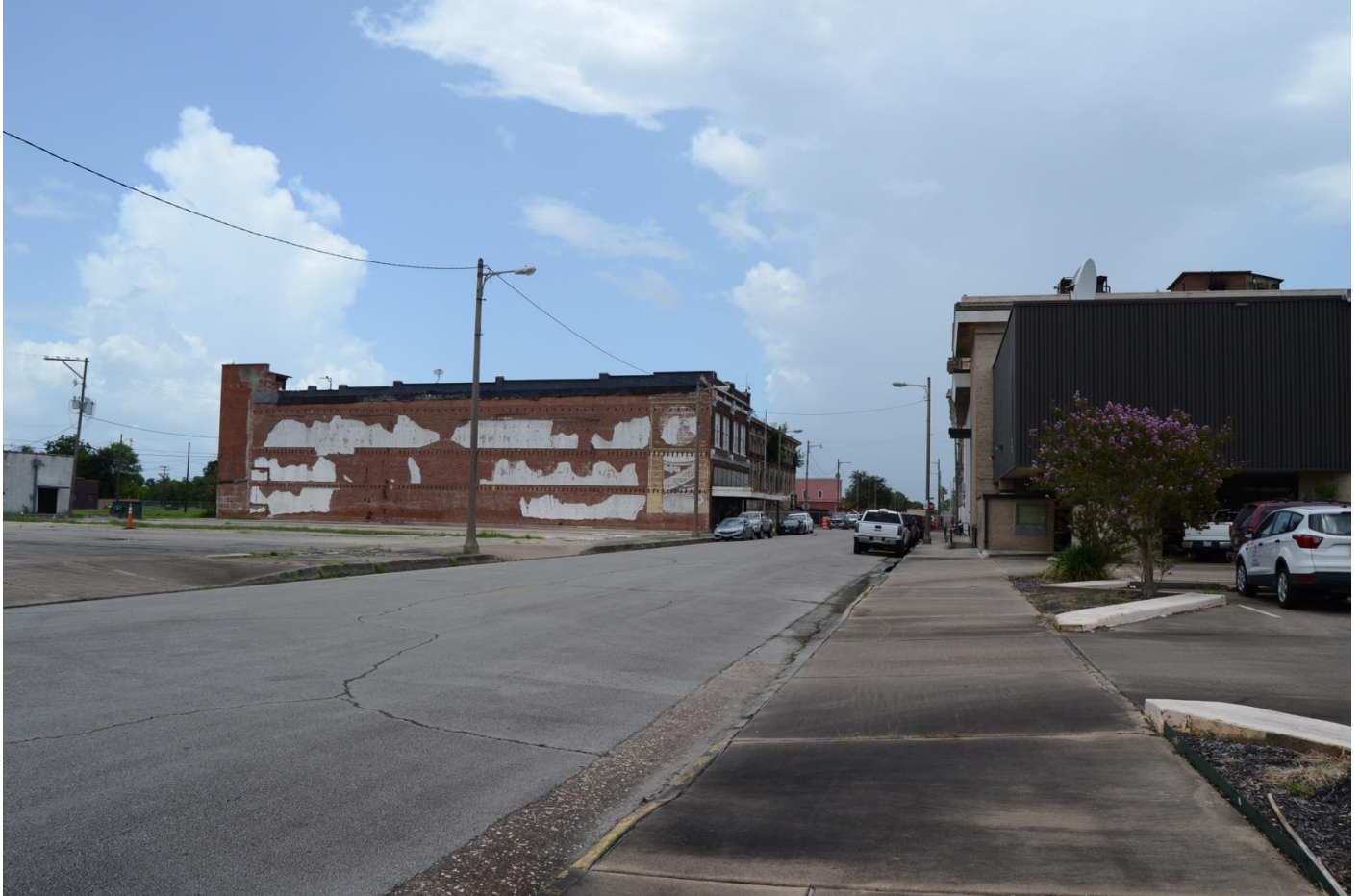
Photo 9. Contextual view of 400 block of Fifth Street, facing northeast.
