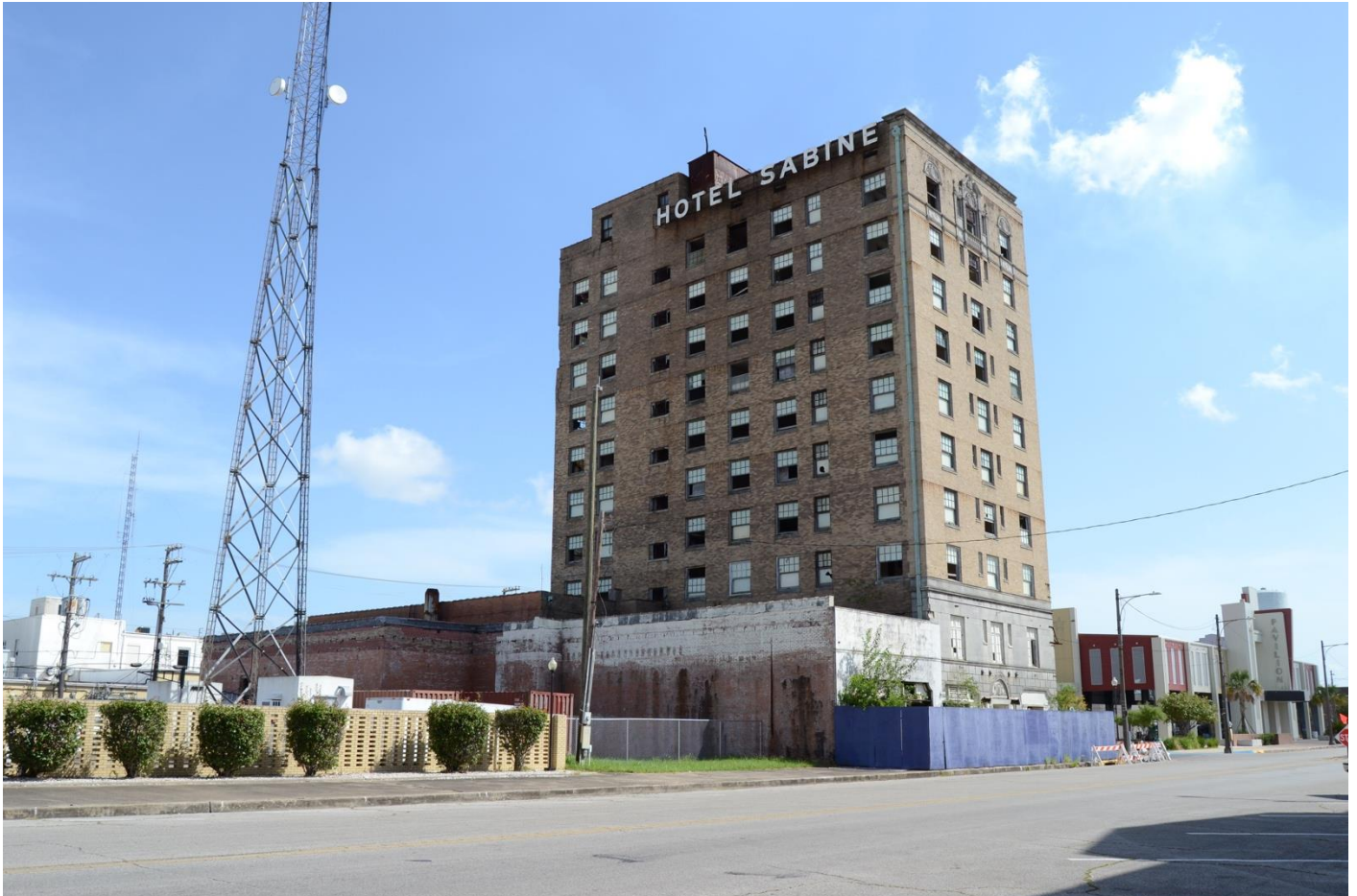
Photo 33. Oblique view of Vaughn Hotel and the one-part commercial block building adjoining it to the northeast (Resources 11-12), facing south.
