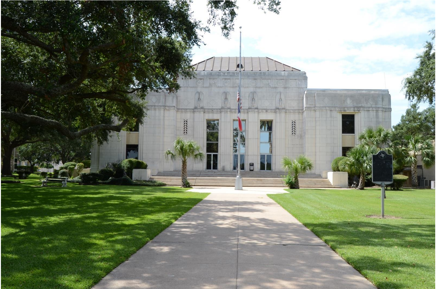
Photo 38. Façade of the South Jefferson County Office Building (Resource 16), facing northwest.
