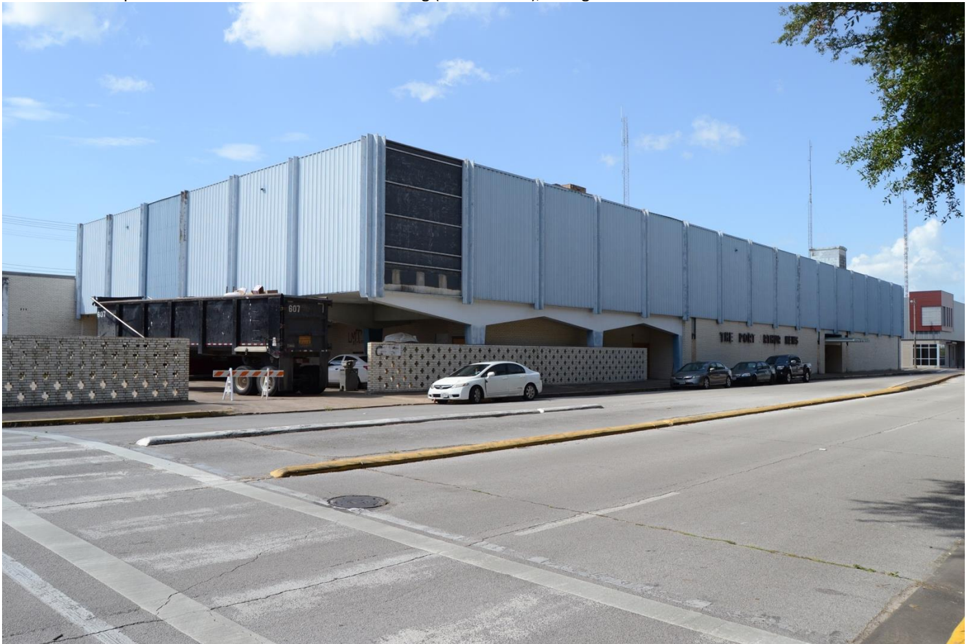
Photo 36. Oblique view of the Port Arthur News building (Resource 14), facing north-northeast.
