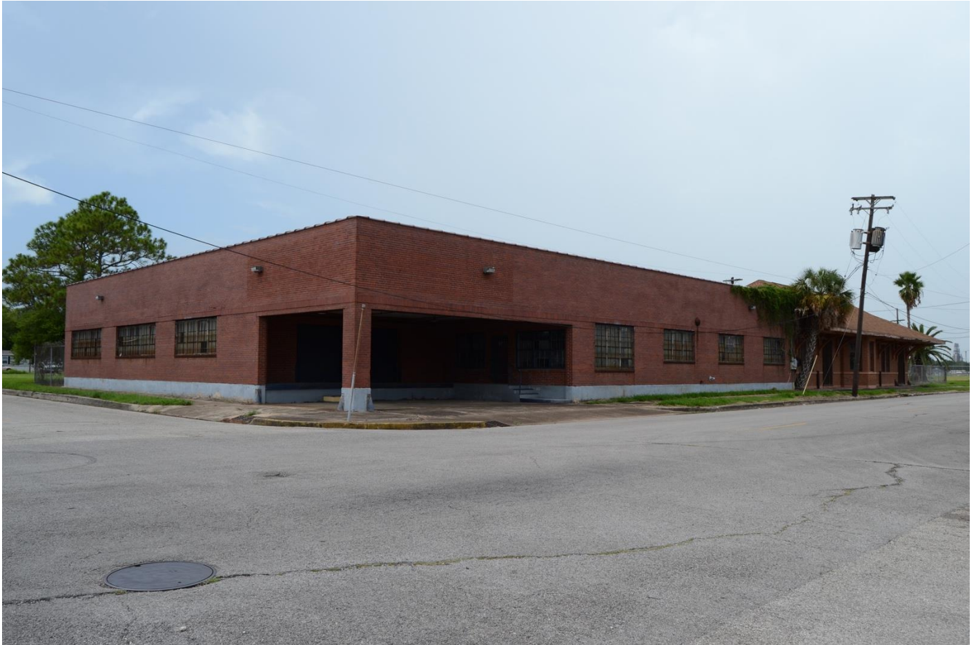
Photo 24. Oblique view of the Railway Express Agency, Inc. Office and Warehouse building (Resource 2), facing west.
