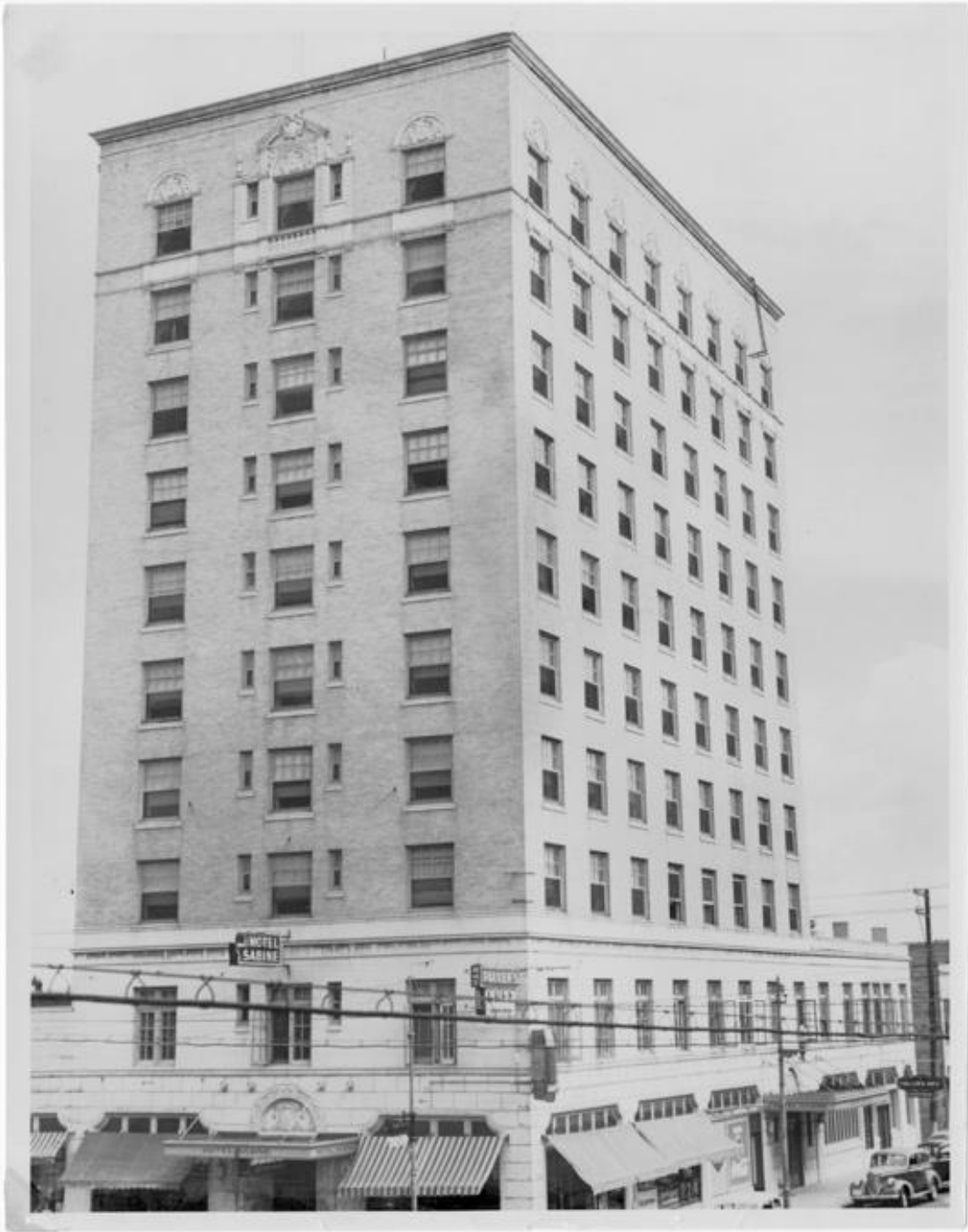
Figure 14. Early view of Vaughn Hotel (Resource 11), a 10-story Renaissance Revival-style hotel built by local doctor Ed W. Vaughn in 1929. It features stone cladding at the first and second floors, rusticated treatments, curved archways, and Classical Revival sculptural motifs. Situated at 600 Procter Street, the building is currently the tallest building in Port Arthur. Date unknown. Source: The Portal to Texas History.
