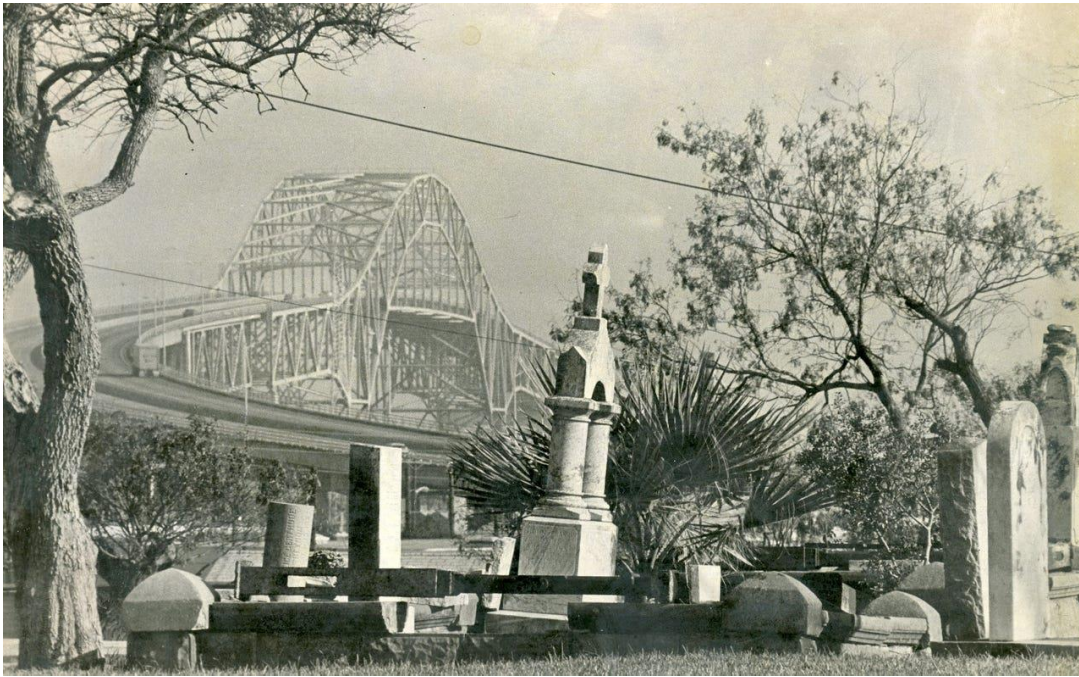
Figure 6. The Harbor Bridge and IH-37 in the background of Old Bayview Cemetery, 1975. Source: Corpus Christi Caller-Times, photo by Murray Judson.
