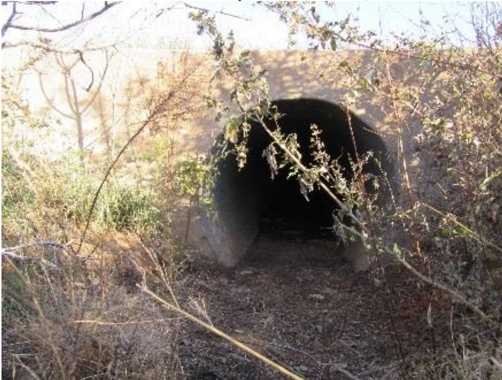
Photo 21: Feature No. H-02 Concrete Pipe Culvert (south side)
