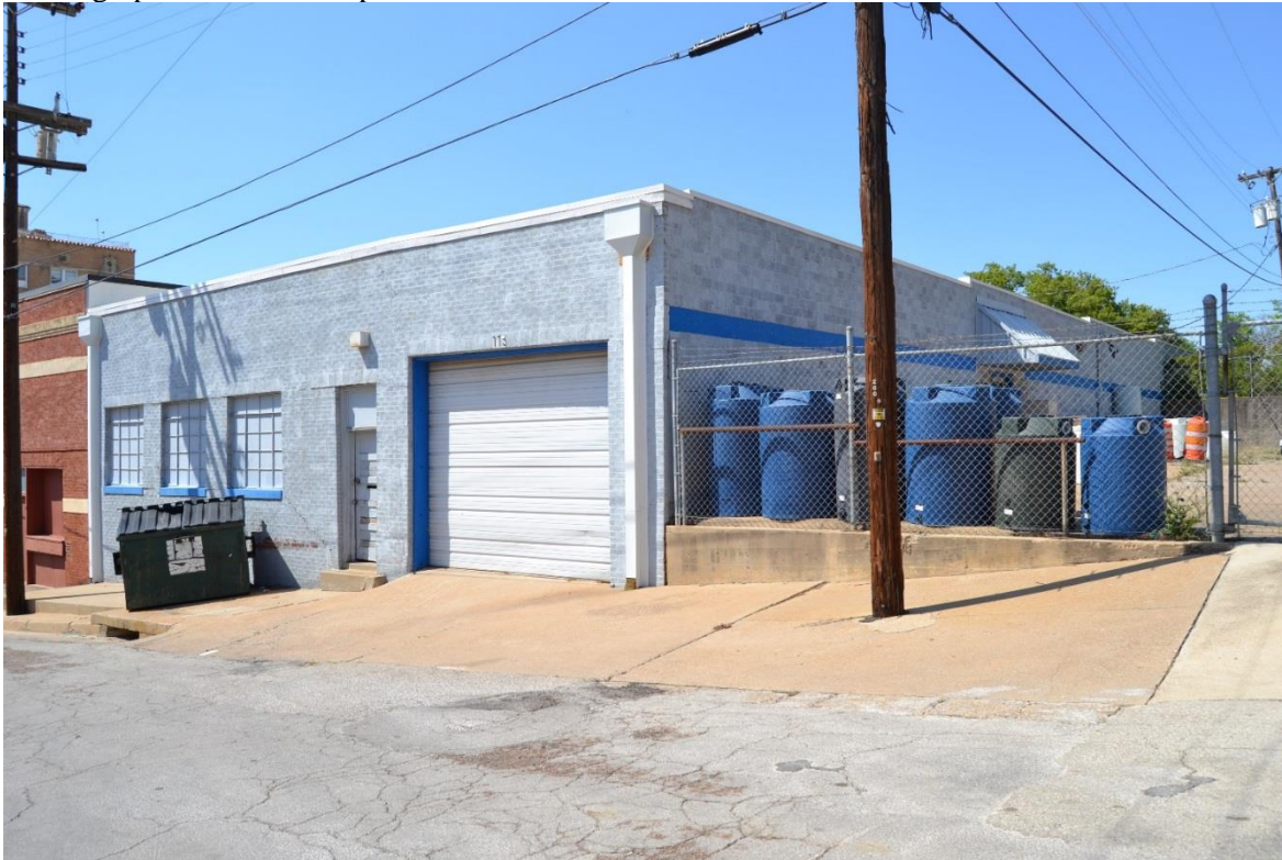
Photo 51. Oblique view of an auto repair shop at 113 NE 3rd Street (Map ID 12429). Camera facing northwest.
