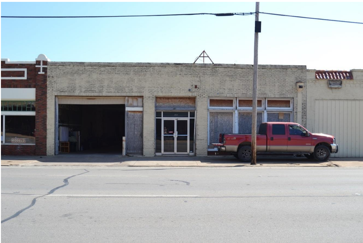
Photo 44. Façade of one-part commercial block building at 205-207 W Hubbard Street (Map ID 12447). Camera facing south.
