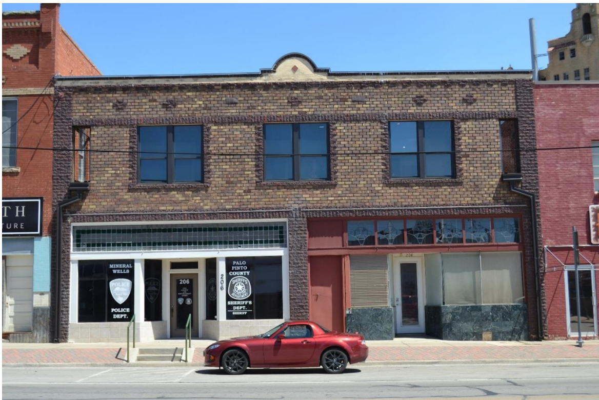
Photo 36. Two-part commercial block building at 204-206 N Oak Avenue (Map ID 12085). Facing east.
