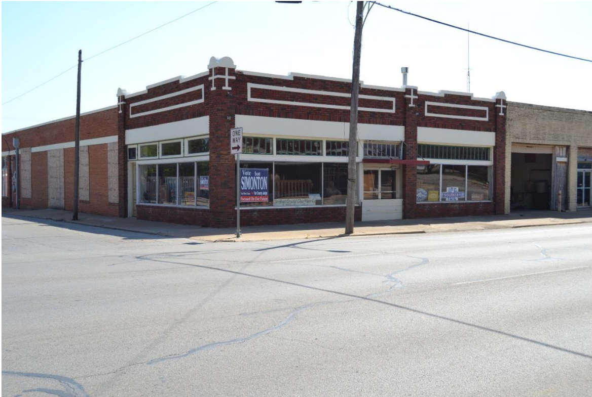
Photo 41. Oblique view of an auto sales building at 201 W Hubbard Street (Map ID 12450). Facing southwest.
