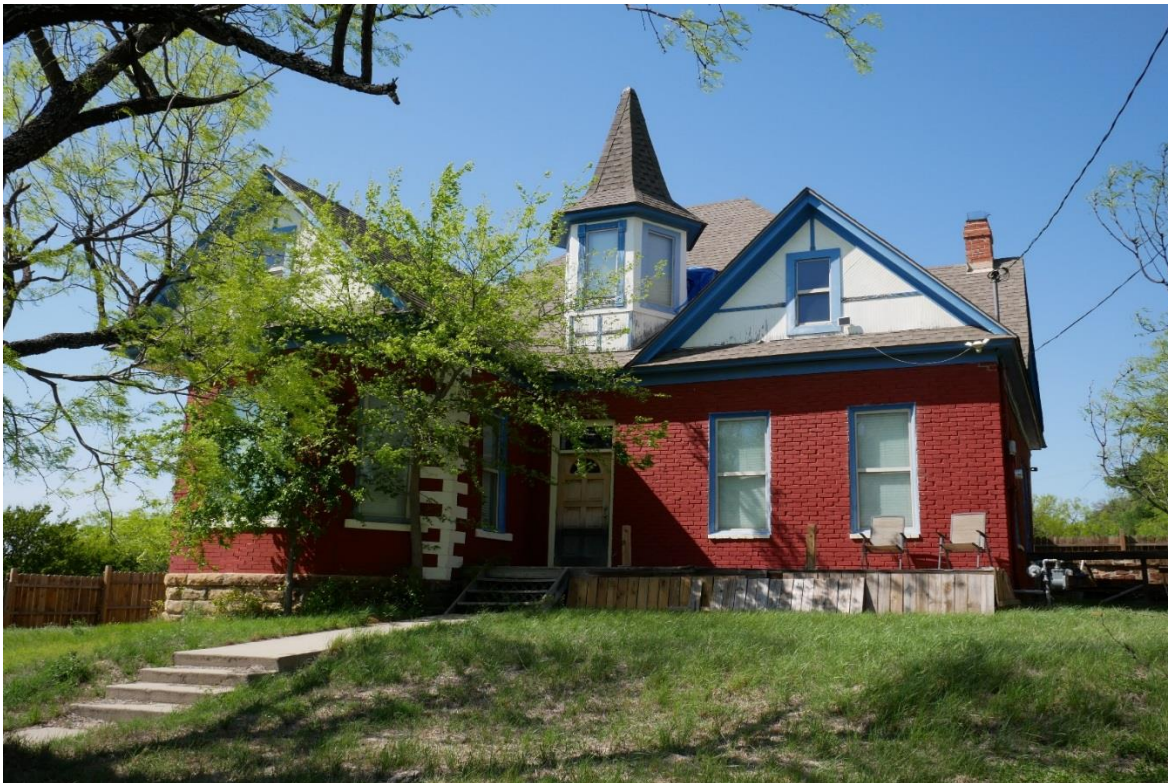
Photo 26. Oblique view of the Thompson House (Map ID 13005). Camera facing northwest.
