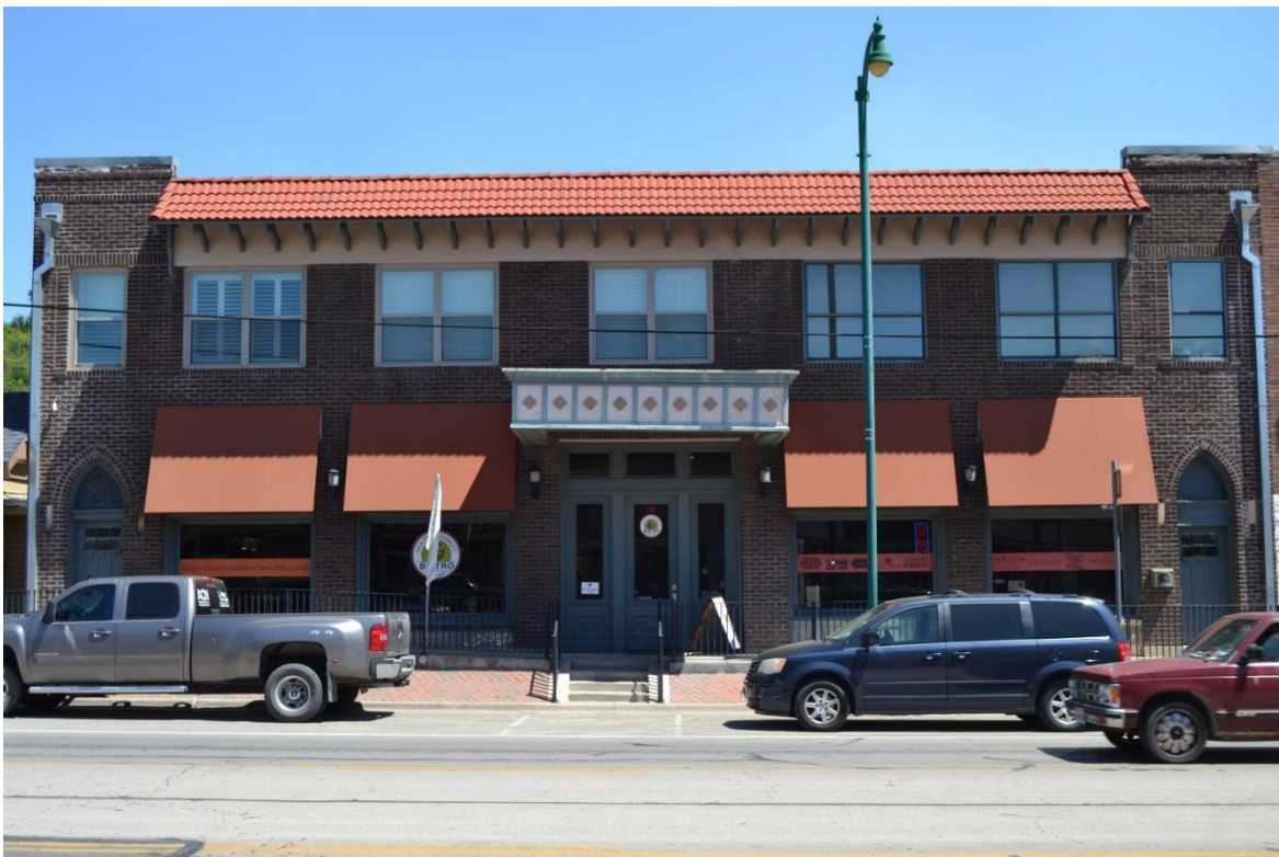
Photo 38. Façade of the Wylie Building (Map ID 12072). Camera facing east.
