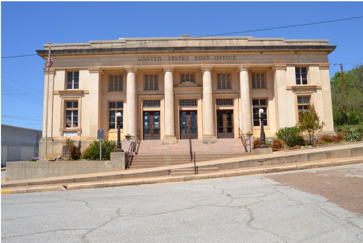
Photo 10. Façade of the Post Office (Map ID 11865). Camera facing north.
