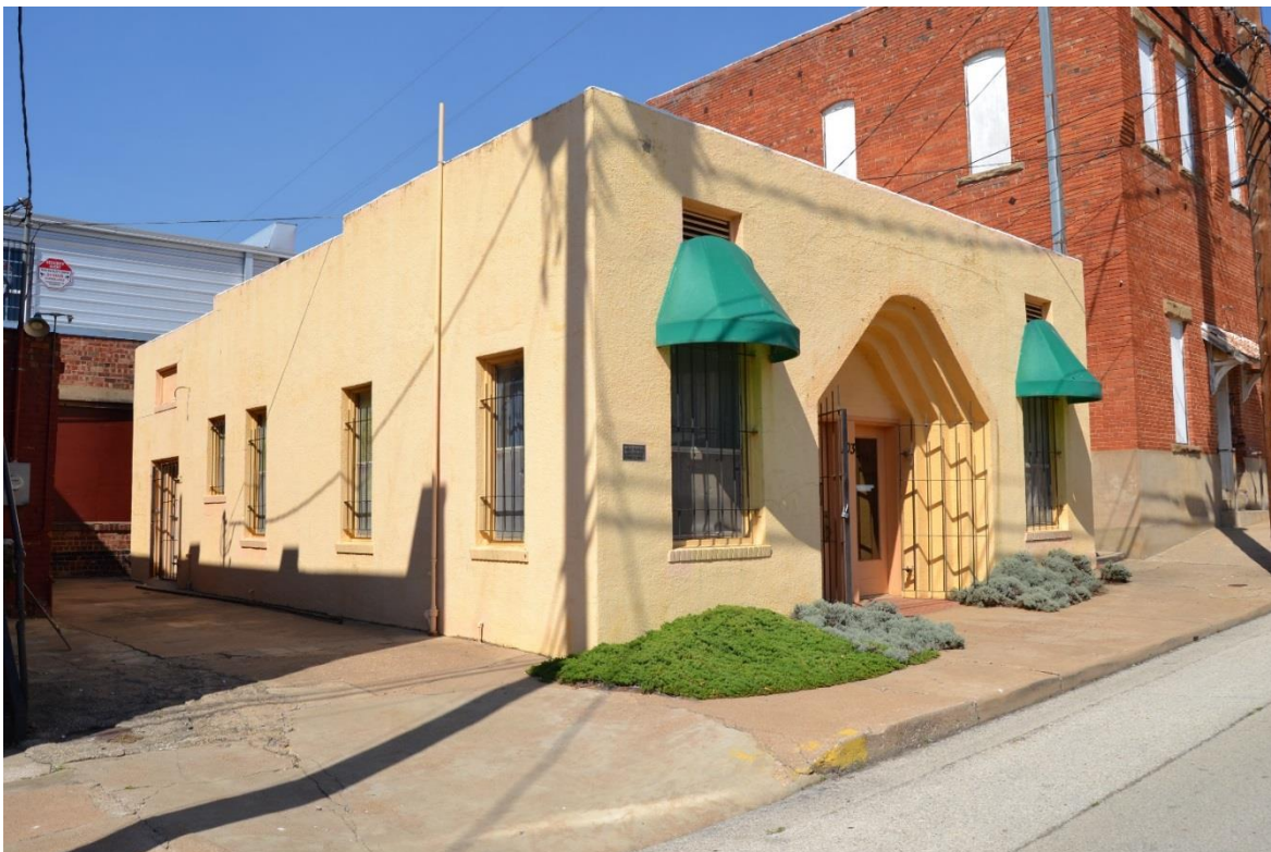
Photo 50. Oblique view of the City Water Office building (Map ID 12471). Camera facing northeast.
