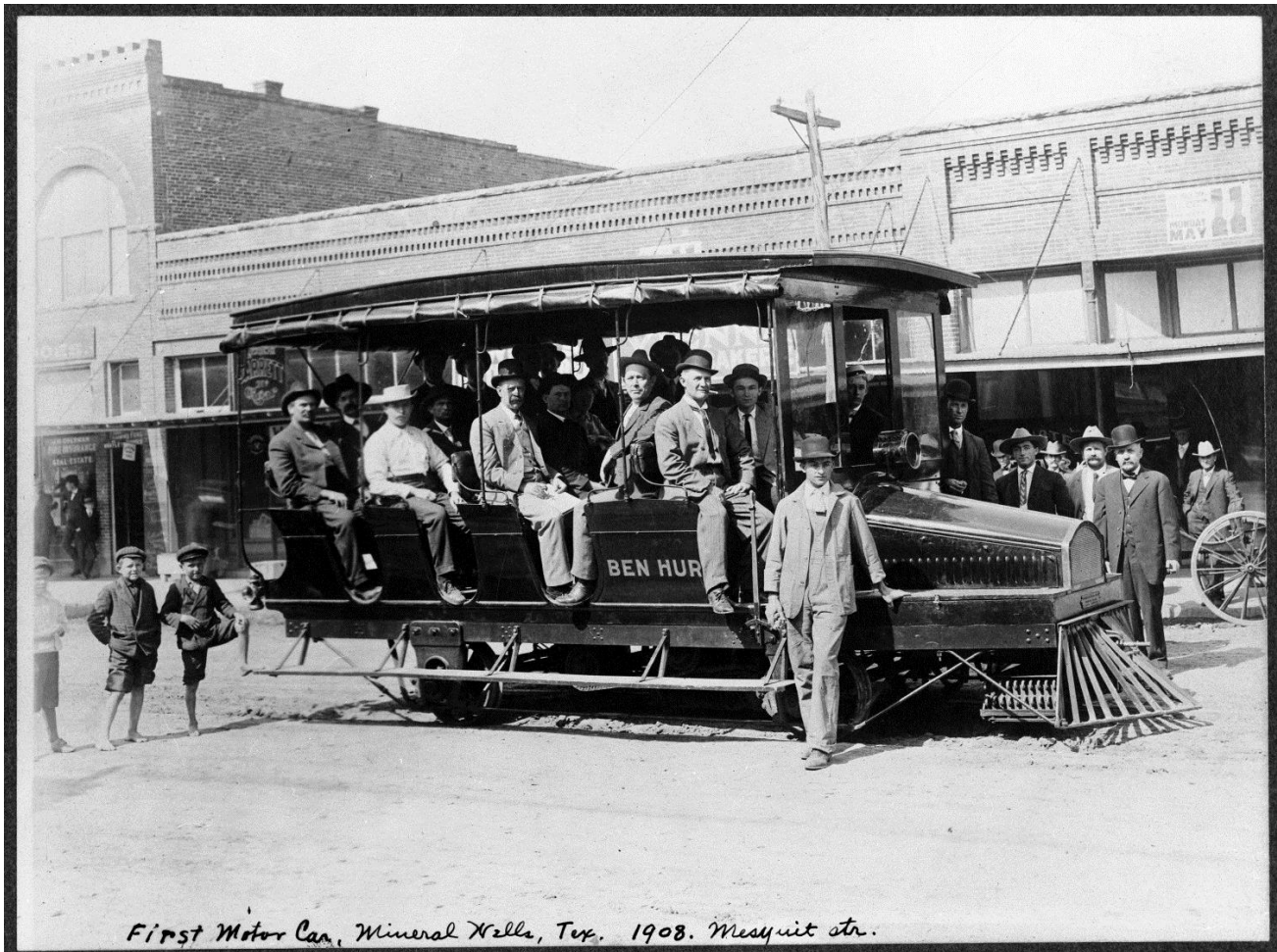
Figure 32. Photograph taken between 1908 and 1909 of one of the gas-powered motor cars that ran along E 1st Avenue in downtown to Lake Pinto on the Mineral Wells Lakewood Motor Car Scenic Railway. This particular motor car was named Ben Hur. Source: The Portal to Texas History, A. F. Weaver Collection, Boyce Ditto Public Library, Mineral Wells, Texas.
