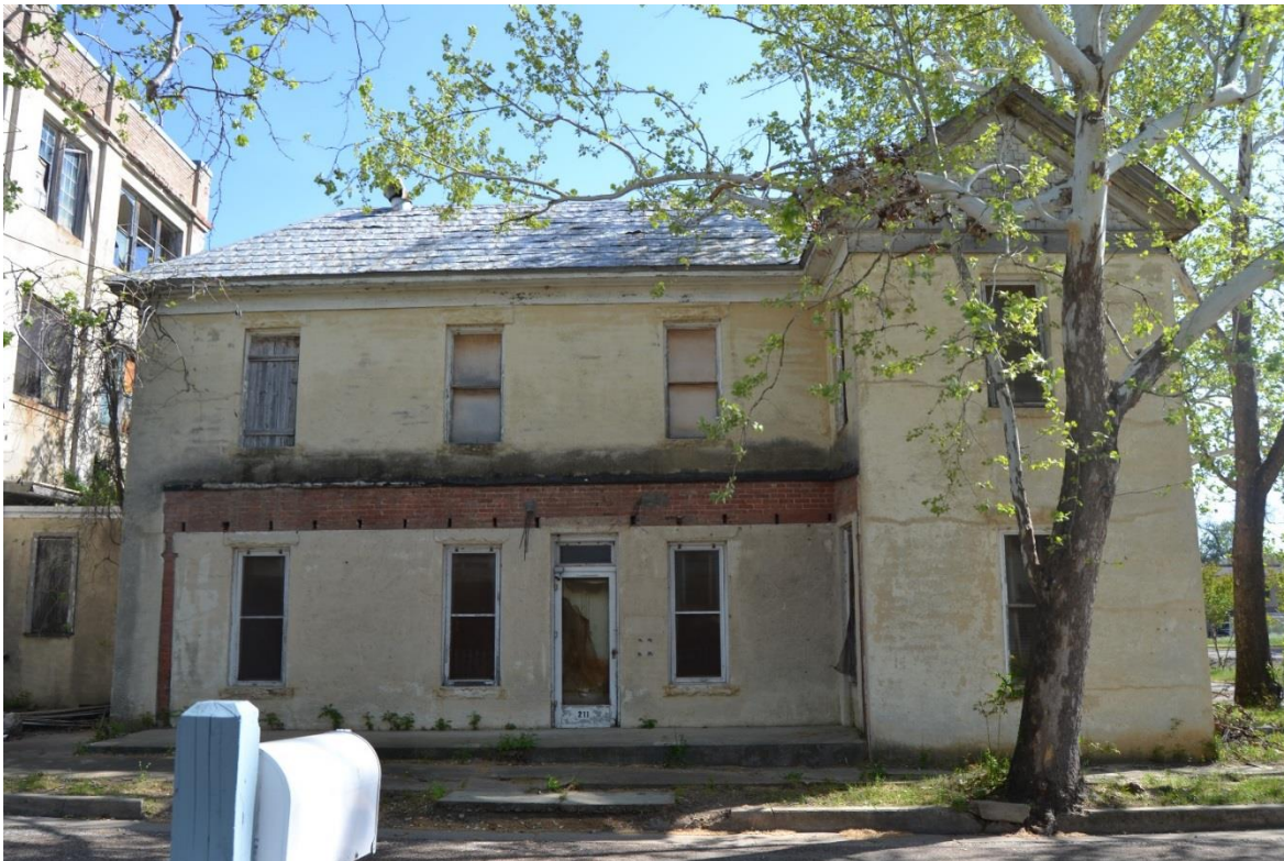
Photo 24. Façade of the Wayside Inn (Map ID 15358). Camera facing south.
