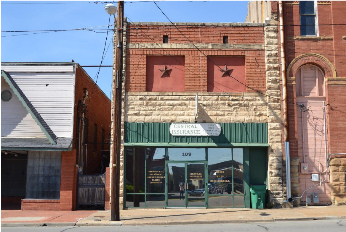
Photo 57. 109 E. Hubbard Street (Map ID 12465), an example of a historic-age noncontributing building.
