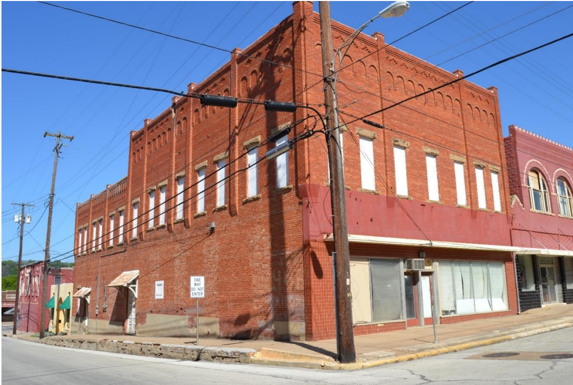
Photo 25. Oblique view of commercial block building at 201 NE 1st Avenue (Map ID 11777). Camera facing northwest.
