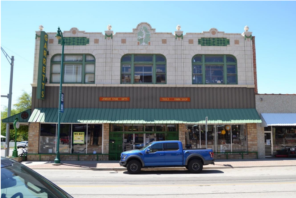
Photo 39. Façade of the Montgomery Ward building (Map ID 11839). Camera facing west.
