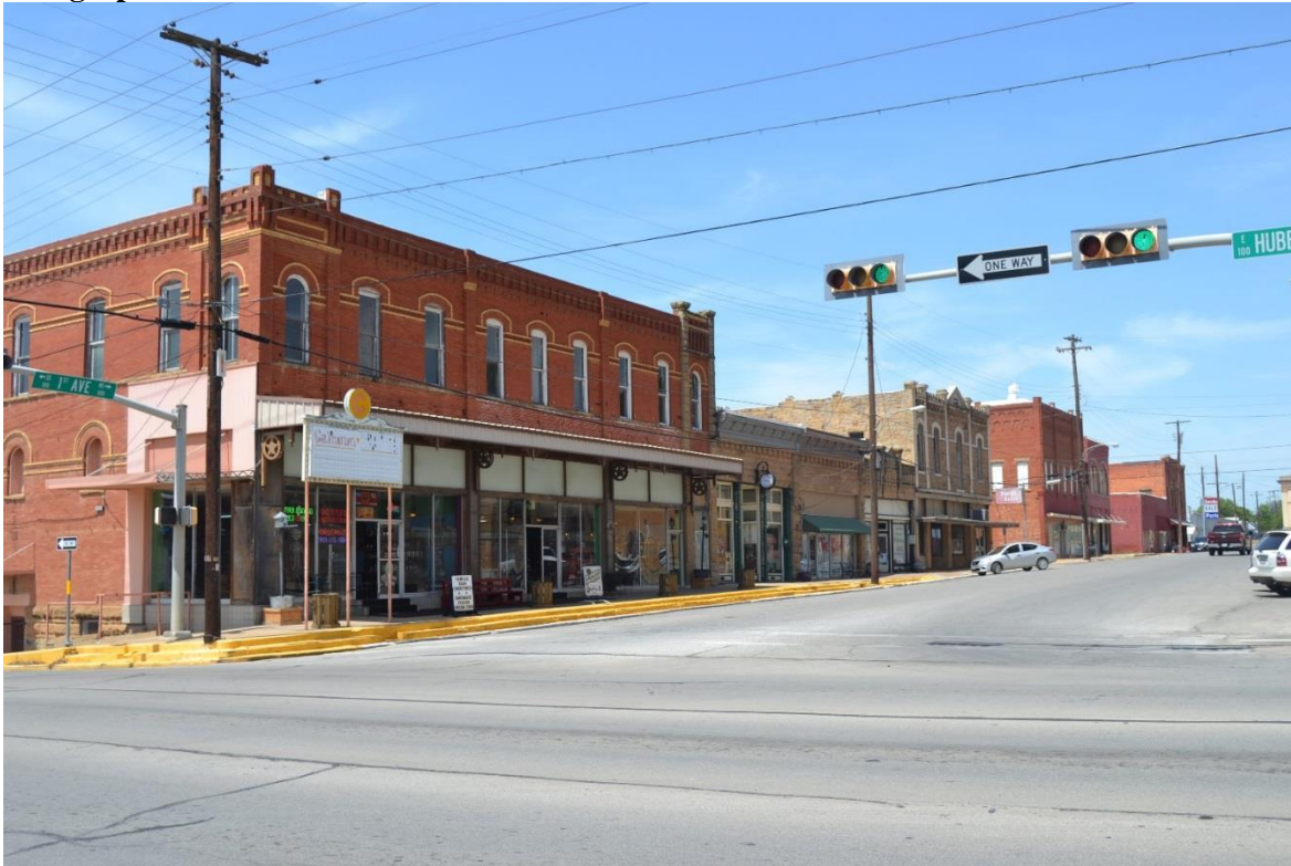
Photo 1. Contextual view of 100 block of NE 1st Avenue taken from Hubbard Street. Camera facing northwest.
