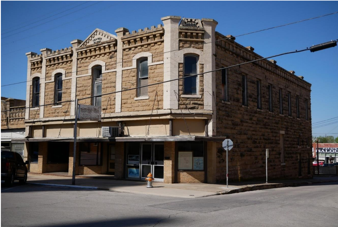
Photo 31. Oblique view of the Yeager Building (Map ID 11988). Camera facing southwest.
