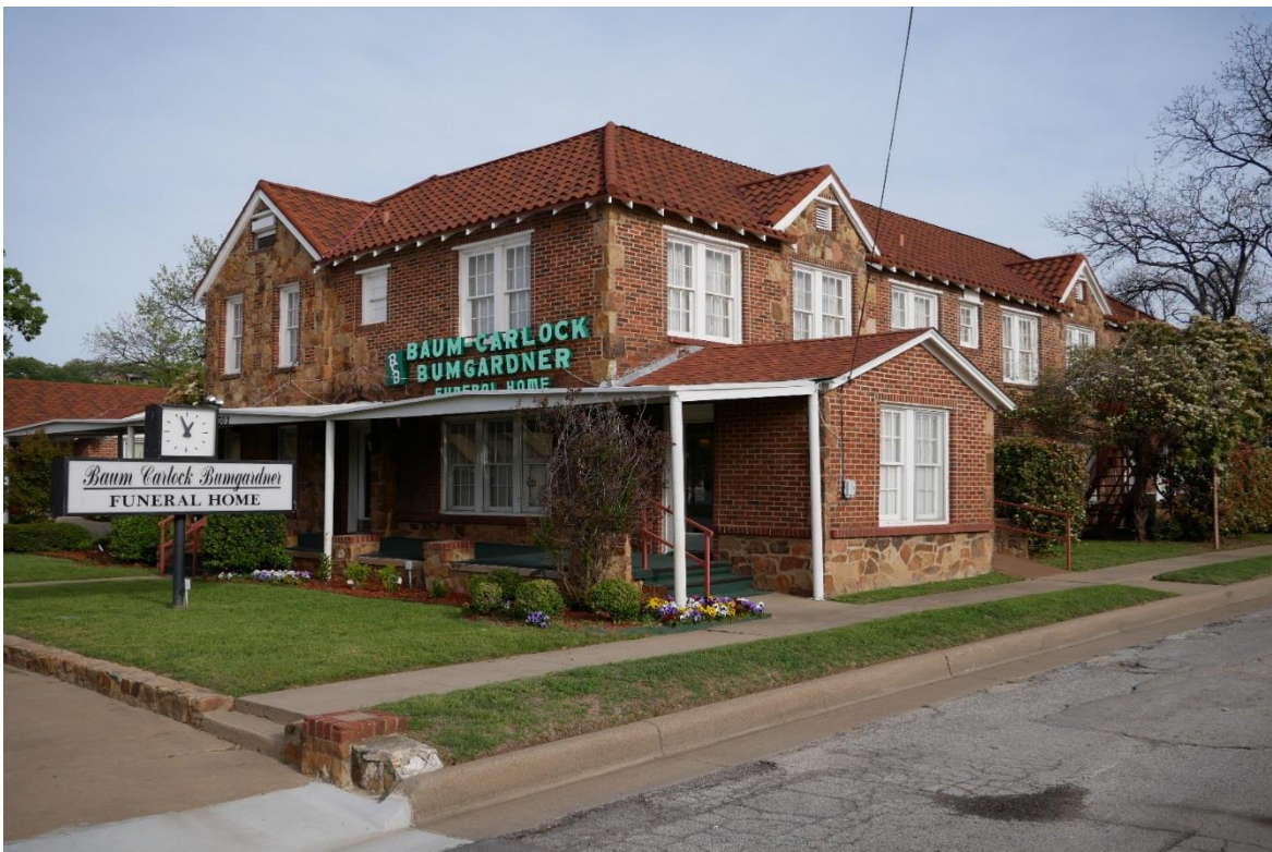
Photo 40. Oblique view of the Baum-Carlock Funeral Home (Map ID 12583). Camera facing northwest.
