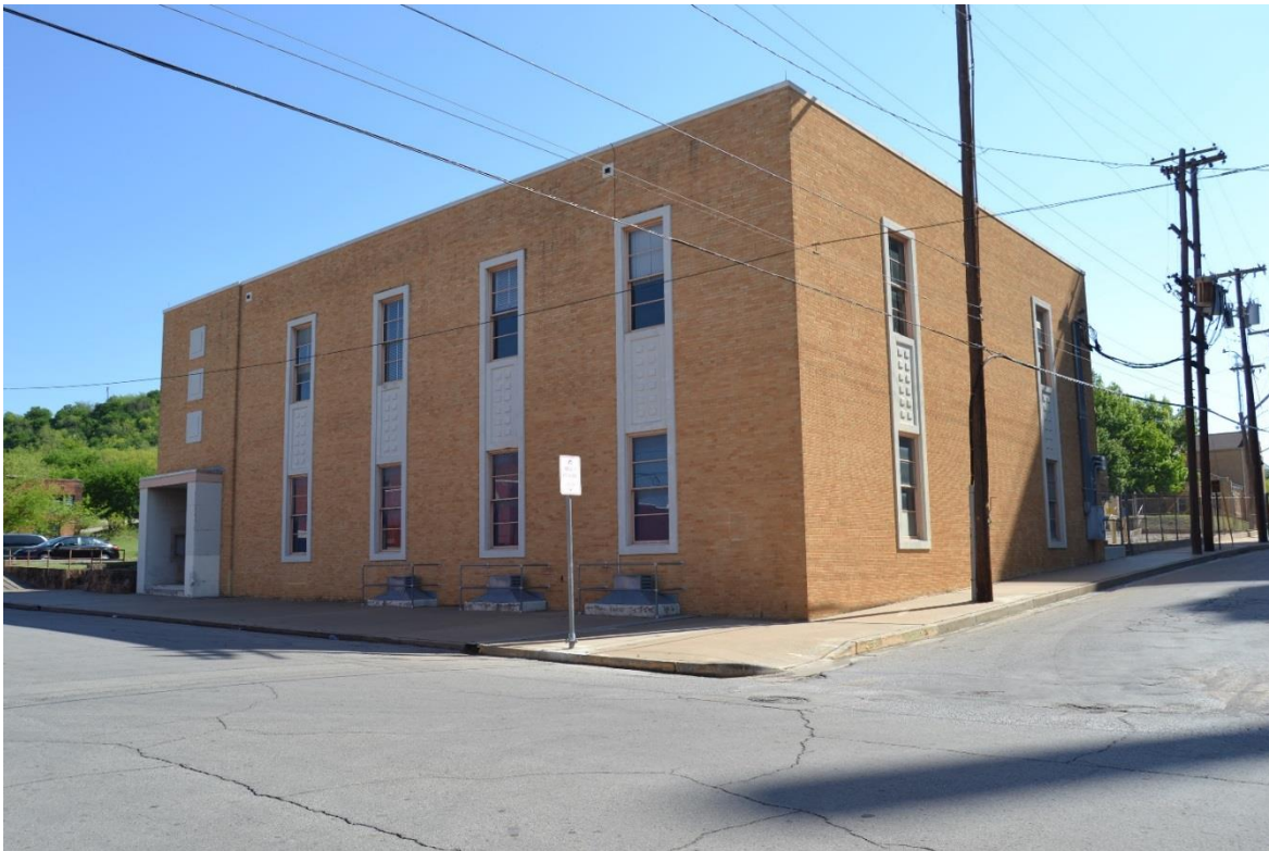
Photo 48. Oblique view of Southwester Telephone building (Map ID 11783). Camera facing northeast.
