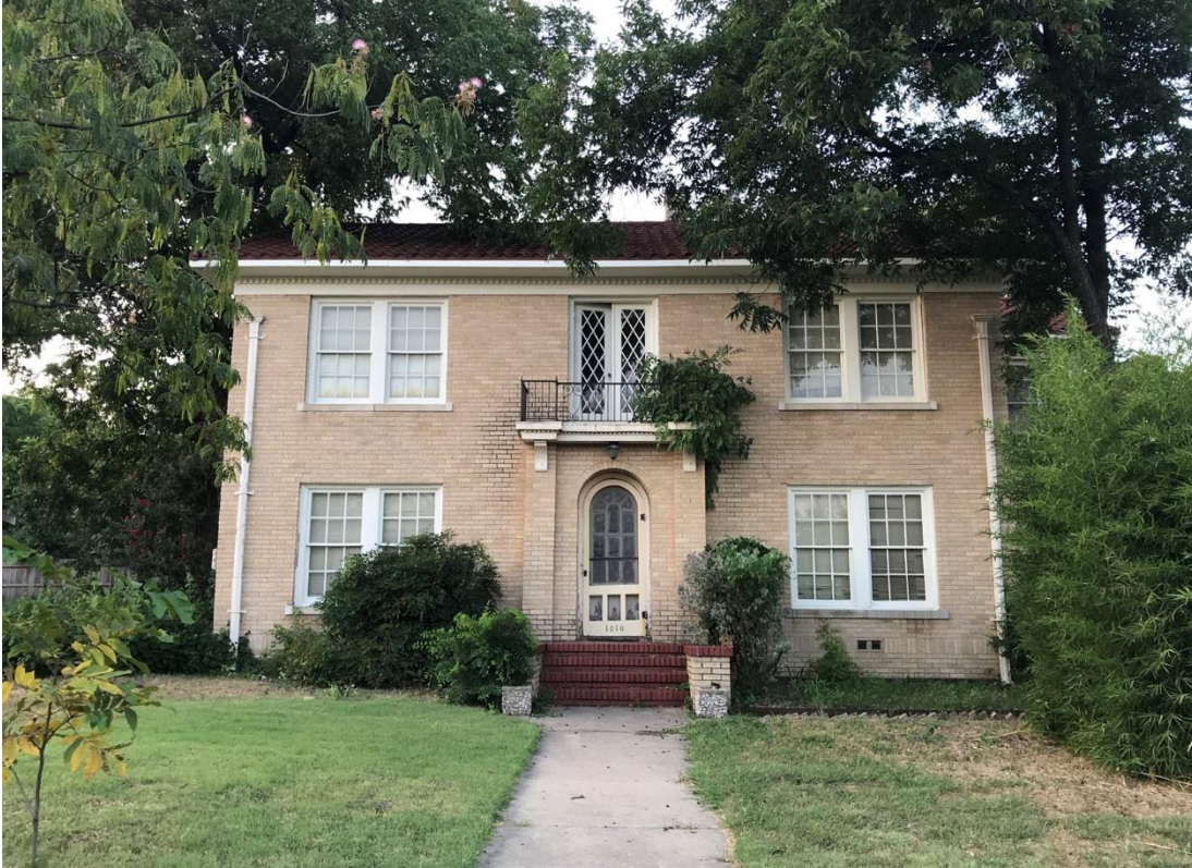
Photo 14: 1010 West Hickory (Property 206)
