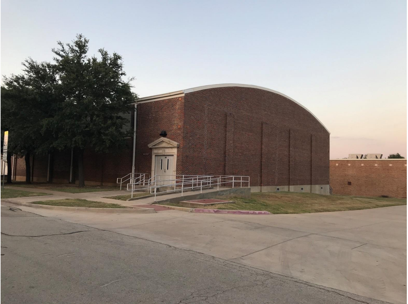
Photo 21: High School Gymnasium (Property 44b)
