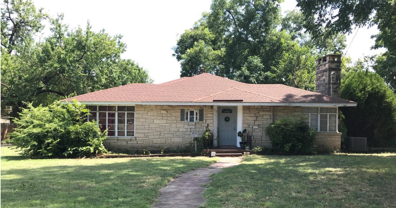
Photo 16: 815 West Hickory (Property 186)
