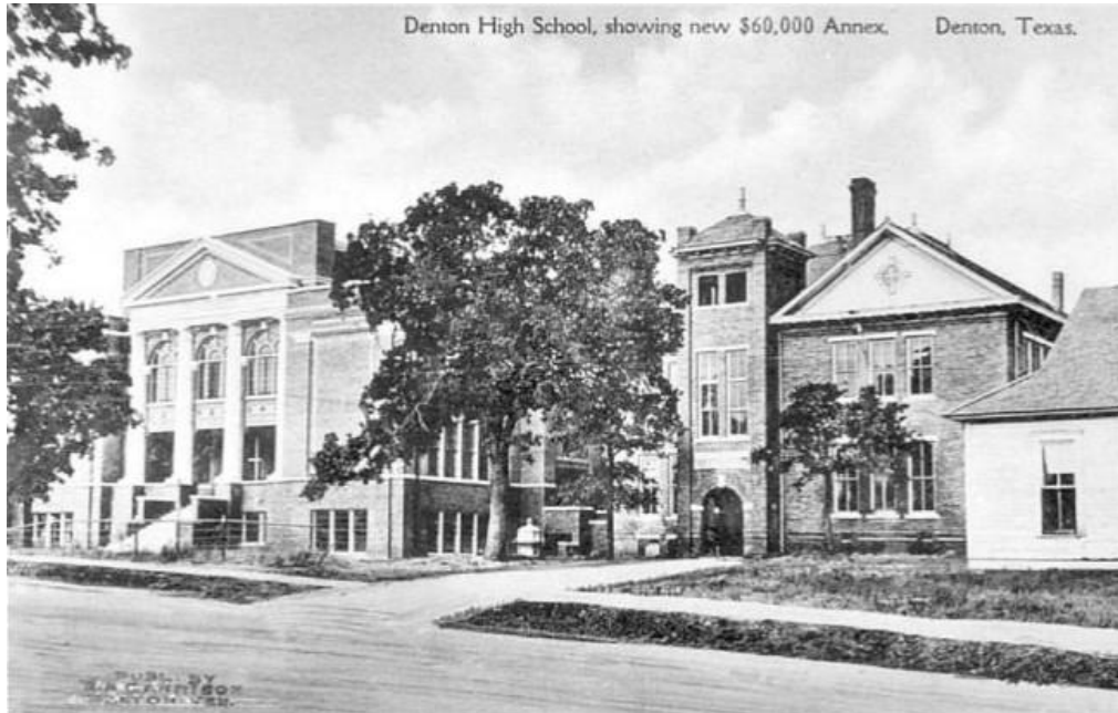
Figure 6: The Senior High School fronting Congress Street with the former High School at Denton and Gregg Streets becoming the Junior High School in 1924.
