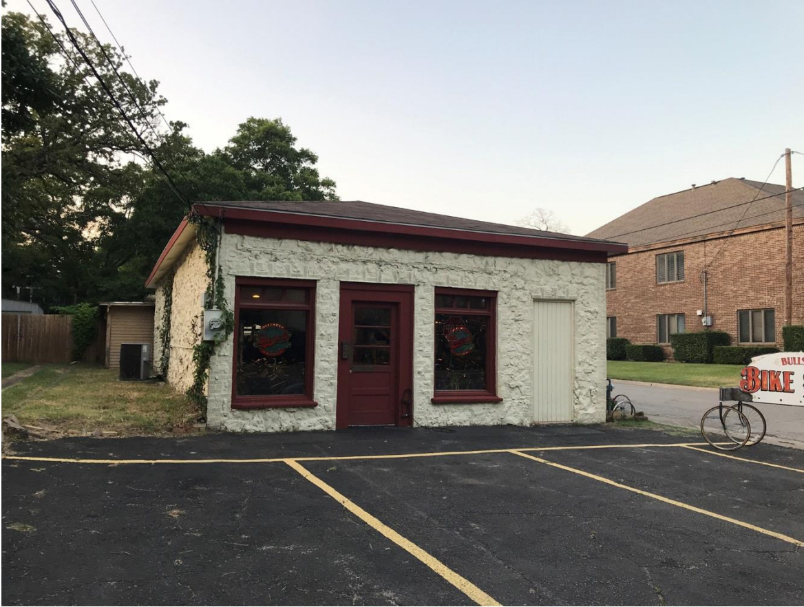
Photo 17: 700 West Hickory (Property 172)
