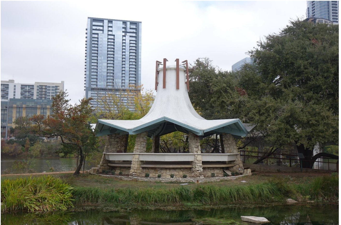
Photo 2 South elevation Camera facing north
