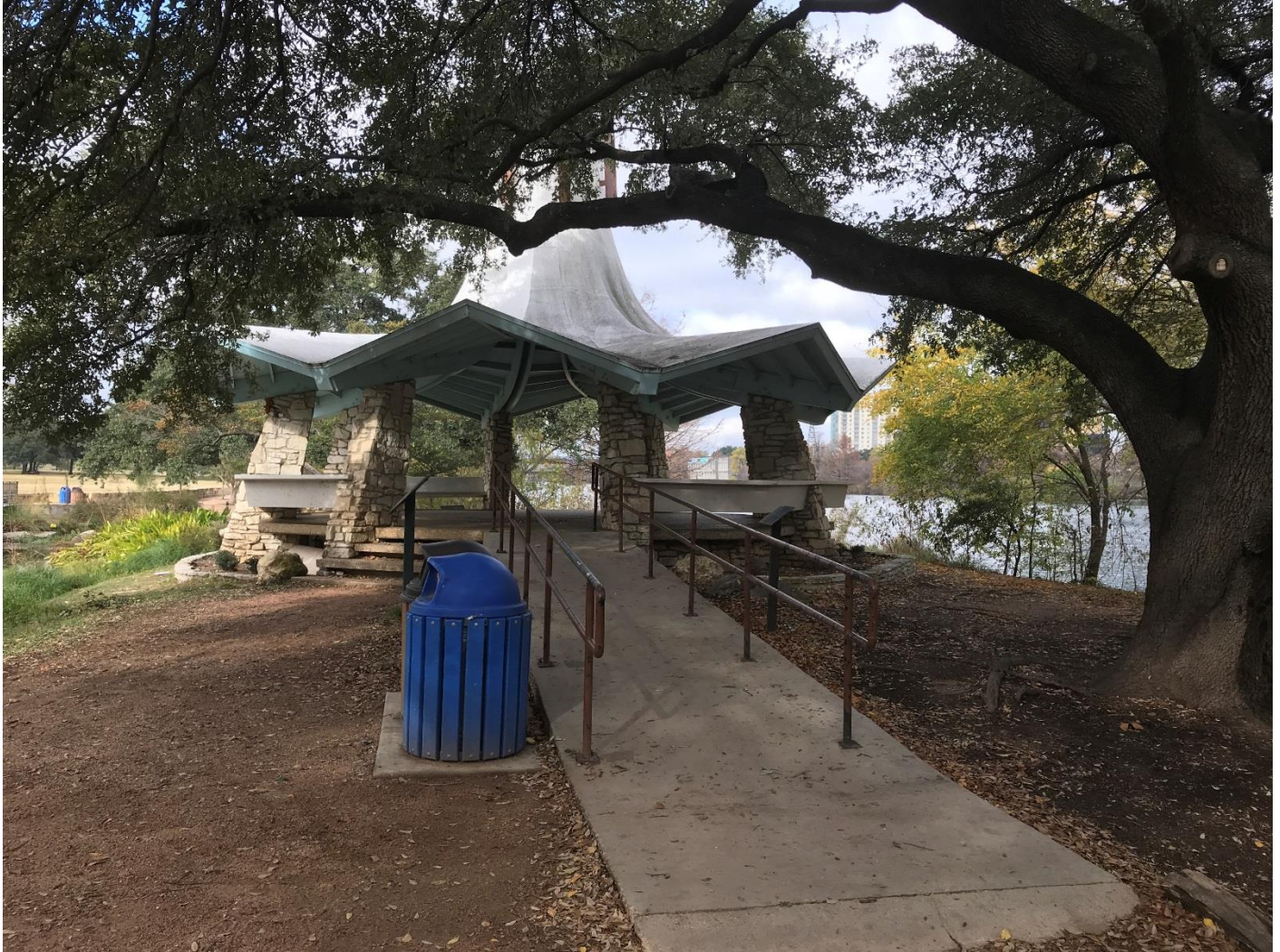
Photo 4 East elevation Camera facing west
