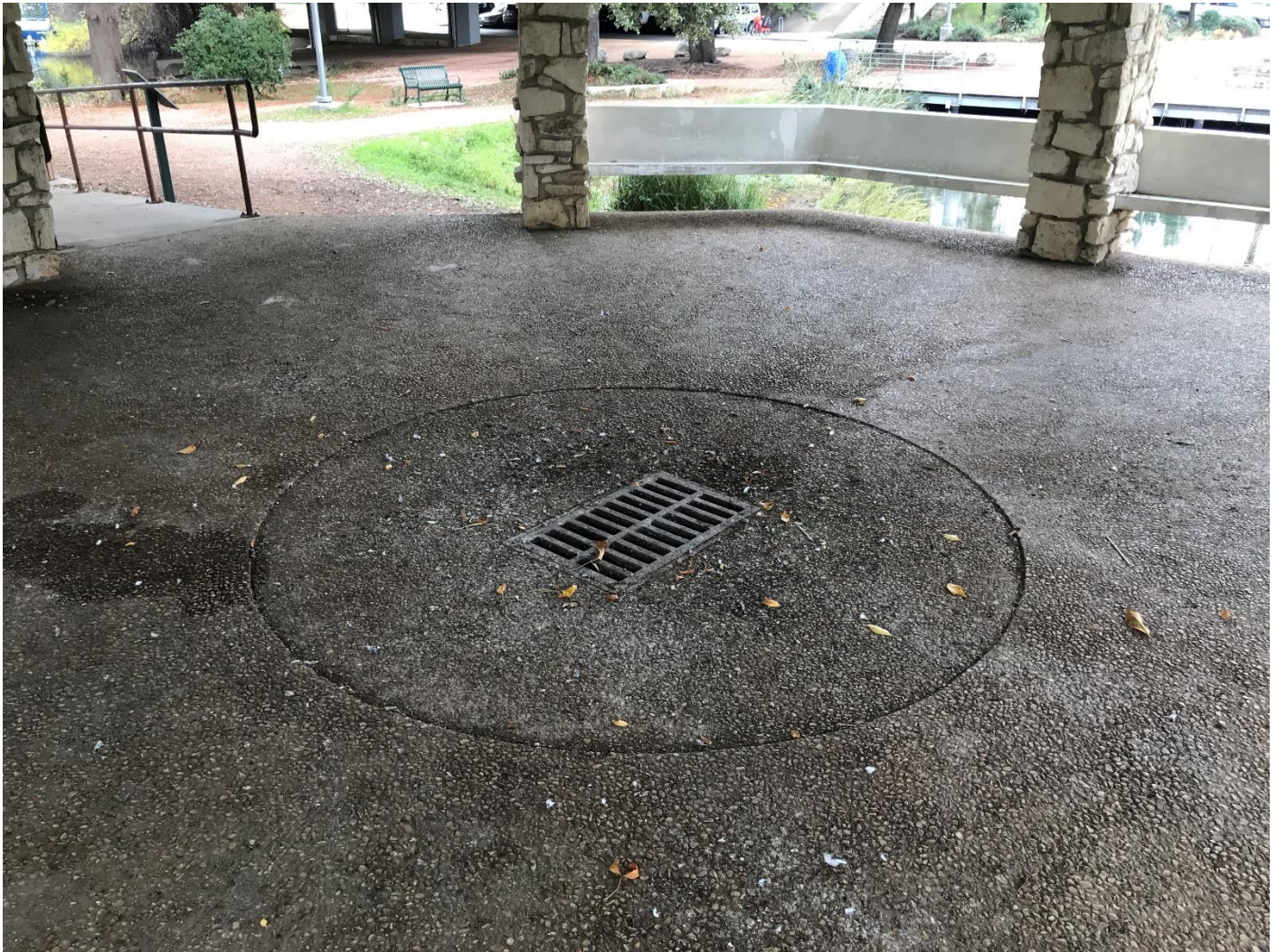
Photo 12 Cover with drain opening over central fountain Camera facing southeast
