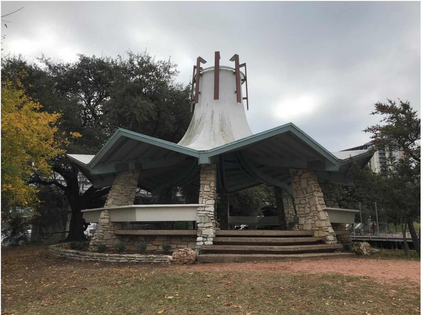
Photo 3 West elevation with steps Camera facing southeast
