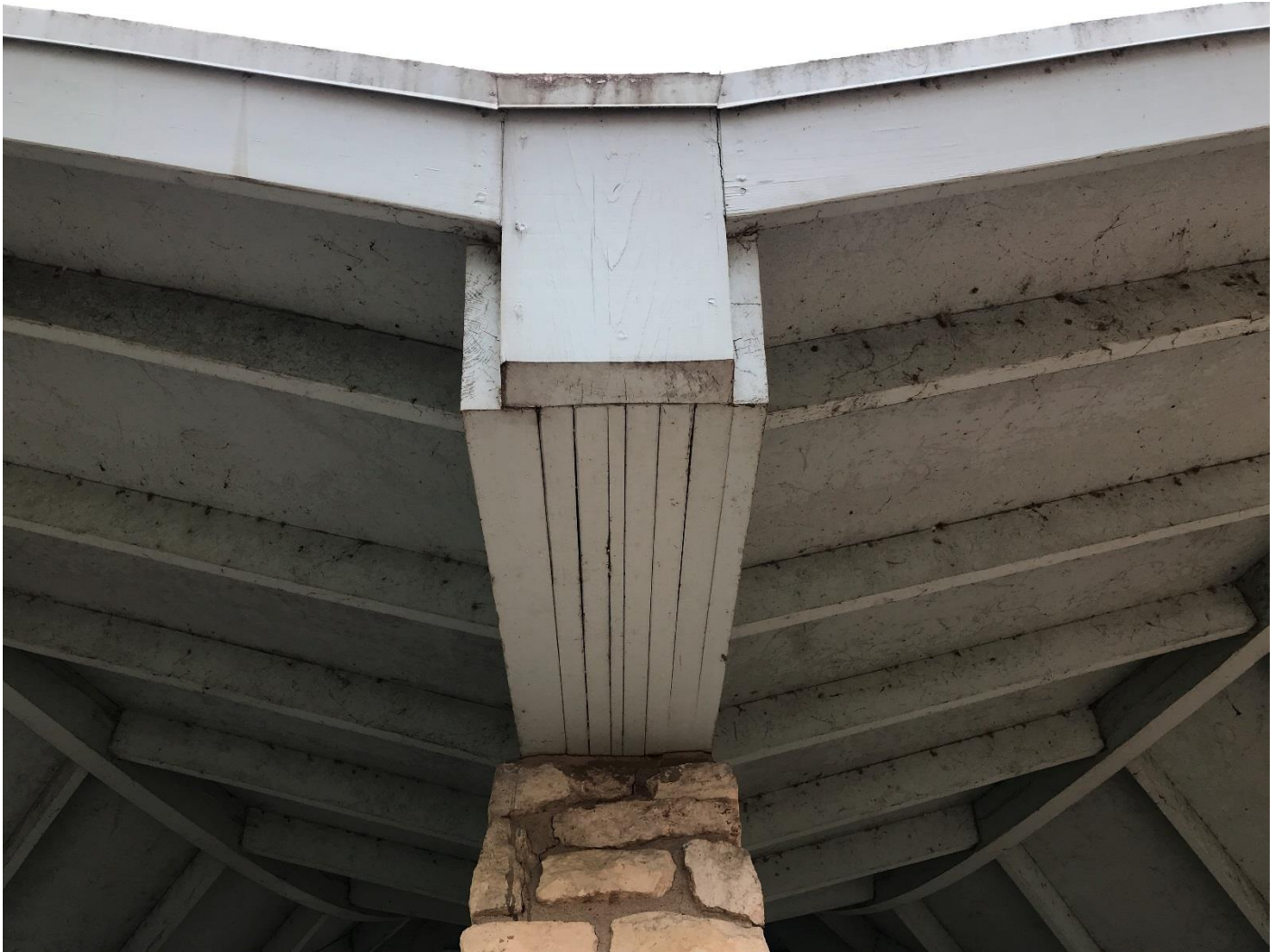
Photo 10 Detail of typical Glulam joist Camera facing east
