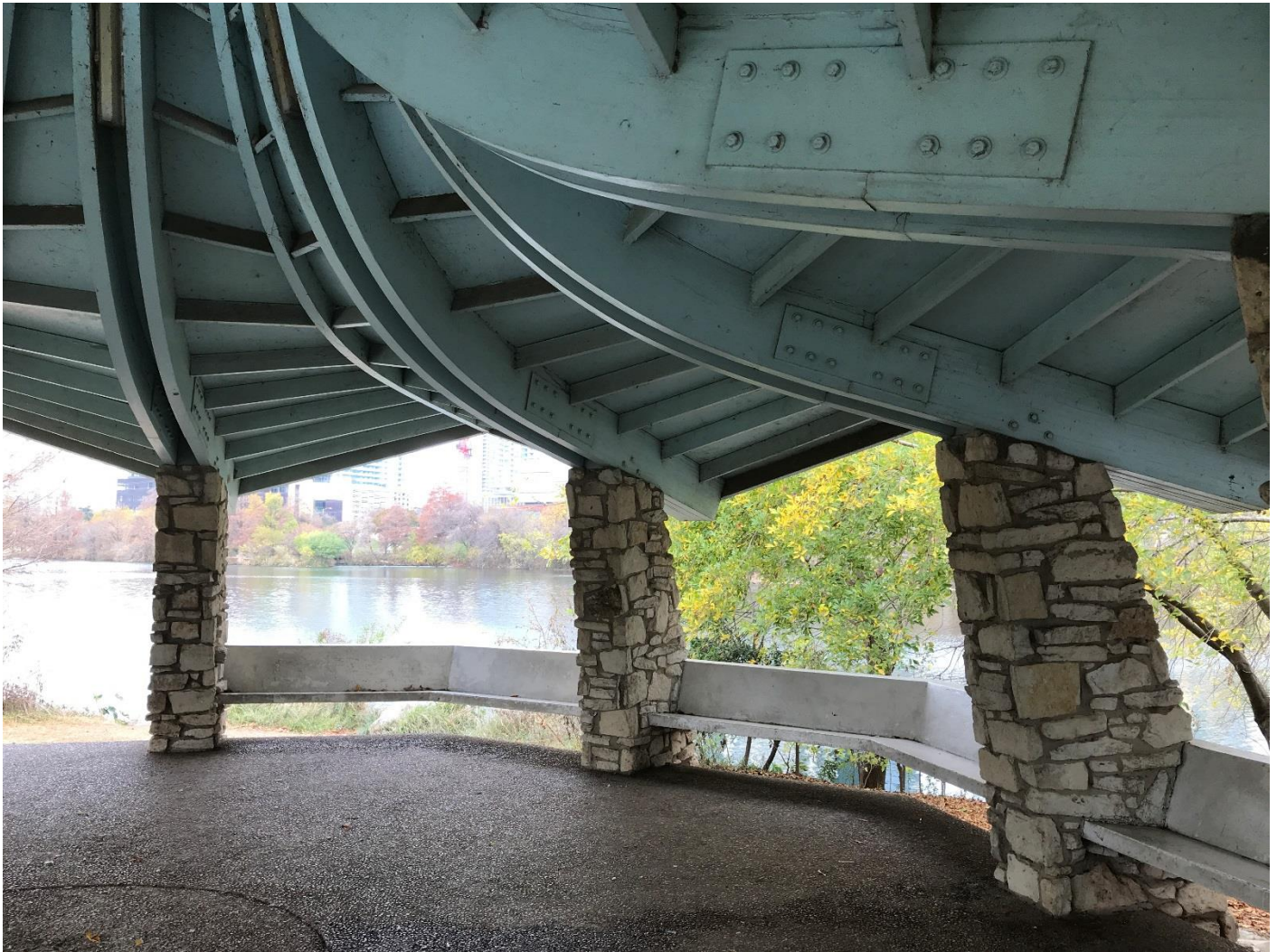
Photo 9 Glulam roof structure Camera facing northeast
