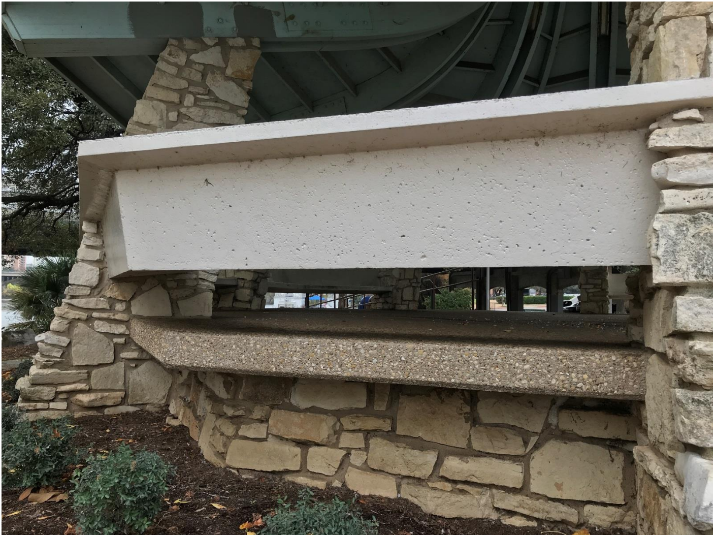
Photo 7 Concrete seating Camera facing west
