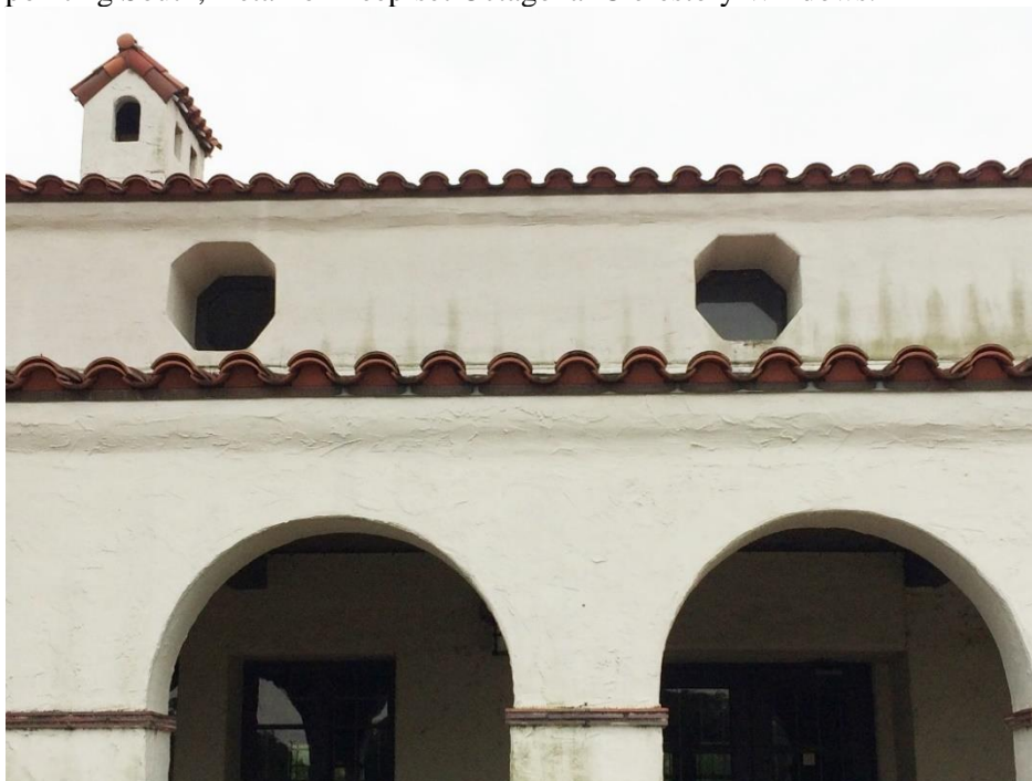
Photo 4 – Camera pointing South, Detail of Deep-set Octagonal Clerestory Windows.
