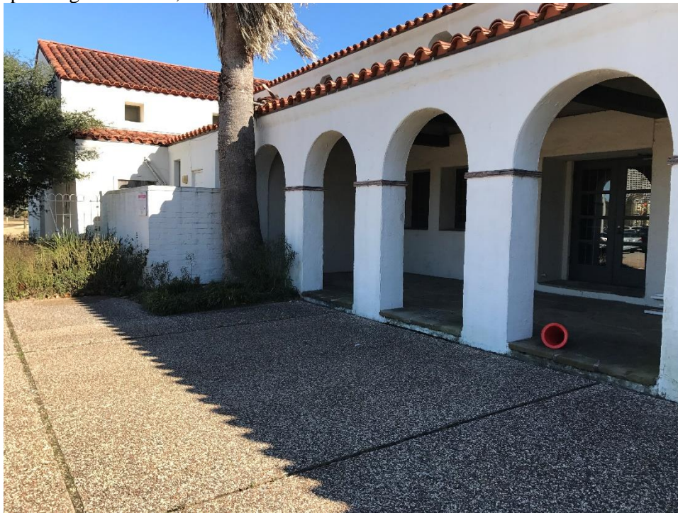
Photo 3 – Camera pointing South/East, Detail of Portico Columns.
