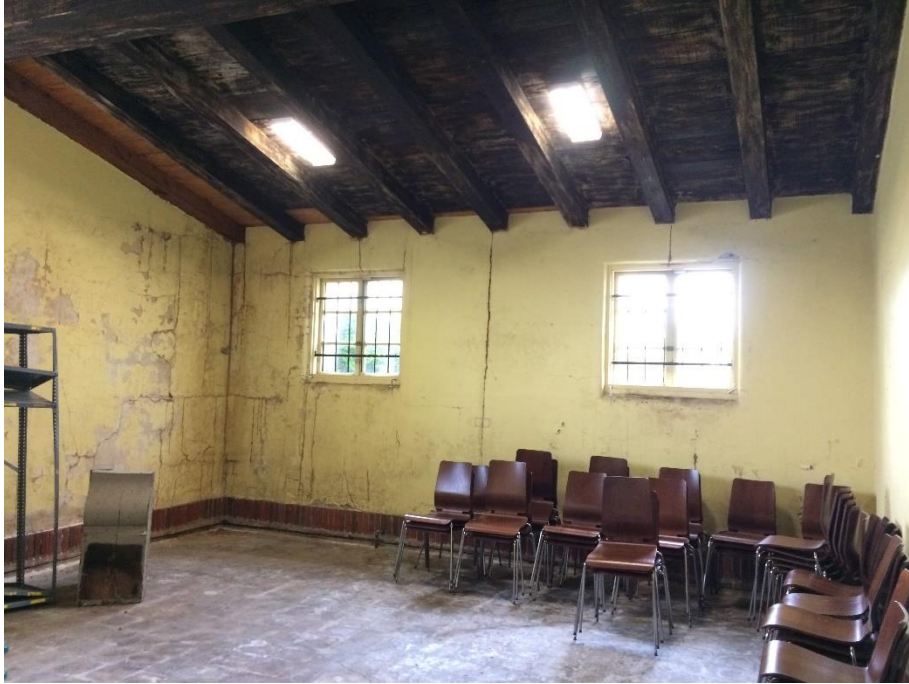
Photo 15 – Camera pointing North/West, Women’s Locker
