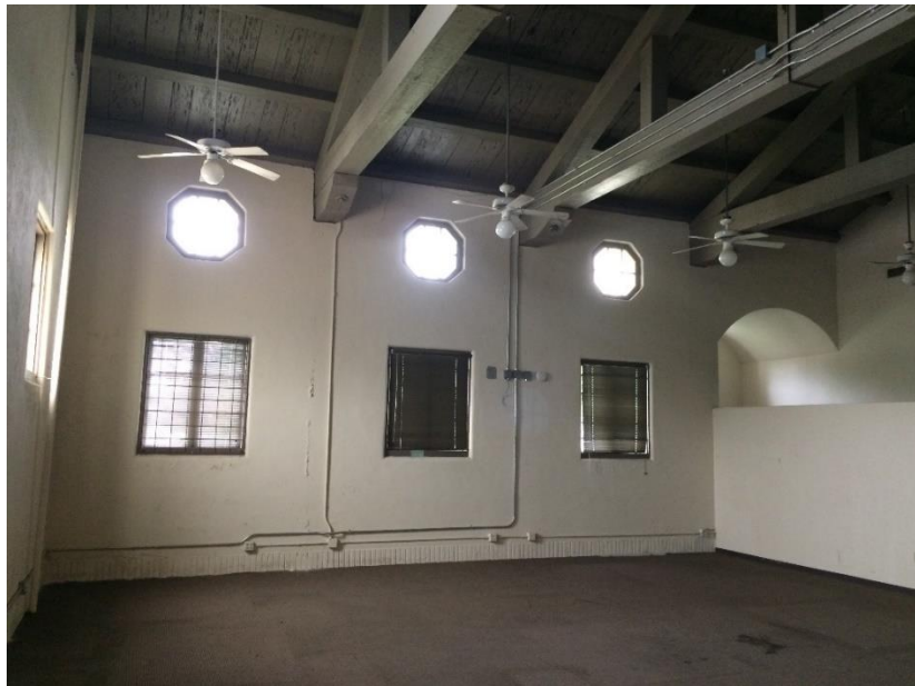
Photo 18 – Camera pointing East, Office 2.
