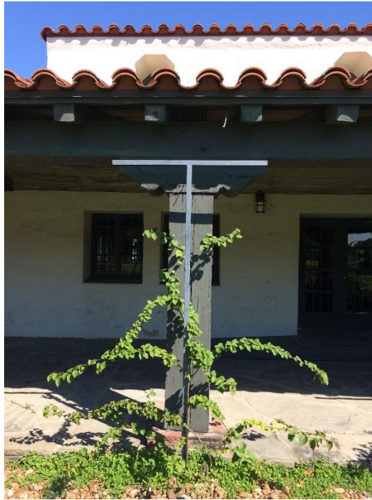
Photo 11 – Camera pointing North, Veranda Column
