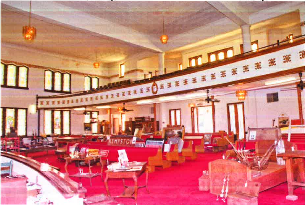
Photo 11: First floor interior showing structural beams and interior ornament. Sanctuary. View southeast.
