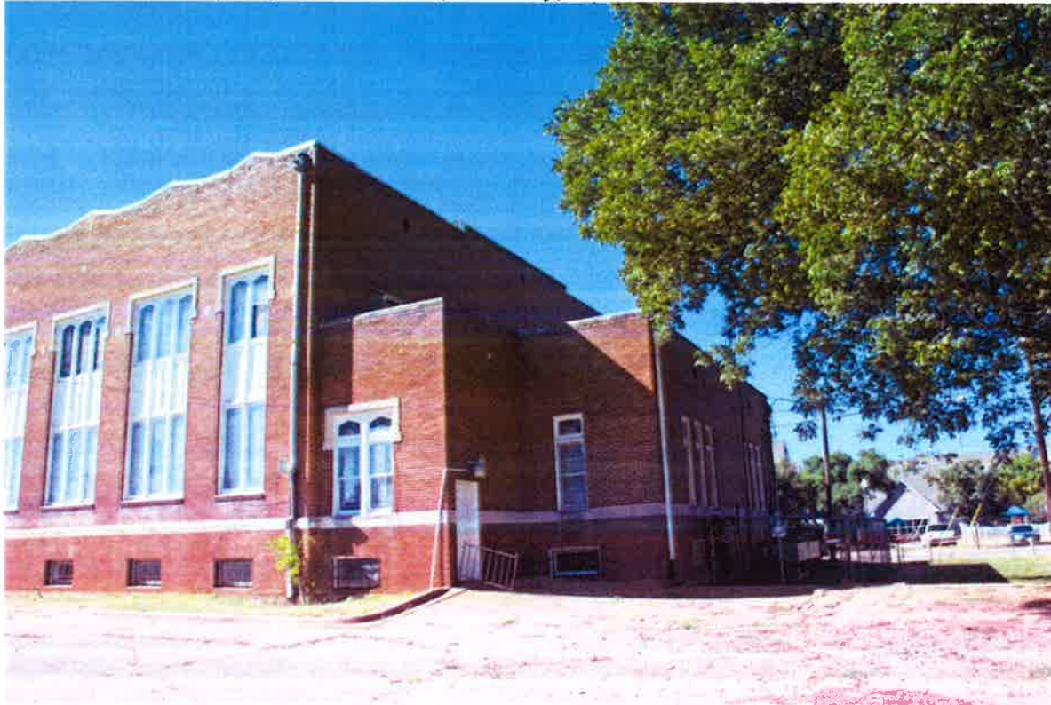
Photo 5: Northeast (Rear) and Southeast (Secondary) Elevations. View southwest.
