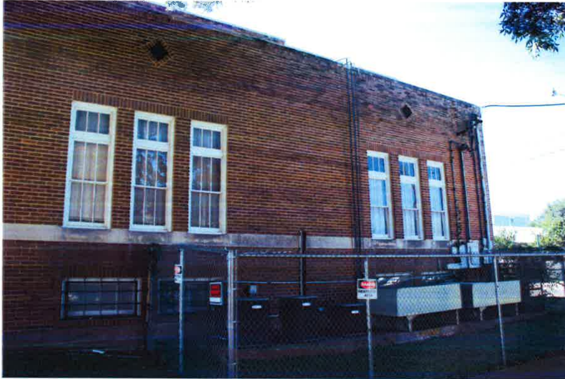
Photo 6: Northeast (Rear) Elevation. View southwest.
