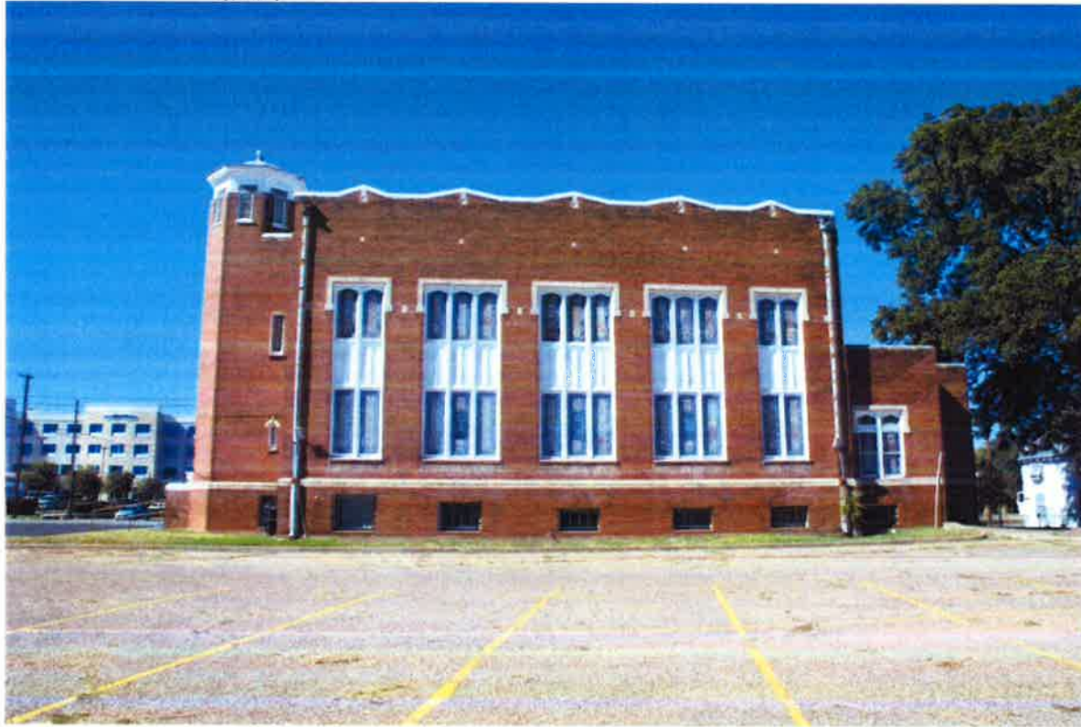
Photo 4: Southeast (Side) Elevation. View southwest.
