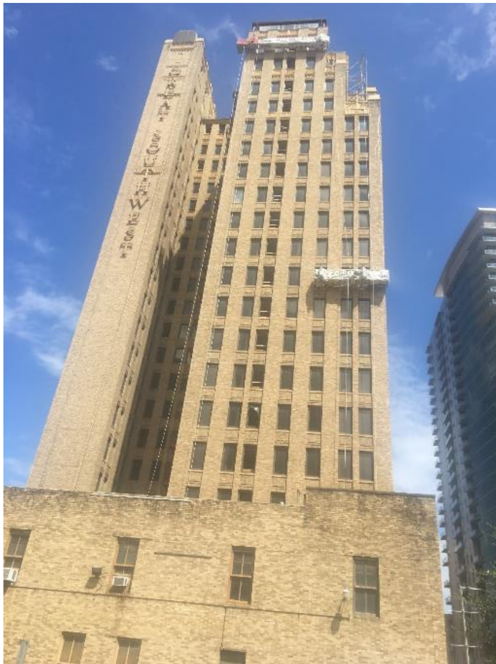
Photo 5: South elevation Camera facing north Date: 2018
