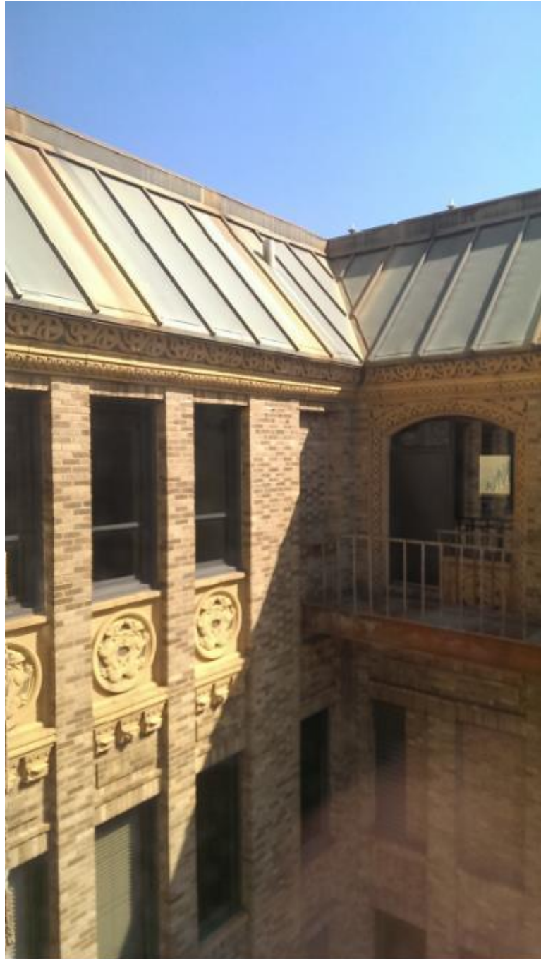
Photo 13: Exterior view of 21 st floor typical terra cotta detailing and copper roof Camera facing east Date: 2015
