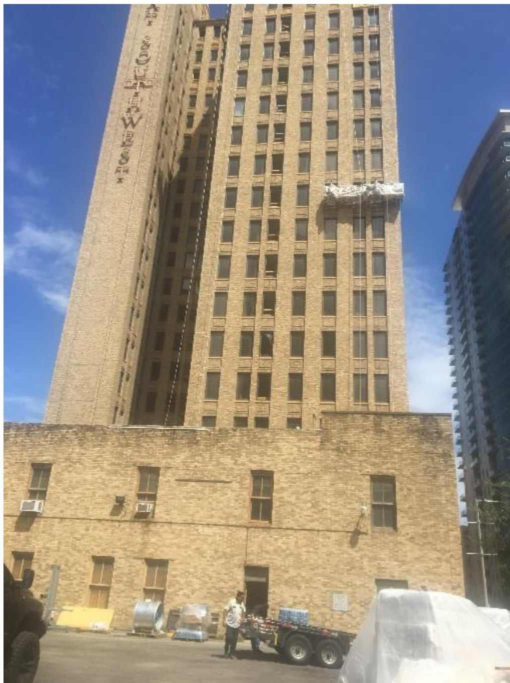
Photo 6: South elevation Camera facing north Date: 2018
