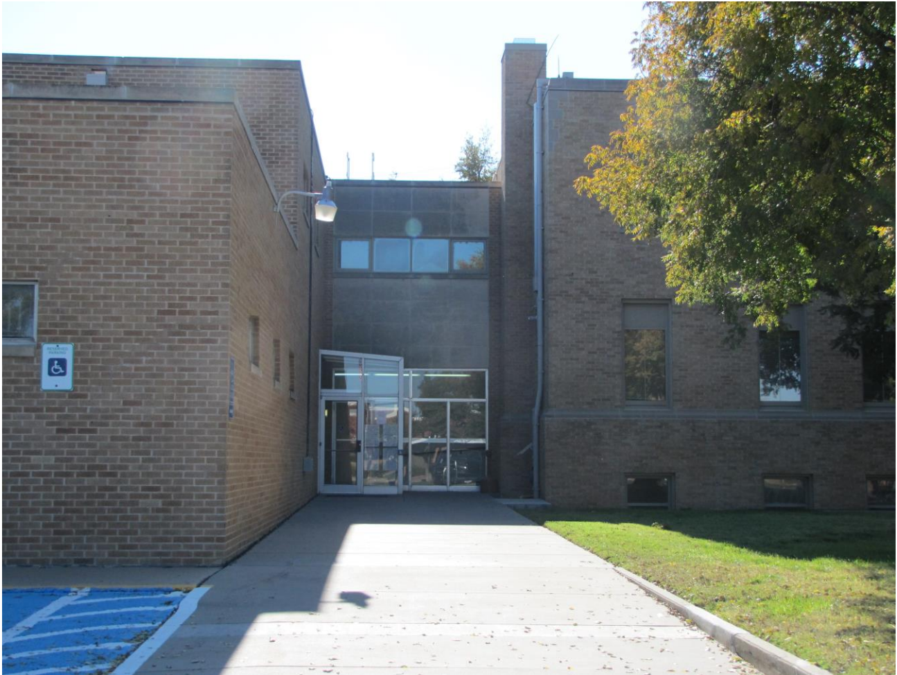
Photo 9: View of hyphen connection original courthouse and addition. Camera facing southwest.
