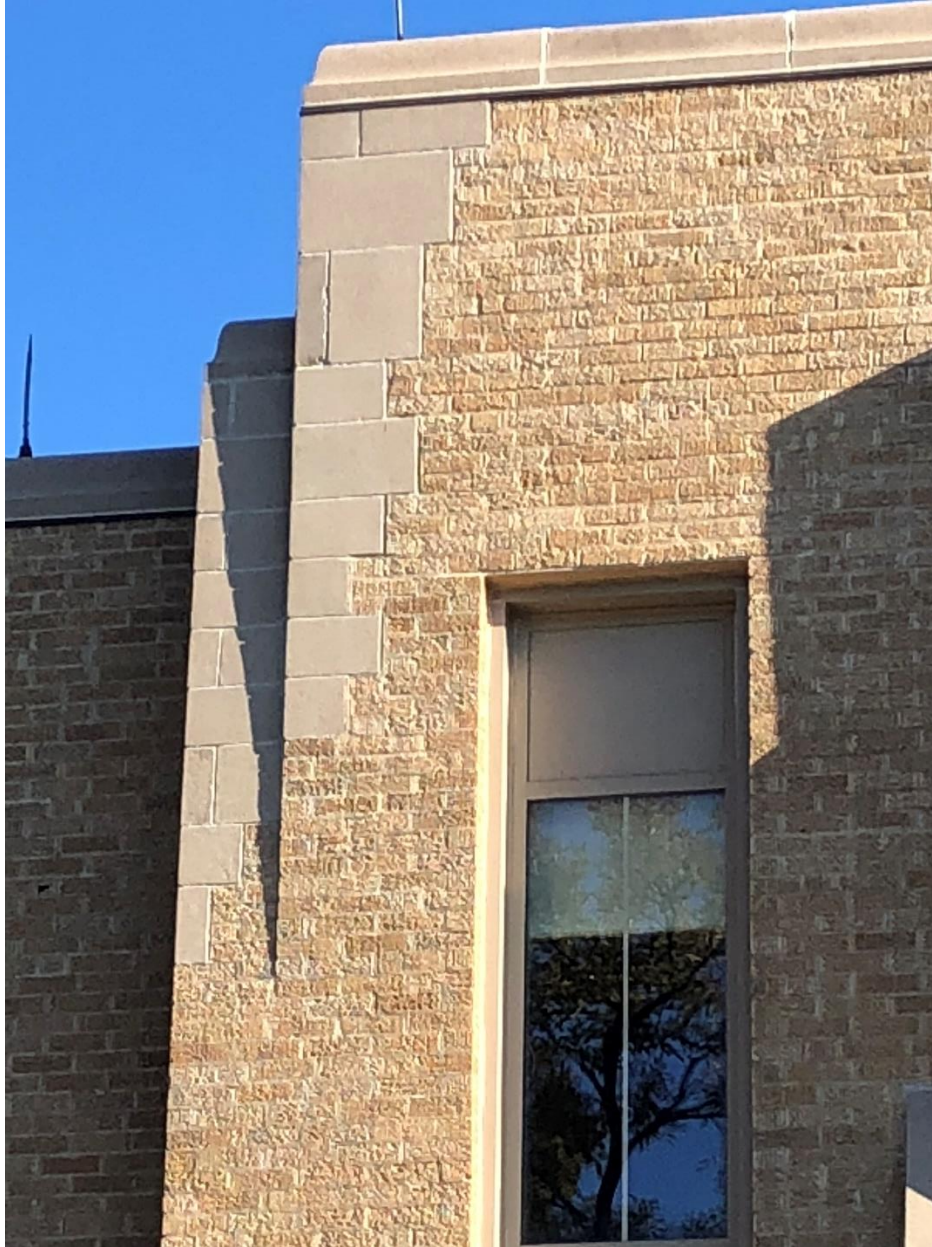
Photo 11: Stepped quoin detail on primary (northwest) elevation.
