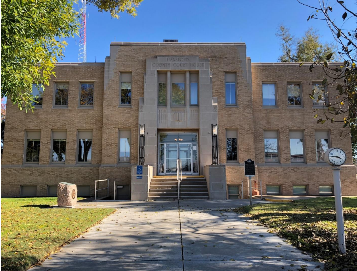
Photo 2: view of primary (northwest) elevation. Camera facing southeast.
