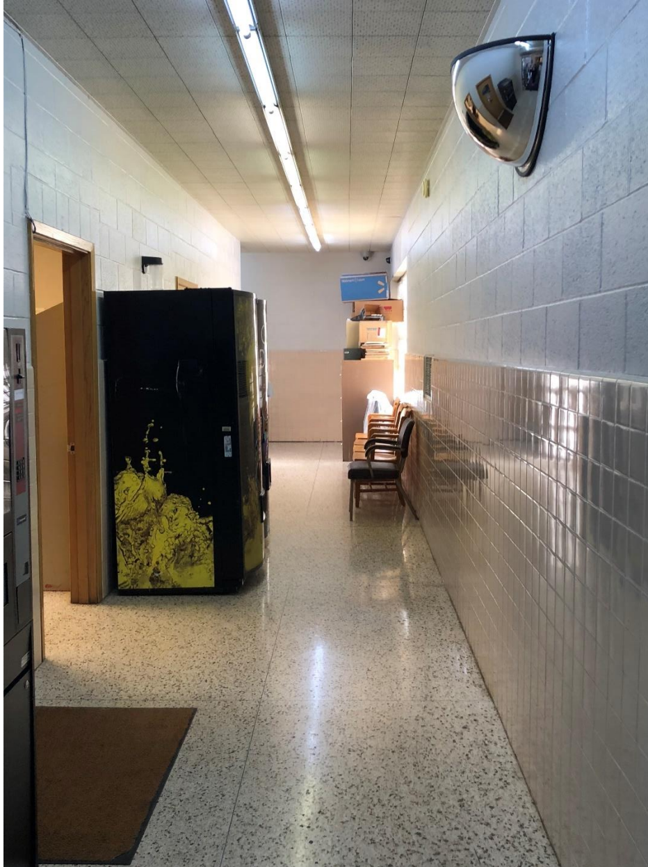
Photo 18: Typical first floor corridor in addition. Camera facing southeast.
