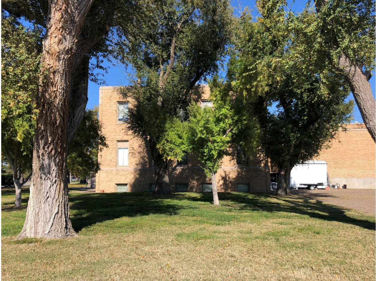
Photo 6: View of southwest elevation of 1931 courthouse. Camera facing northeast.
