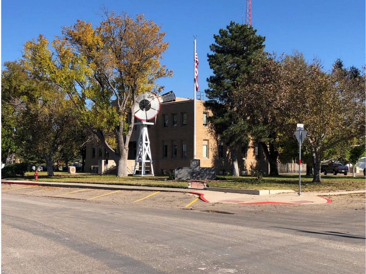
Photo 5: View of northwest and southwest elevations of 1931 courthouse. Non-contributing windmill visible. Camera facing east.
