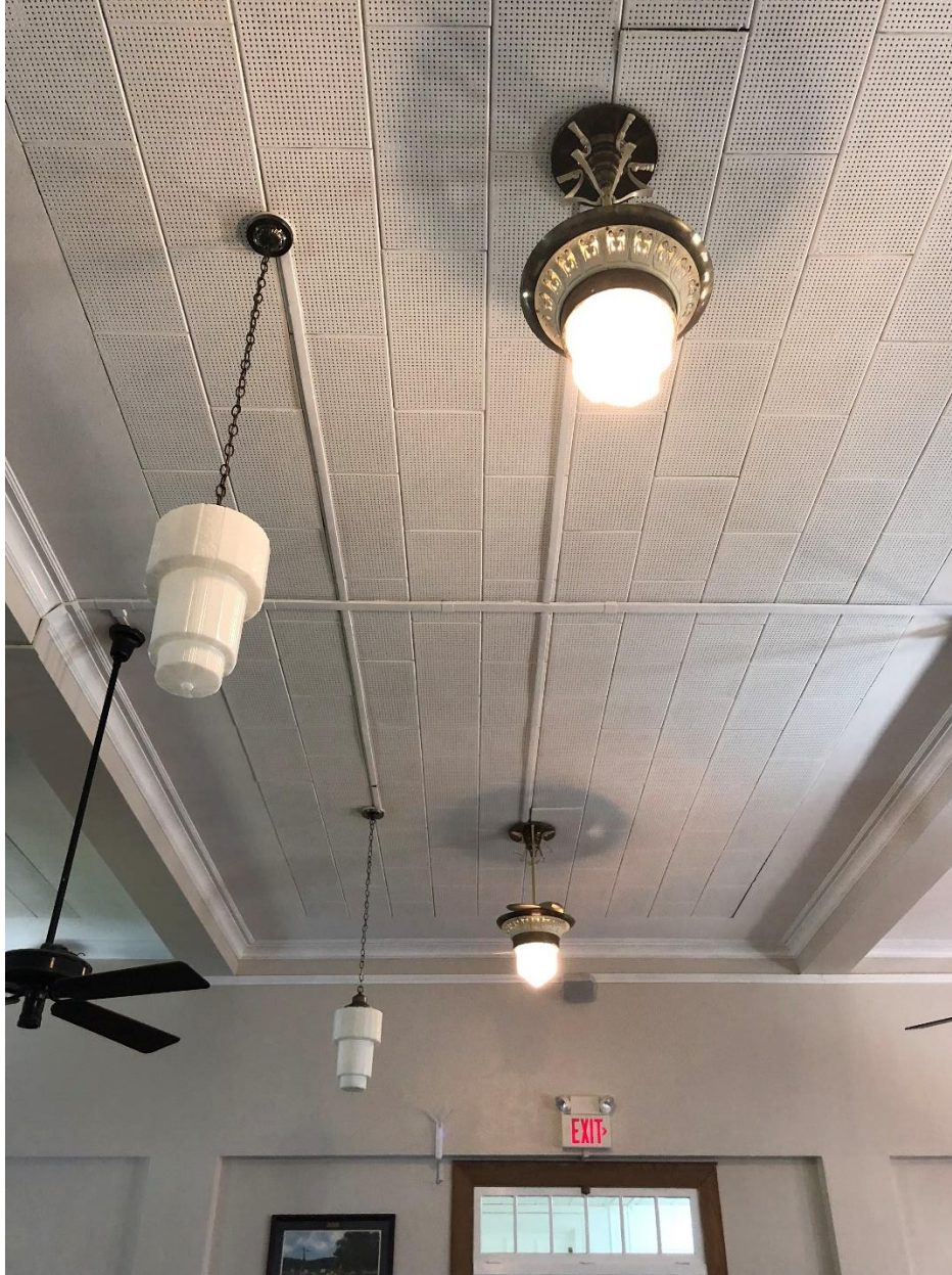
Photo 16: Original light fixtures in district courtroom.
