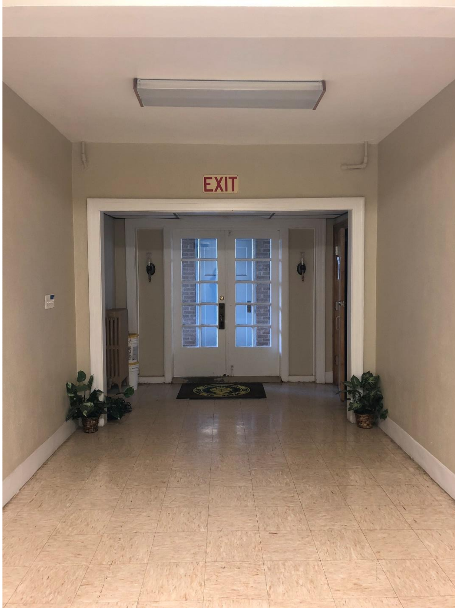
Photo 12: View of basement vestibule with original doors visible. Camera facing northwest.
