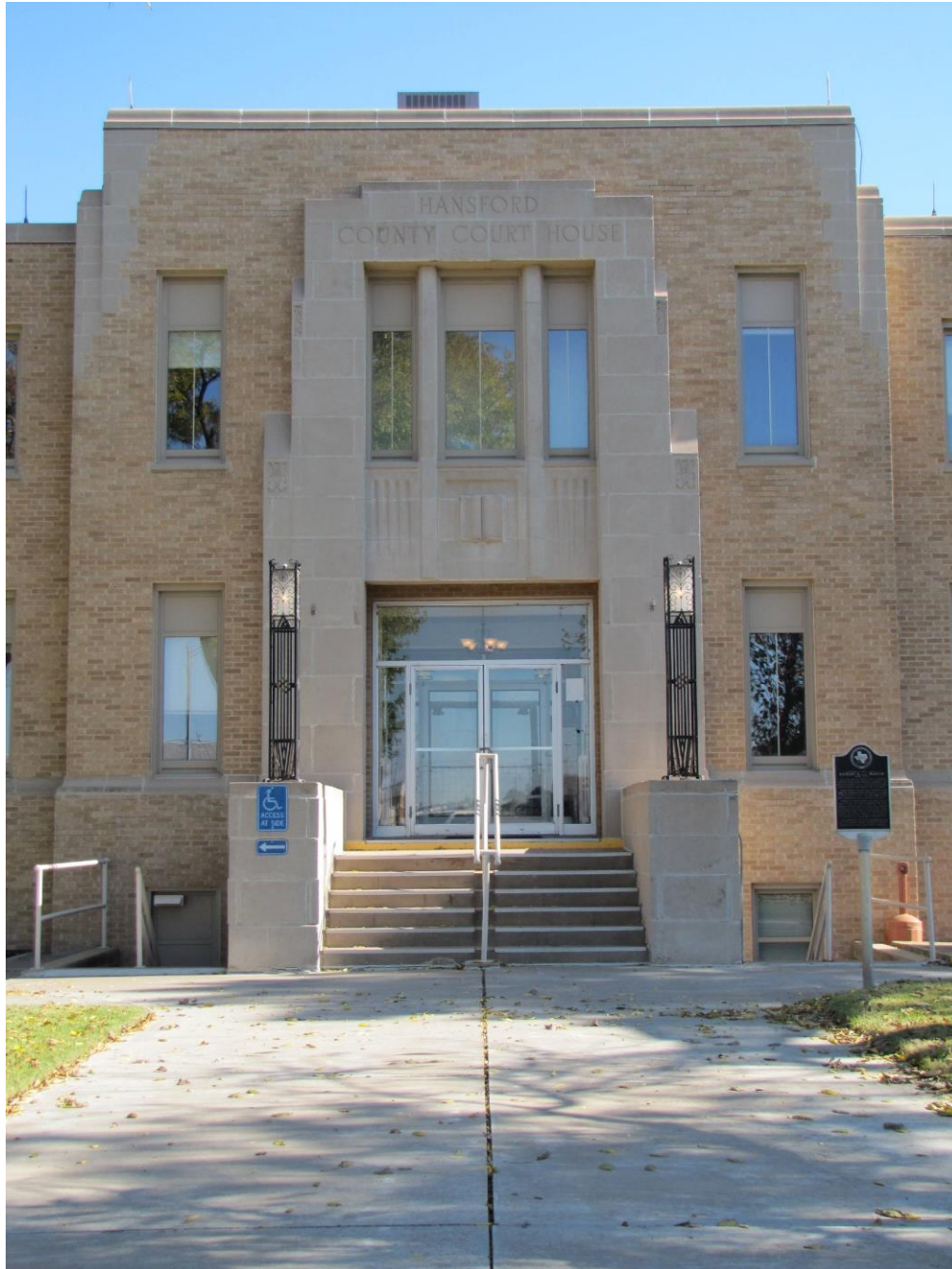
Photo 3: View of central entrance bay on primary (northwest) elevation. Camera facing southeast.
