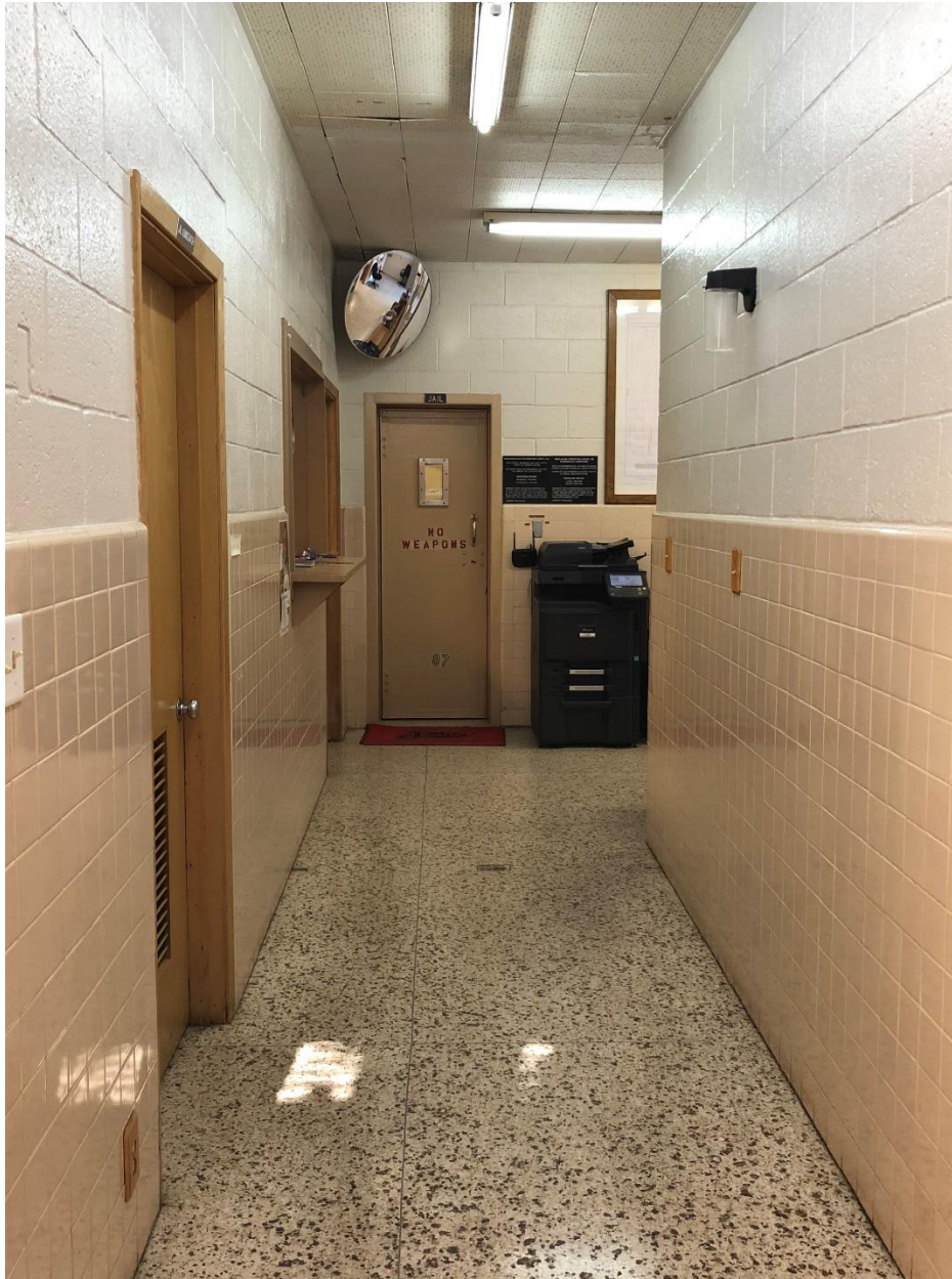
Photo 19: First floor corridor in addition showing entrance to jail. Camera facing northeast.
