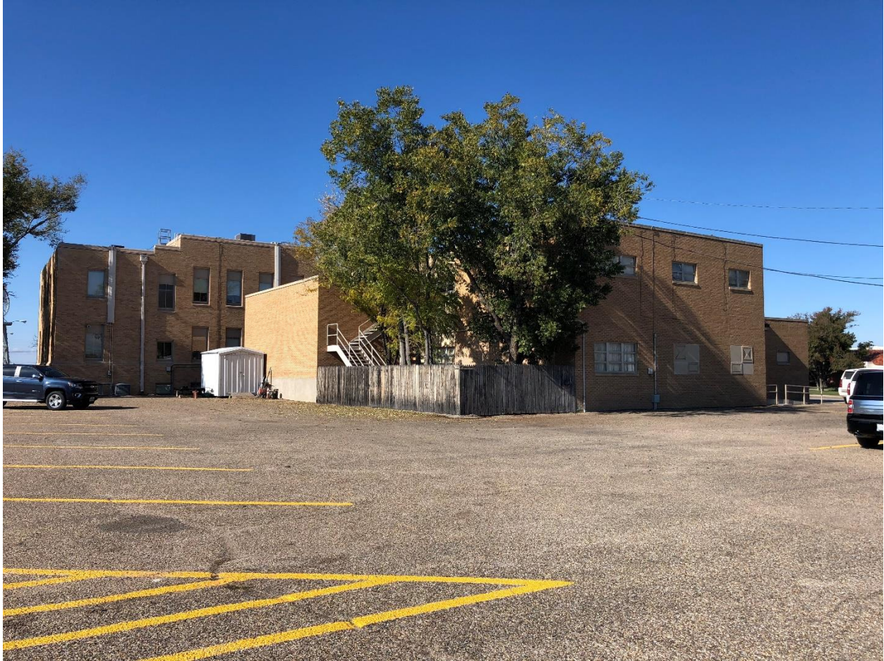
Photo 7: View of rear elevation of 1931 courthouse and 1958 addition. Camera facing north.
