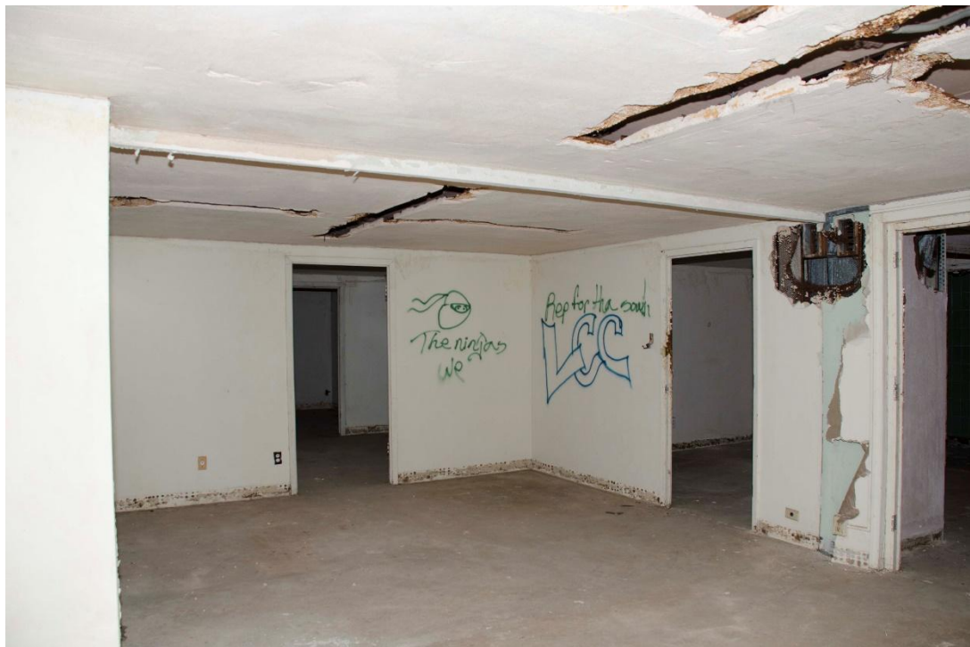
Photo 16: Fourth floor interior. Typical office. View south.
