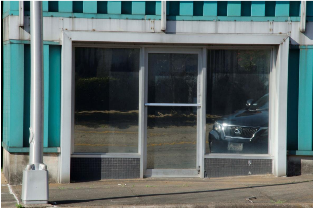
Photo 8: North (Primary) Elevation, detail of entrance. View south.
