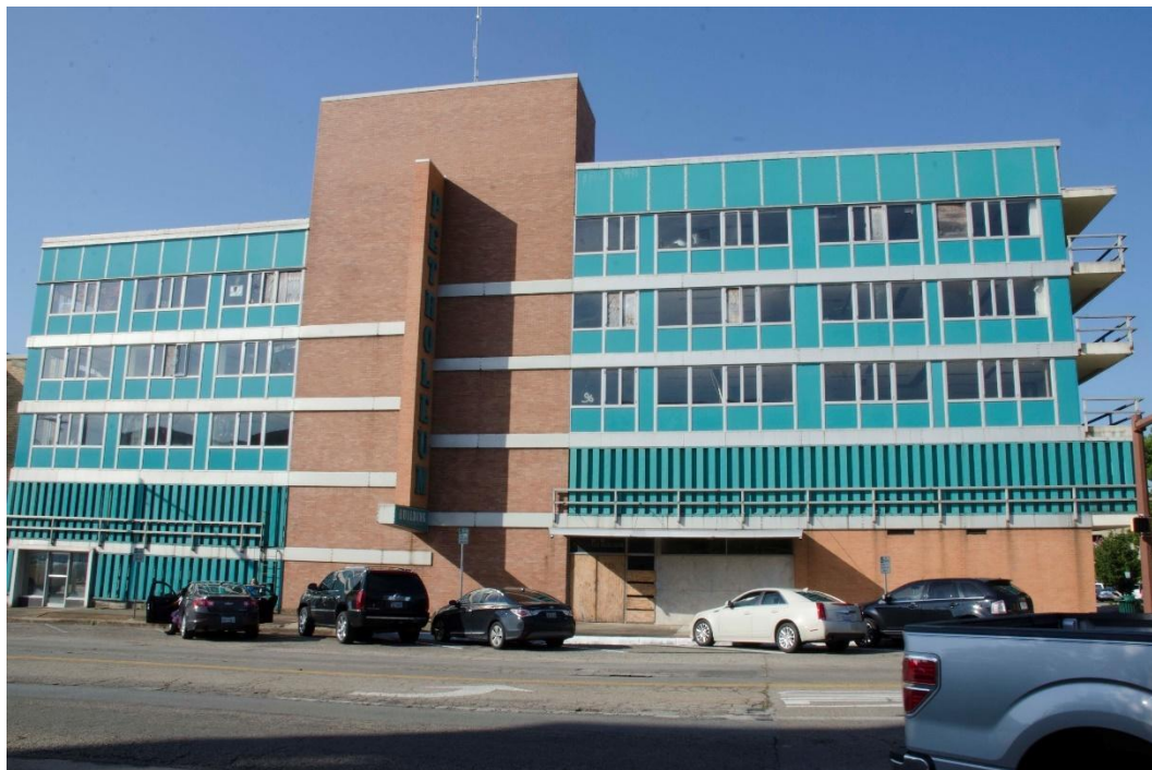
Photo 4: North (Primary) Elevation. View south.
