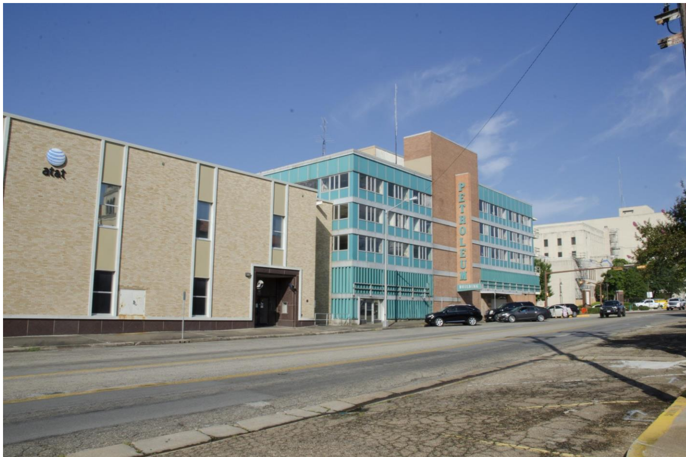
Photo 5: East and North (Primary) Elevations. View west.
