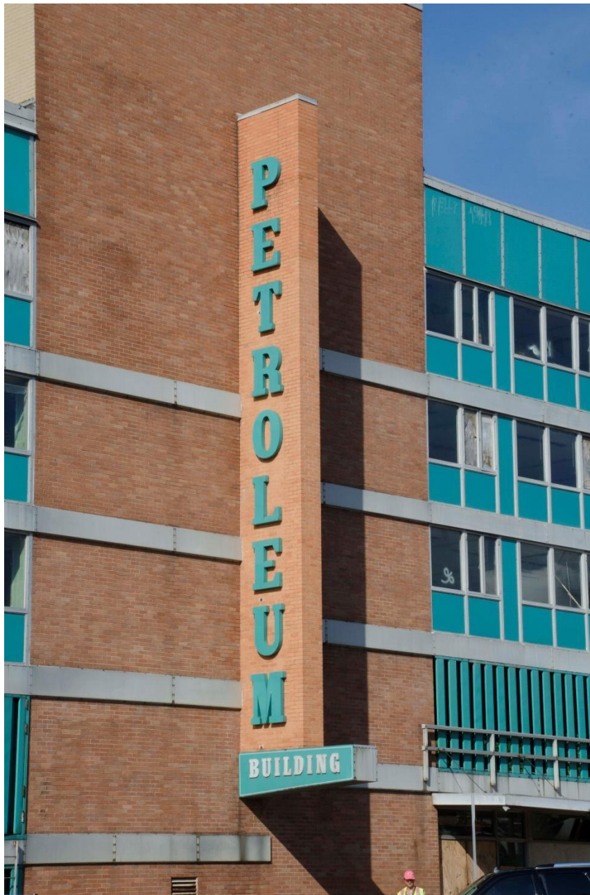
Photo 7: Signage Detail, North (Primary) Elevation. View southwest.
