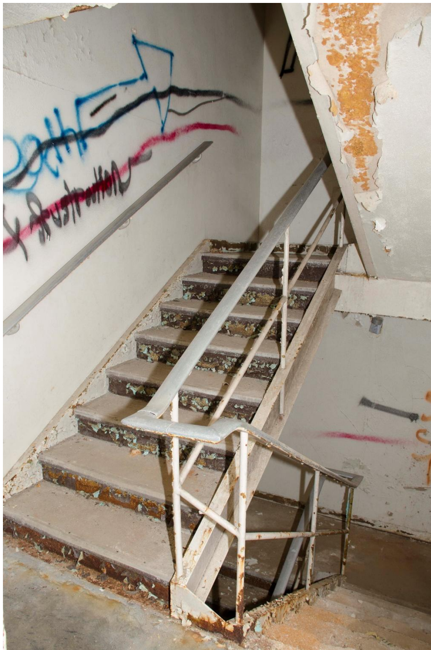
Photo 13: Third floor interior, detail of stair. View west.
