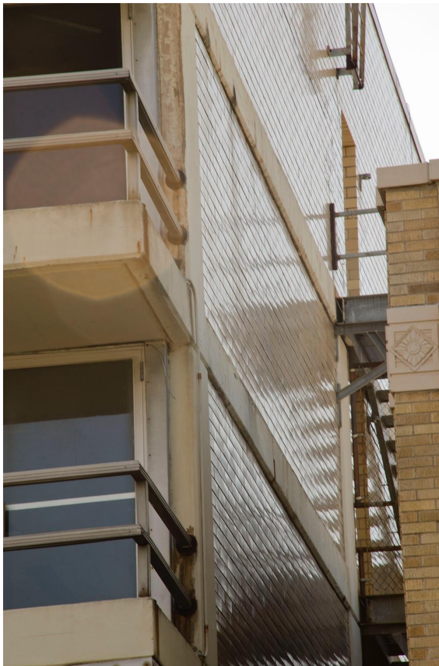
Photo 6: South Elevation. View east.
