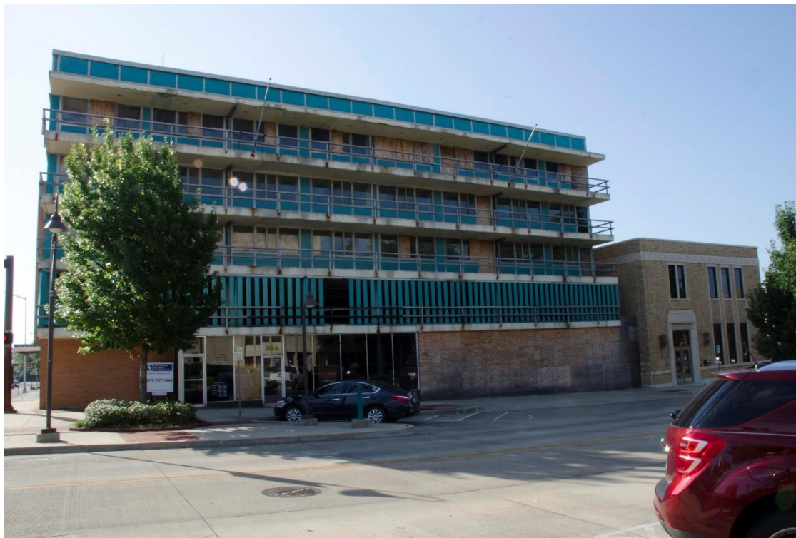
Photo 2: West (Secondary) Elevation. View southeast.
