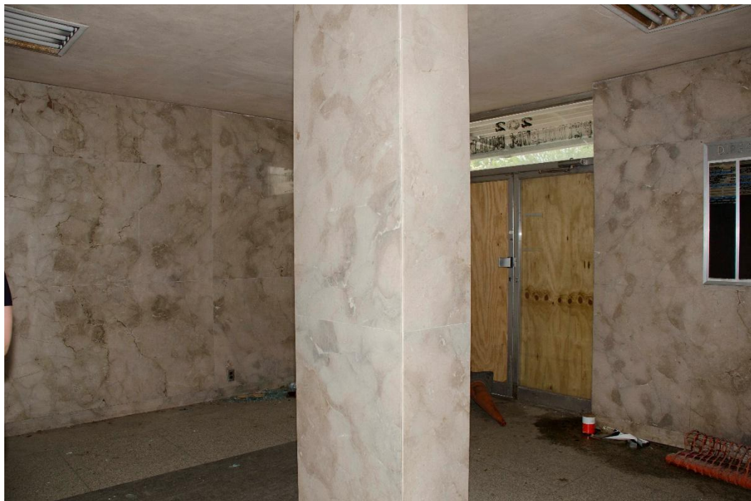
Photo 11: First floor interior. View northwest.
