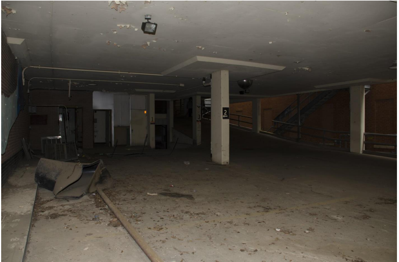
Photo 9: Parking garage ramp, first floor. View southeast.
