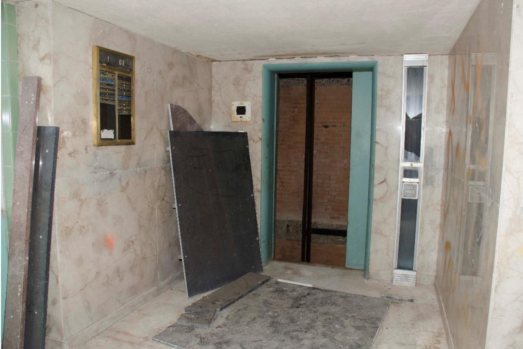
Photo 12: Third floor interior. View north.
