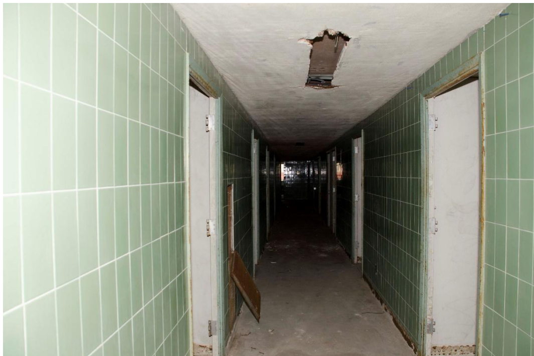
Photo 15: Fourth floor interior. View north.
