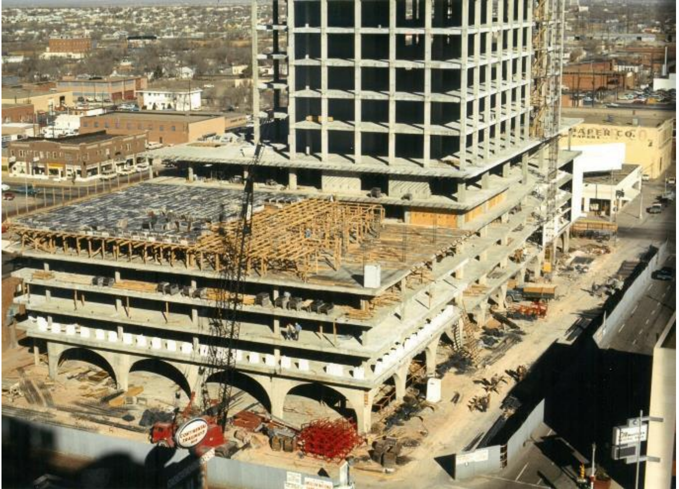
Figure 3: American National Bank Building and SPS Tower Under Construction, facing northwest c.1969 Source: Building Owner
