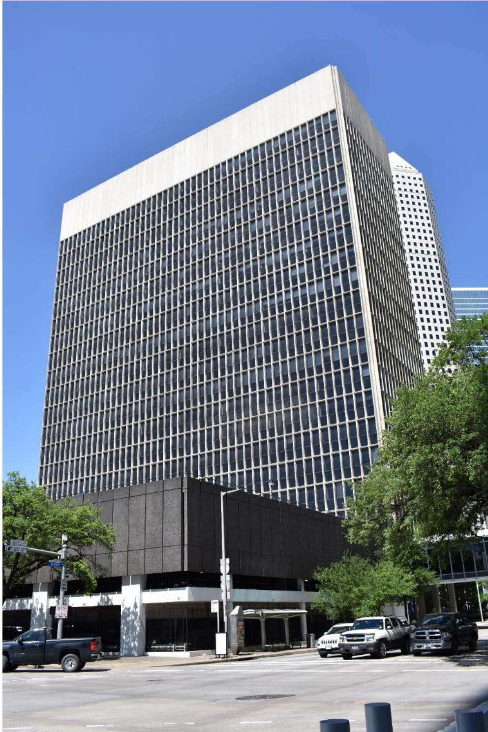
Photo 3 (TX_HarrisCounty_500Jefferson_0003) South (rear) elevation of office tower, view northwest
