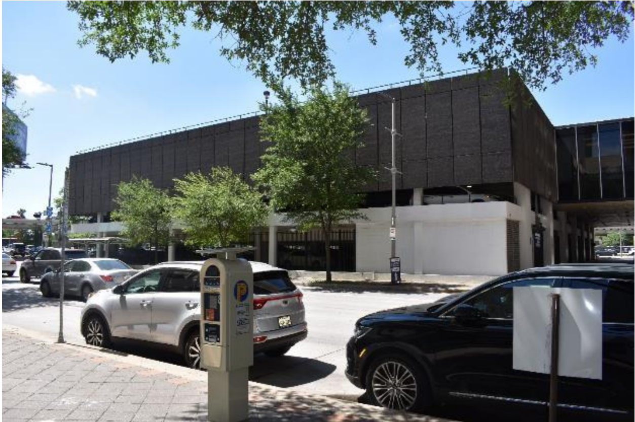
Photo 5 (TX_HarrisCounty_500Jefferson_0005) East (side) elevation of garage, view southwest
