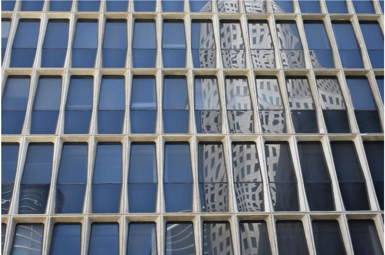
Photo 8 (TX_HarrisCounty_500Jefferson_0008) Mo-Sai panels on north façade, typical, view south
