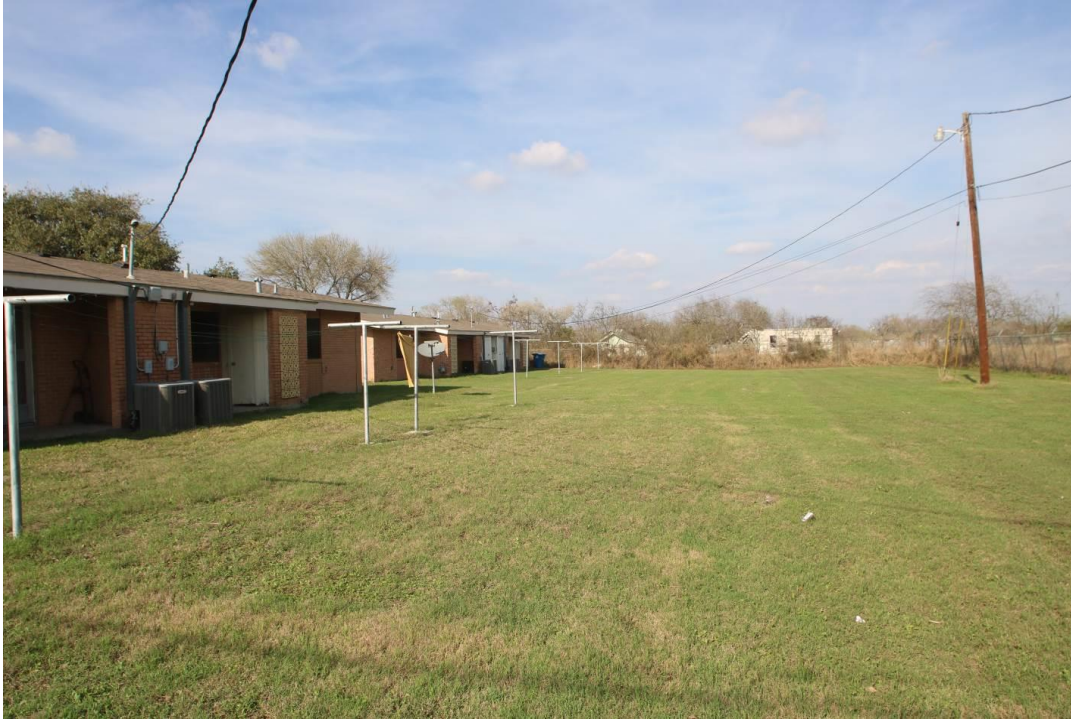
View of Rear Lawn with Building 2 (left) and Building 3 (right), looking northeast
