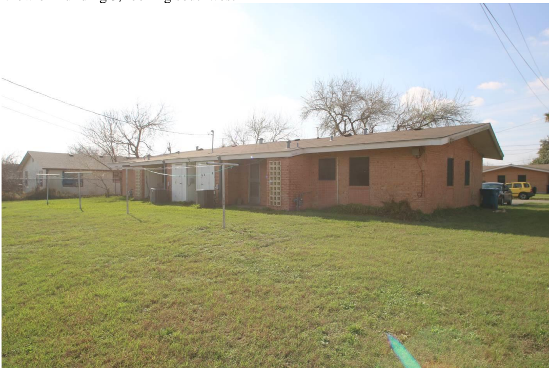
View of Building 3, looking southwest
