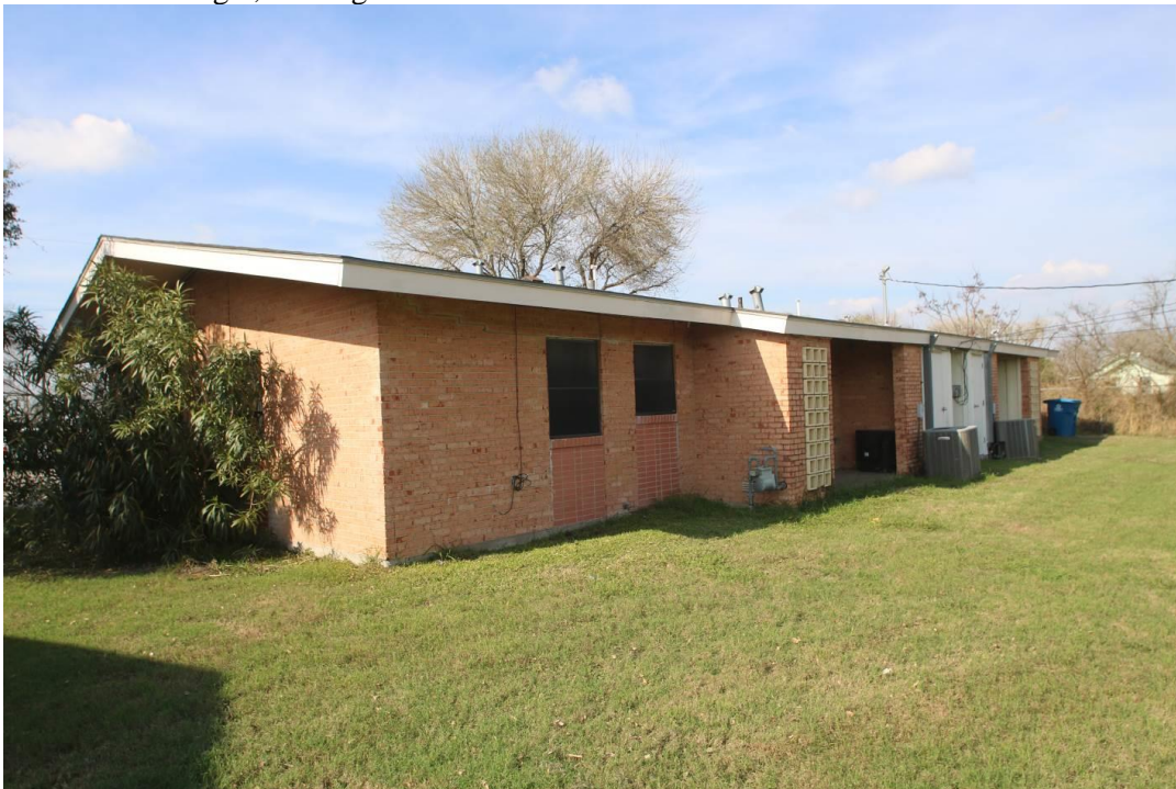
View of Building 1, looking northwest
