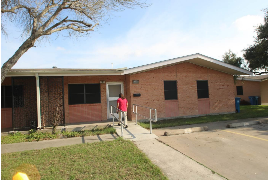
View of Building 1, looking southeast
