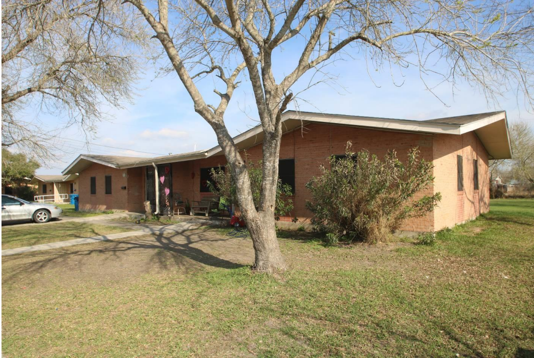
View of Building 3, looking northeast
