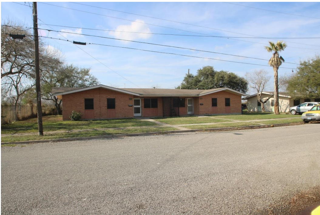
Photo 8 View of Building 4, looking east
