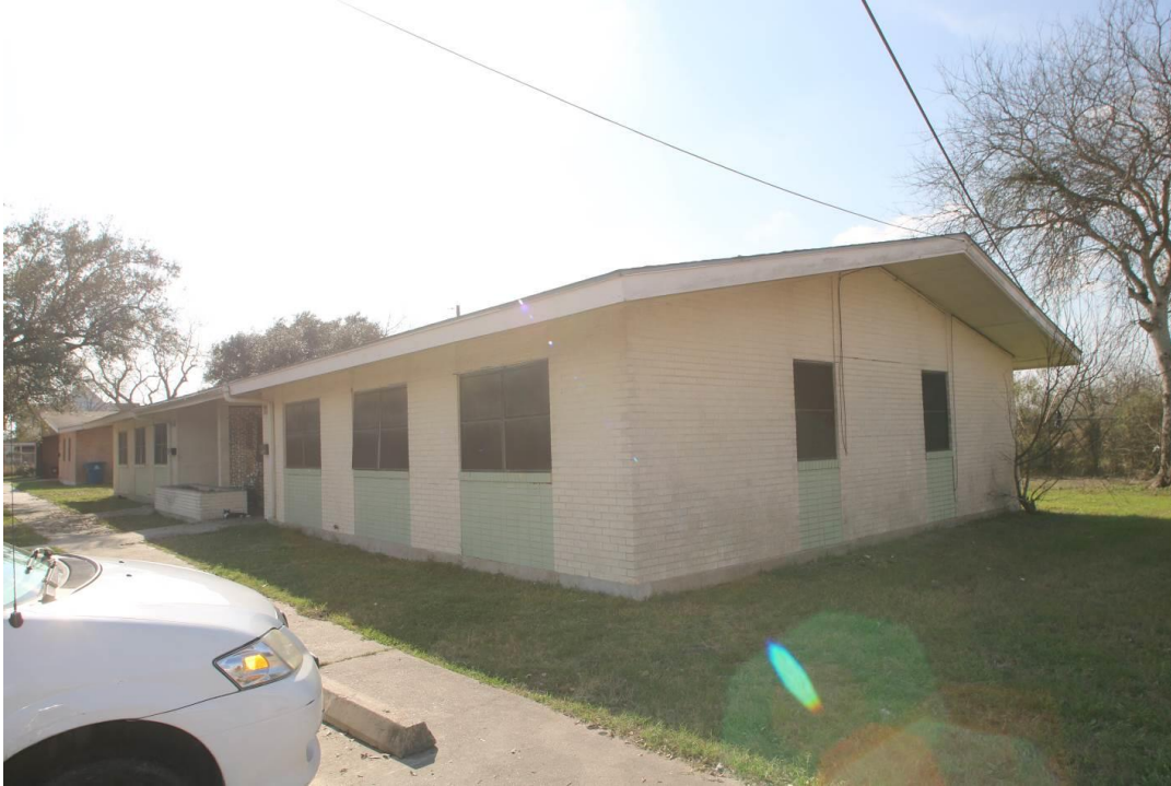
Photo 7 View of Building 5, looking southwest
