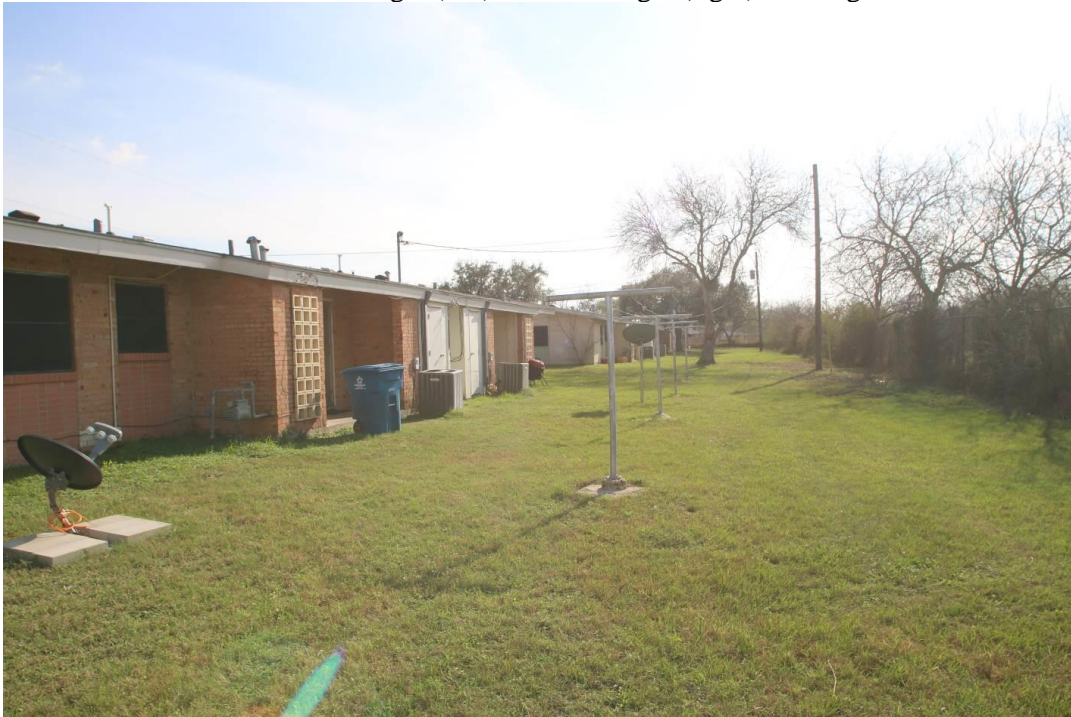
View of Rear Lawn with Building 6 (left) and Building 5 (right), looking southwest
