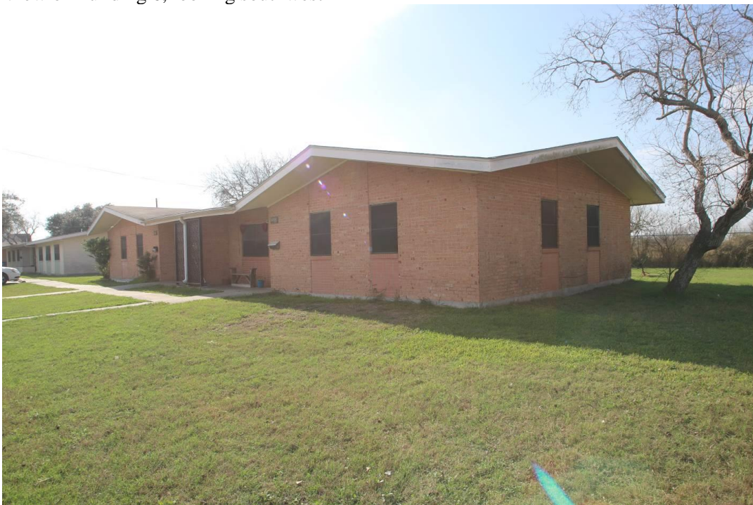
Photo 6 View of Building 6, looking southwest
