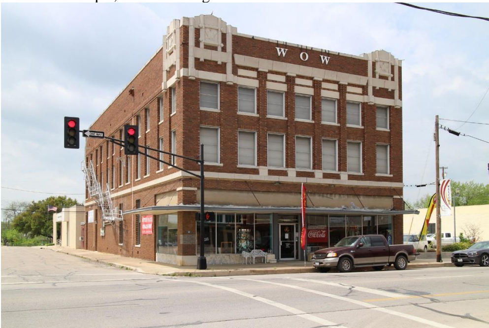
Photo 38 Building at 201 N. Main Street (Property #92) Southeast oblique, camera facing northwest
