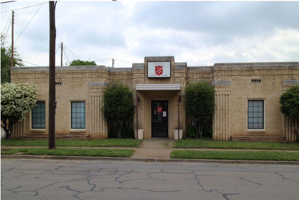
Photo 16 Building at 111 S. Anglin Street (Property #7) West elevation, camera facing east
