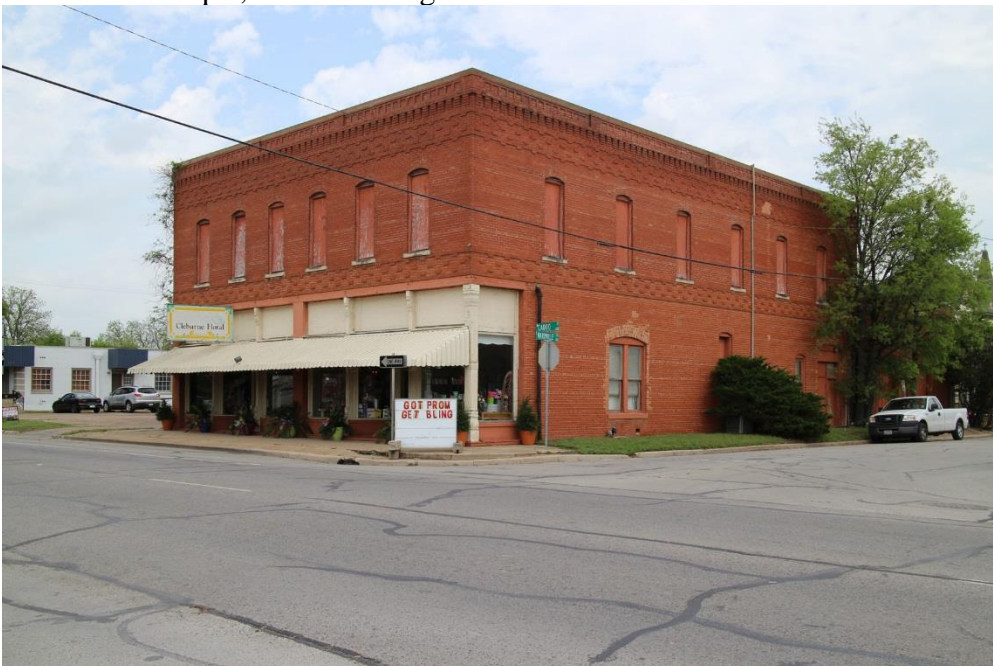
Photo 22 Building at 202-204 N. Caddo Street (Property #18) Southwest oblique, camera facing northeast
