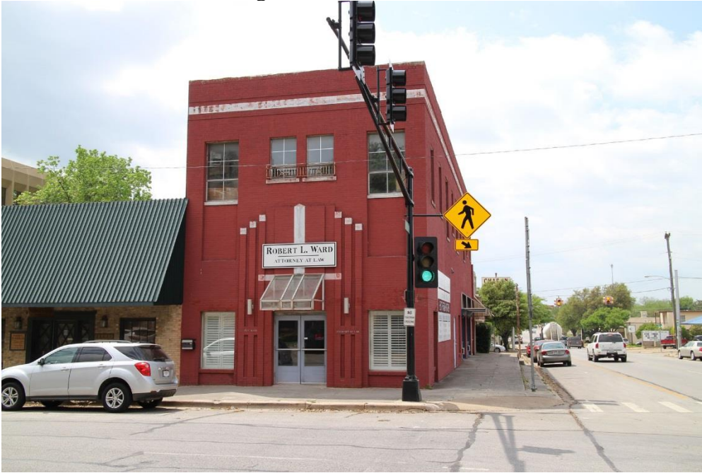
Photo 35 Building at 15 N. Main Street (Property #88) East elevation, camera facing west
