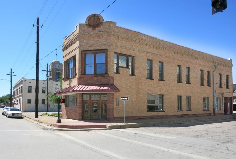
Photo 25 Building at 115 E. Chambers Street (Property #37) Southeast oblique, camera facing northwest
