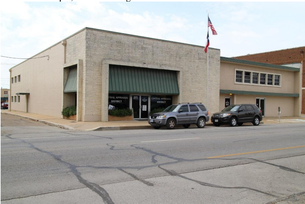
Photo 36 Building at 109-111 N. Main Street (Property #89) Southeast oblique, camera facing northwest
