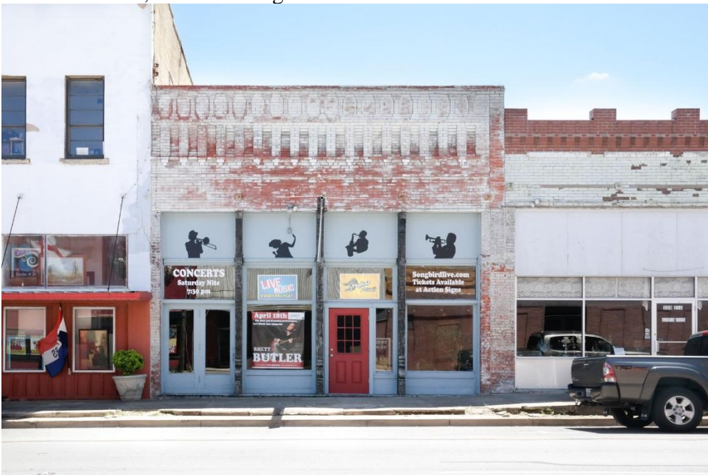
Photo 32 Building at 210 E. Henderson Street (Property #68) North elevation, camera facing south
