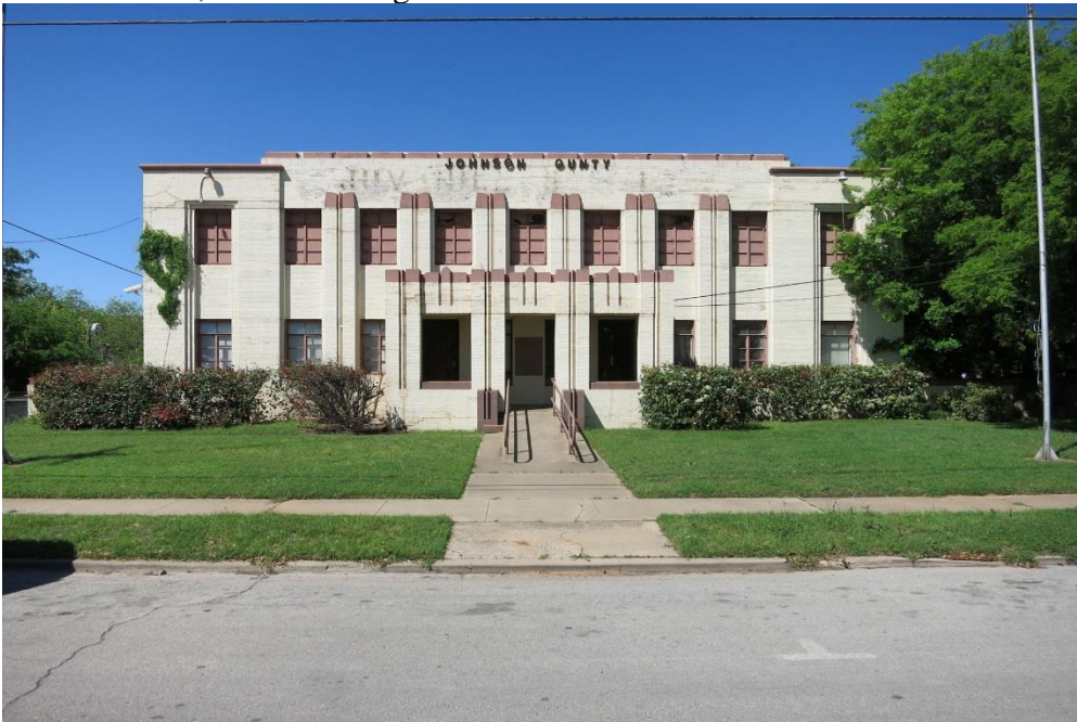
Photo 42 Building at 110 S. Mill Street (Property #114) East elevation, camera facing west
