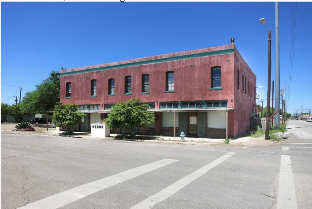
Photo 34 Building at 419-423 E. Henderson Street (Property #76) South elevation, camera facing north
