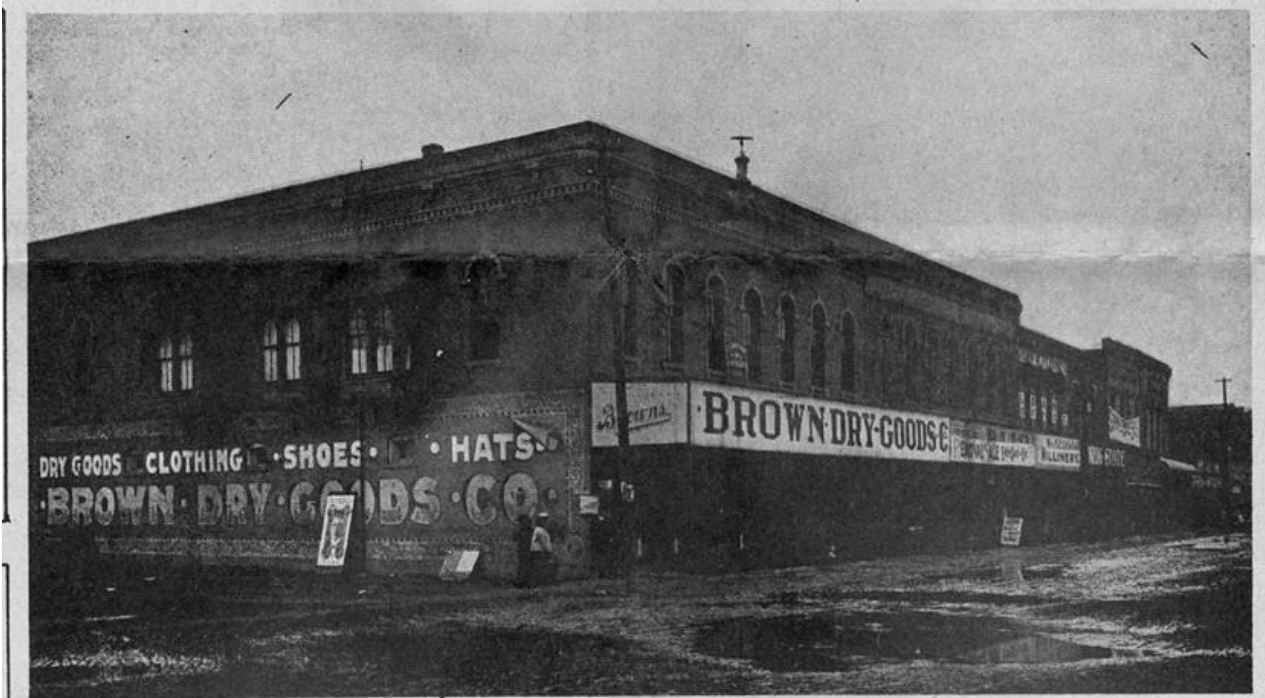
South Side of Public Square at Turn of Century
