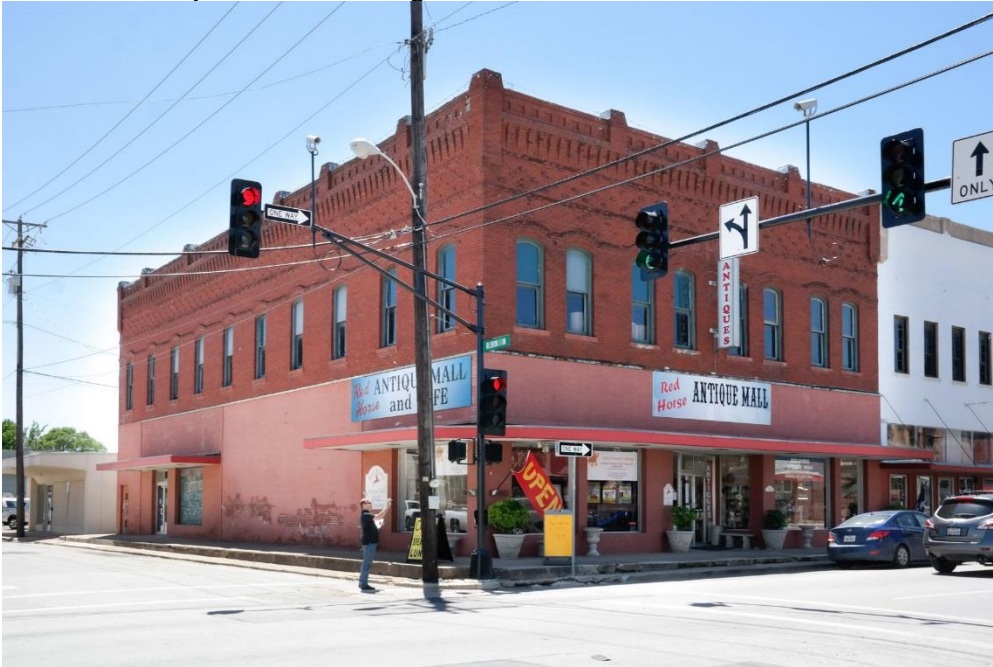
Photo 33 Building at 216 E. Henderson Street (Property #72) Northeast oblique, camera facing southwest
