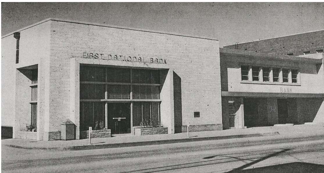
Figure 17: 109 N Main Street, First National Bank.
