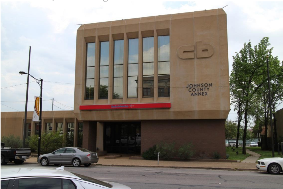
Photo 48 Building at 1 N. Main Street (Property #84) – Noncontributing / Outside Period of Significance East elevation, camera facing west
