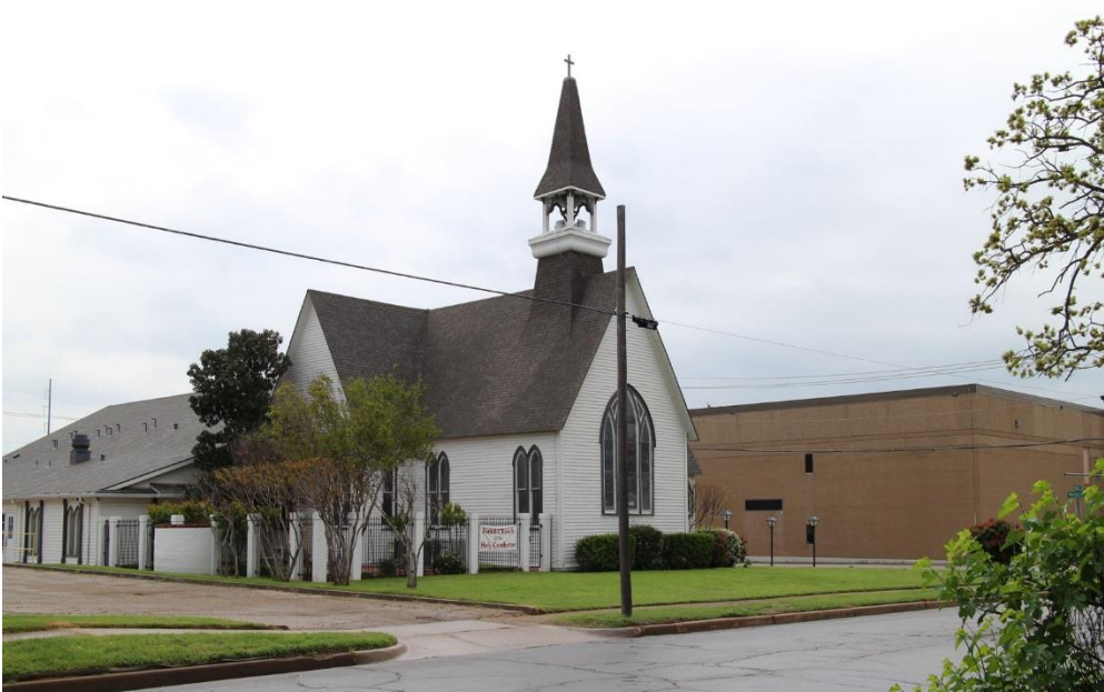
Photo 46 Building at 209 E. Wardville Street (Property #124) Northwest oblique, camera facing southeast
