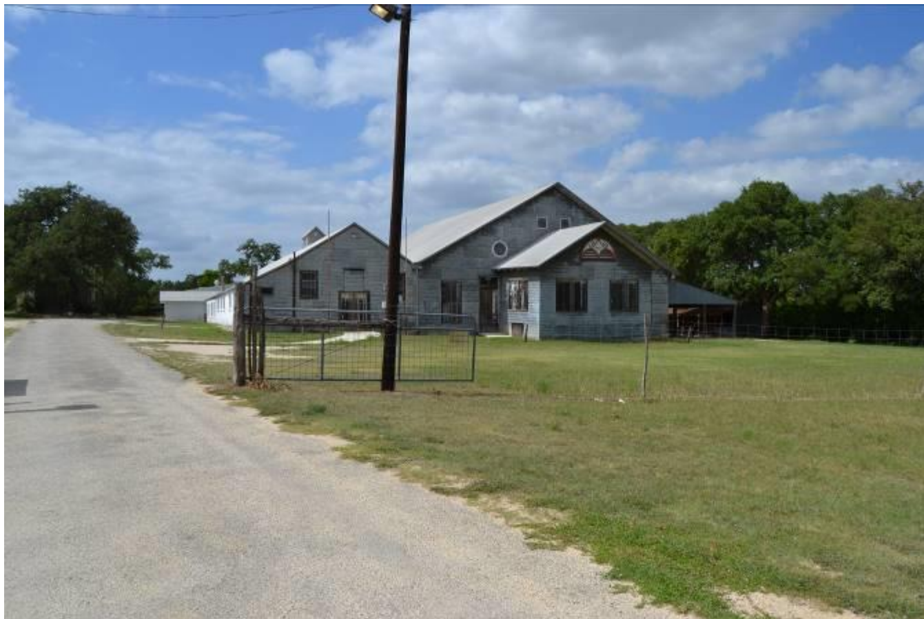
Photo No. 2. Contextual view of drive coming in from southeast and running along west side of Anhalt Hall, view facing northeast.
