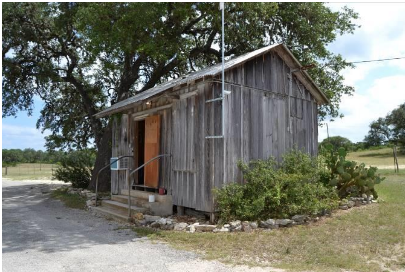
Photo No. 30. View of outhouse (Resource d), view facing southwest.
