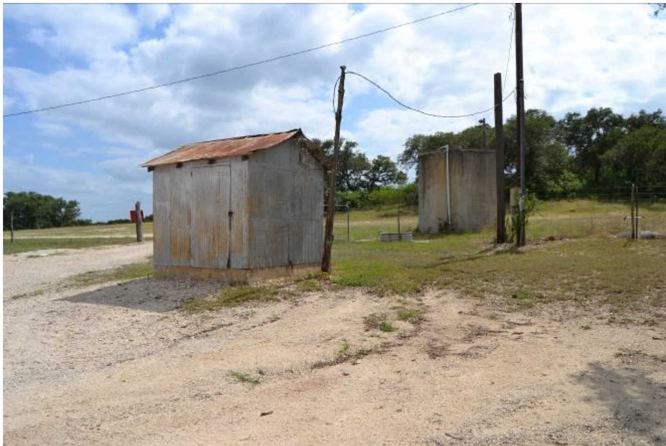
Photo No. 32. View of well house (Resource f) and cistern (Resource c), view facing west.
