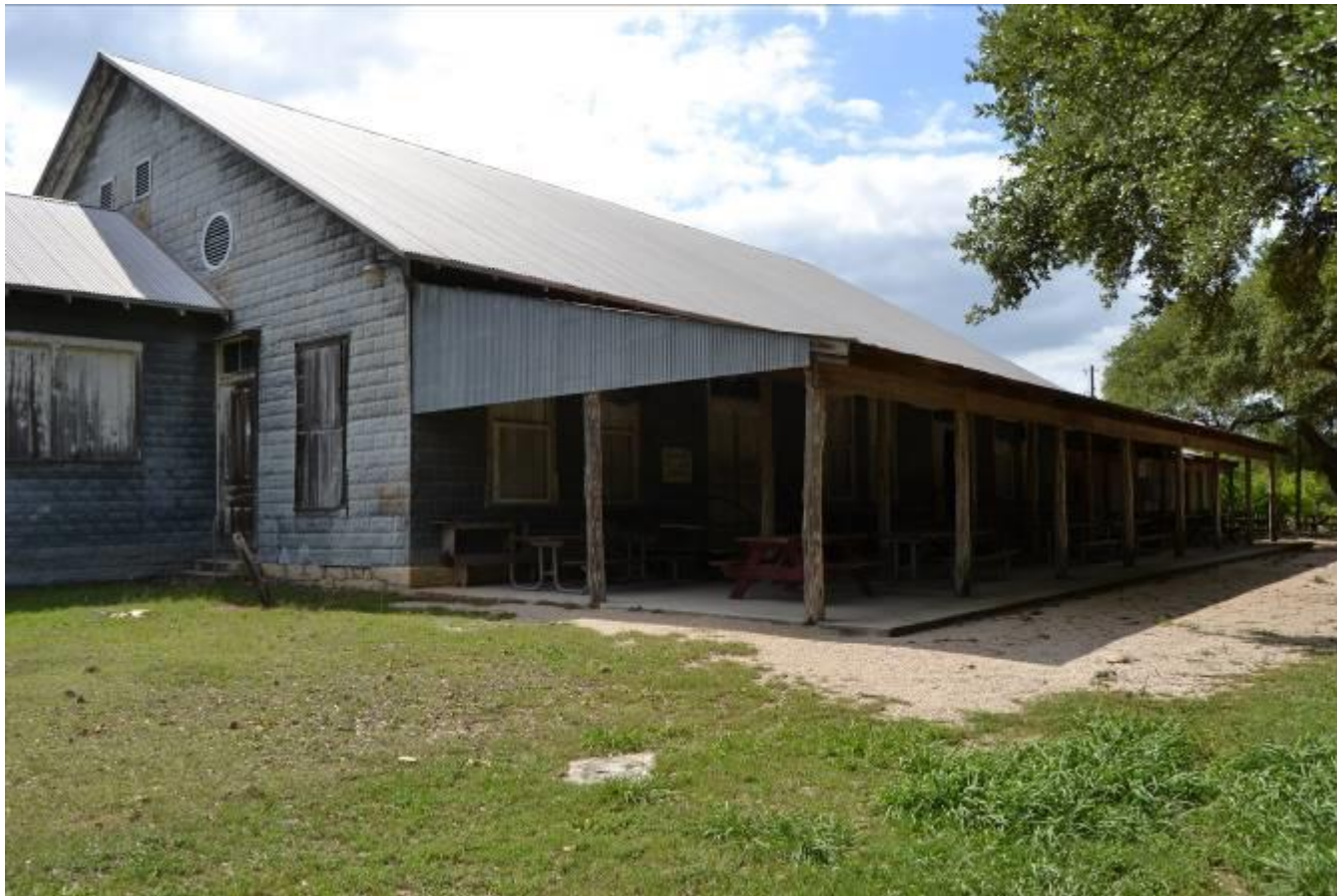
Photo No. 8. Oblique view of side east façade of Anhalt Hall, view facing northwest.
