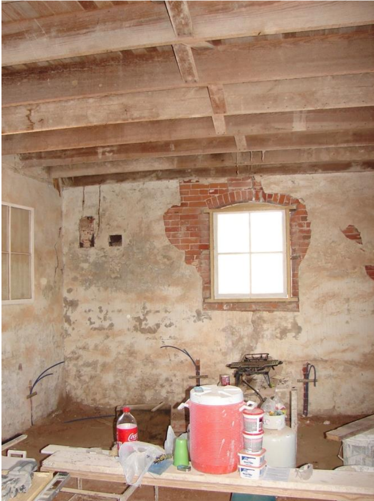
Figure 6: Segmental Arch Window Opening in Resource A Source: San Antonio Conservation Society
