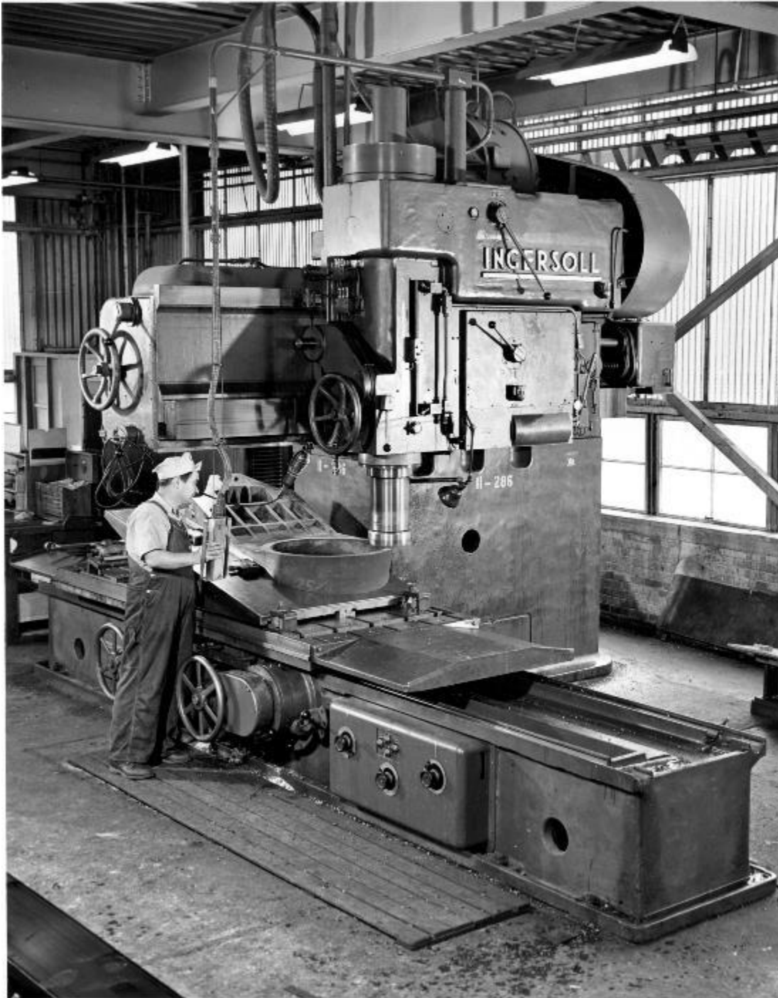
Figure 9: Photo of Building #11 interior during manufacturing. Steel interior structure, concrete floor, brick and corrugated glass exterior visible, c. 1956. Courtesy University of Missouri, St. Louis – St. Louis Mercantile Library
