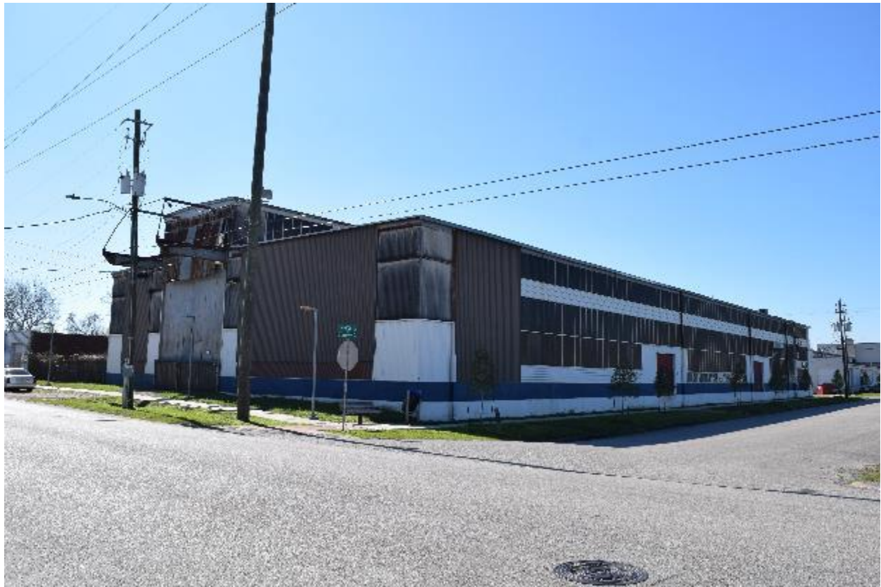
Photo 25 – North (rear) and west elevations of Building #21, view southeast, February 2017.
