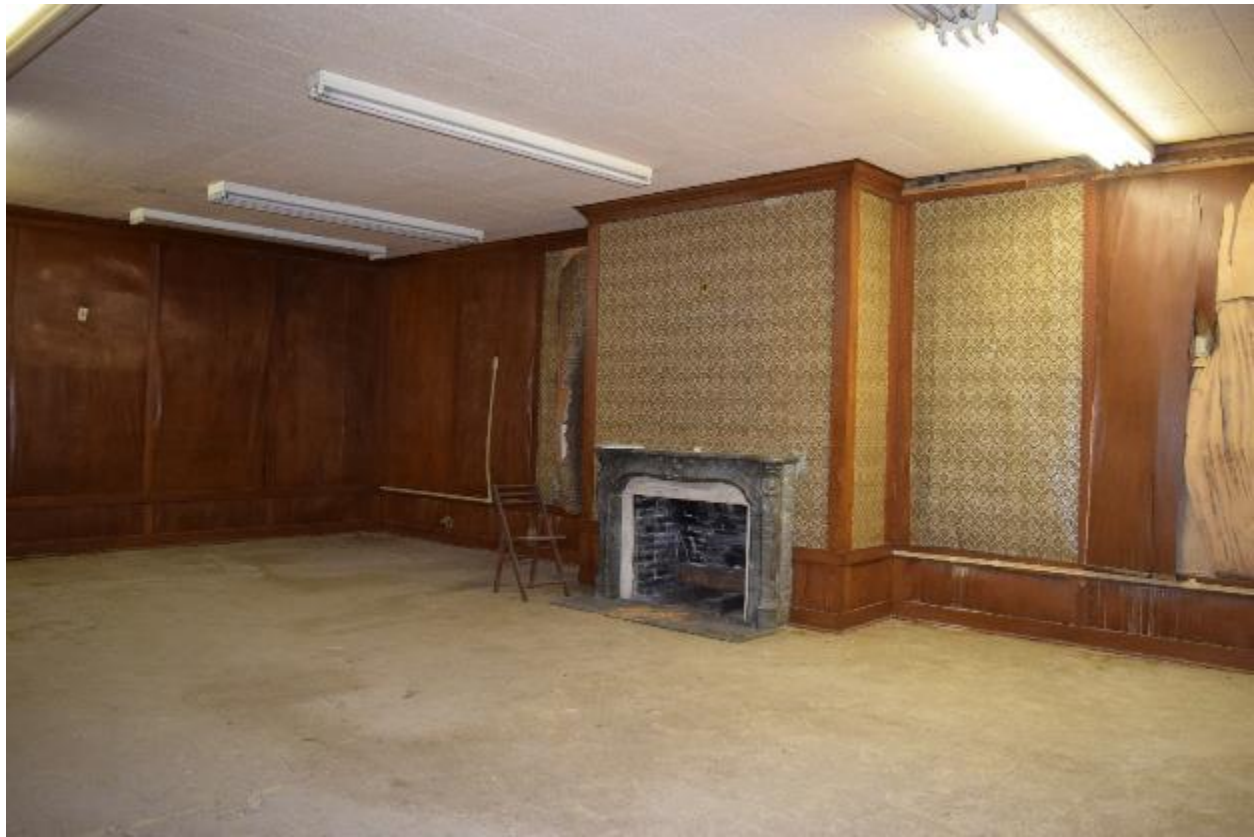
Photo 18 – Second floor conference room in Building #13 showing original ceiling, fireplace, and wood paneling, view south, February 2017.
