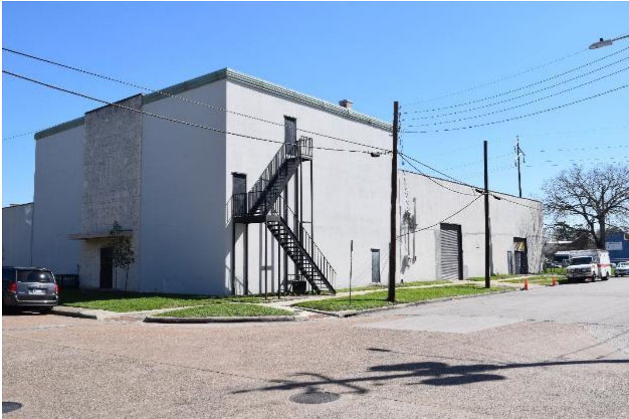
Photo 16 – West (front) and south elevations of Building #13 (left), view northeast, February 2017. South elevations for Buildings #15 and #19 are visible on right.
