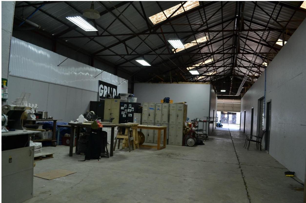
Photo 24 – Interior of Building #18, view north, June 2017. Building #18’s structural independence from Building #20 is visible on left.
