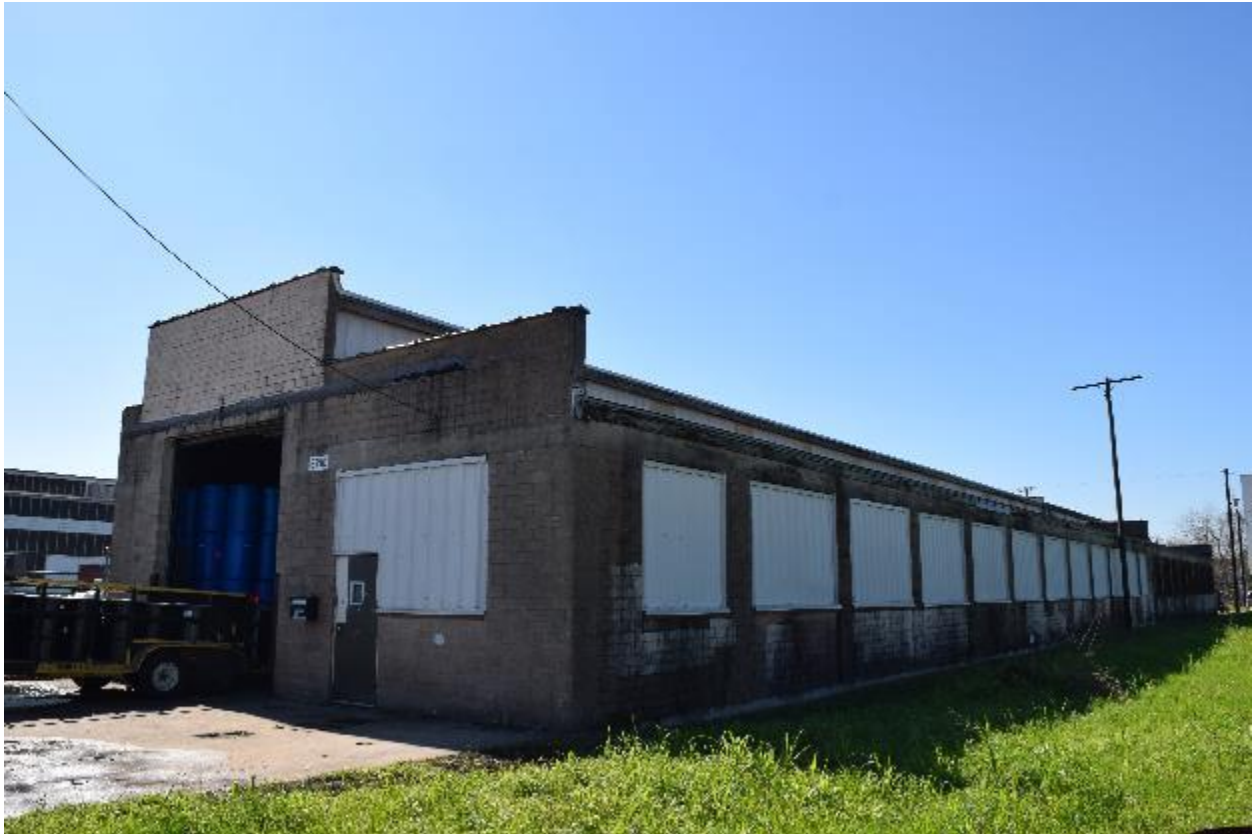
Photo 8 –North (rear) and west elevations of Building #9, view southeast, February 2017.
