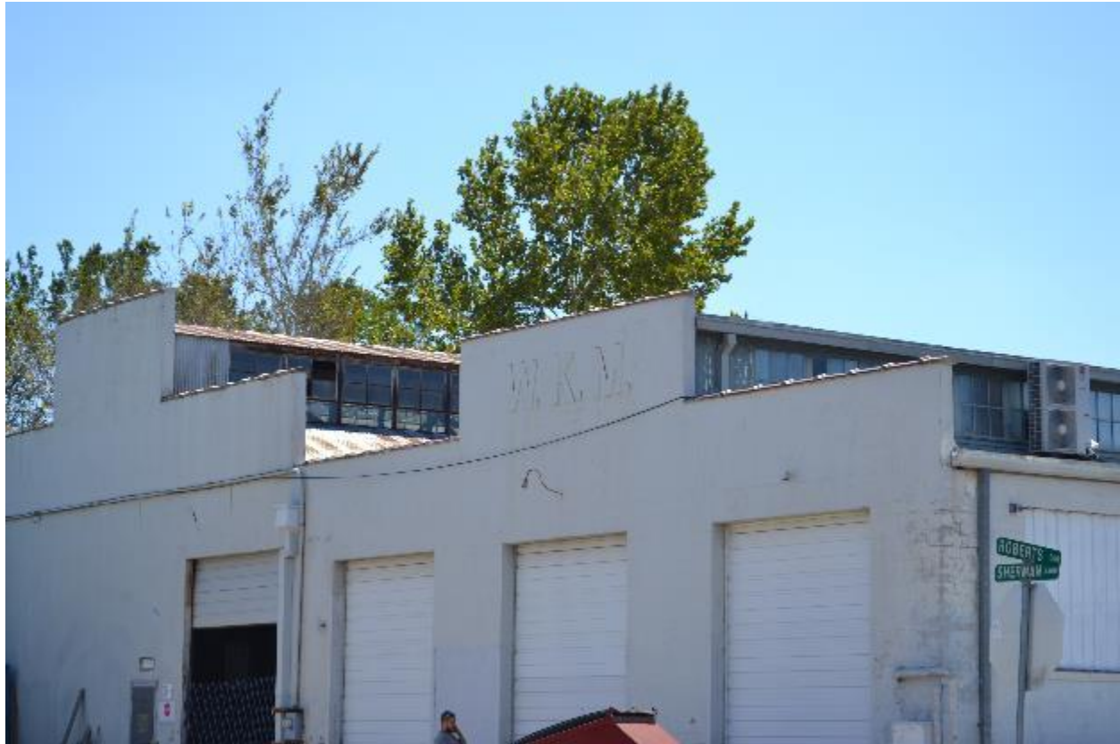
Photo 11 – Detail of remaining W-K-M signage on the north elevation of Building #10, view southeast, September 2017
