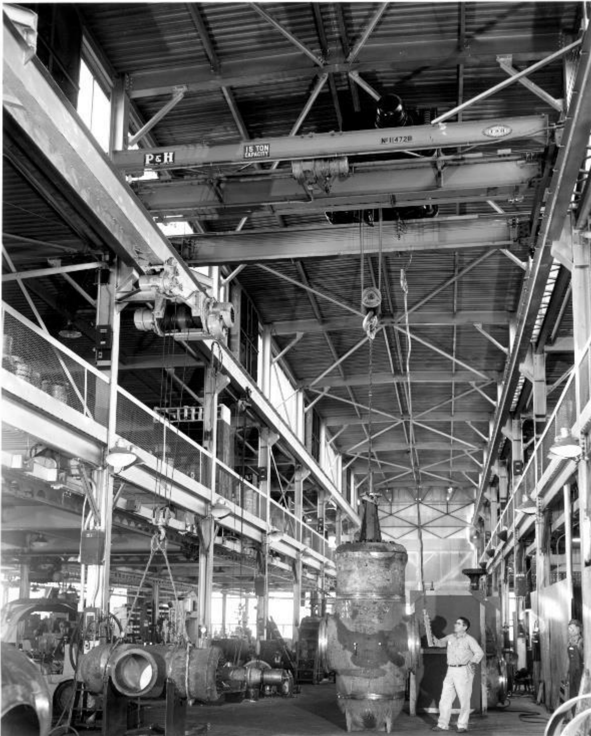
Figure 10: Photo of Building #11 interior during the production of a gate valve. Steel interior structure, double-height manufacturing space, and clerestory windows visible, c. 1956.
