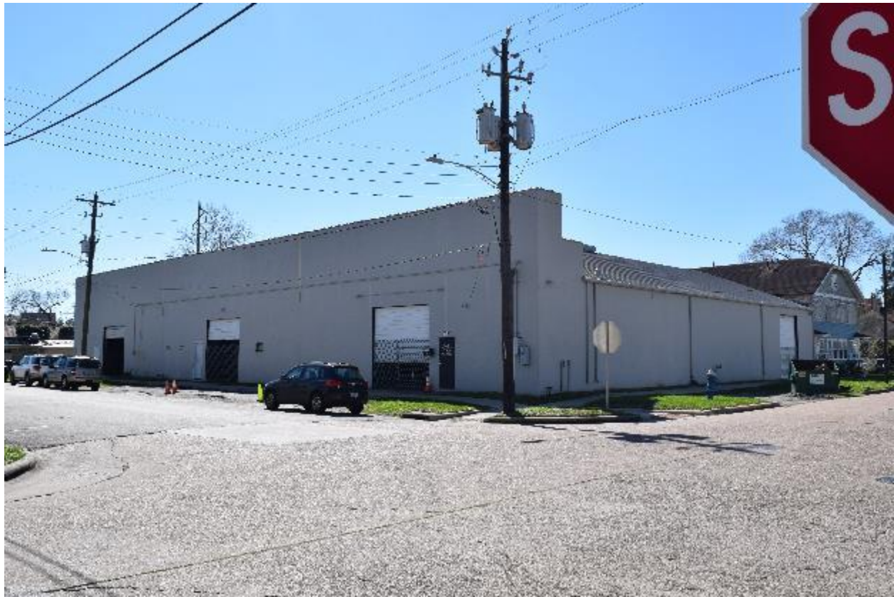
Photo 23 – North elevation of Building #18 (far left) and north and west elevations of Building #20, view southeast, February 2017.
