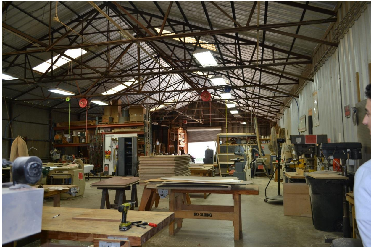
Photo 20 – Building #19, view south, October 2017. Party wall between Building #19 and Building #15 is visible on the right.
