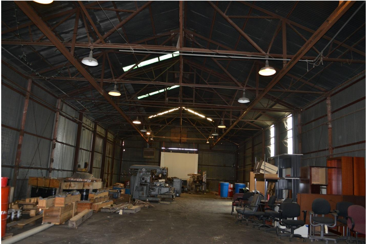
Photo 22 – Interior of Building #17, view north, June 2017.
