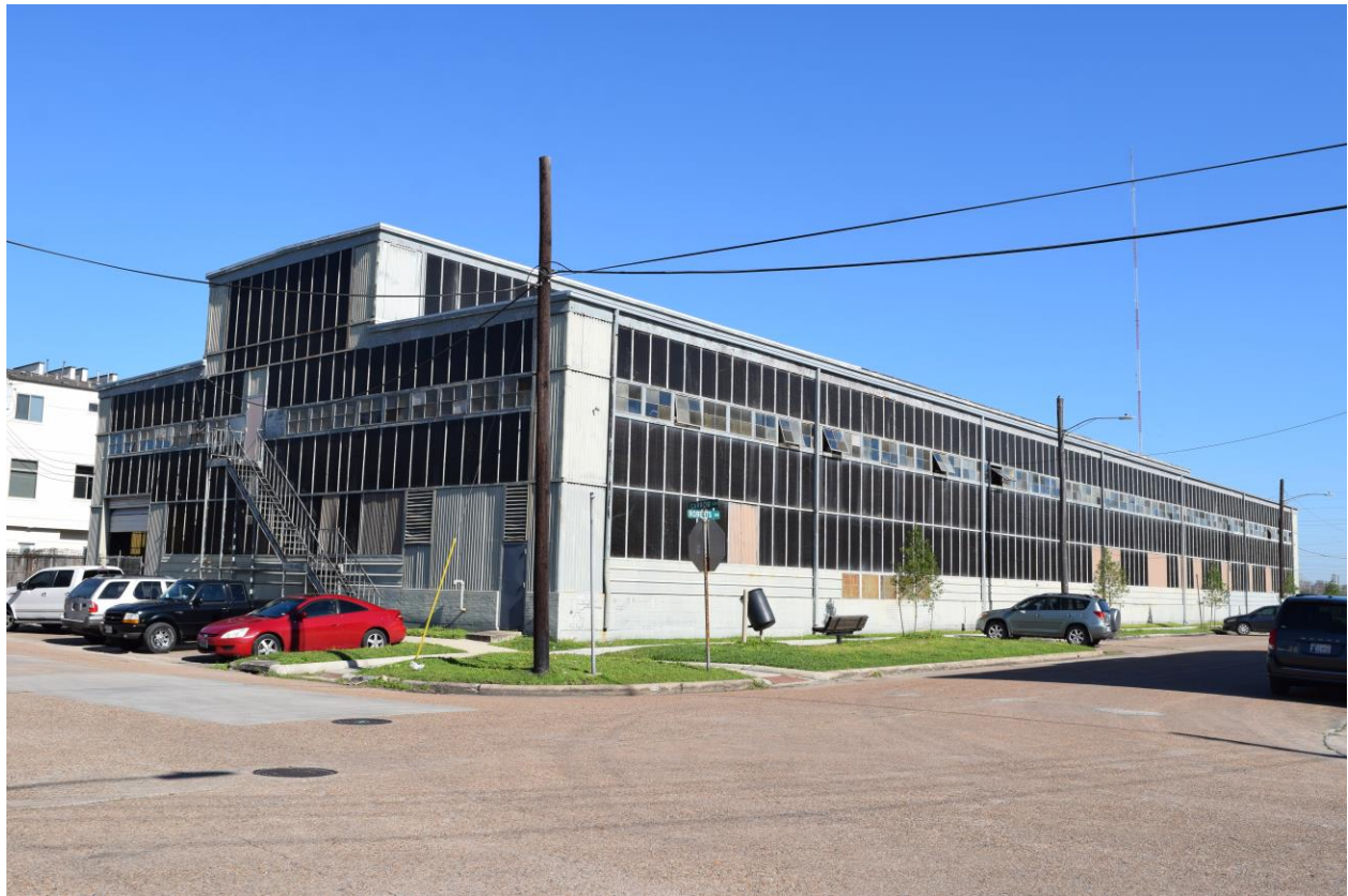
Photo 14 – South (rear) and east elevations of Building #11, view northwest, February 2017.
