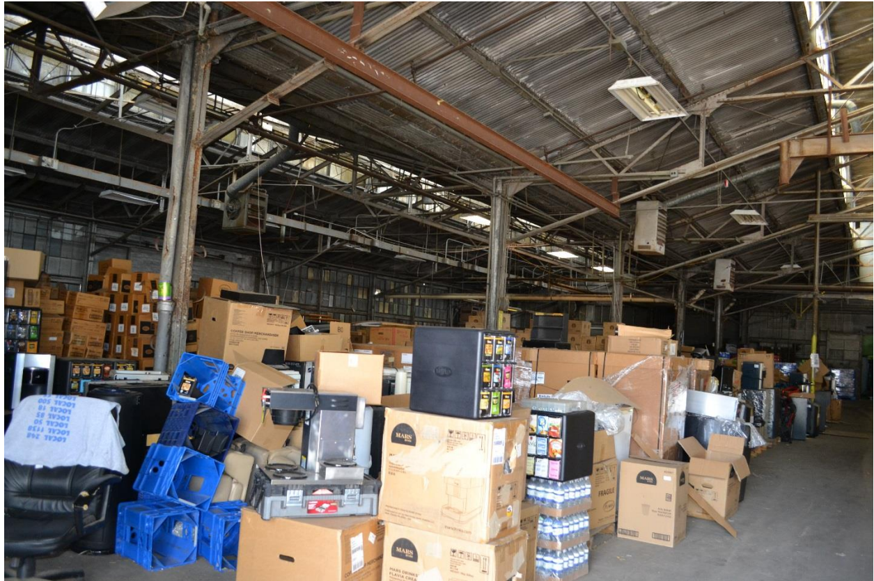
Photo 6 – Building #6, interior view southeast, June 2017.
